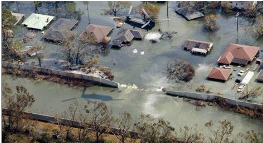
Figure 3.189 Tilting of walls in composite levee due to differential settlements (courtesy Y Deniaud, CETMEF)
