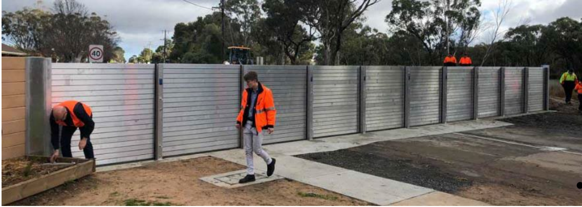
Type 1 Temporary Levee
