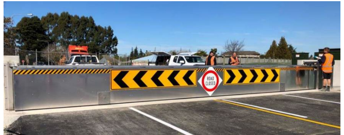
Type 2 Temporary Levee
