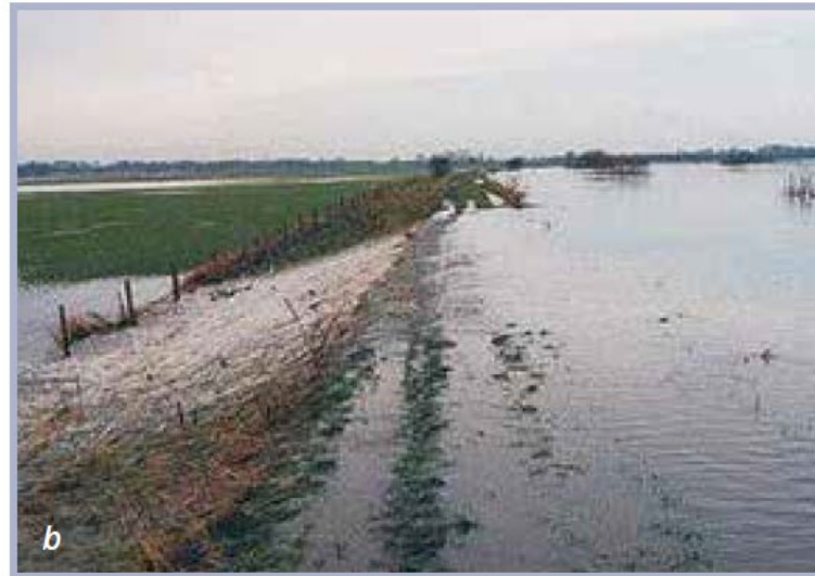
Figure 3.170 External erosion of the landward side of a levee due to overflowing (courtesy Y Deniaud, CETMEF)
