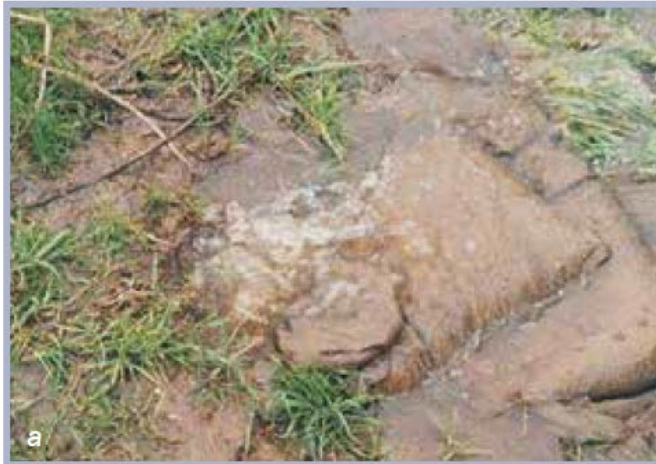
Figure 3.158 Seepage (a) and major release of water in leveed area (b) (courtesy Defra) Images source: International Levee Handbook (CIRIA, 2013)
