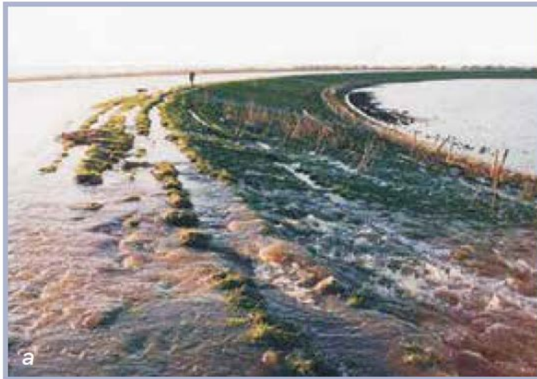
Figure 3.156 Localised overtopping (a) and overflowing (b) (courtesy Defra)
