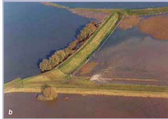
Figure 3.158 Seepage (a) and major release of water in leveed area (b) (courtesy Defra) Images source: International Levee Handbook (CIRIA, 2013)
