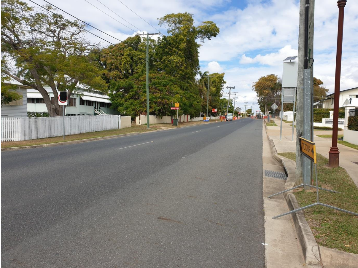
Photograph 5: Looking south from the Ferguson Street intersection, once again showing consistent spacing of point hazards on the left (eastern) side. This is the release point for southbound vehicles leaving the St Peter's school zone (the 60km/h sign is covered in the photograph). The northbound lane of Upper Dawson Road is currently closed for roadworks, which will include the marking of edge lines through to Brecknell Street.
