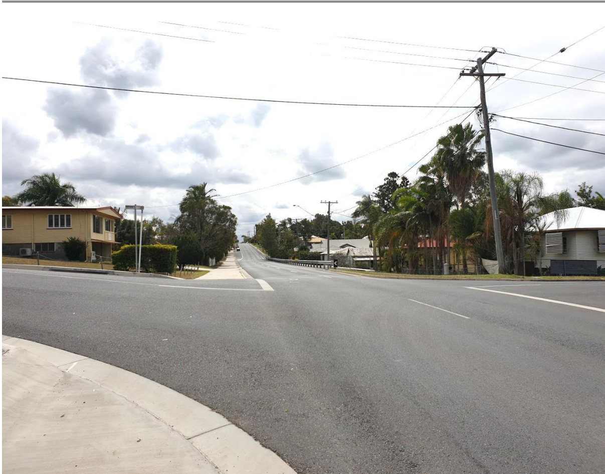
Photograph 2: Looking north from the Nathan Street intersection. There is 50m of steel guard rail running along the right (eastern) side of the carriageway to provide protection from the drop-off to the Upper Dawson Rd Service Road. From this point, the carriageway width increases and edge lines are marked from MacGregor Street. The crest at King Street can be seen in the distance.
