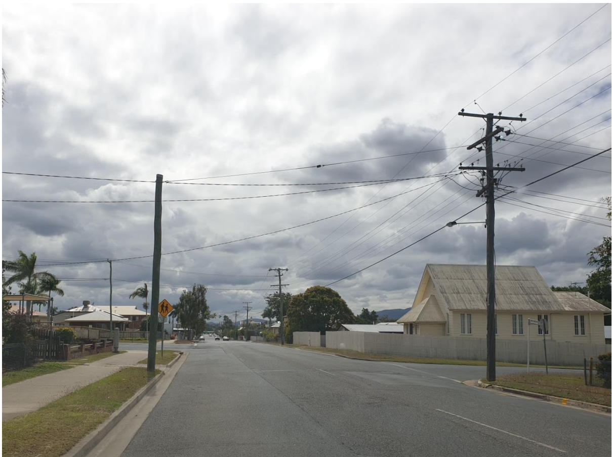
Photograph 9: Looking north, showing the Church Street intersection. Edge lines are not marked in this section, but the carriageway is still wide enough to accommodate a 3.3-3.5m lane with a \geq 2.0\text{m} parking lane on each side.
