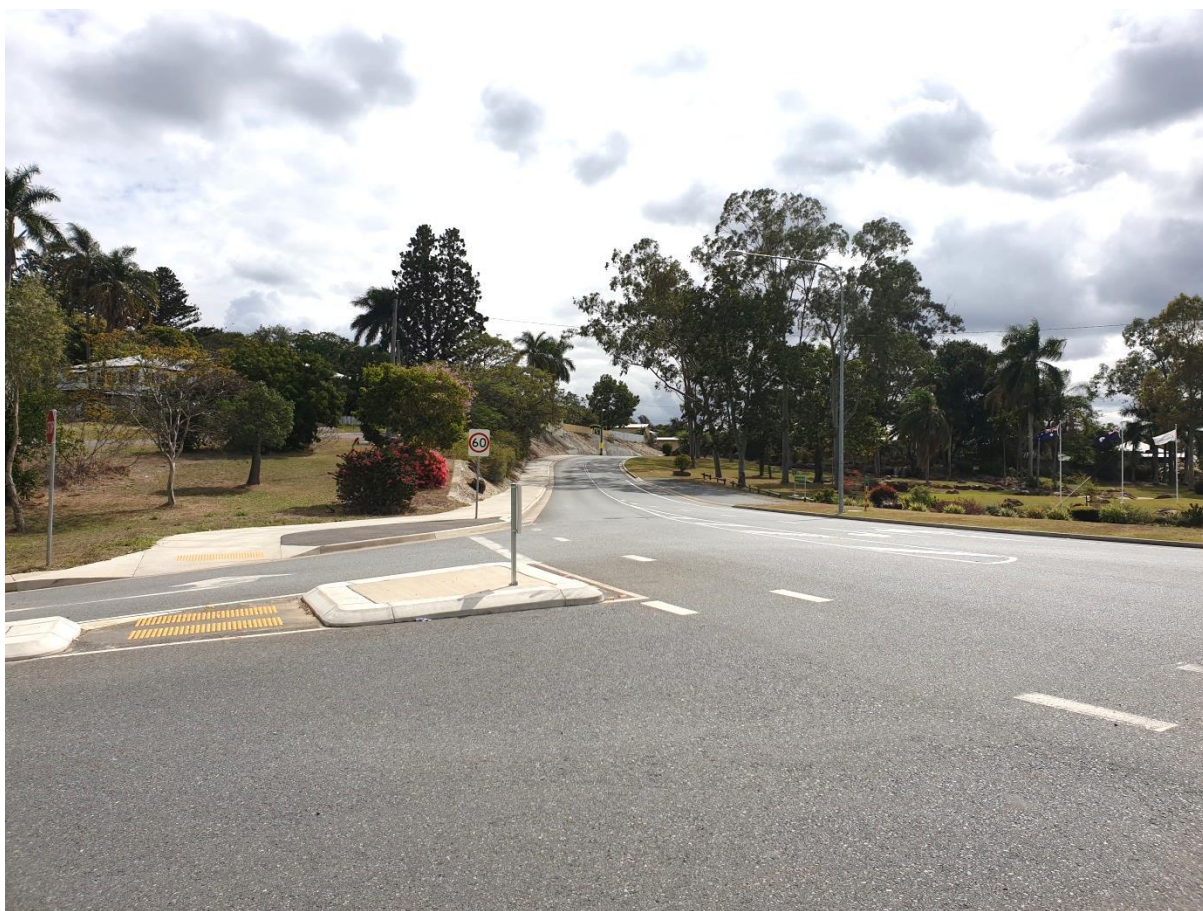
Photograph 1: Start of the speed zone, looking north along Upper Dawson Road from Blackall Street. Here, the carriageway width has been restricted to remove shoulders and allow width for a shared footpath.
