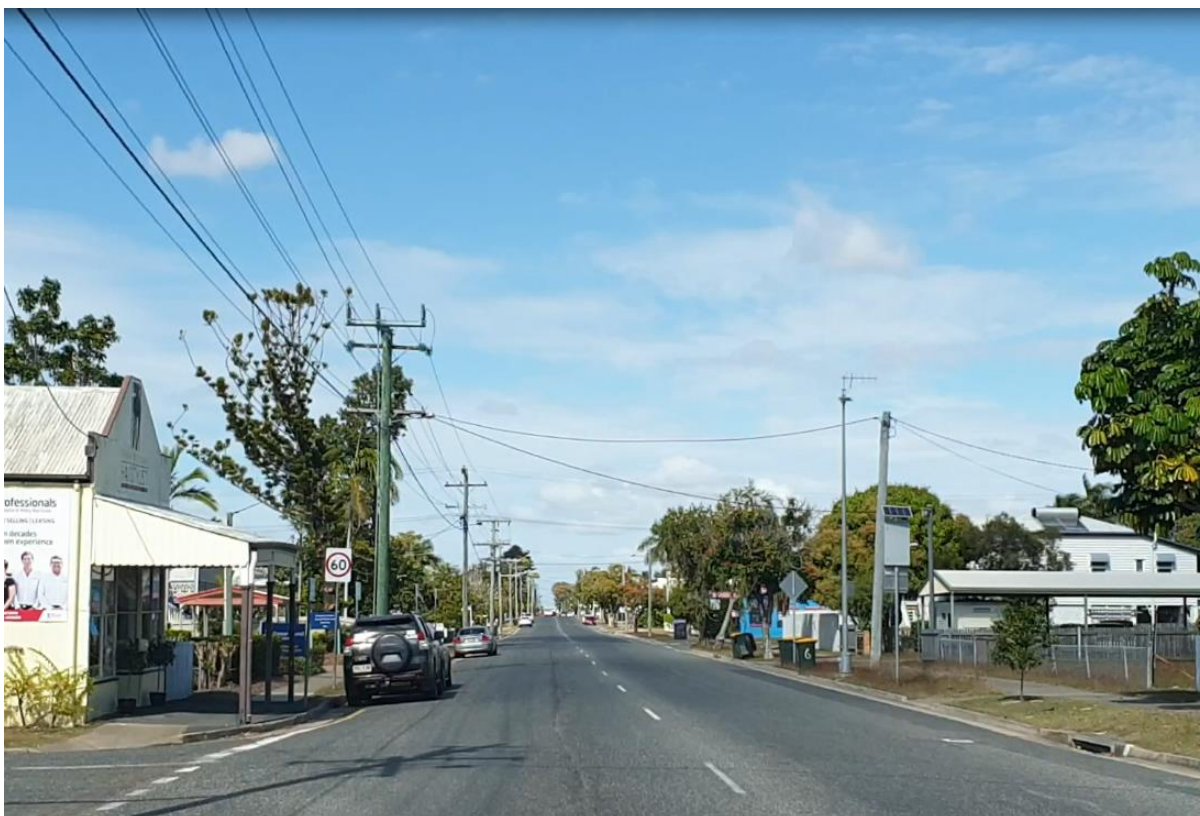
Photograph 11: Looking south, at the Margaret Street intersection. This is the northern end of the speed zone. Note the close spacing of point hazards on the right (western) side.
