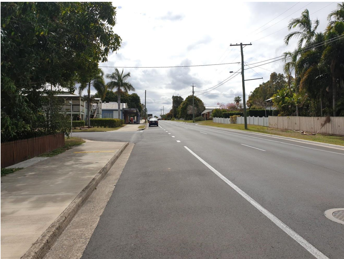
Photograph 4: Looking north towards Lamington Street, a consistent spacing of power poles can be seen on the right (eastern) side, while point hazards are sporadic on the left (western) side. The edge lines have been marked at \geq 2.0\text{m} to accommodate car parking in the shoulders.
