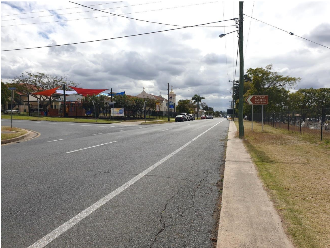
Photograph 7: Looking north, showing the Spencer Street intersection. Note the presence of parked cars along the school frontage, and the irregular placement of point hazards on the left (western) side with long spacings between.
