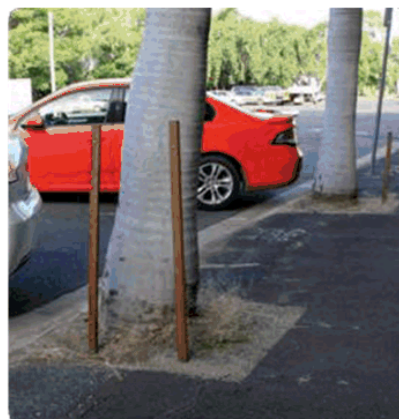
An inappropriate interface between footpath and tree trunk.
