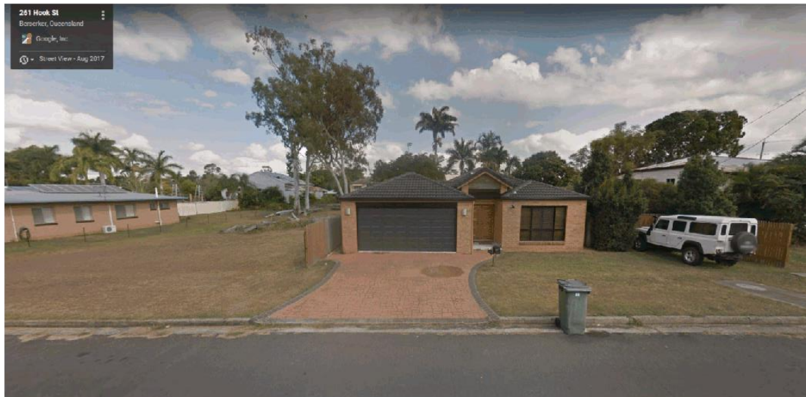
Figure 1: Photograph of the property located at 261 Hook Street, Berserker. The house is slab on ground, with a finished floor level of 19.21m AHD (at the door). Ground elevation ranges from 18.8m AHD to 19.25m AHD.
