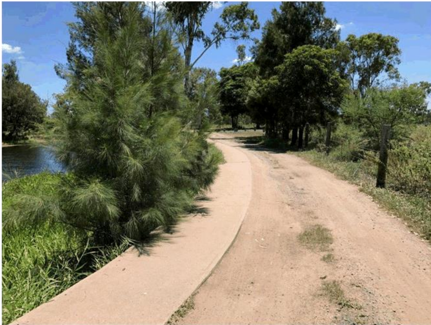
Figure 4. Erosion of northern creek bank (note undermined path >300mm)
