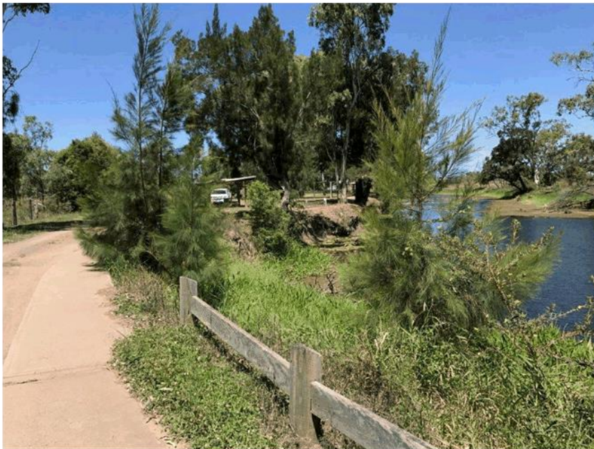
Figure 5. Erosion of northern creek bank (note missing bollards and proximity to pathway)
