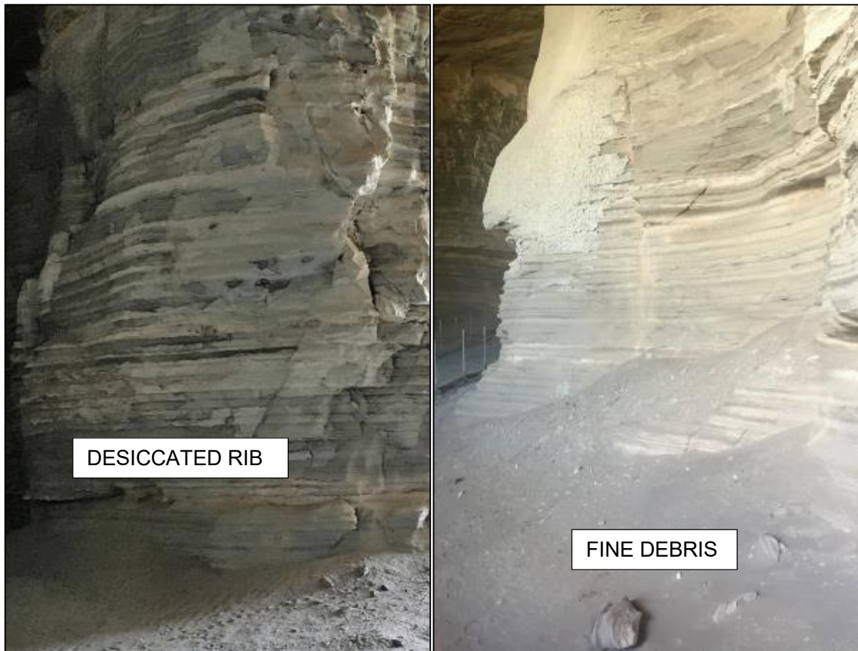
Figure 4-3 Erosive Processes on Siltstone Ribs.
