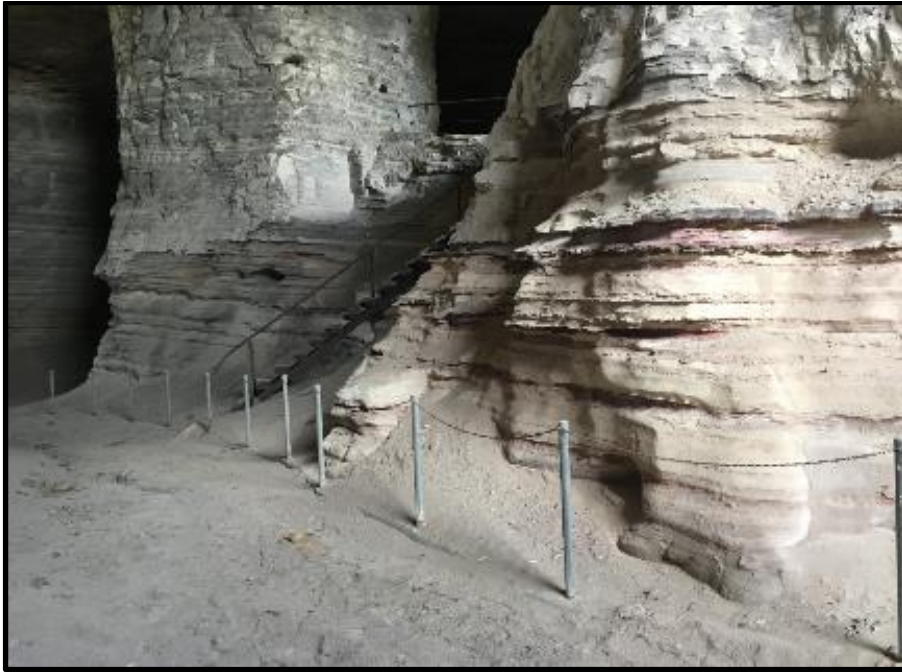
Figure 4-4 Wind Erosion of Siltstone Ribs at the Base of Pillar G.
