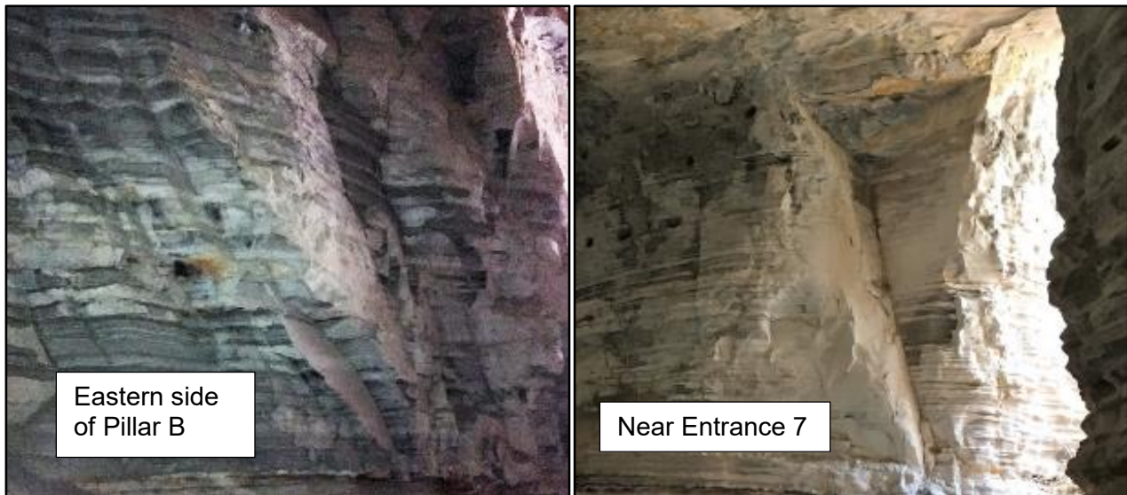
Figure 4-7 Joint Controlled Failures of Siltstone Ribs.
