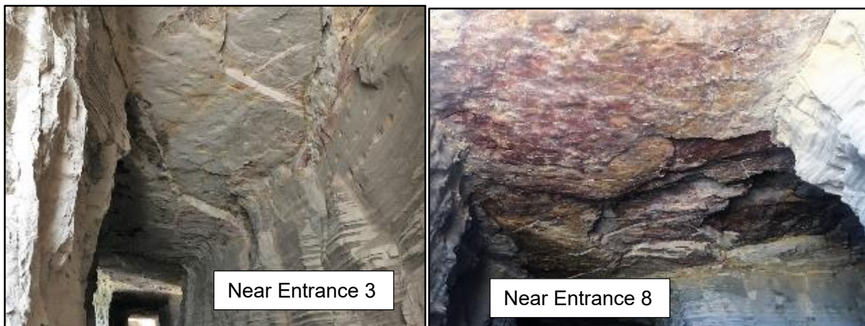
Figure 4-8 Joint Controlled Failure of Sandstone Roof.
