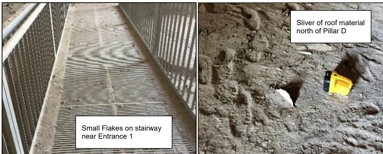
Figure 4-9 Flaking of Small Sized Roof Material.
