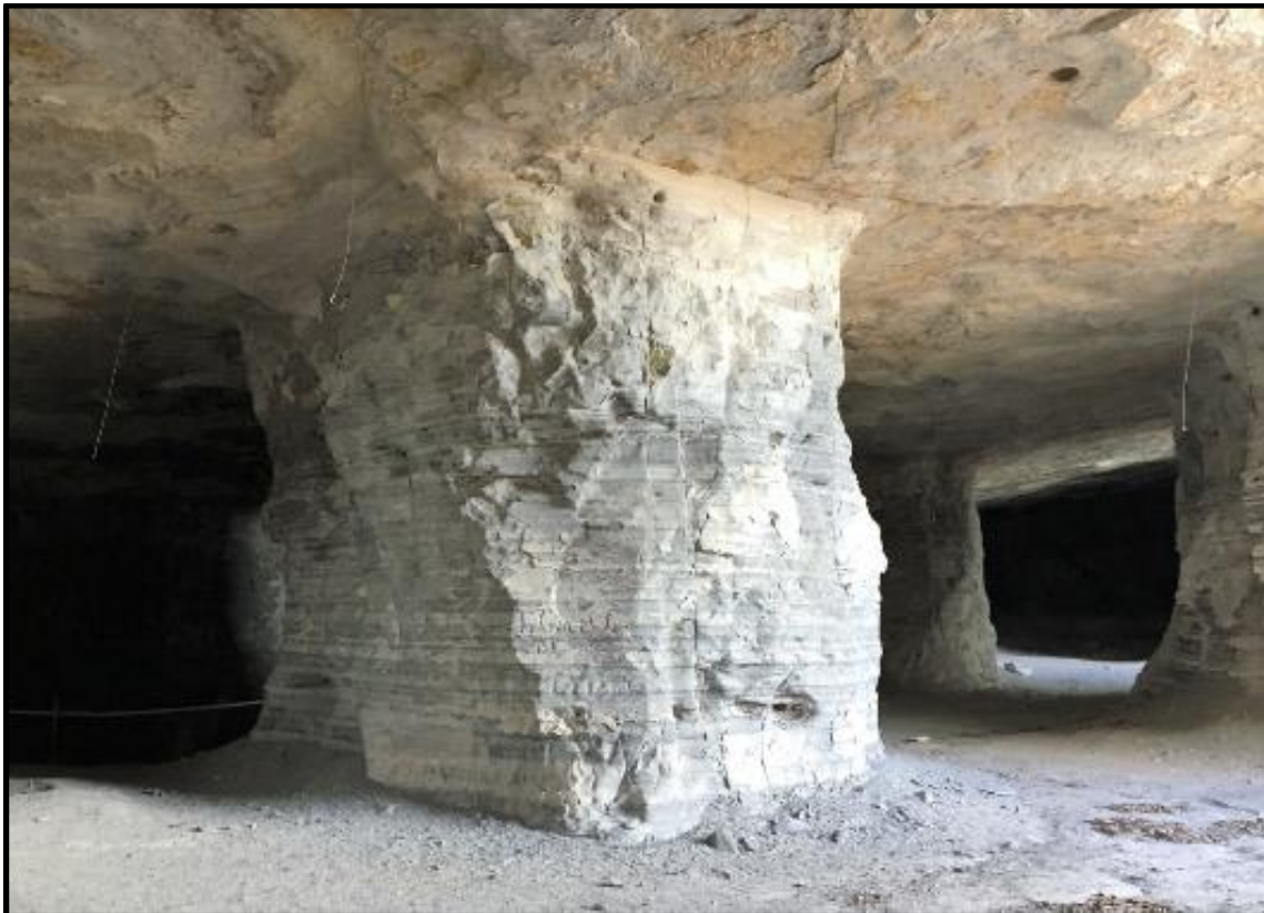
Figure 4-32 Installed Convergence Pins and Wires Hanging from the Roof near Pillar H.
