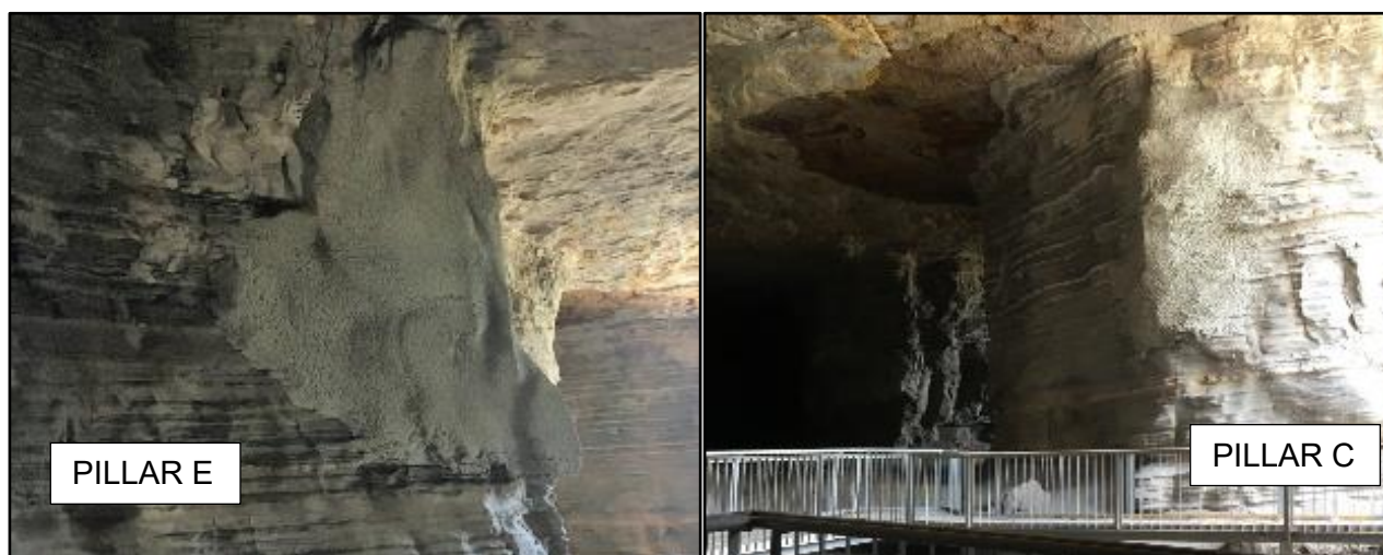
Figure 4-2 Shotcreting of Corners near Entrance 1.
