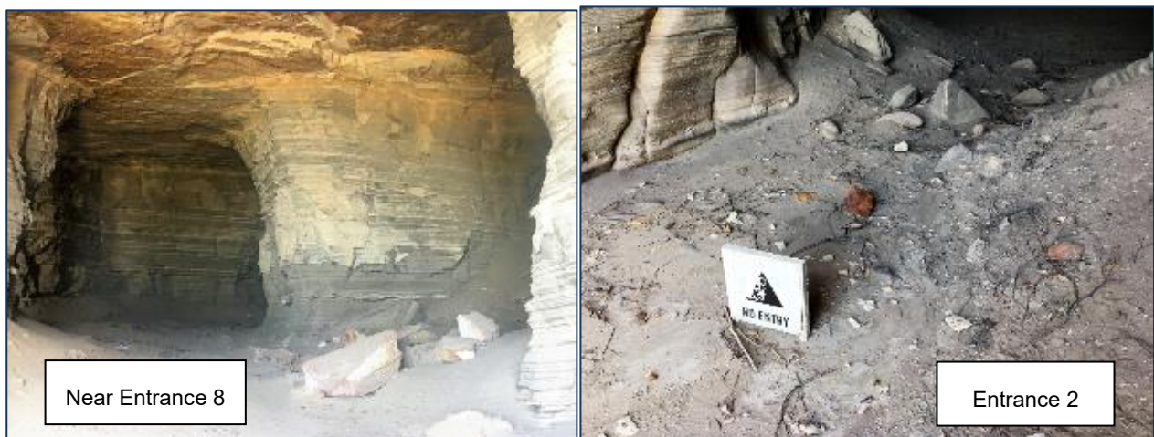
Figure 4-10 Existing Roof Fall Areas – February 2019.
