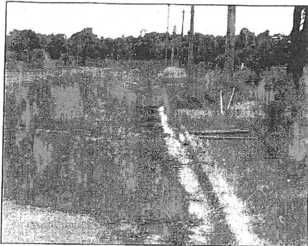
3. Existing kerb and channel ponding water
