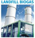
The Landfill Biogas system works by extracting greenhouse gases, such as methane, which are produced when organic matter in the landfill breaks down.
