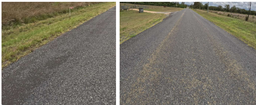
Figure A.2.5 Ravelling / Stripping on a spray sealed road
