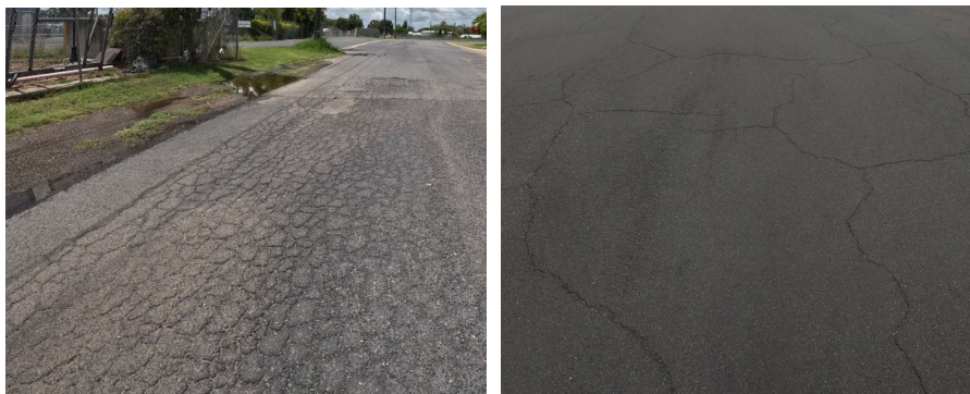
Figure A.2.3 Structural Cracking and Environmental Cracking (L – R)
