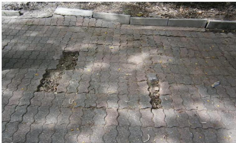
Uneven and missing pavers in the driveway a trip hazard.
