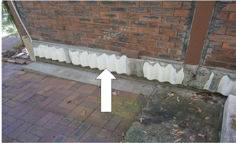
Super six Asbestos along the concrete slab edge.
