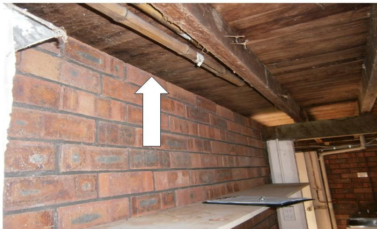
No support at the top of the brick walls.
