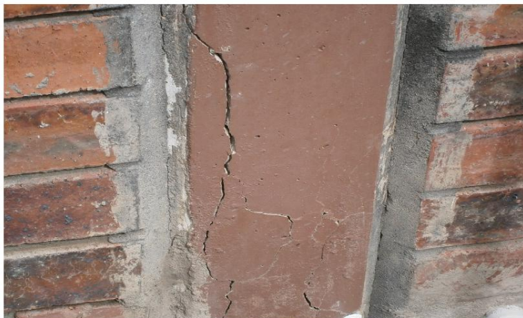
Concrete post breaking apart.
