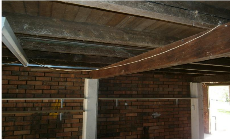
Phone cable not secured.
