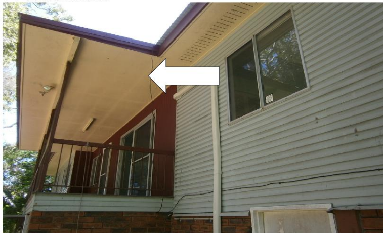
T V Cable not secured.
