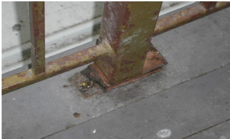
Foot plate rusted on the western side verandah post
