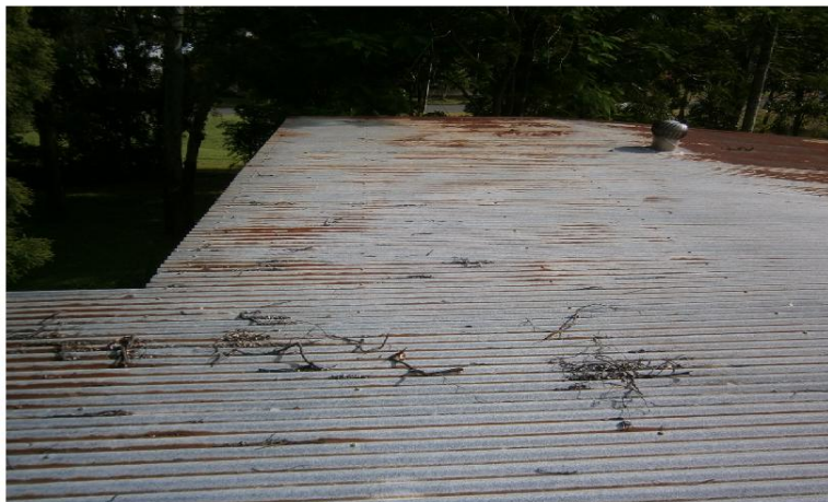
Rusted roofing iron .
