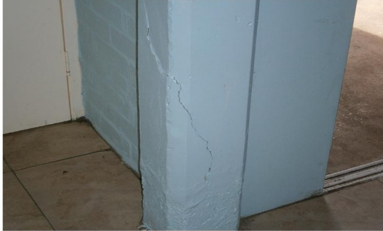
Concrete posts breaking apart.
