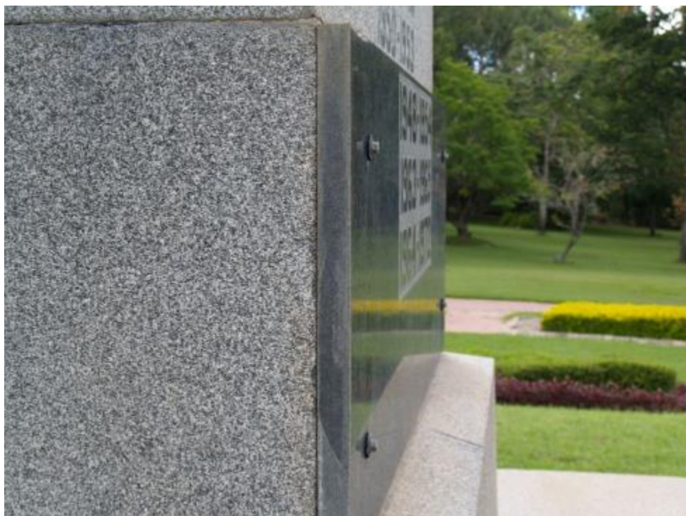
Fig. 5 Black granite slab bolted onto Western face.
