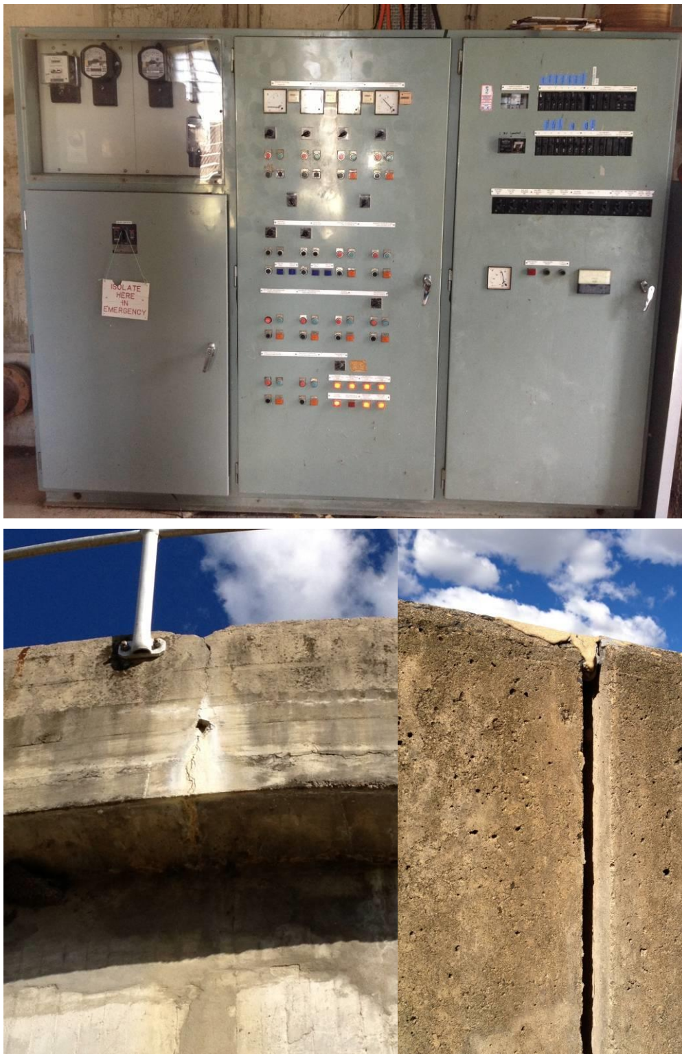
Figure 1. Photographs showing the ageing electrical switchboard (top) and the commencement of structural failure in the clarigester (bottom left) and trickling filter tank (bottom right).
