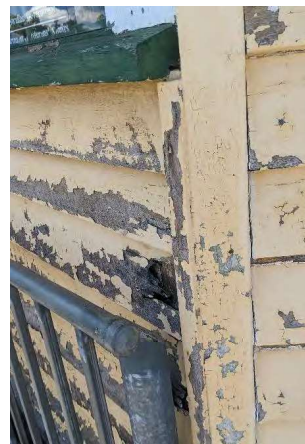
Figure 24: Damage to paint and weatherboards of northern elevation (AHS 2023).
