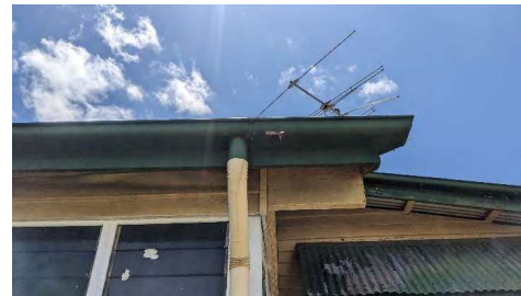
Figure 22: Rust damage to gutter of the western elevation (AHS 2023).
