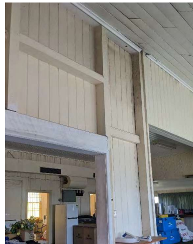
Figure 33: Infilled section of early door (AHS 2023).
