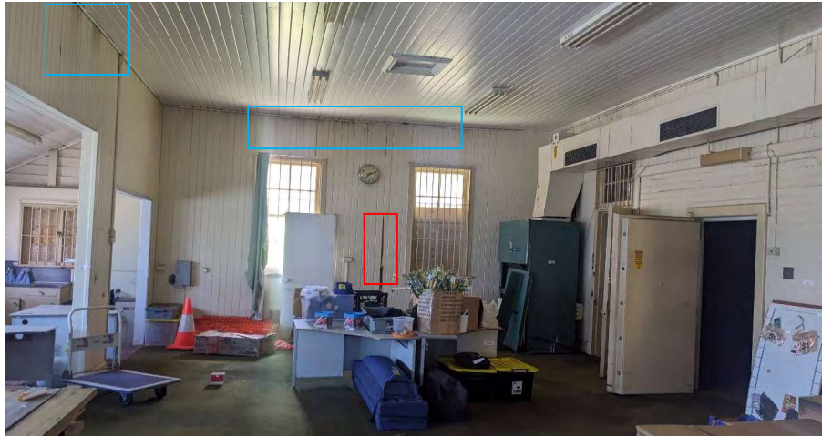
Figure 28: Main Office Area showing eastern and southern walls and the presence of damage from water ingress [Blue] and insect activity [Red] (AHS 2023).
