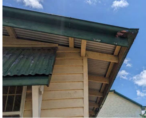
Figure 21: Rust damage to gutter of the western elevation (AHS 2023).
