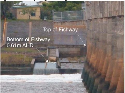
The EarthTech report obtained a model output from CSIRO providing a time-level duration curve for the tidal level at the Fitzroy Barrage, see Figure 2. EarthTech calculated the percentage of time that the tidal level on the estuary side of the barrage was above 0.61 m, i.e. when the fish could access the fishway, as 32.8% of the time, or on average approximately eight hours per day.
