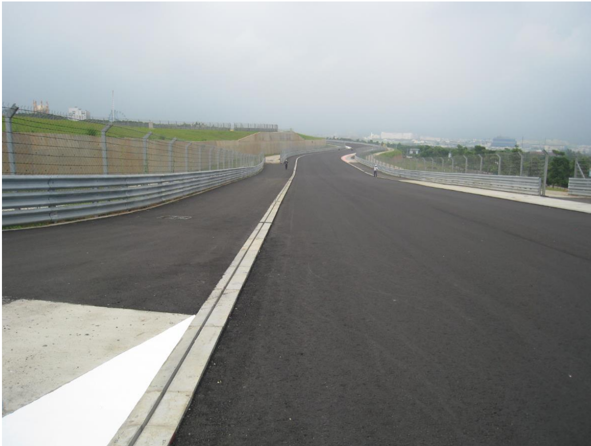
Figure 37 Slot drainage integrated into track edge (mid construction)
