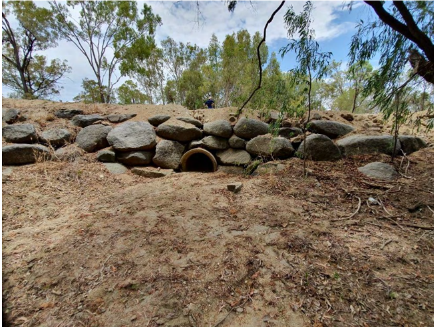
Figure 26 Quarry Access Road, Four Mile Creek Culvert
