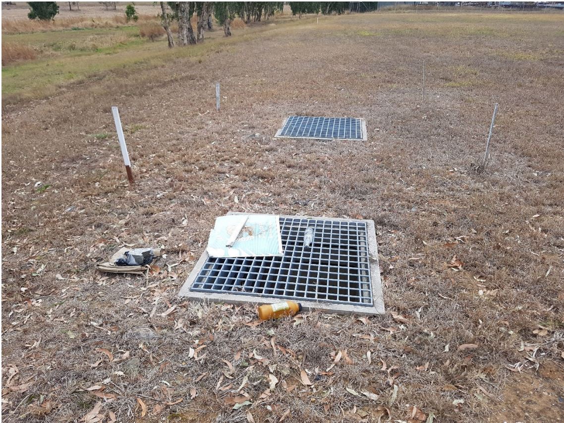
Photograph 3 – Existing field inlet pits at rear of site
