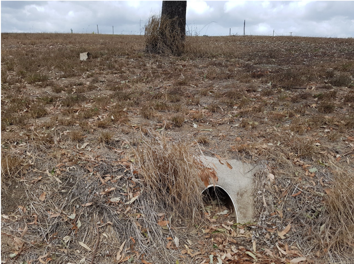
Photograph 4 – Outlet from existing field inlets to Splitters Creek
