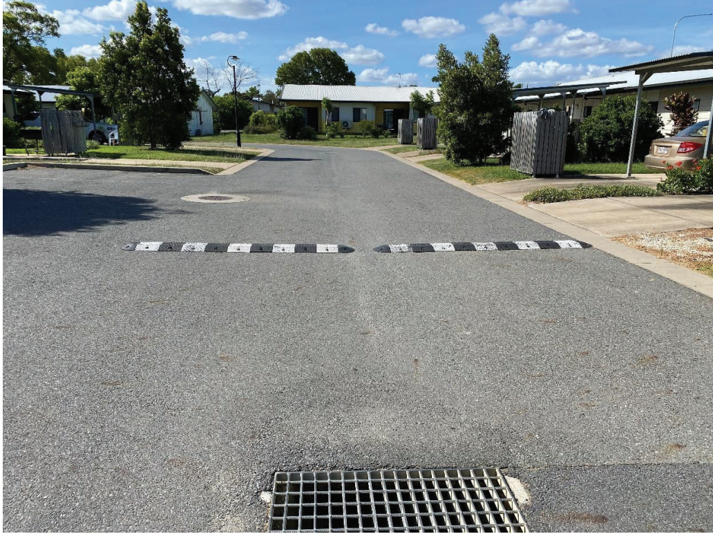
Road profile of access road inside Proposed Lot 1, looking east
