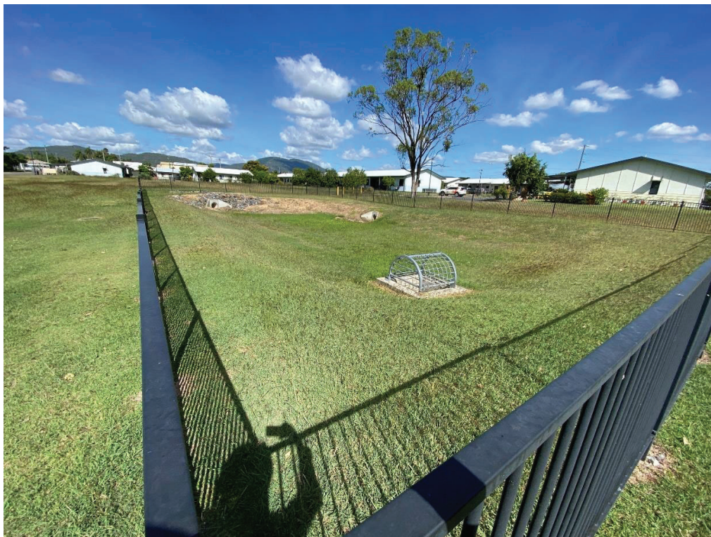
Existing stormwater basin located in Proposed Lot 3
