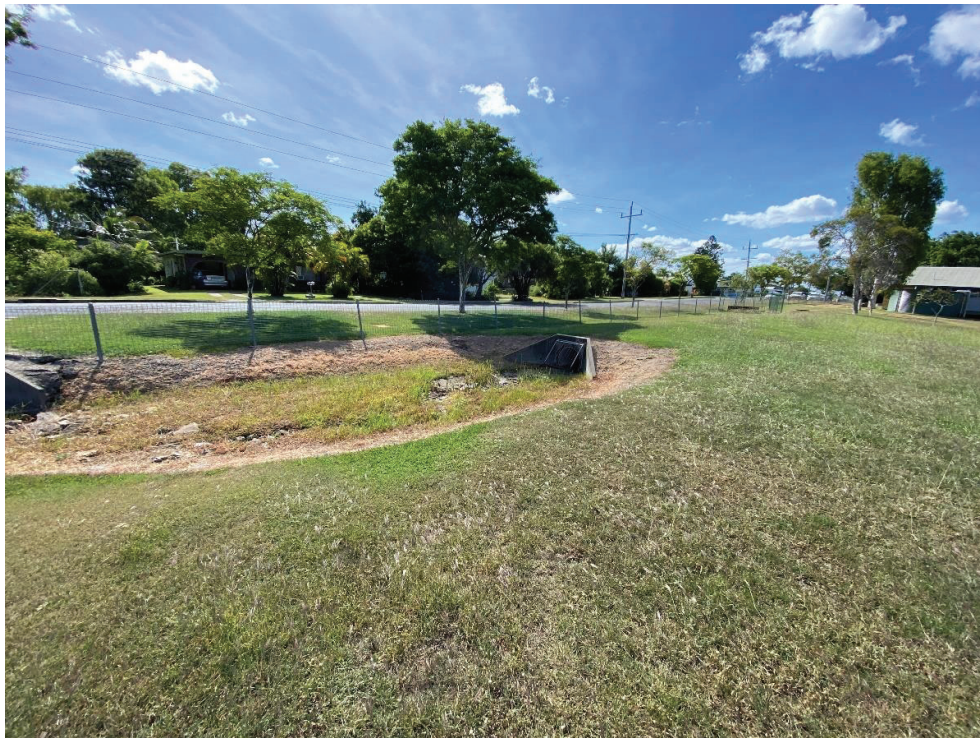
Age care facility drainage outlet. The headwall in the centre of the photo discharges to the headwall on the left-hand side of the photo (these stormwater flows bypass the stormwater basin)
