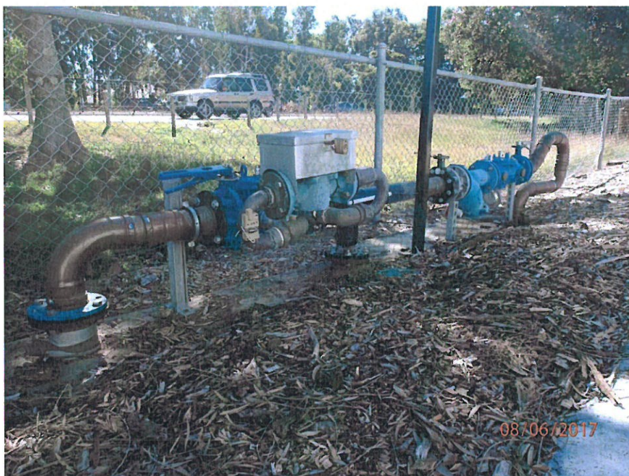
Figure 1: Water Meter Assembly immediately to the north of the existing Cinema building
