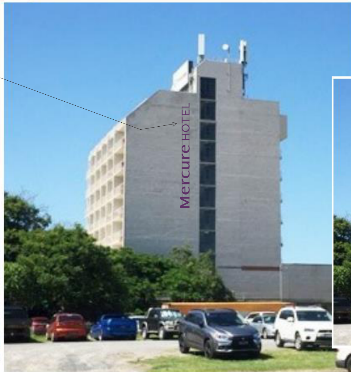
ILLUMINATED MERCURE HOTEL SIGN 12.9m x 1.17m
