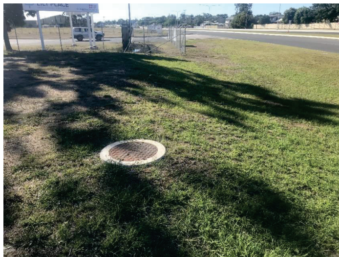
Figure 8 – Existing Sewer Access Chamber – North-east Corner
