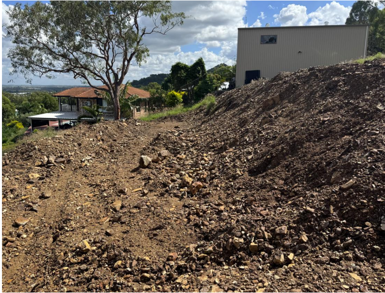
Figure 1 - Zone of building pad.
