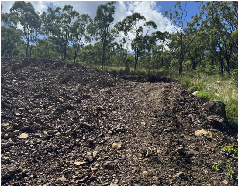
Figure 2 - Initial preparations for concrete driveway.
