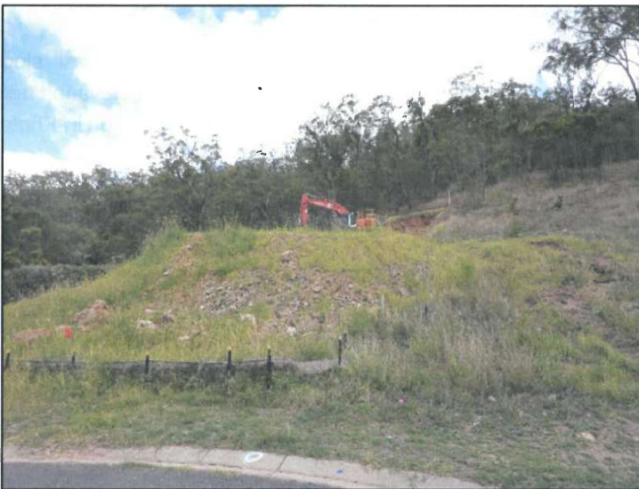
Photograph 3: View of the fill batter from Greenwood Close
