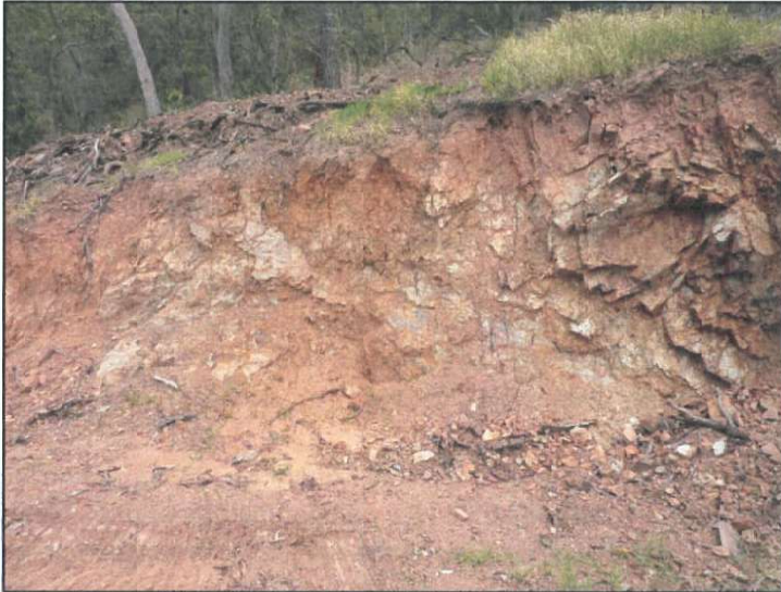
Photograph 2: View of cut face behind the upper platform
