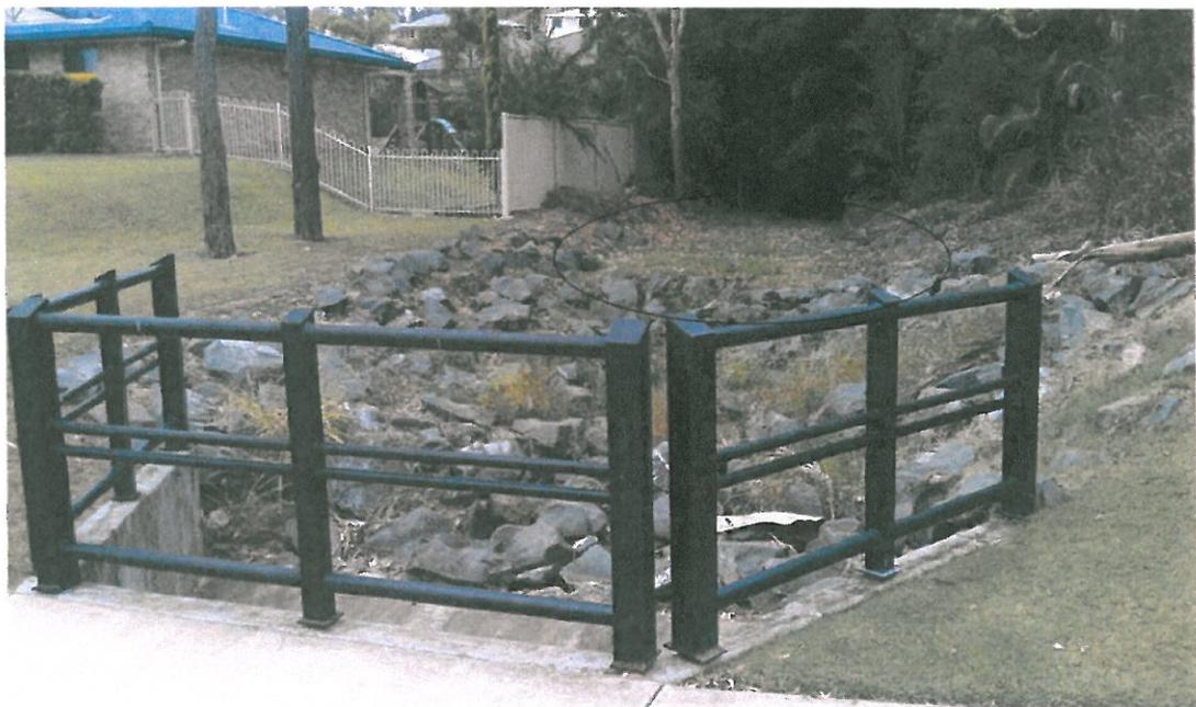
Photo Image: Existing upstream rock protection including sedimentation basin
