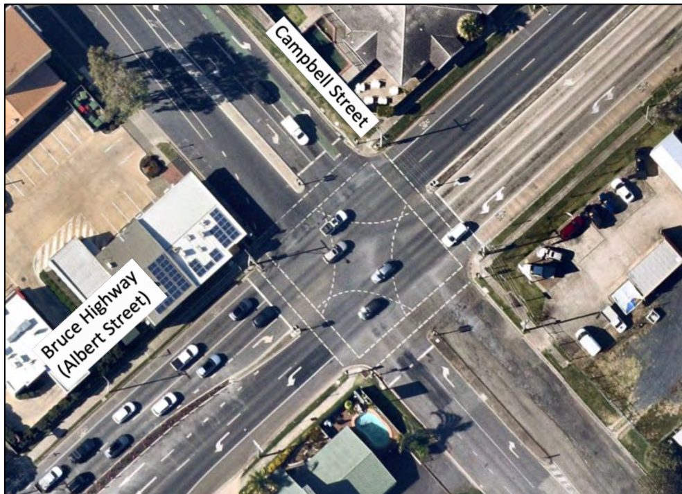
Figure 2.14: Albert Street / Campbell Street intersection [Source: Nearmap]
