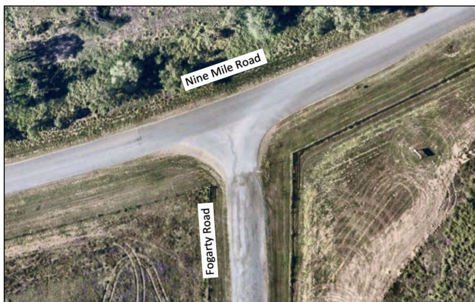
Figure 2.10: Nine Mile Road / Fogarty Road intersection [Source: Nearmap]
