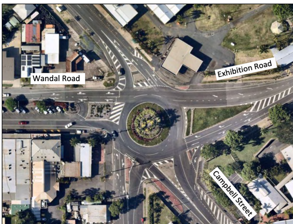
Figure 2.12: Wandal Road / Campbell Street / Exhibition Road roundabout [Source: Nearmap]
