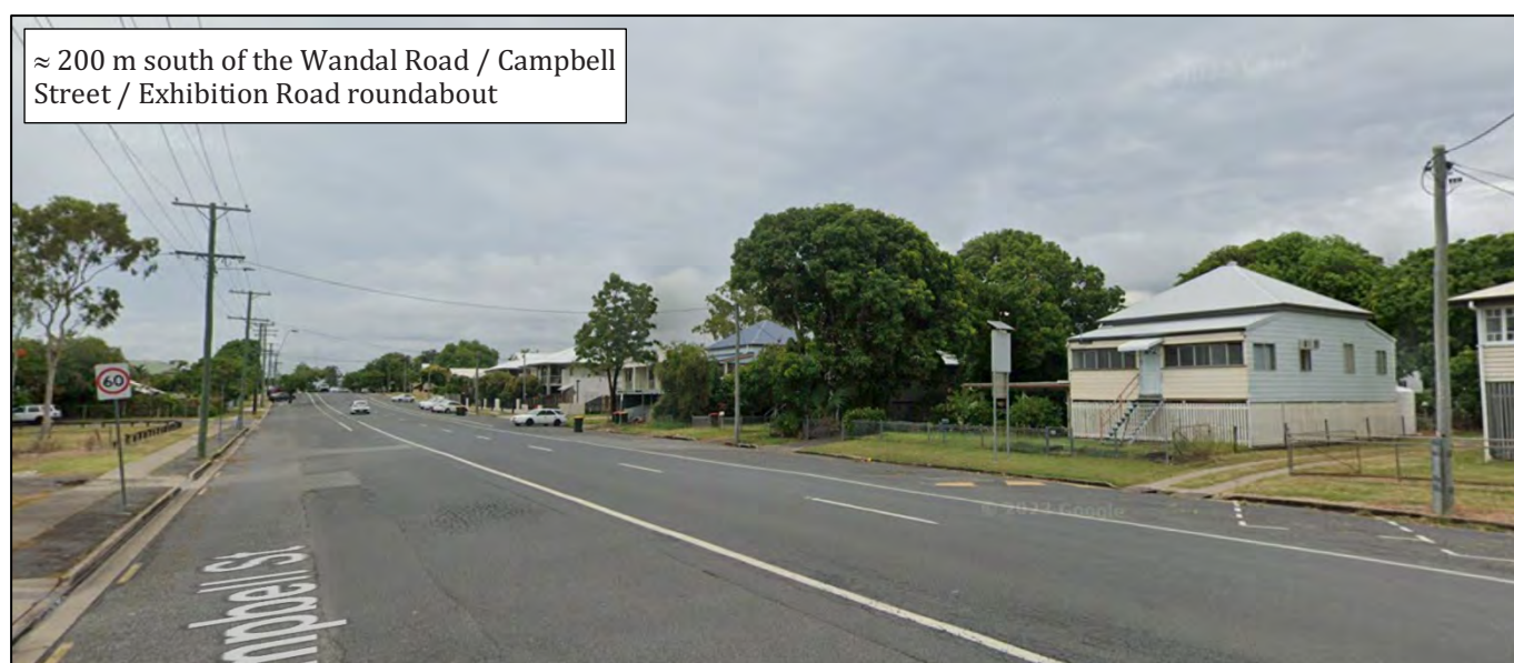
Figure 2.5: Campbell Street pavement conditions in year 2022 [Source: Google Street View]
