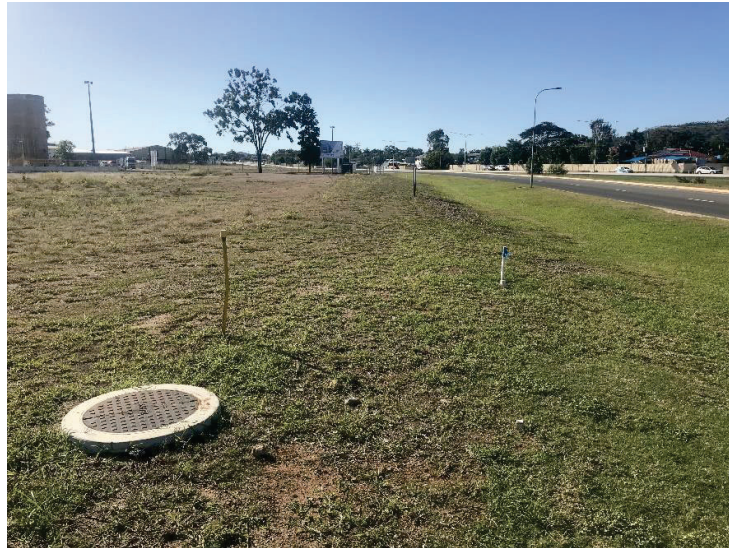
Figure 9 – Existing Sewer Access Chamber – South-east Corner
