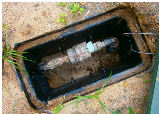
Above: underground water meter in box
