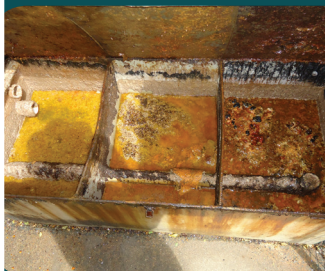
Grease trap pictured - grease, oil and fats collected from a local business
