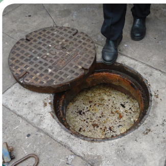
Sewer man hole pictured - grease, oil and fats collected from a local business
