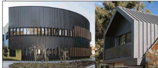
Metal Cladding Type- Lysaght Longline 305 or similar approved
