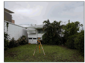
SOUTH WEST VIEW
