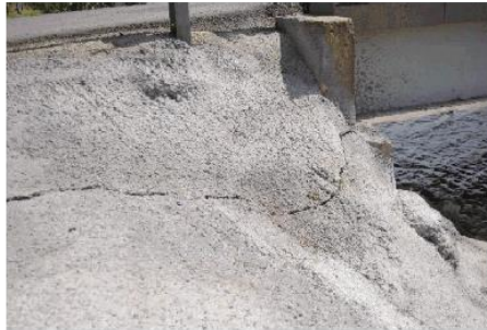
Photo 6: PRO to RHS A1. Note crack
