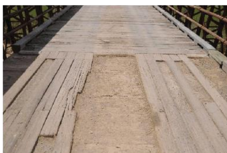
Photo 12: Longitudinal decking boards missing
