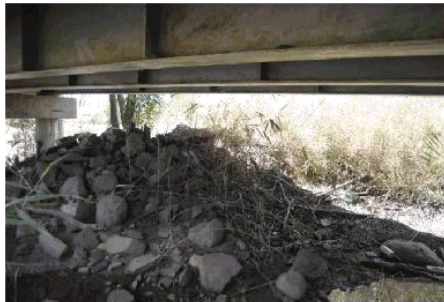
Photo 9: rubble under Span 4 adjacent to A2
