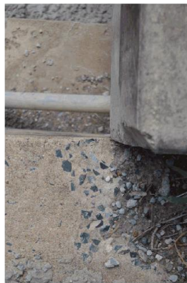
Photo 15: Spalling concrete at top of ballast wall from impact of deck slab
