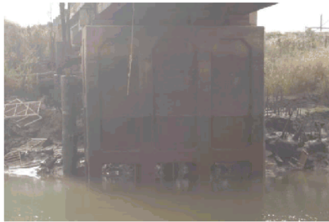
Photo 18: Pier 2 face 1 (previous 2013 inspection). Note water level
