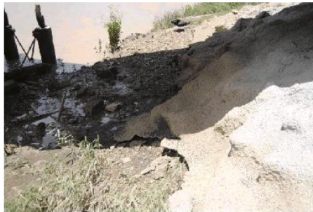
Photo 8: A1 toe of PRO showing minor scour under
