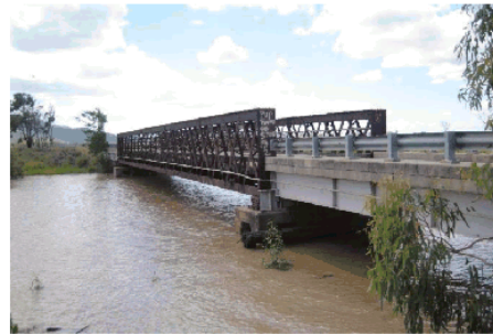
Photo 19: Side view of bridge. Note water level against piers
