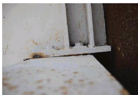
Photo 17: View of top of headstock girder showing tilt and separation between deck beam and headstock girder
