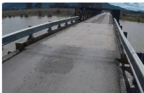
Photo 5: AP1. Note repair and crack at rear of abutment
