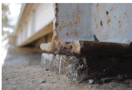
Photo 16: Headstock Girder at Pier 1 looking towards A1 showing tilt of girder
