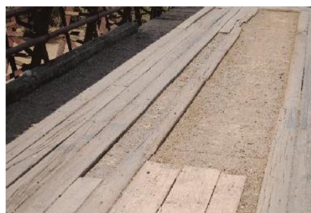
Photo 11: Longitudinal decking boards missing
