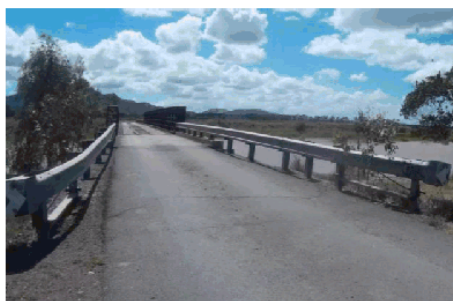
Photo 4: AP1. Note transverse crack
