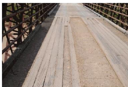
Photo 13: Longitudinal decking boards missing, note kerb board missing LHS
