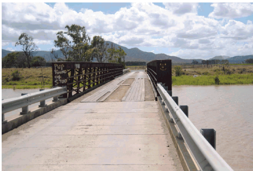
Photo 1 – View of Bridge from Approach 1
