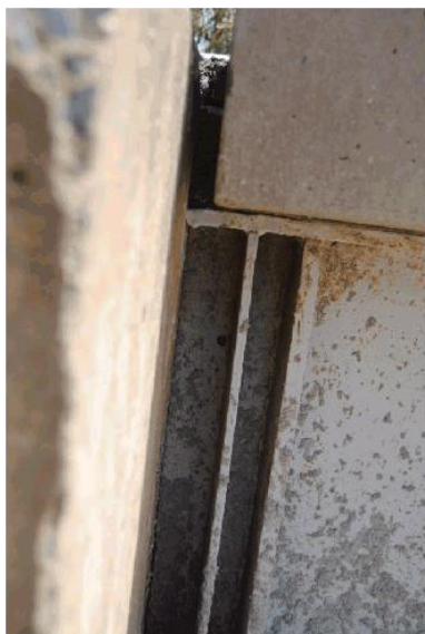
Photo 14: Girder at A1 hard up against ballast wall
