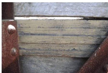
Photo 10: Deck construction – structural plywood layers
