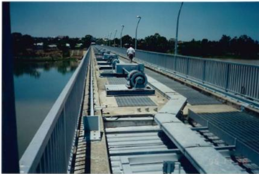
Barrage view along bridge towards right bank. Shows gate lifting hoists
