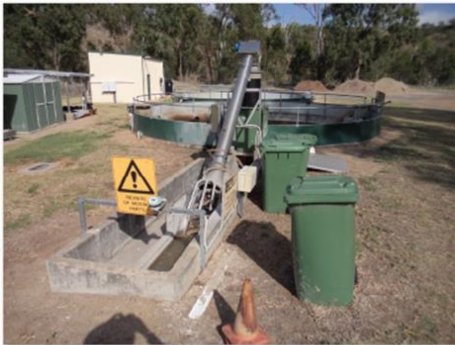
Figure 5.37 : Mt Morgan Sewerage Treatment Plant
