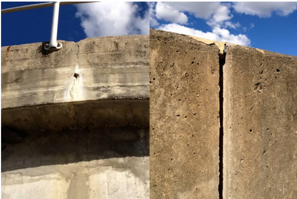
Figure 1. Photographs showing the ageing electrical switchboard (top) and the commencement of structural failure in the clarigester (bottom left) and trickling filter tank (bottom right).
