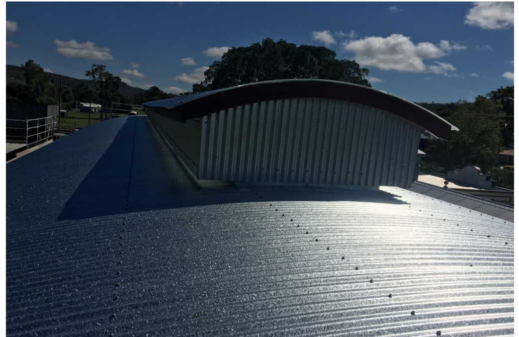
Mt Morgan Railway – Roof replacement completed
