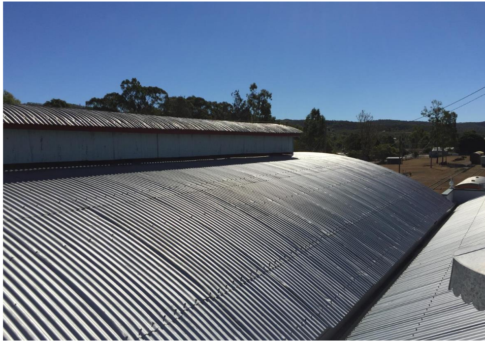
Mt Morgan Railway – Before roof replacement
