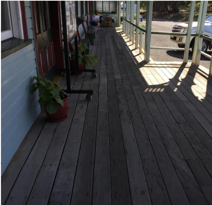
Before deck replacement
