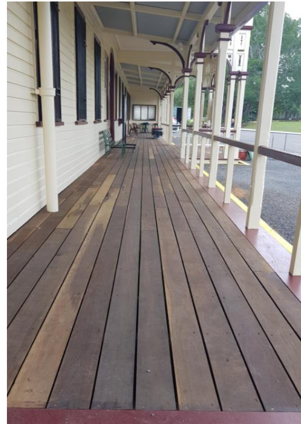
Deck Replacement Completed
