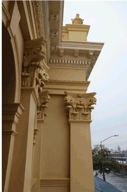
Figure 9: Pilaster decoration from first floor balcony (EHP, March 2017)
