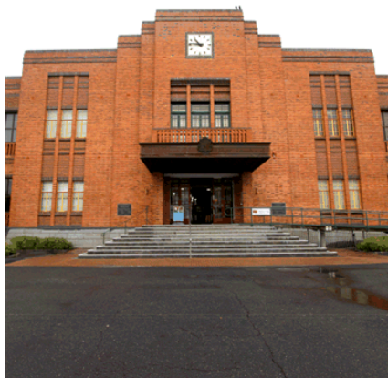
Figure 1: Rockhampton Town Hall (EHP, March 2017)
