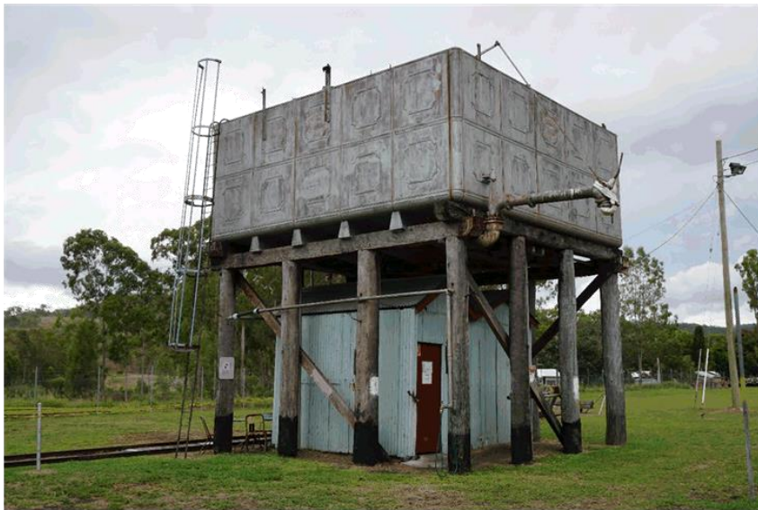
Figure 8: Mount Morgan Railway Station, water tank, from southeast (EHP, 2017)
