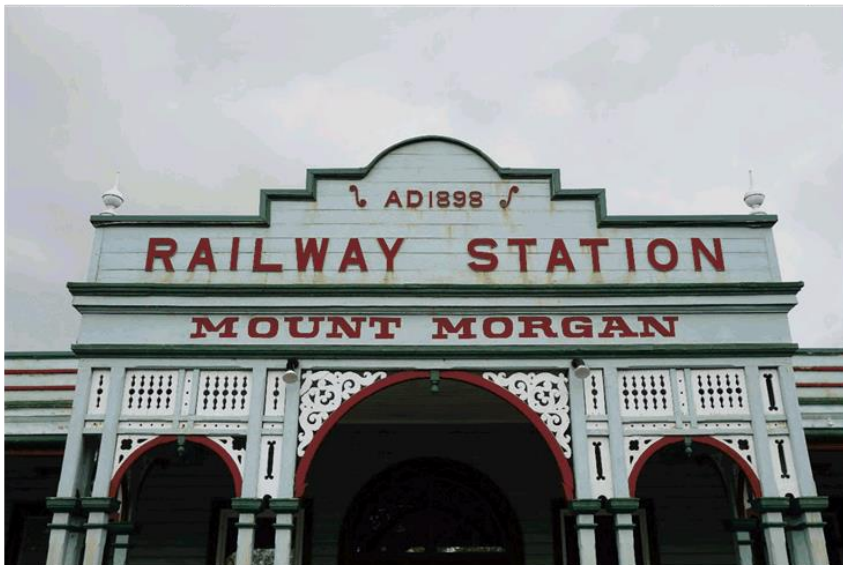
Figure 4: Mount Morgan Railway Station, entrance portico with decorative timber work, from east (EHP, 2017)
