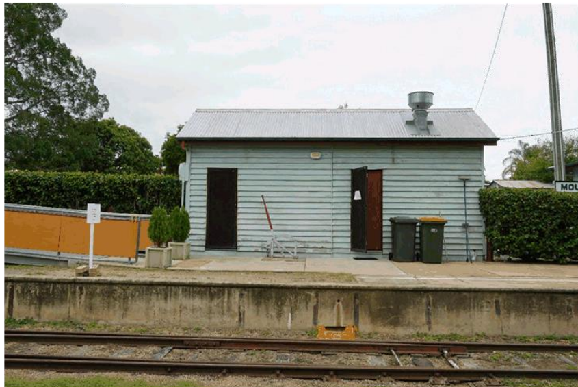
Figure 9: Mount Morgan Railway Station, shunter's / guard's room, from west (EHP, 2017)
