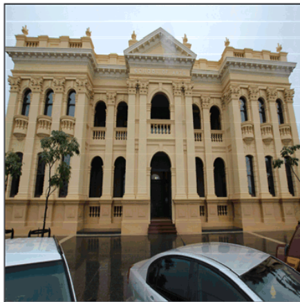
Figure 1: Rockhampton School of Arts (EHP, March 2017)
