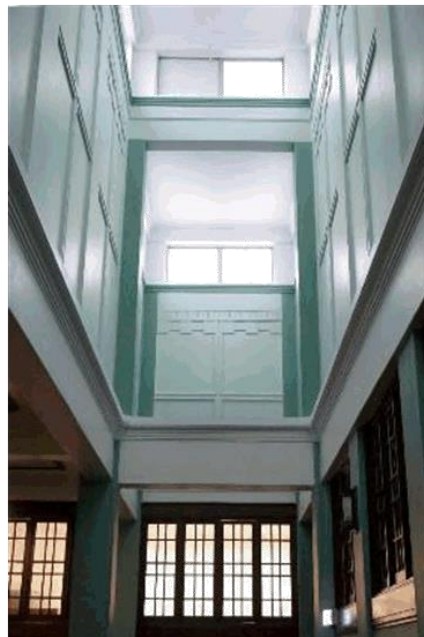
Figure 6: Light well above central stairs, Rockhampton Town Hall (EHP, March 2017)
