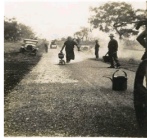
Laying bitumen on Bouldercombe Road, early 1930s
