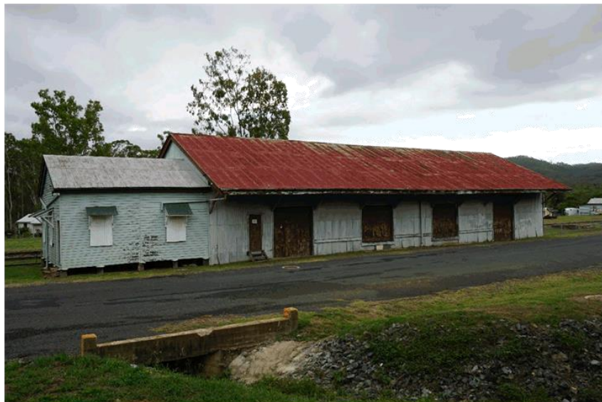
Figure 10: Mount Morgan Railway Station, goods shed, from southeast (EHP, 2017)
