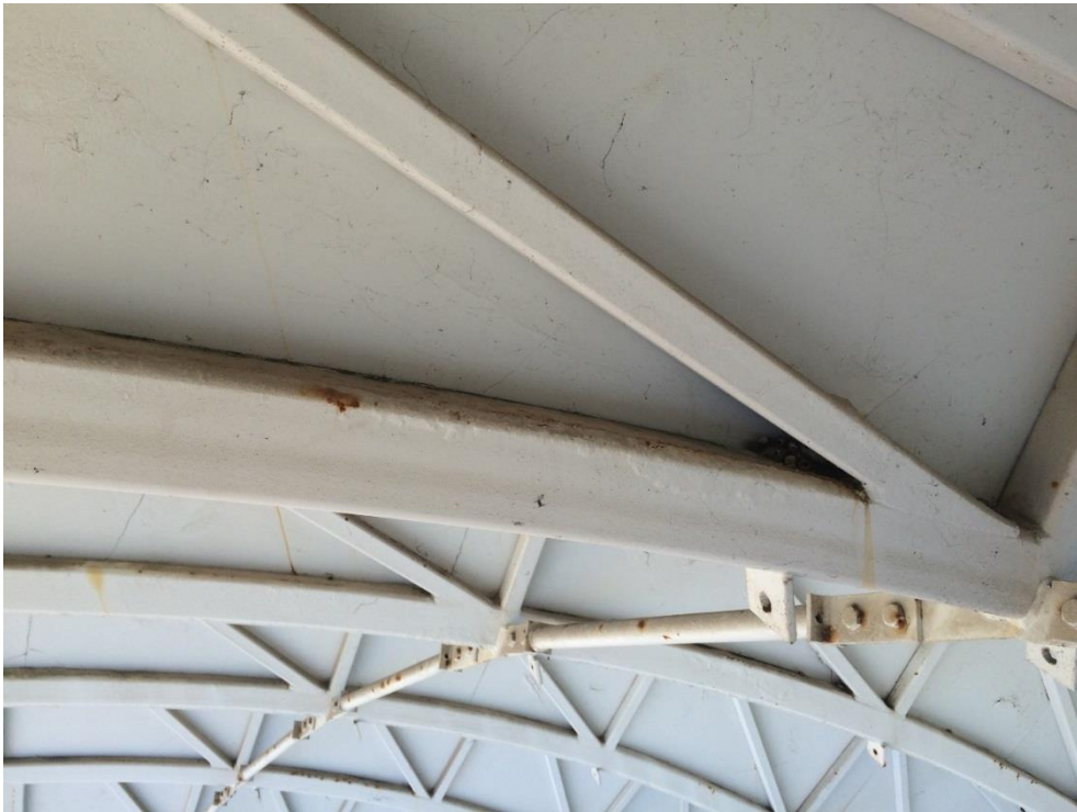
Photo 139 - Minor corrosion to bottom chord of truss
