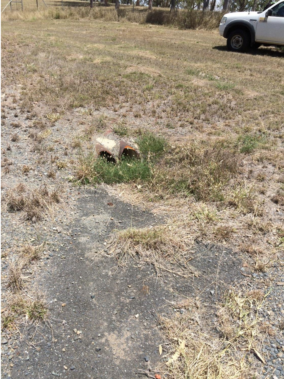
Photo 229 - Stormwater outlet from front of sound shell discharging at north west of sound shell
