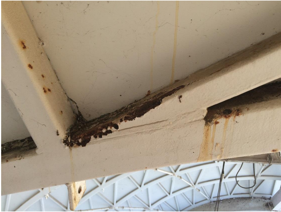
Photo 109 - Minor corrosion to web member
