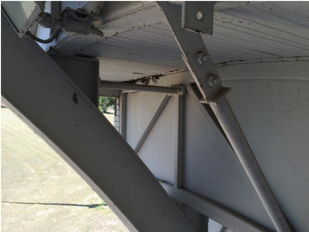
Photo 163 - Minor corrosion to bottom plate
