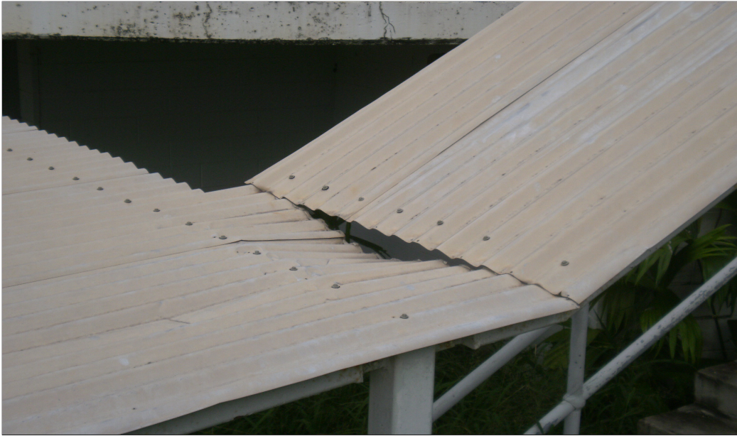
Damaged roofing iron to covered walk way (photo 9)
