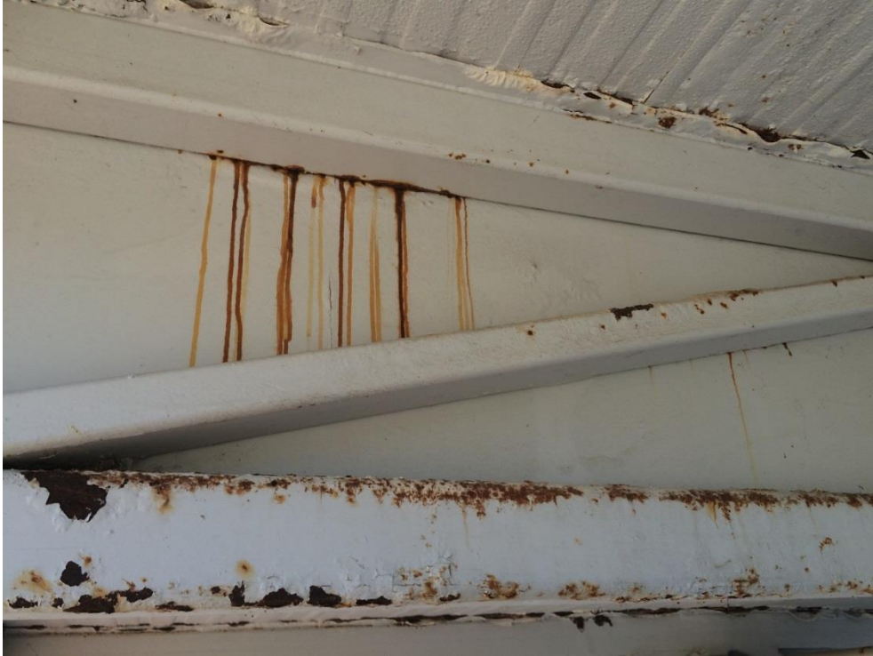
Photo 194 - Heavy corrosion to top plate and bottom chord
