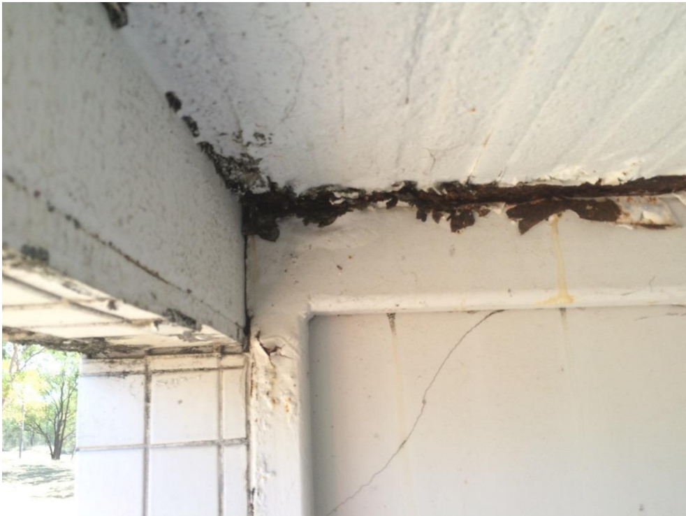
Photo 181 - Heavy corrosion to top plate and top chord of truss
