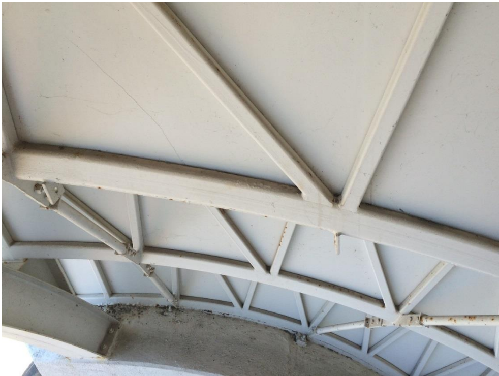
Photo 165 - Minor corrosion to bottom plate
