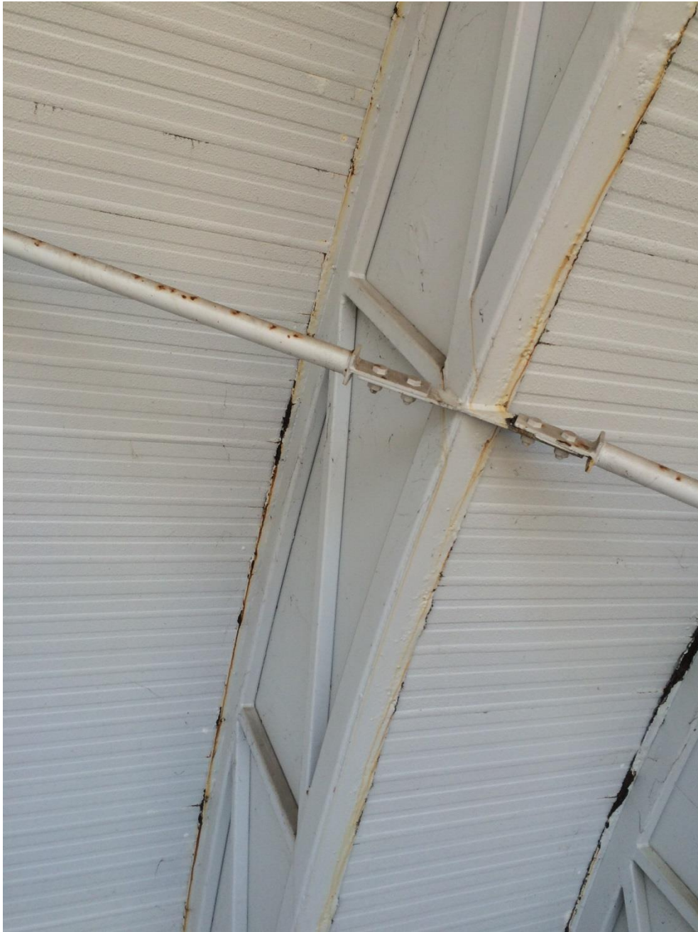
Photo 120 - Minor corrosion to truss top and bottom plate
