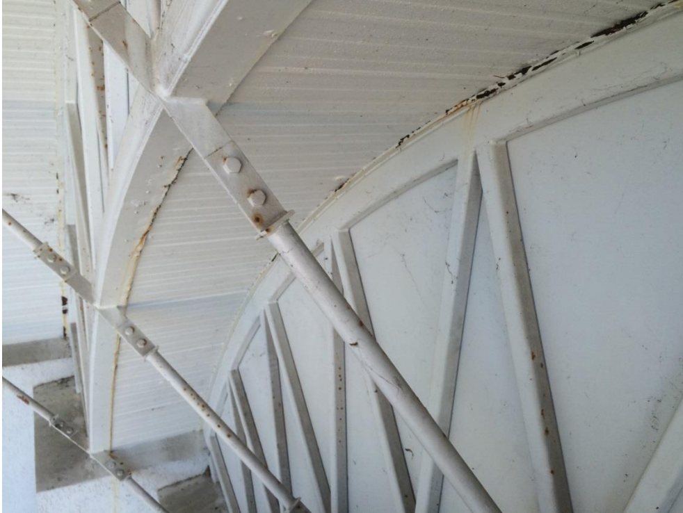
Photo 025 - Struts generally in good condition
