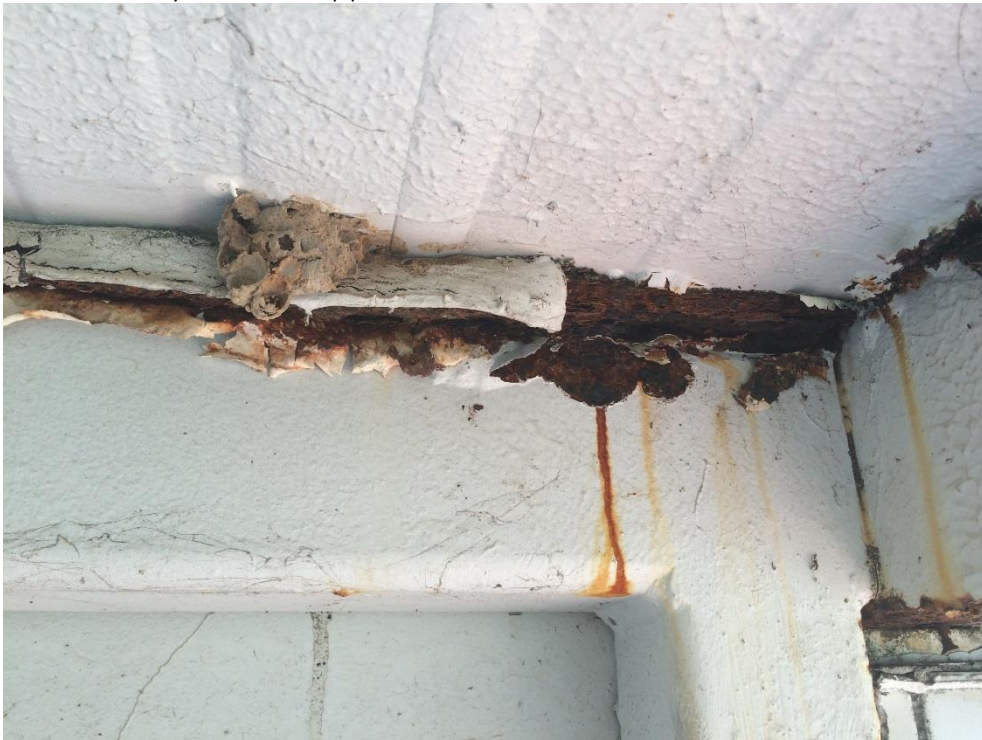
Photo 088 - Heavy corrosion to top plate
