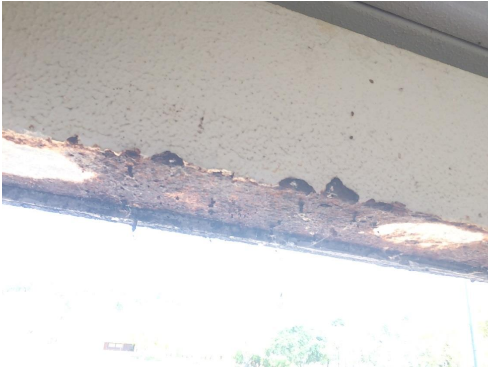
Photo 103 - Heavy corrosion to fascia
