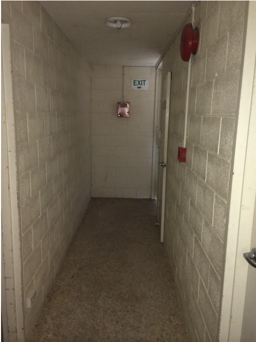
Photo 246 - Lower ground floor corridor
