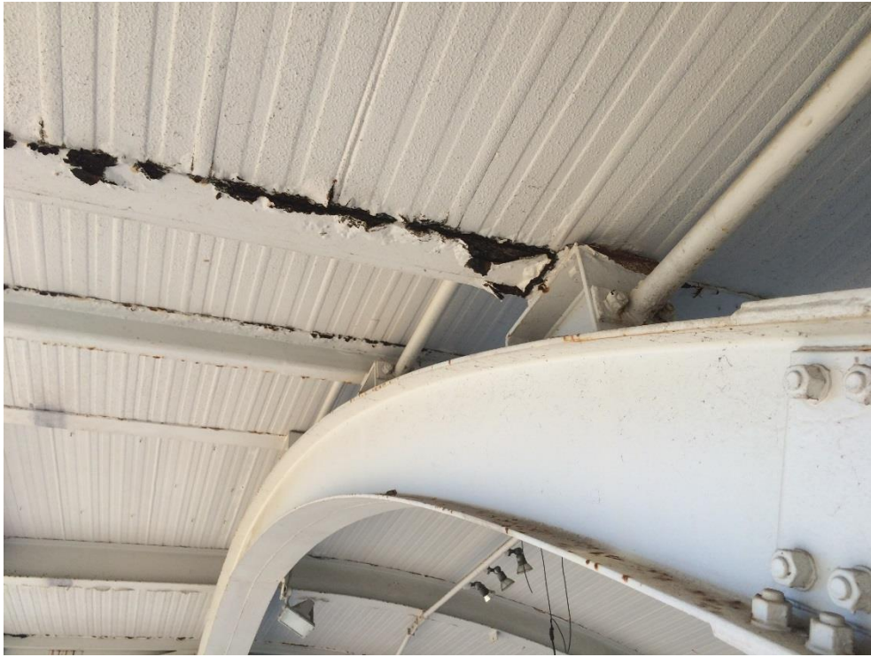
Photo 070 - Heavy corrosion to bottom plate
