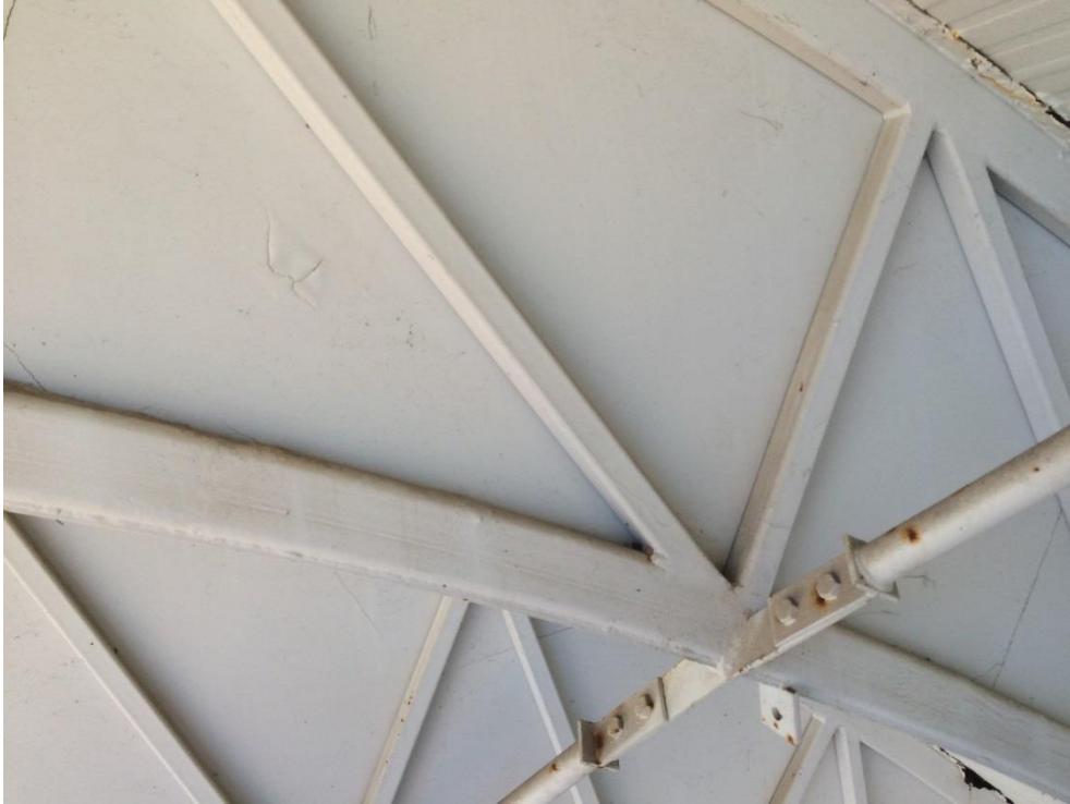
Photo 160 - Minor corrosion to bottom chord
