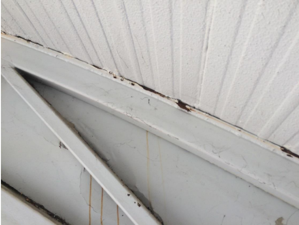
Photo 136 - Heavy corrosion to top plate
