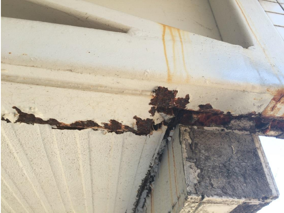
Photo 078 - Heavy corrosion to truss bottom chord at the exterior face of the soundshell
