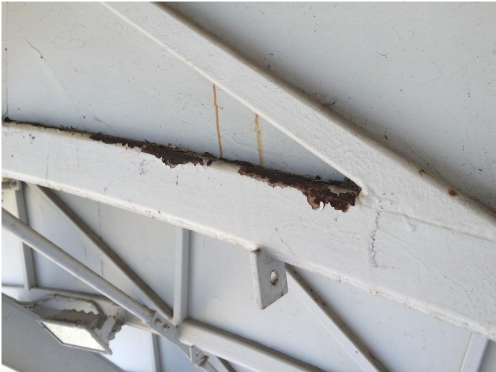
Photo 151 - Heavy corrosion to bottom chord
