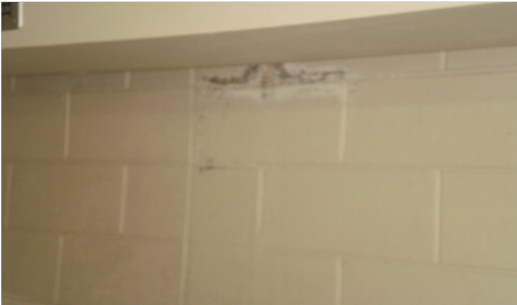
Internal paintwork in poor condition (photo 18)
