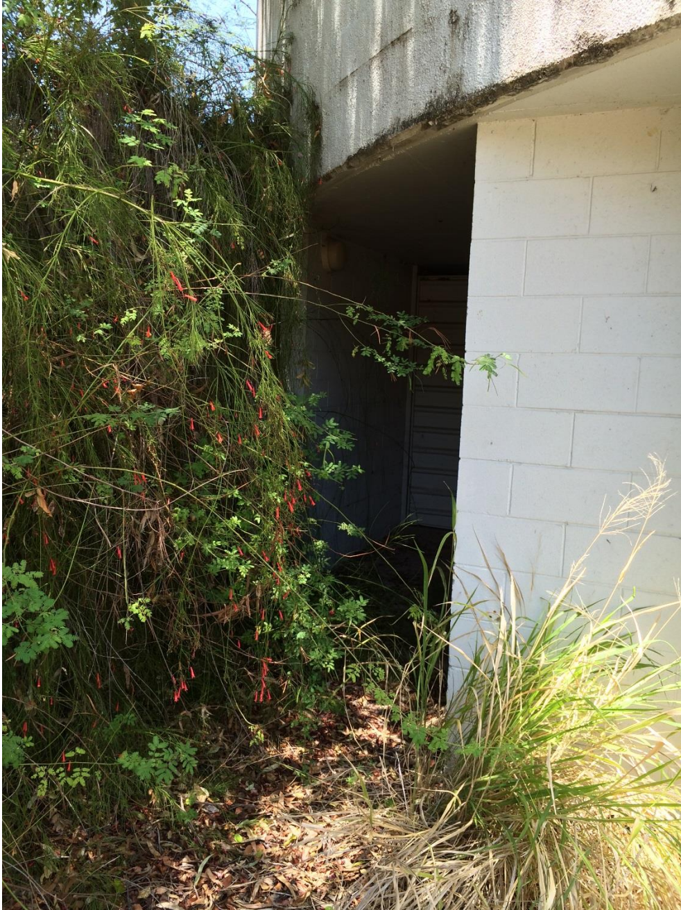
Photo 237 - Entrance to lower ground floor
