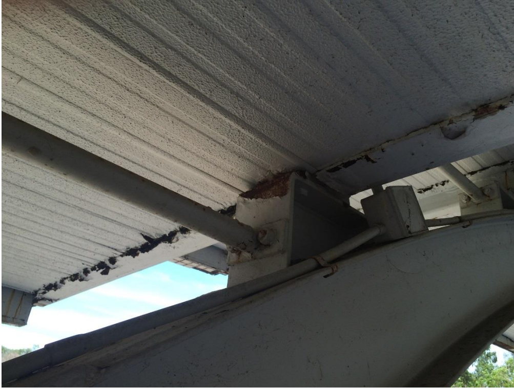
Photo 065 - Minor corrosion to bottom plate and stub
