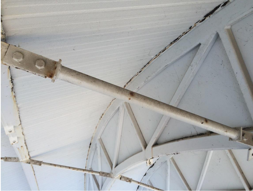
Photo 059 - Heavy corrosion to top plate
