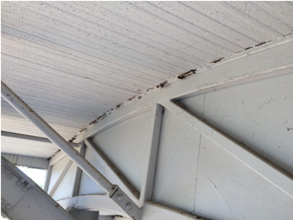
Photo 149 - Heavy corrosion to top plate
