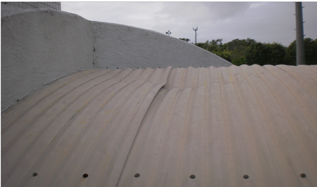
Damaged roofing iron to covered walk way (photo 8)
