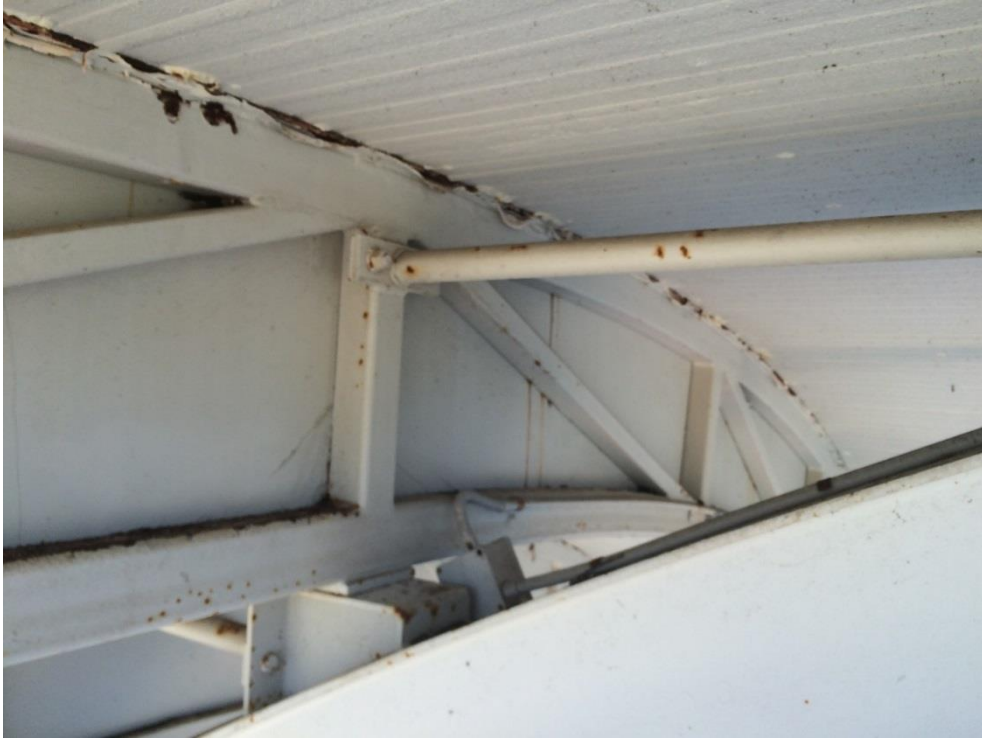
Photo 190 - Minor corrosion to bottom chord
