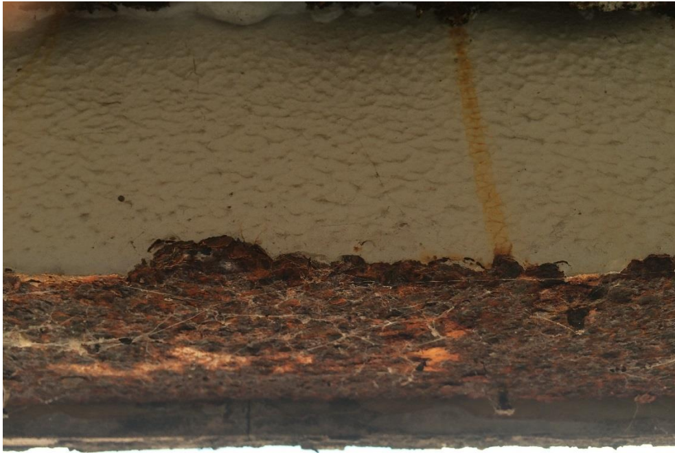
Photo 093 - Heavy corrosion to fascia
