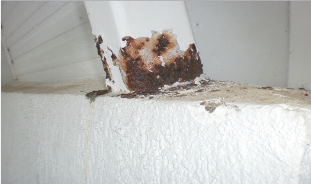
Rusted Structural Steel (photo 1)
