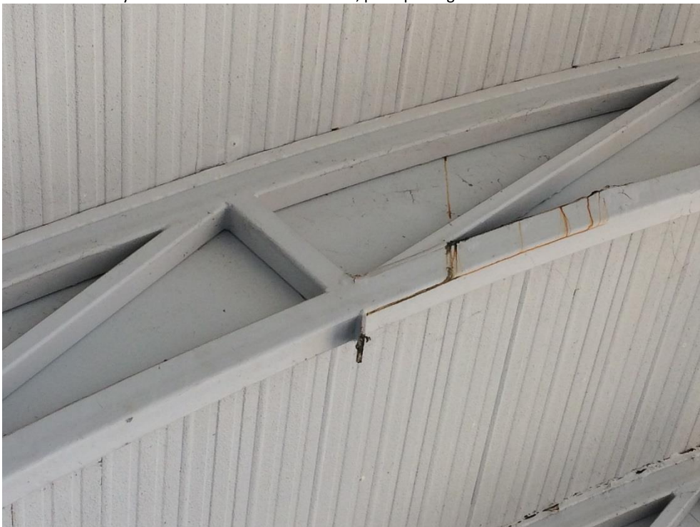
Photo 117 - Heavy corrosion to truss bottom chord, paint peeling off
