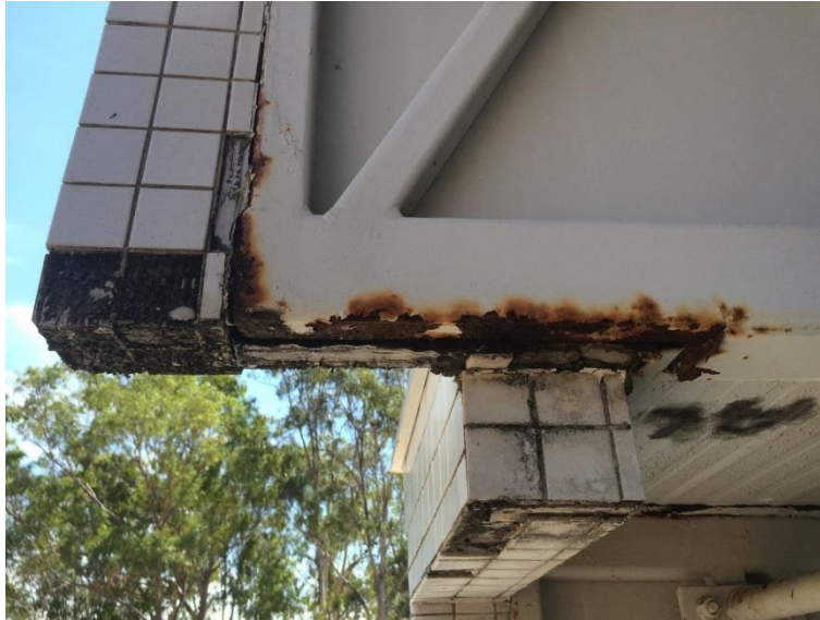
Figure 12 - Corrosion of bottom chord at the exterior face of the sound shell
