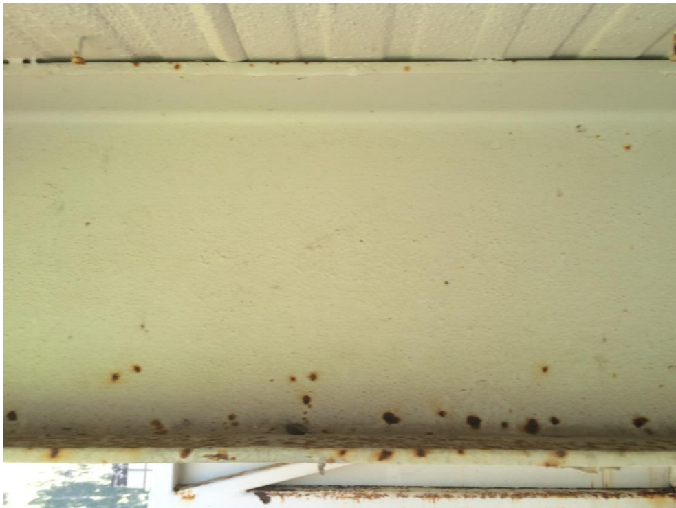
Photo 199 - Minor corrosion to roof beam
