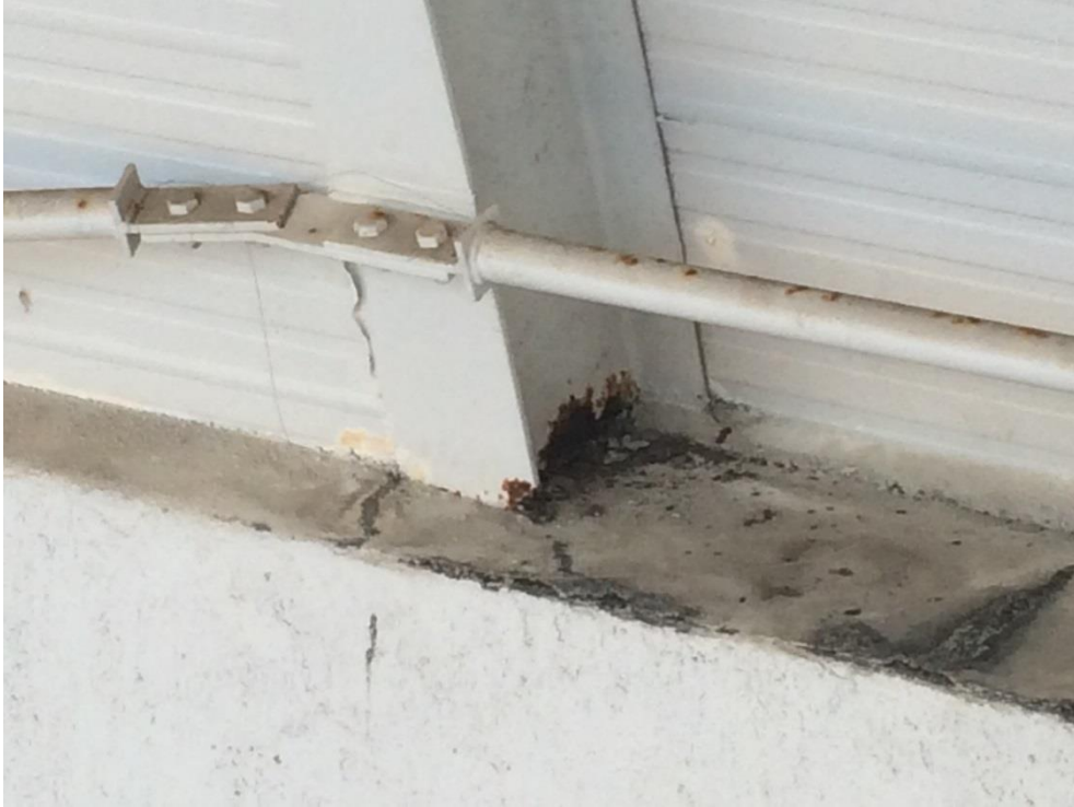
Photo 130 - Heavy corrosion to web of roof beam
