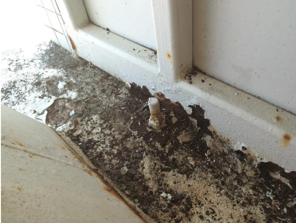
Photo 172 - Heavy corrosion to tab plate and nut
