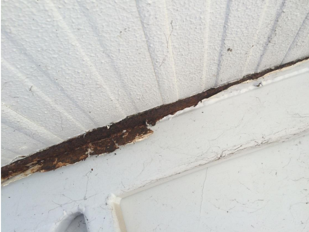
Photo 049 - Heavy corrosion to top plate
