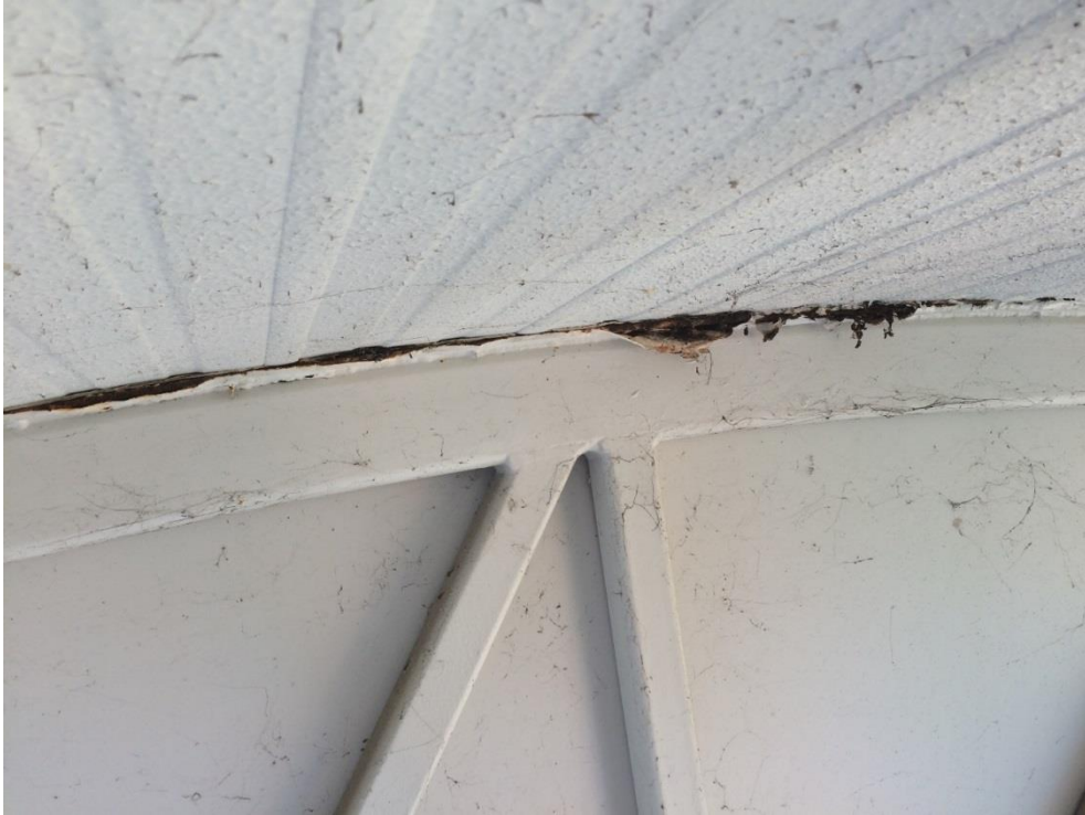
Photo 031 - Heavy corrosion to top plate
