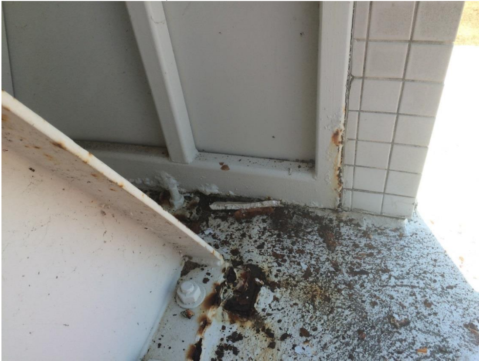
Photo 006 - Corrosion to truss tab plate
