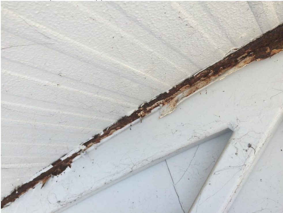
Photo 050 - Heavy corrosion to top plate
