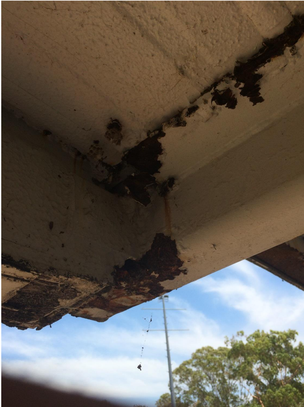
Photo 082 - Minor corrosion to truss bottom chord at the exterior face of the soundshell
