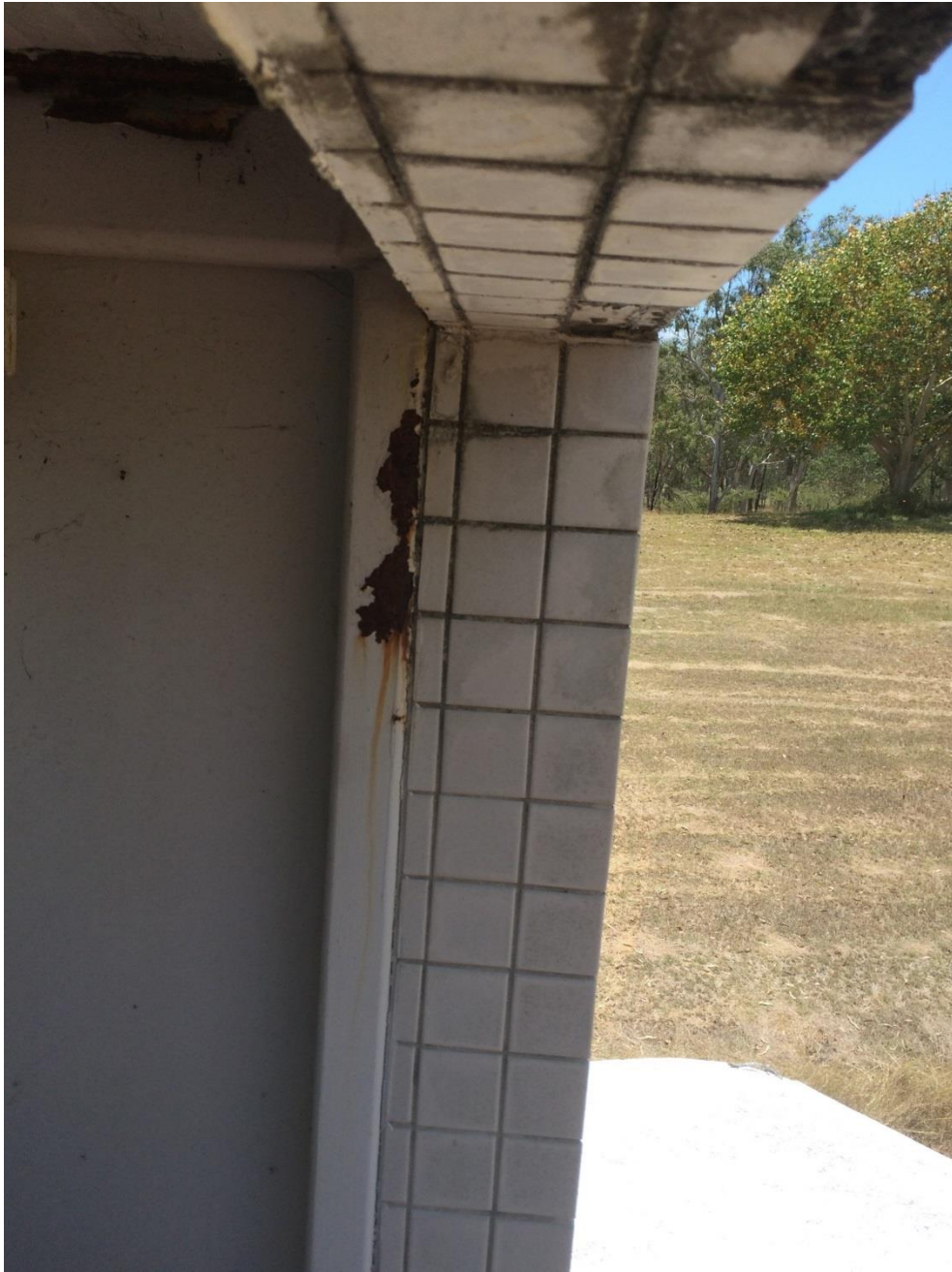
Photo 007 - Corrosion to truss web at end
