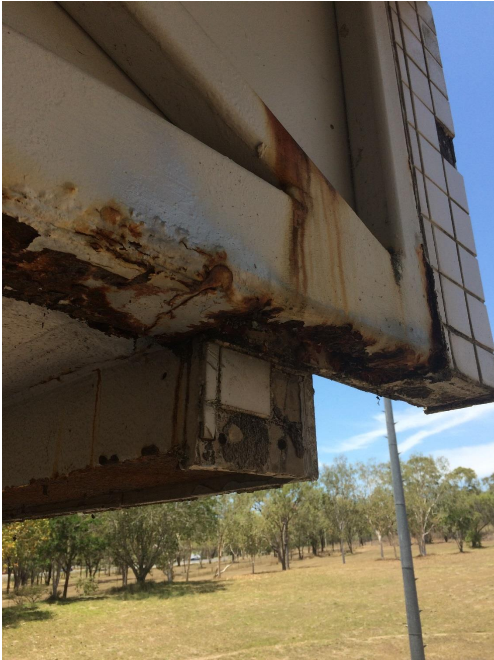
Photo 073 - Heavy corrosion to truss bottom chord at the exterior face of the soundshell
