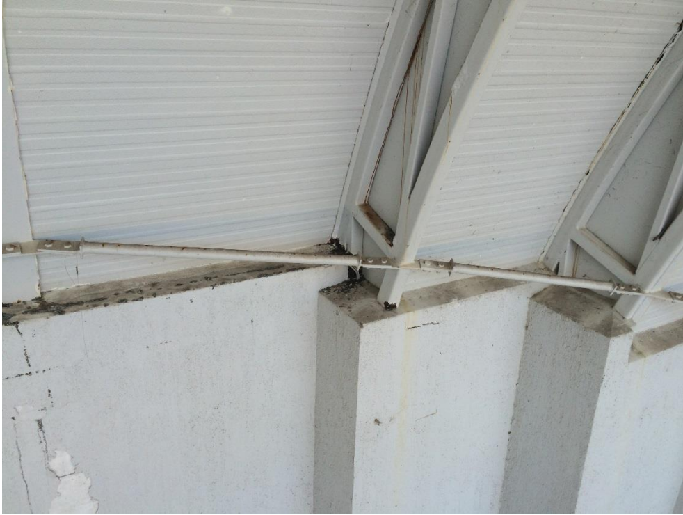
Photo 112 - Heavy corrosion to truss at concrete interface
