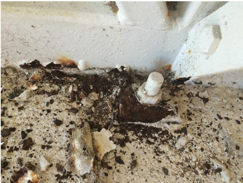
Photo 173 - Heavy corrosion to tab plate and nut
