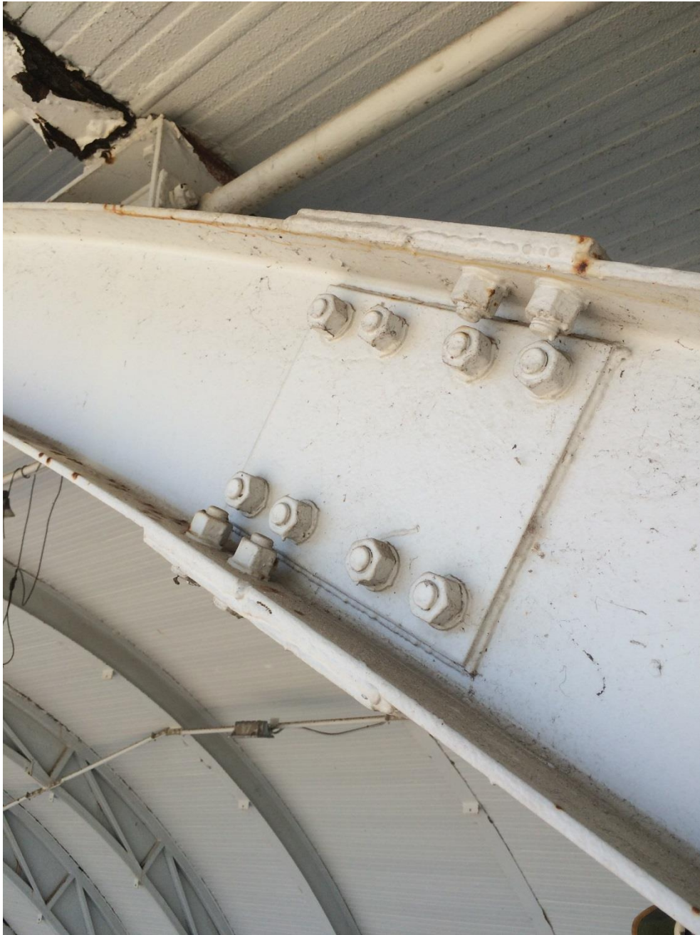
Photo 072 - Splice in good condition
