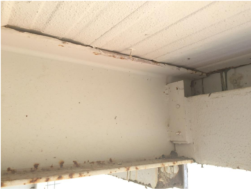
Photo 098 - Minor corrosion to roof beam
