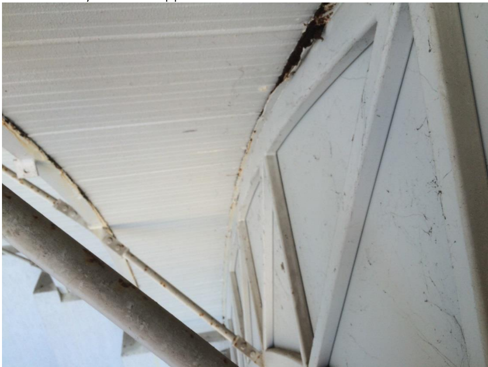
Photo 044 - Heavy corrosion to top plate
