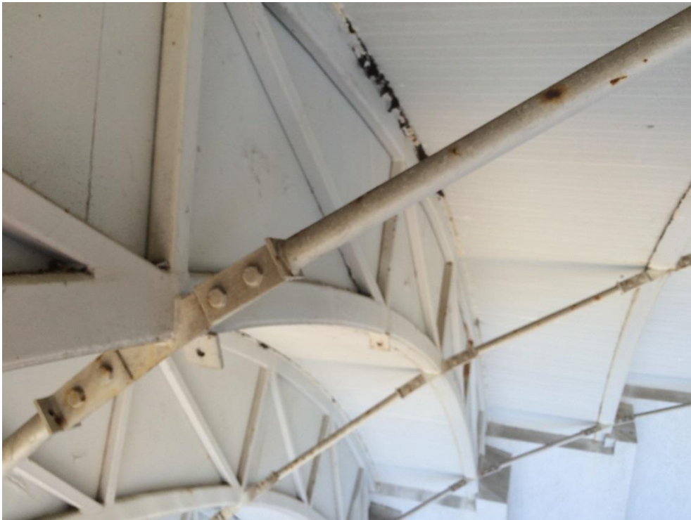
Photo 153 - Minor corrosion to top plate
