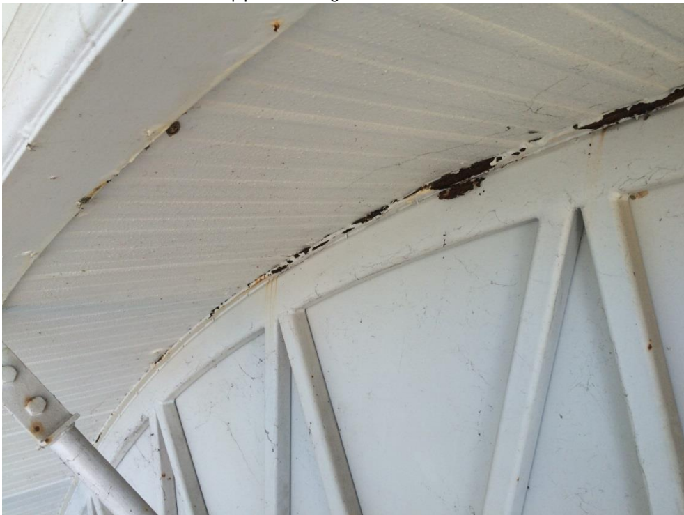
Photo 024 - Heavy corrosion to top plate all along
