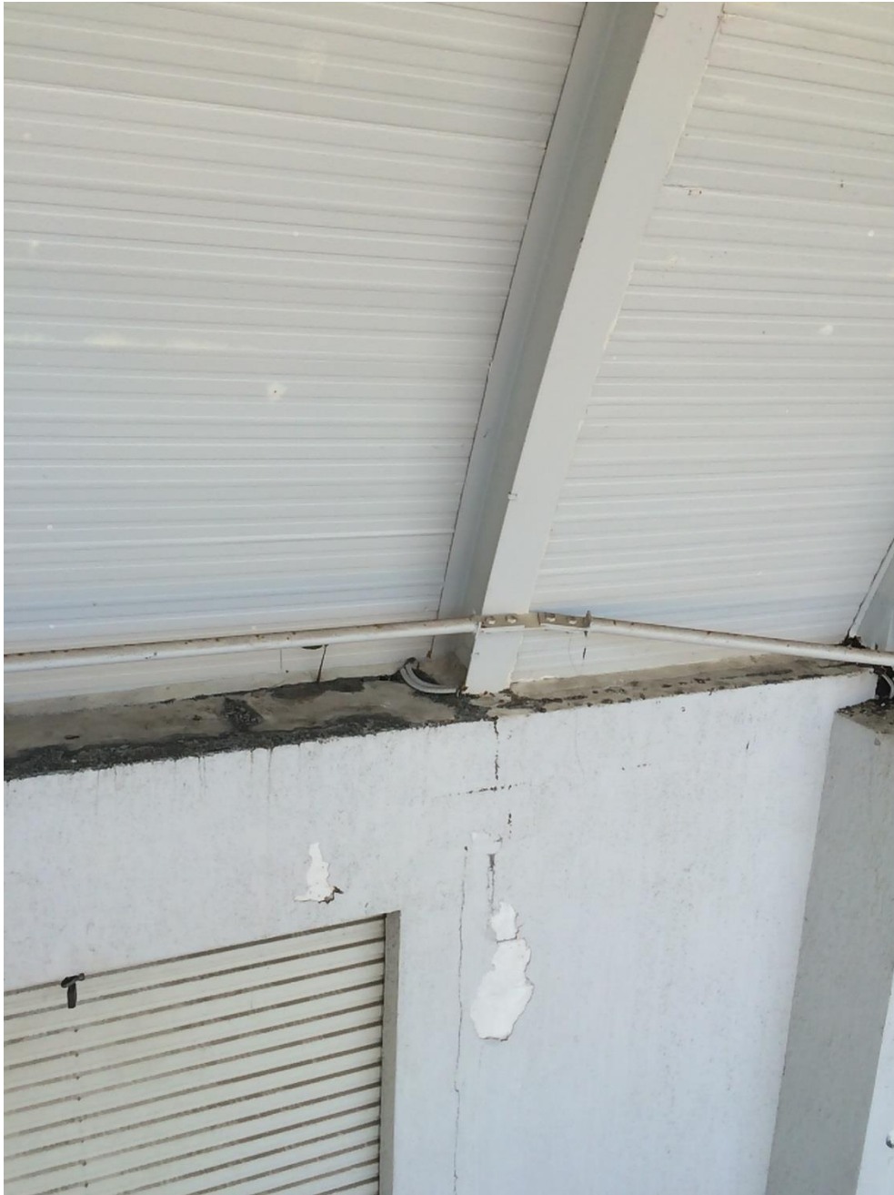
Photo 111 - Minor corrosion to roof beam to concrete interface
