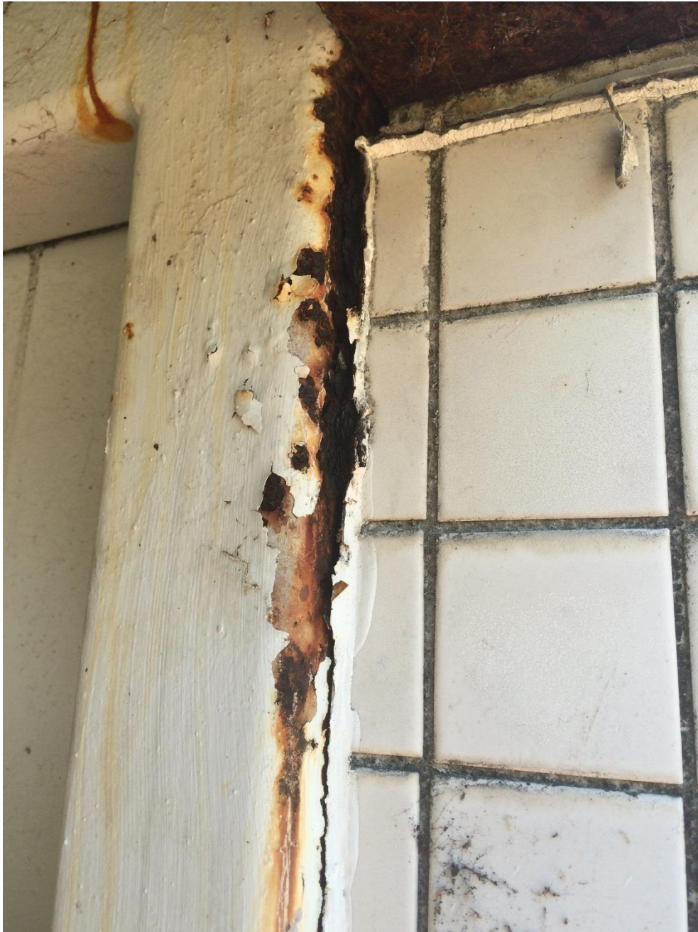
Photo 089 - Heavy corrosion to truss web at exterior face of the soundshell
