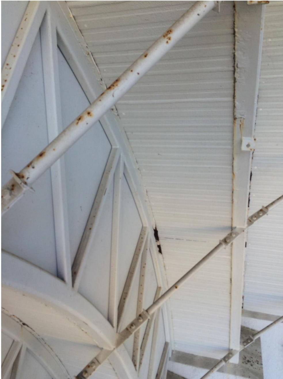
Photo 169 - Minor corrosion to bottom plate and top plate
