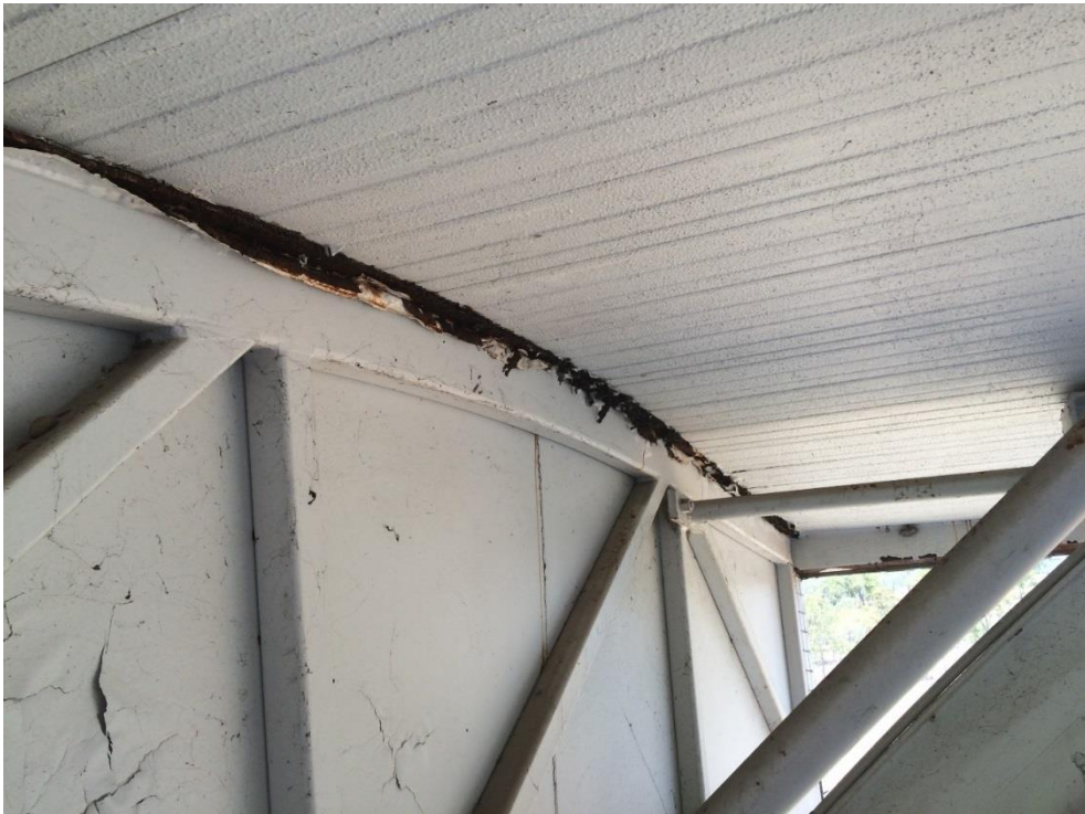
Photo 046 - Heavy corrosion to top plate
