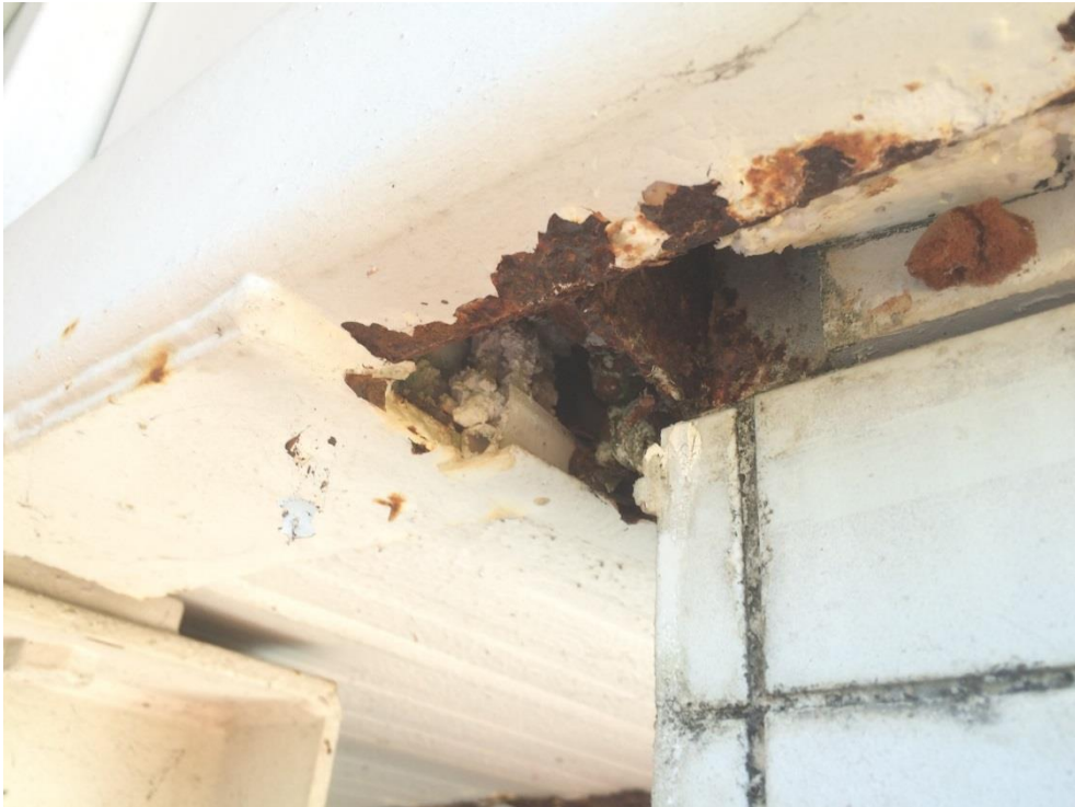
Photo 011 - Corrosion to truss bottom chord and web at end
