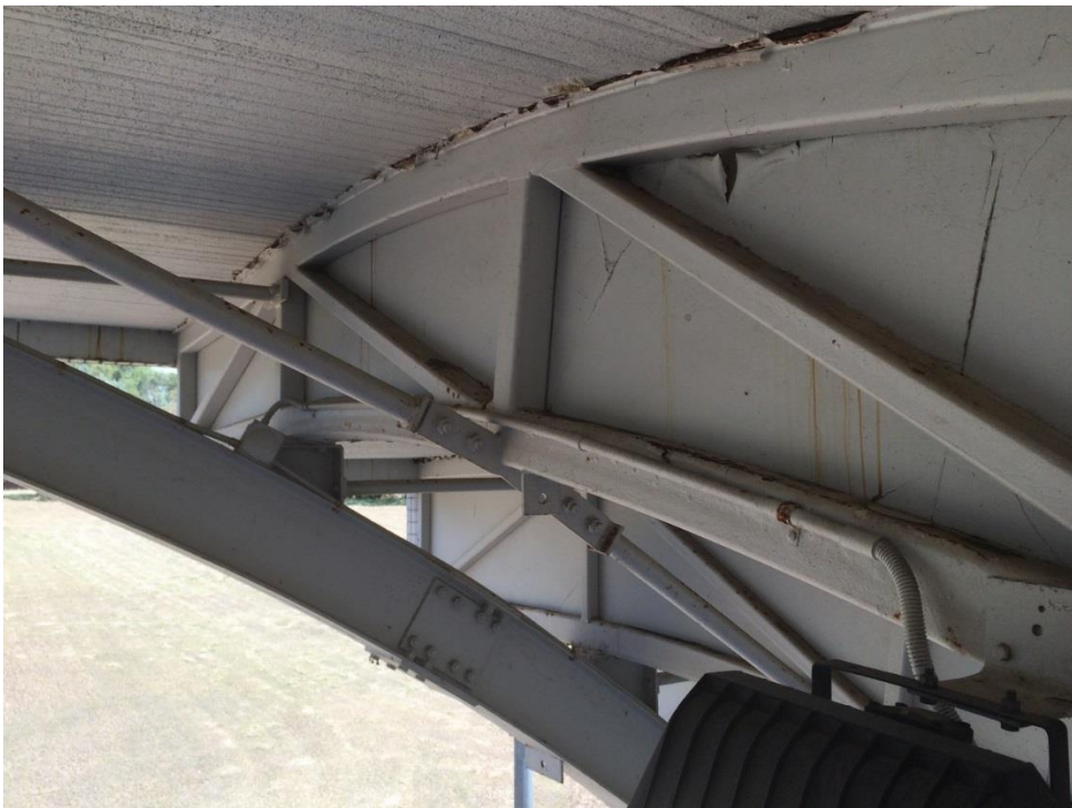
Photo 141 - Minor corrosion to bottom chord of truss and top plate
