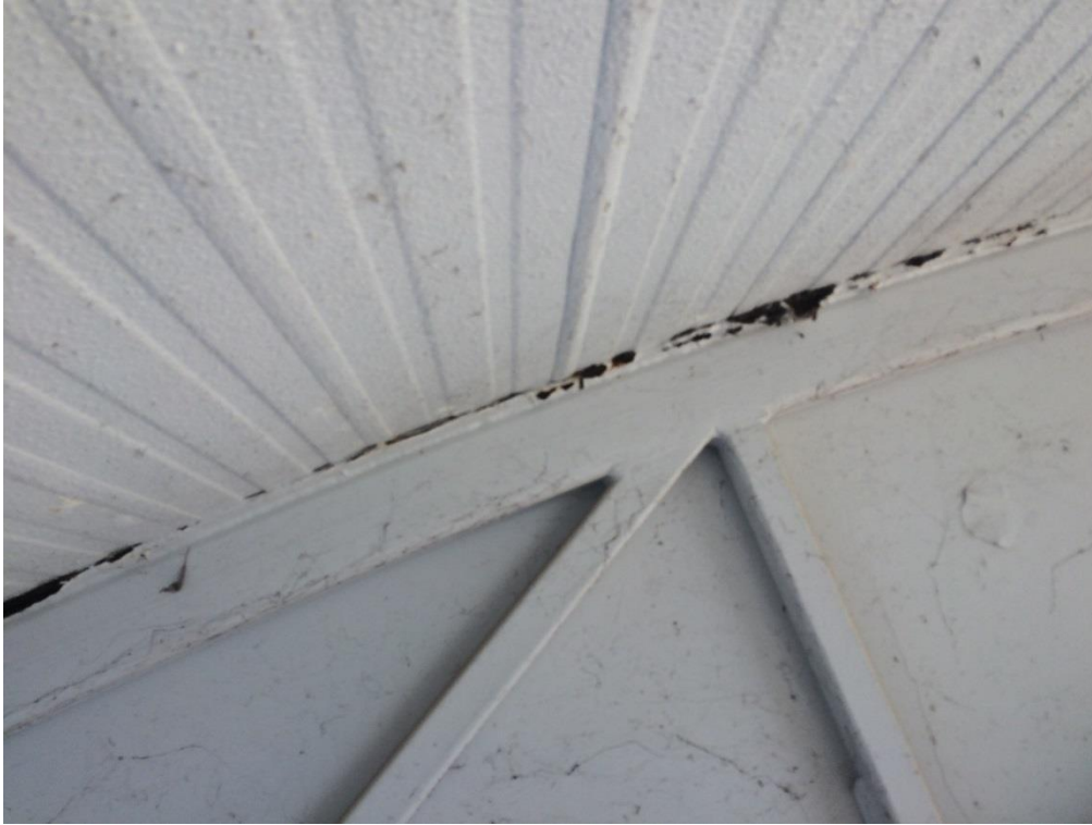
Photo 057 - Heavy corrosion to top plate
