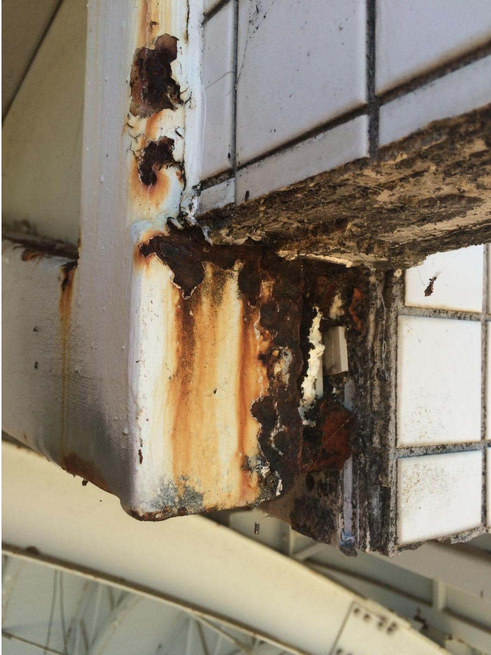
Photo 090 - Heavy corrosion to truss web at exterior face of the soundshell
