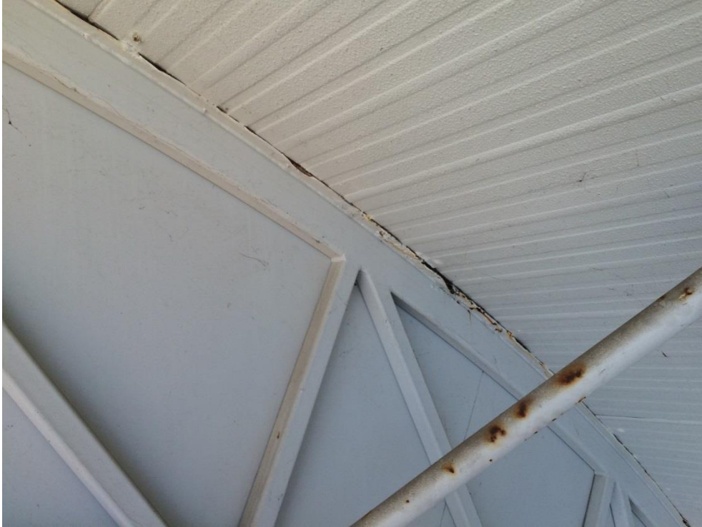
Photo 158 - Minor corrosion to top plate
