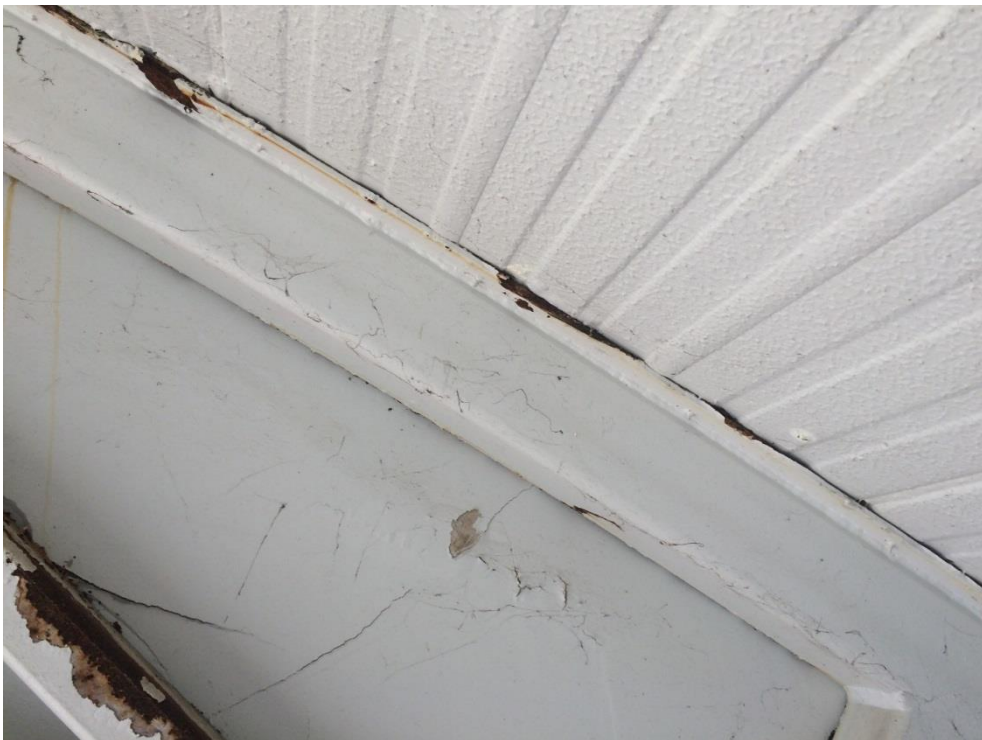
Photo 137 - Heavy corrosion to top plate
