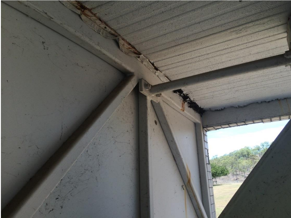
Photo 038 - Heavy corrosion to top plate
