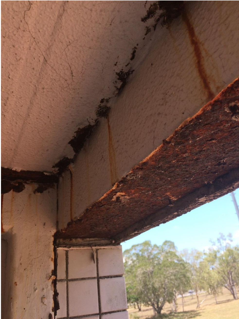
Photo 091 - Heavy corrosion to fascia
