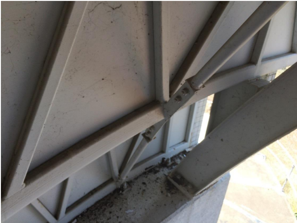
Photo 036 - Minor corrosion to struts
