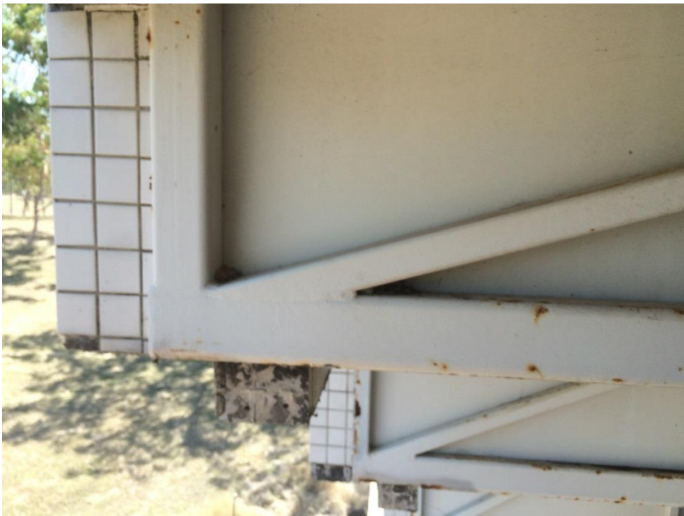
Photo 187 - Minor corrosion to bottom chord
