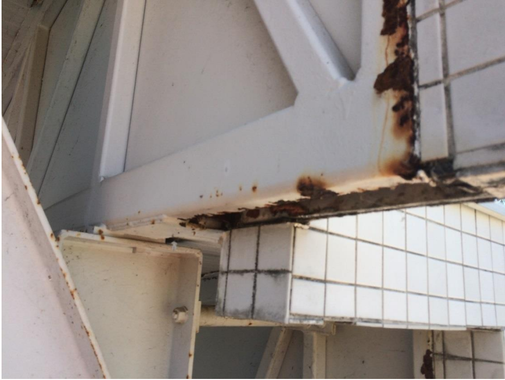
Photo 008 - Corrosion to truss bottom chord and web at end
