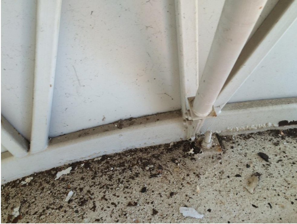
Photo 027 - Heavy corrosion to side of bottom chord
