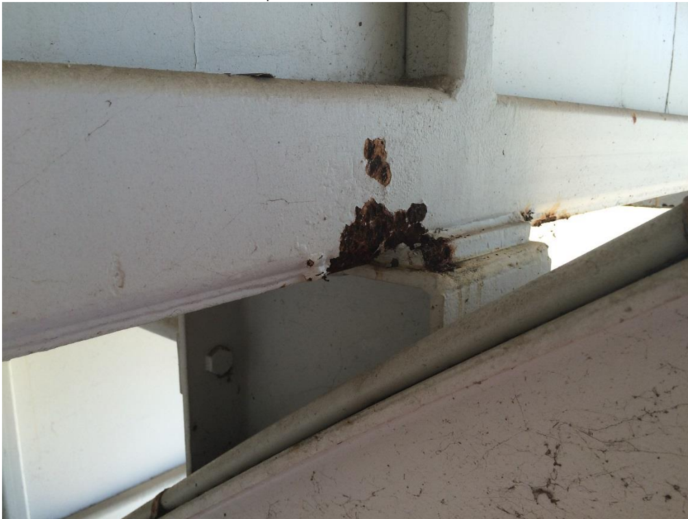
Photo 062 - Minor corrosion to bottom chord at stub
