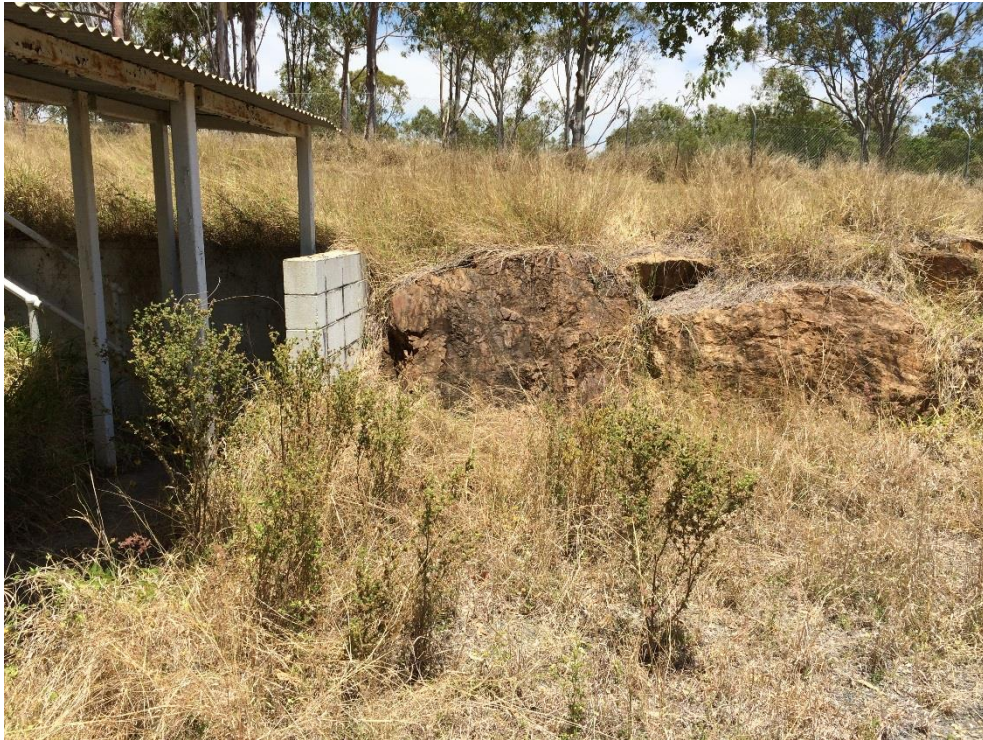
Photo 220 - Overgrown vegetation, boulder wall adjacent covered stairs
