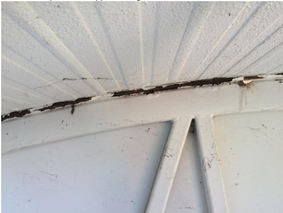
Photo 022 - Heavy corrosion to top plate all along
