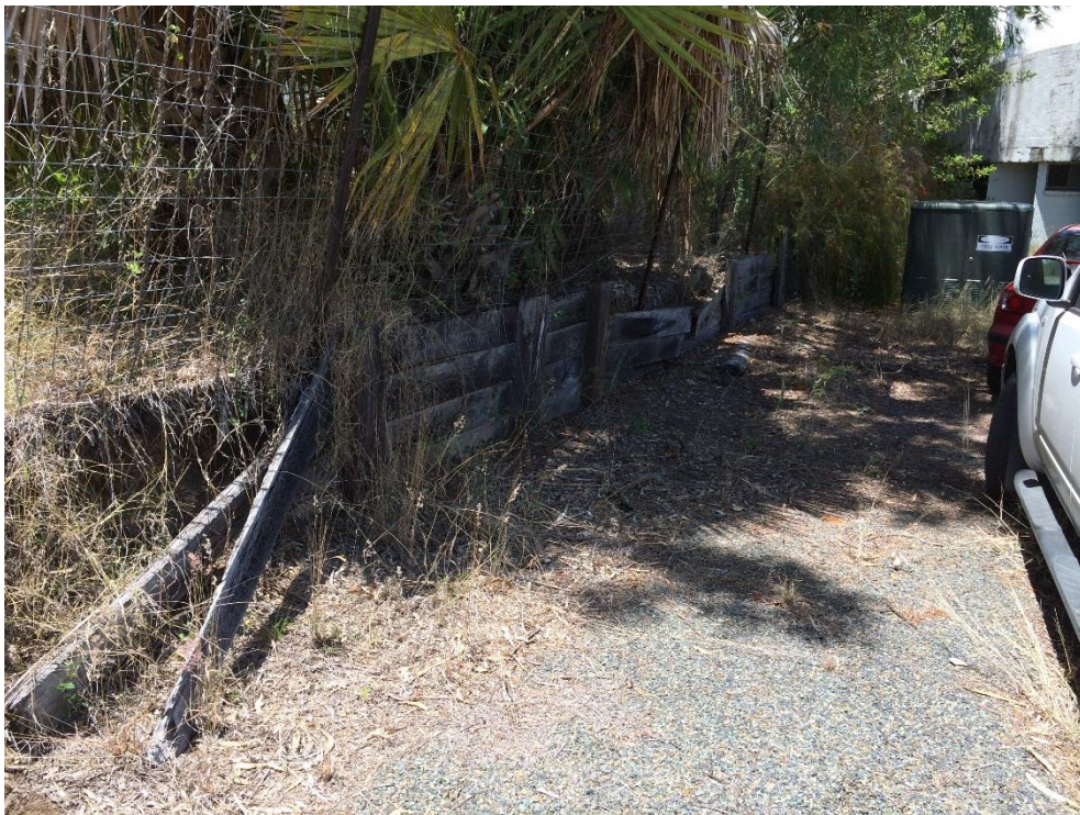
Photo 225 - Timber retaining wall, rotted and collapsed
