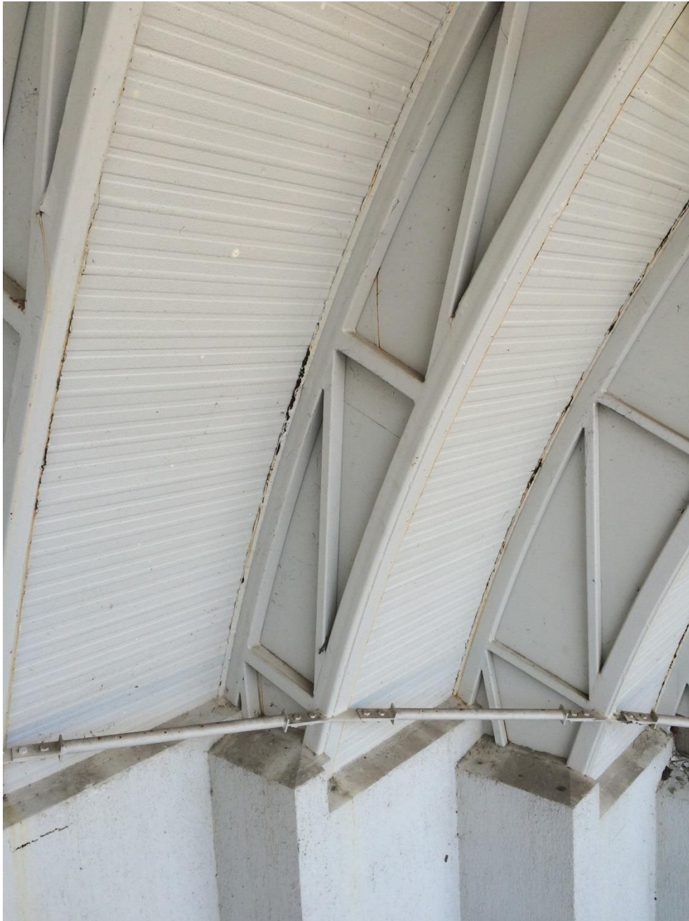
Photo 125 - Minor corrosion to truss top and bottom plate
