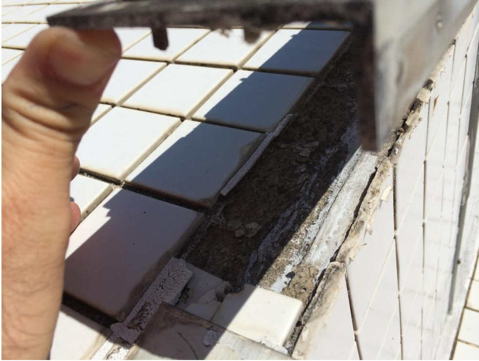
Photo 218 - Detail photo at loose aluminium cladding
