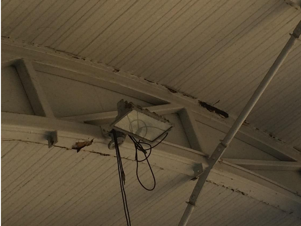
Photo 128 - Minor corrosion to truss top and bottom plate
