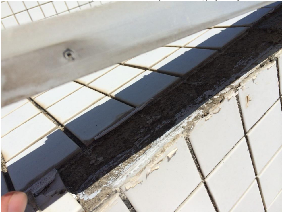
Photo 217 - Detail photo at loose aluminium cladding
