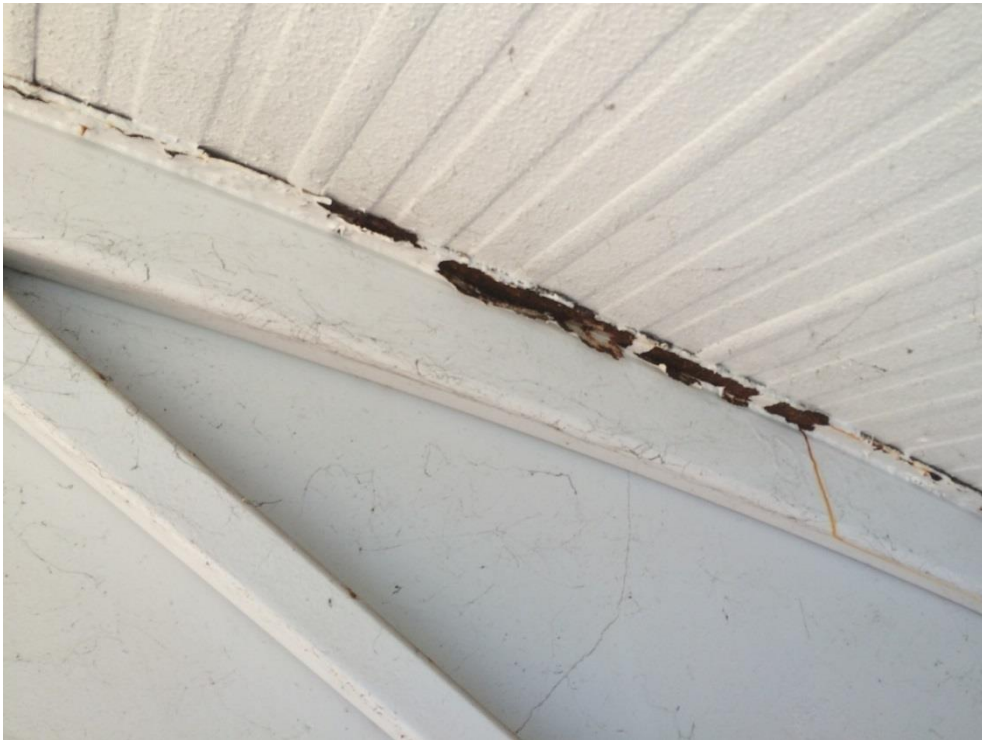
Photo 147 - Heavy corrosion to top plate
