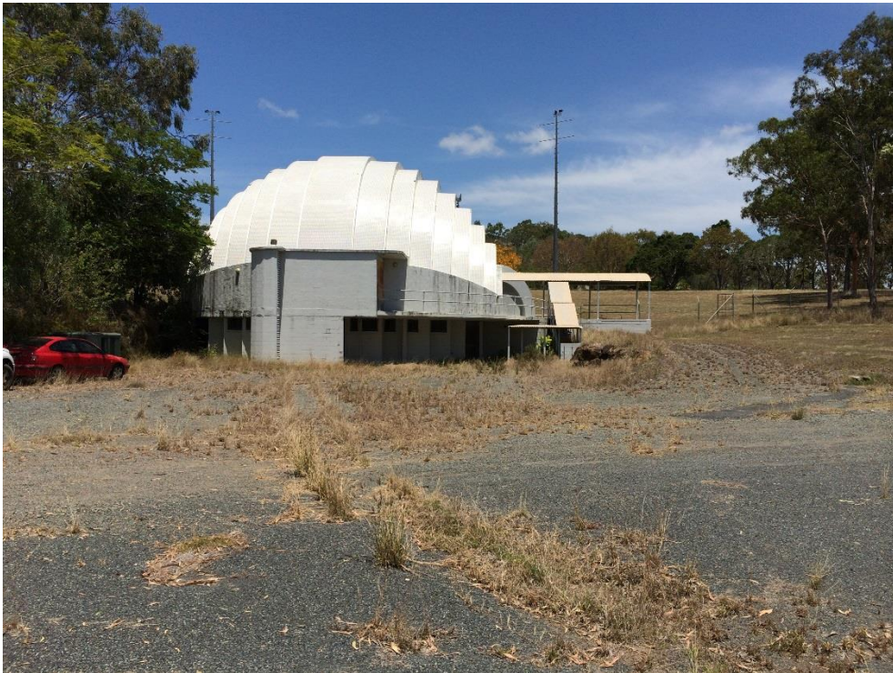
Photo 231 - Rear of sound shell and loading area
