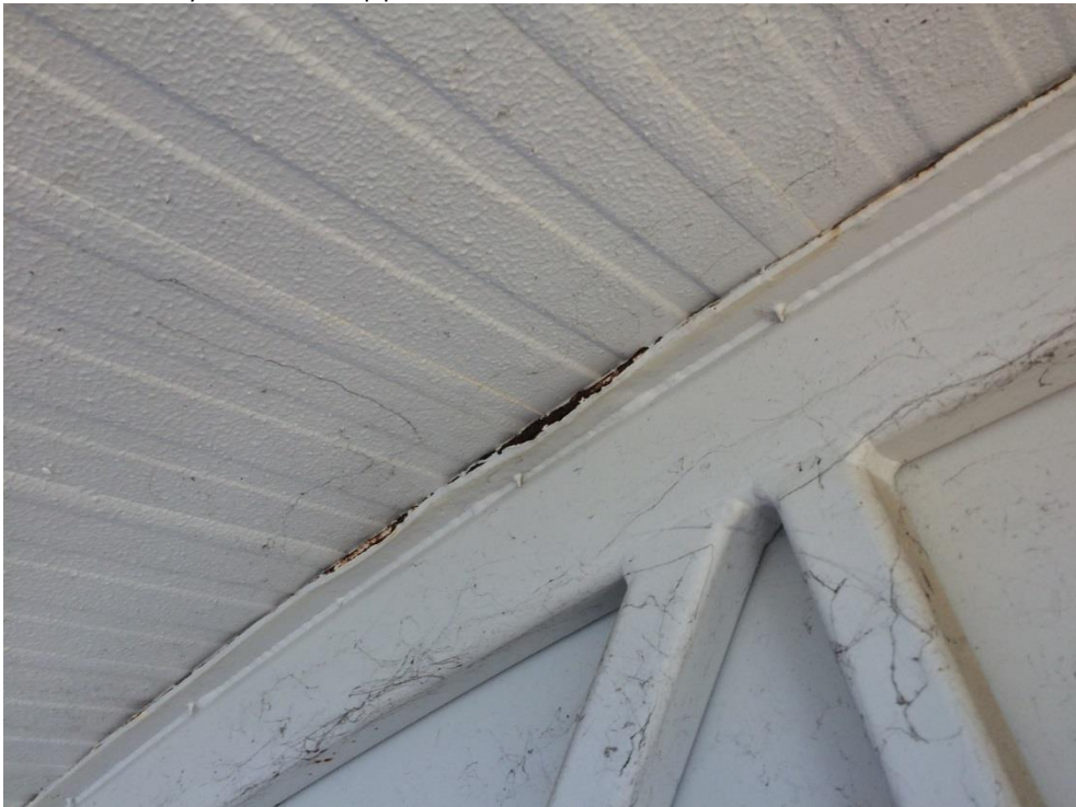
Photo 042 - Heavy corrosion to top plate
