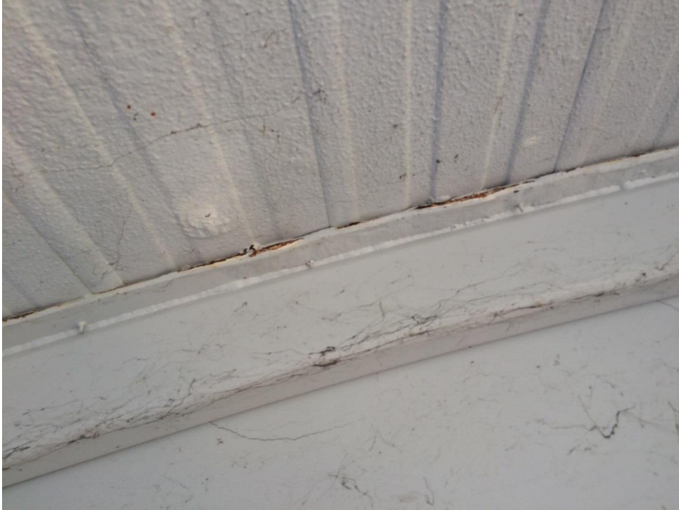
Photo 041 - Heavy corrosion to top plate
