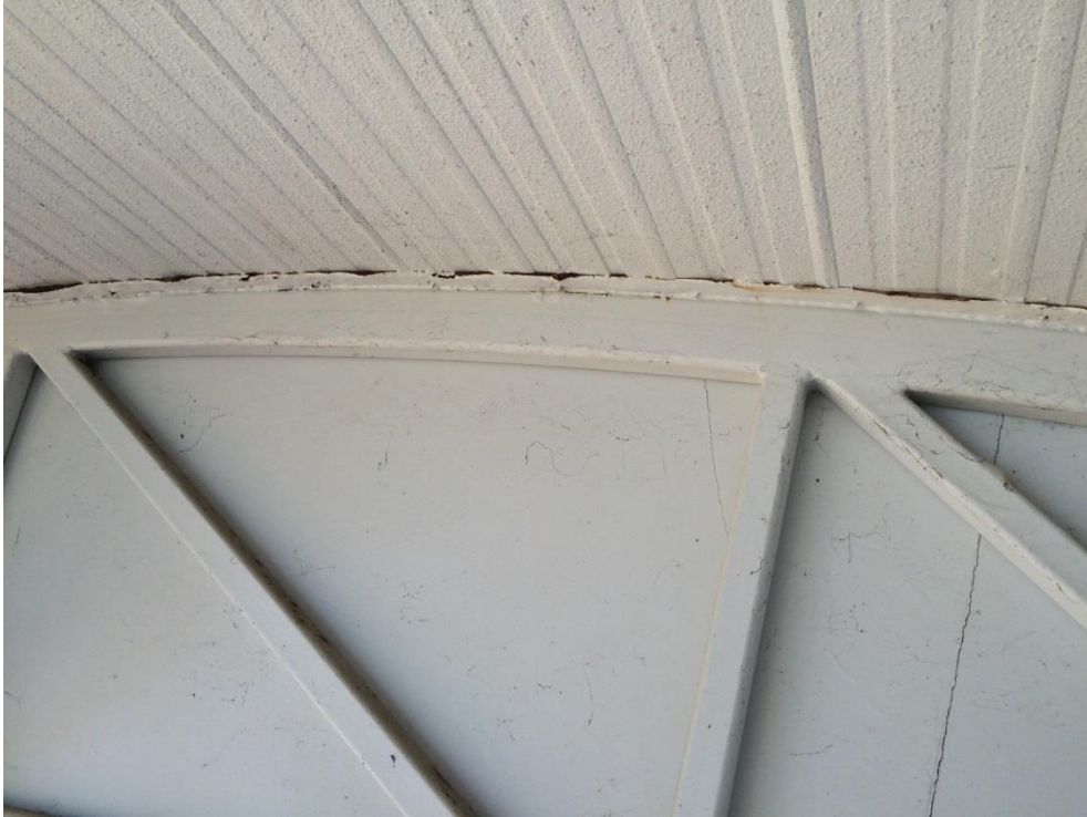
Photo 156 - Minor corrosion to top plate
