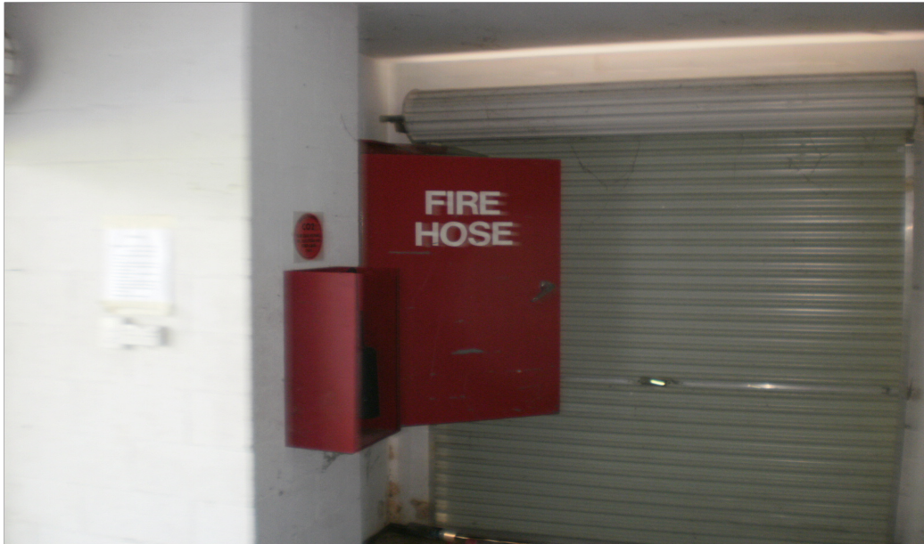
Door damaged on fire hose cabinet (photo 23)
