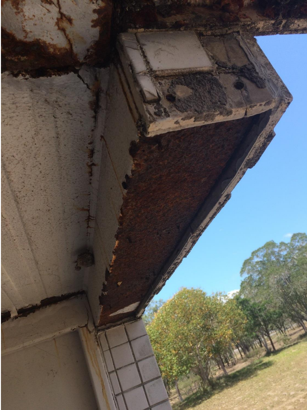
Photo 075 - Heavy corrosion to steel fascia
