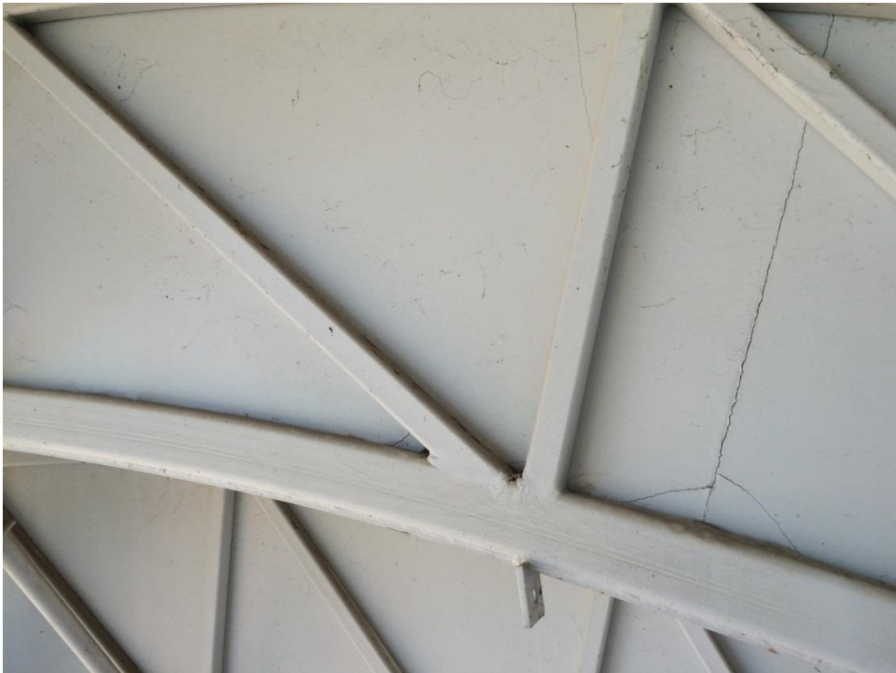
Photo 161 - Minor corrosion to bottom chord
