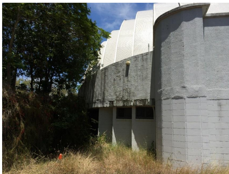
Figure 15 - Rear view of substructure
