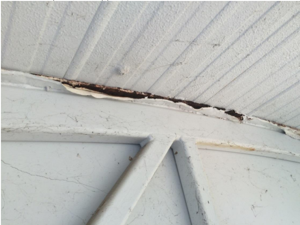
Photo 040 - Heavy corrosion to top plate
