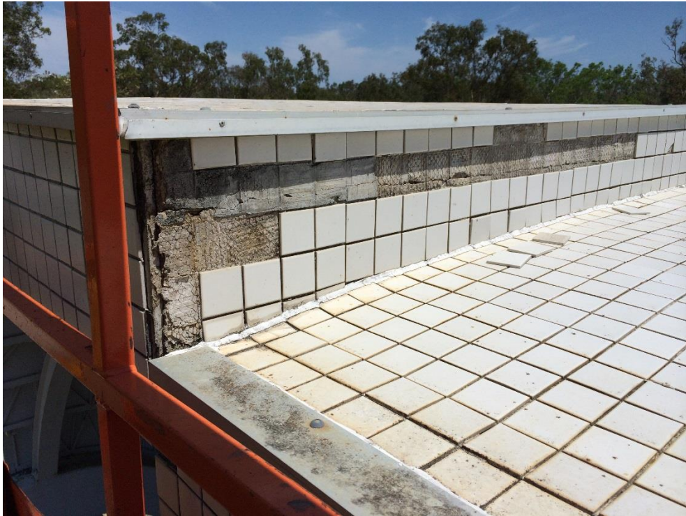
Photo 204 - Tiles missing from vertical surface, aluminium edge capping, evidence of water staining adjacent edge capping
