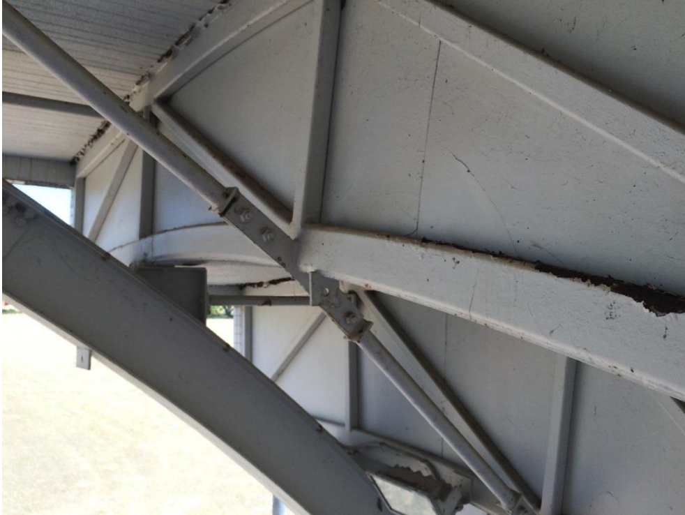
Photo 150 - Heavy corrosion to bottom chord
