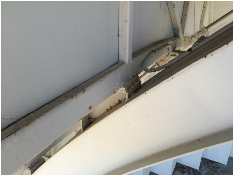
Photo 179 - Minor corrosion to bottom chord of truss
