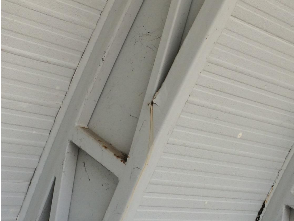
Photo 116 - Heavy corrosion to truss bottom chord, paint peeling off
