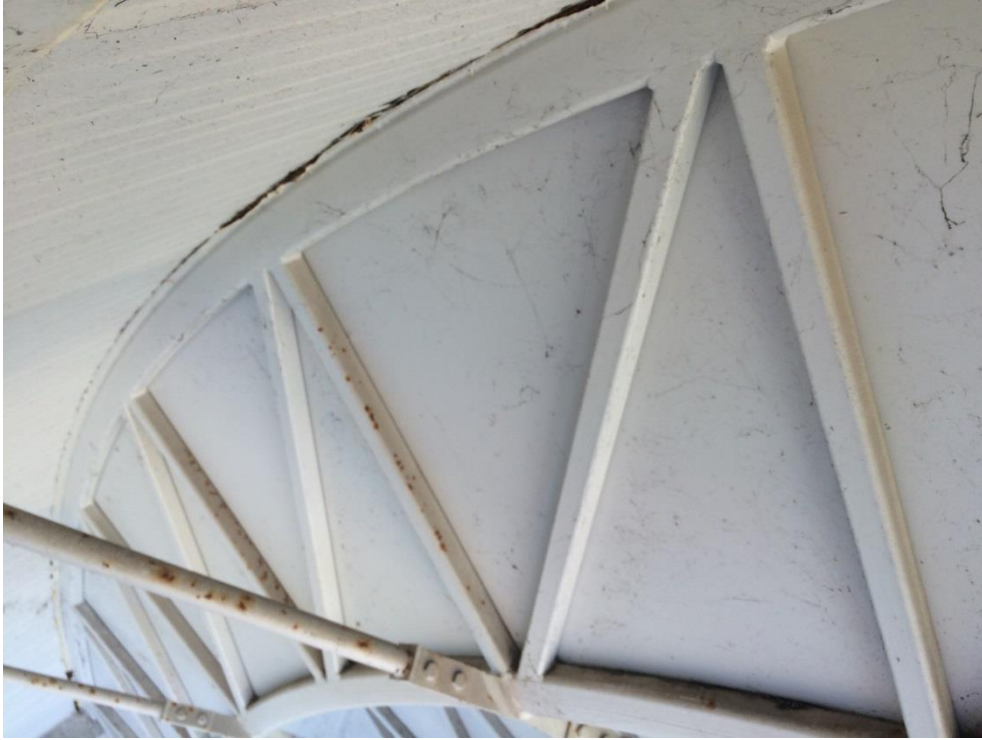
Photo 033 - Minor corrosion to struts
