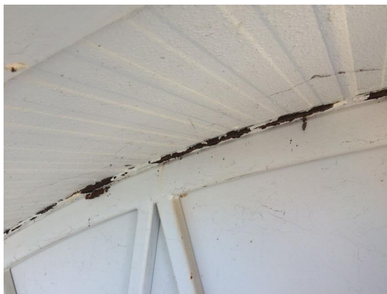
Figure 10 - Corrosion of top plate
