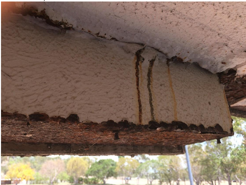
Photo 096 - Heavy corrosion to fascia
