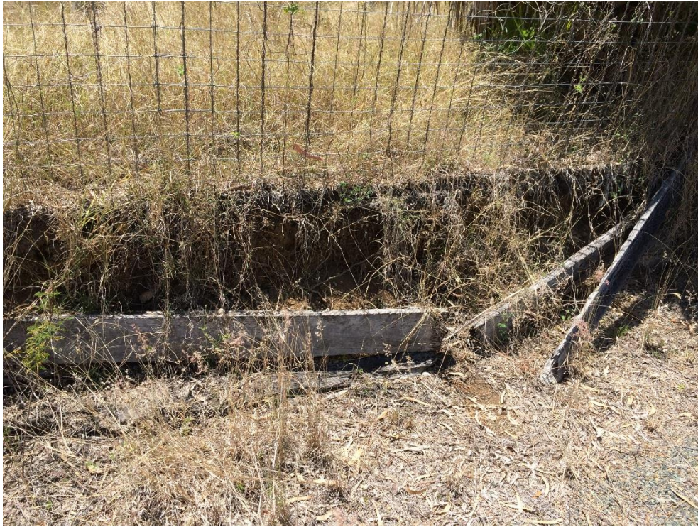
Photo 224 - Timber retaining wall, rotted and collapsed
