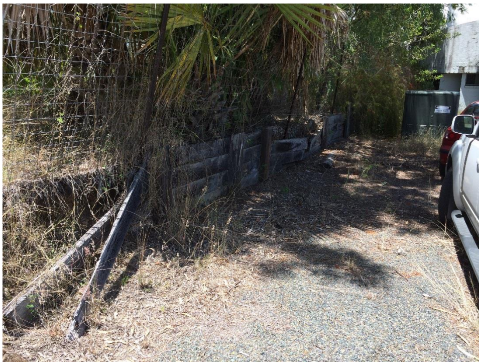
Figure 24- Timber retaining wall
