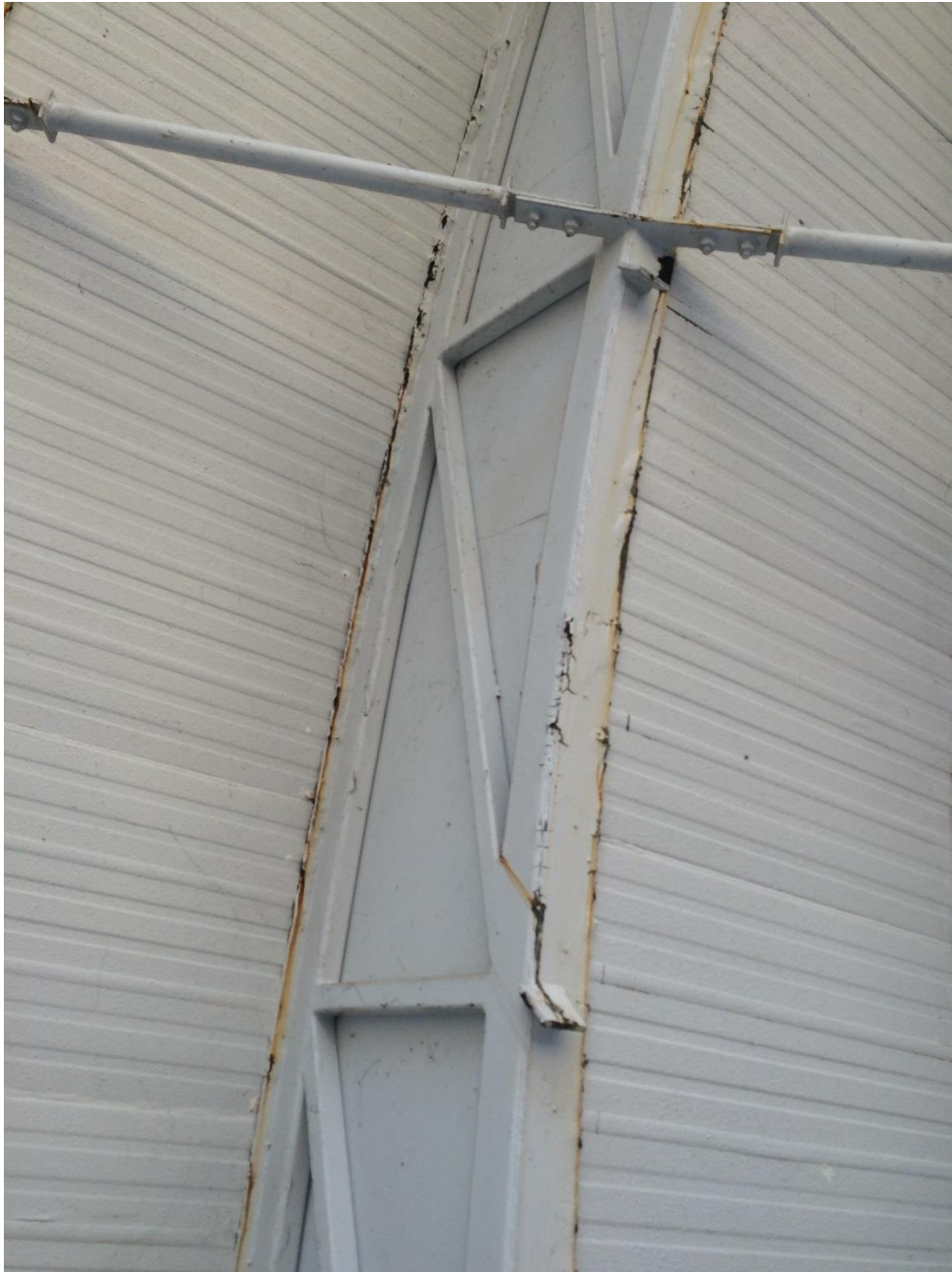
Photo 122 - Minor corrosion to truss top and bottom plate
