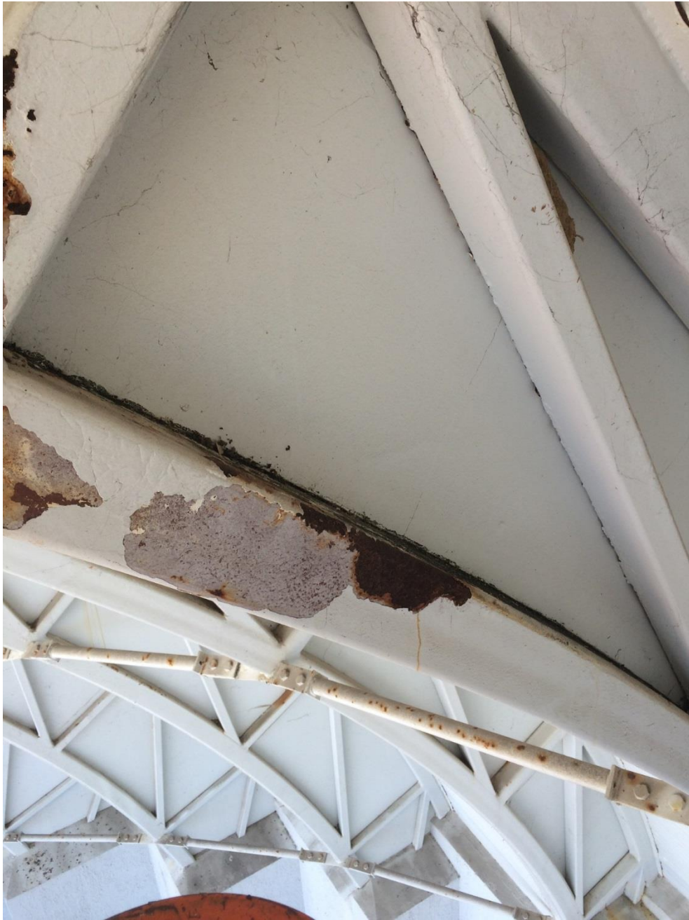
Photo 133 - Minor corrosion to bottom chord
