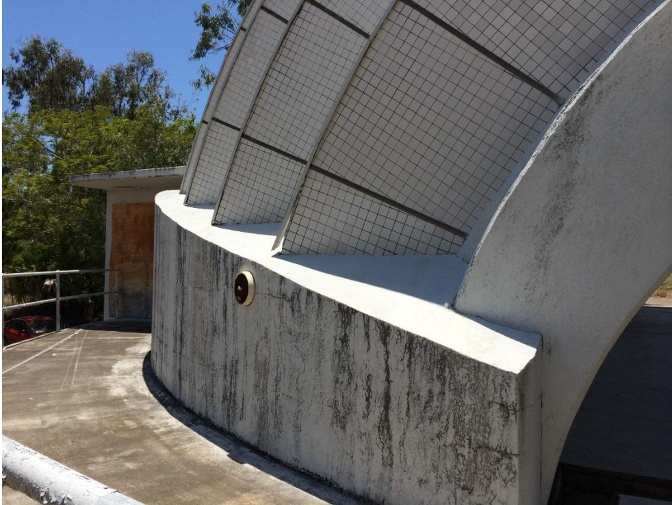
Photo 212 - Rear lower surface of sound shell meeting blockwork plinth. Aluminium capping coming loose
