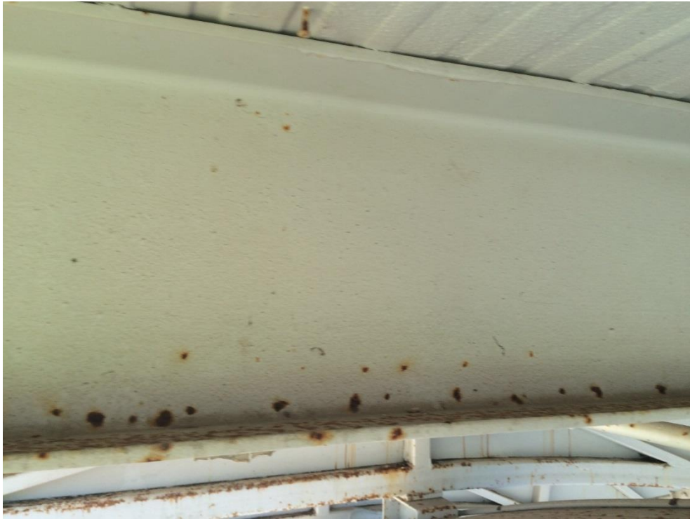
Photo 200 - Minor corrosion to roof beam
