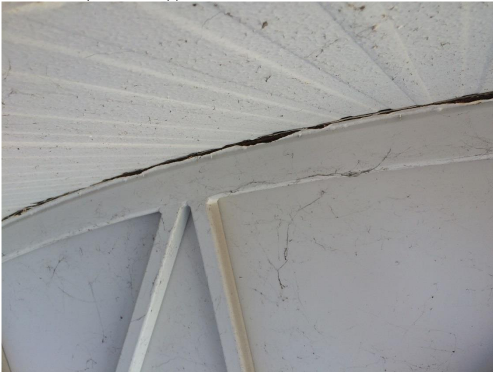
Photo 032 - Heavy corrosion to top plate
