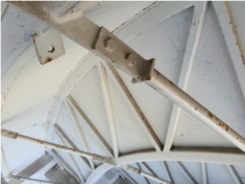
Photo 034 - Minor corrosion to struts
