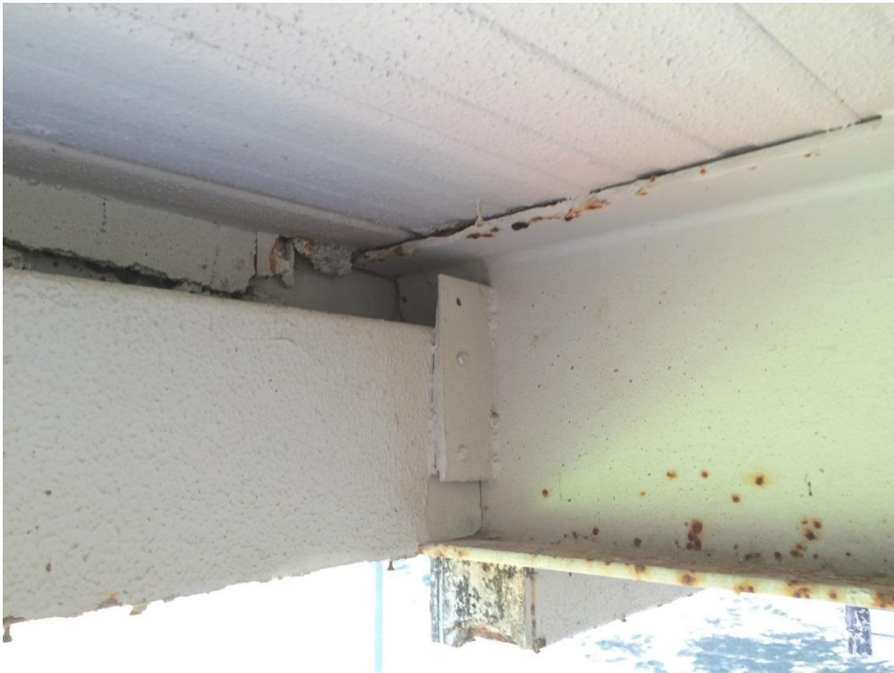
Photo 197 - Minor corrosion to roof beam
