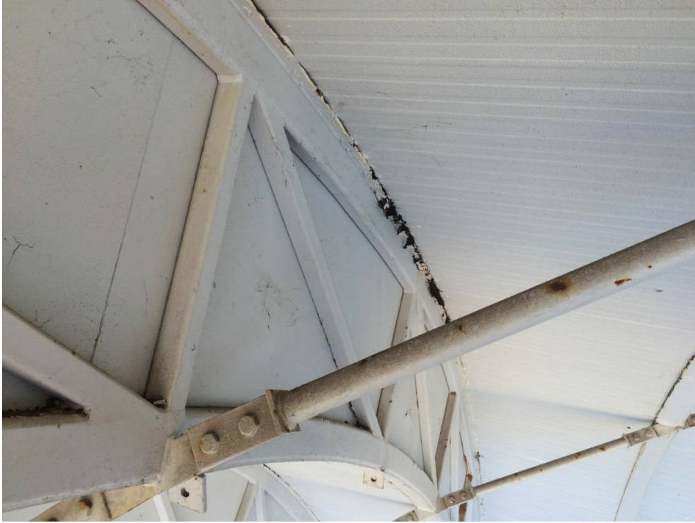
Photo 146 - Heavy corrosion to top plate
