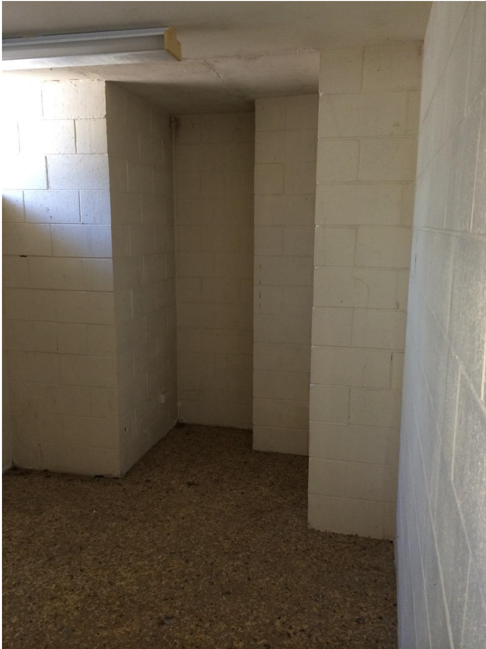
Photo 245 - Lower ground floor corridor
