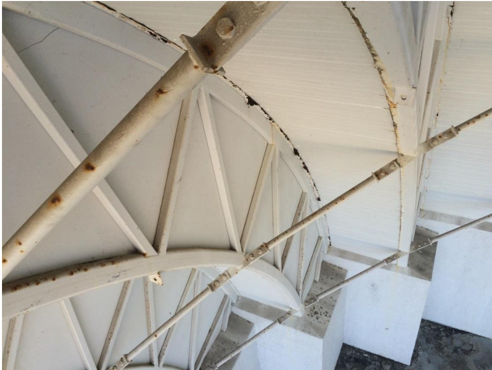
Photo 168 - Minor corrosion to bottom plate and top plate
