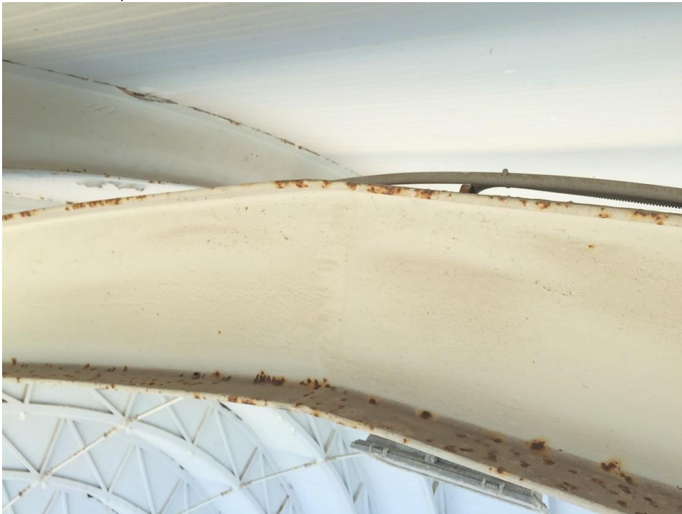
Photo 106 - Minor corrosion to main arch
