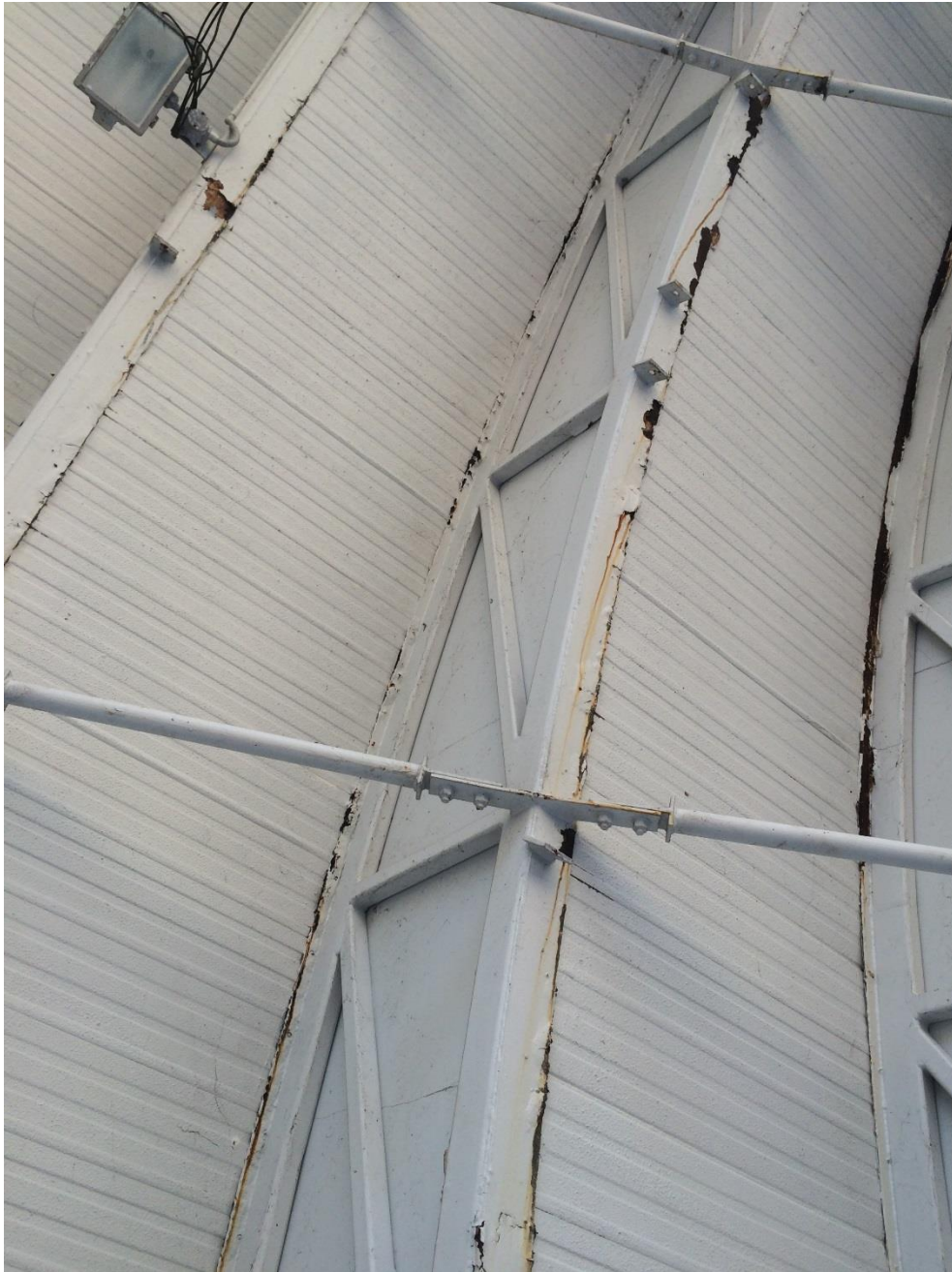
Photo 123 - Minor corrosion to truss top and bottom plate
