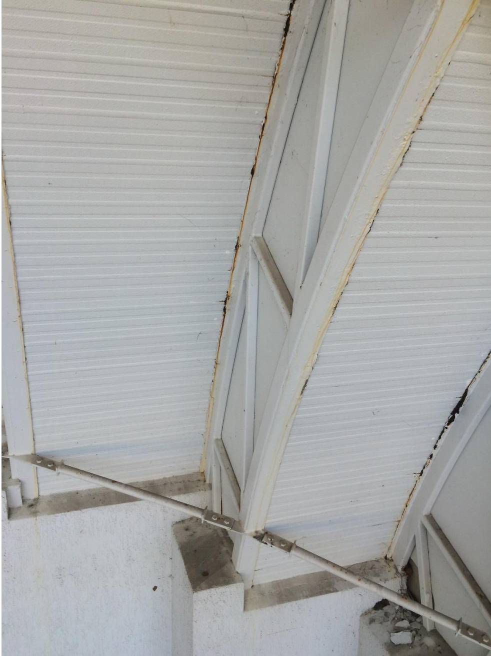
Photo 119 - Minor corrosion to truss top and bottom plate
