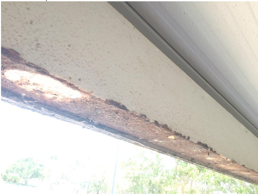
Photo 104 - Heavy corrosion to fascia
