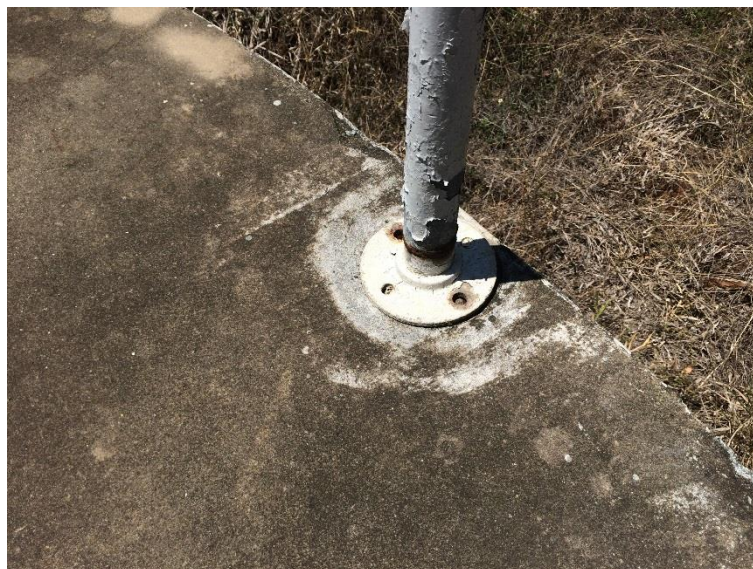
Figure 22 - Bolts missing from stanchions
