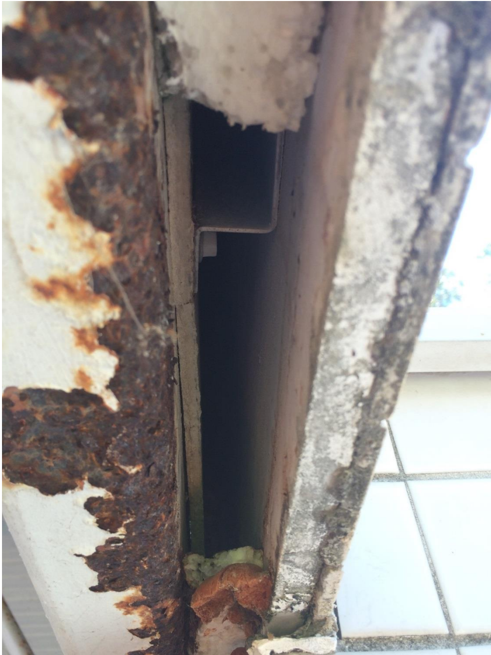
Photo 020 - Heavy corrosion to bottom chord
