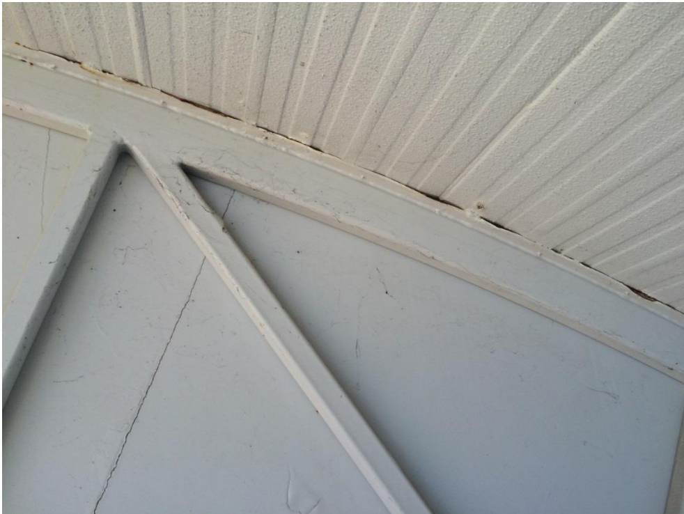
Photo 157 - Minor corrosion to top plate
