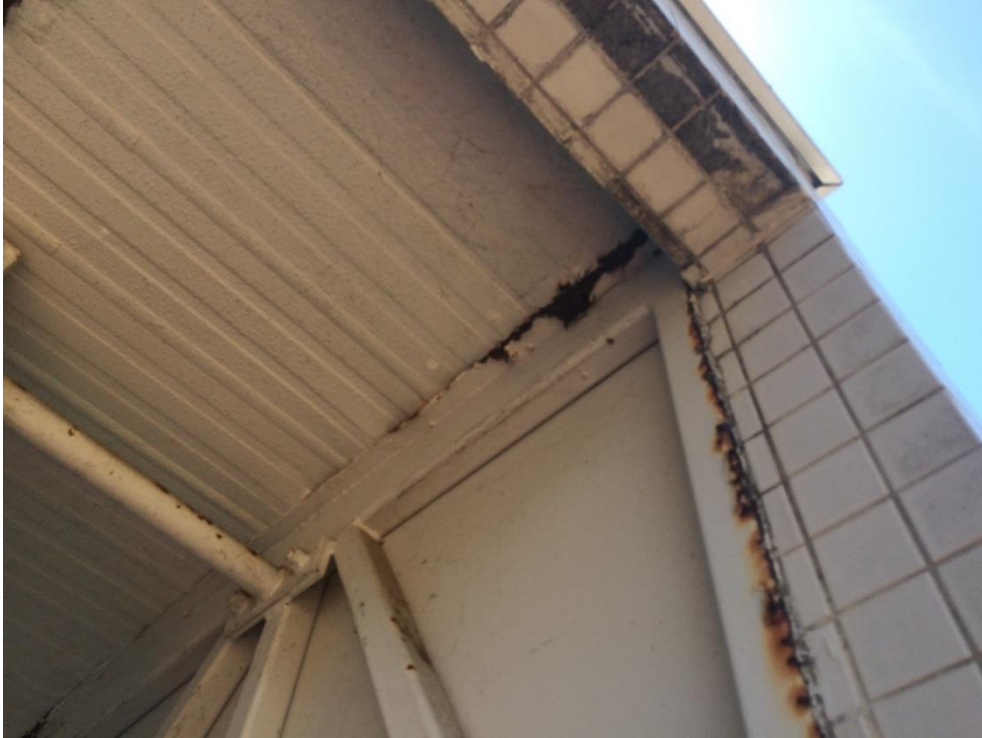
Photo 010 - Corrosion to truss bottom chord and web at end
