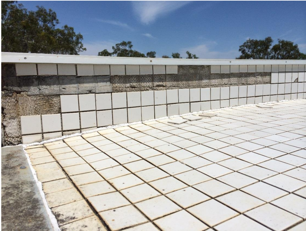
Photo 206 - Tiles missing from vertical surfaces, Horizontal tiled surface at top of sound shell. Evidence of water ponding on horizontal surface
