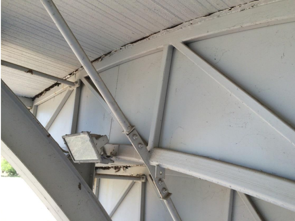
Photo 154 - Minor corrosion to top plate
