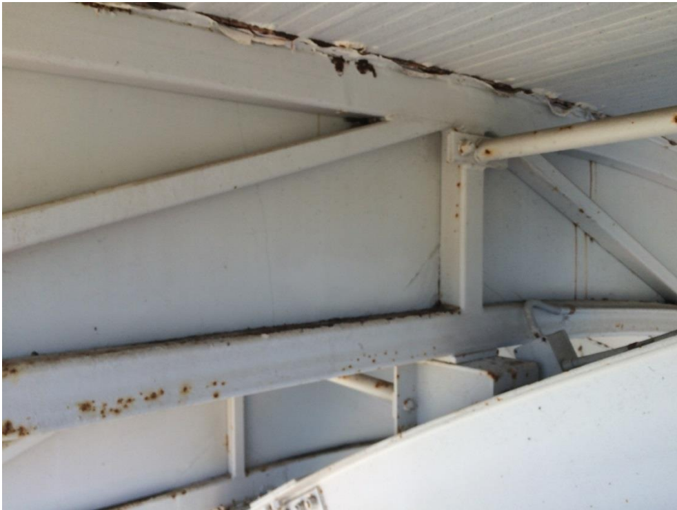
Photo 189 - Minor corrosion to bottom chord
