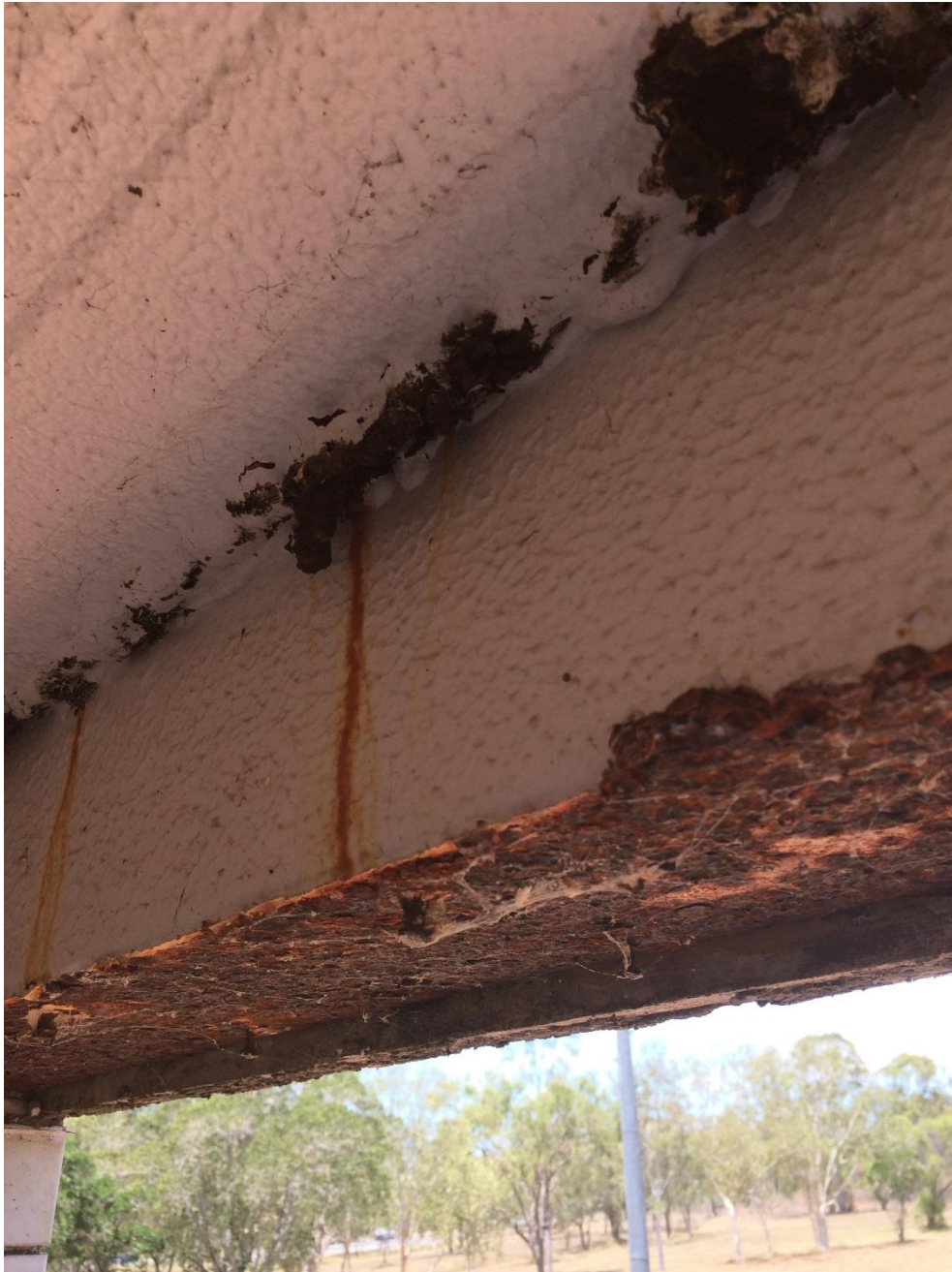
Photo 092 - Heavy corrosion to fascia
