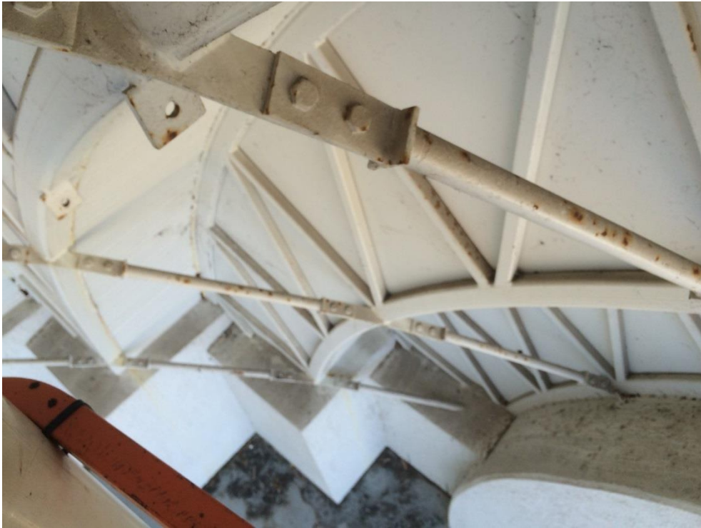
Photo 035 - Minor corrosion to struts
