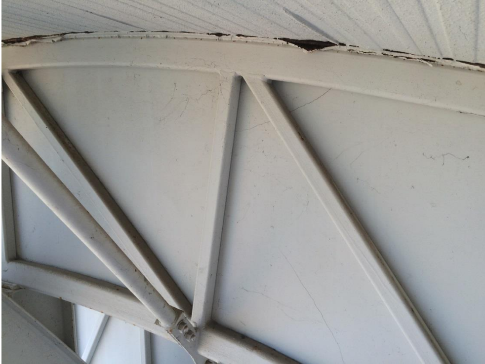
Photo 164 - Minor corrosion to top plate
