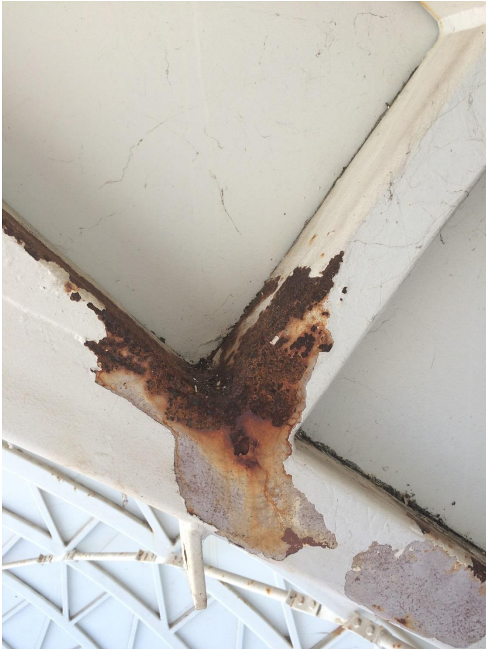
Photo 132 - Minor corrosion to bottom chord and web of truss
