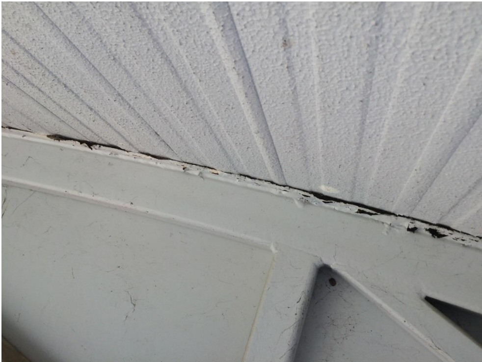
Photo 143 - Minor corrosion to top plate
