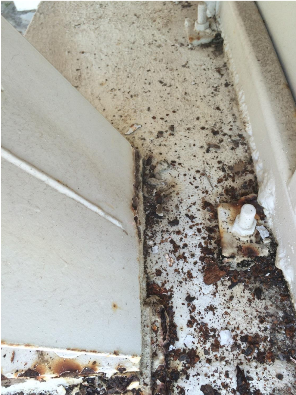
Photo 014 - Minor corrosion to main arch top flange at baseplate
