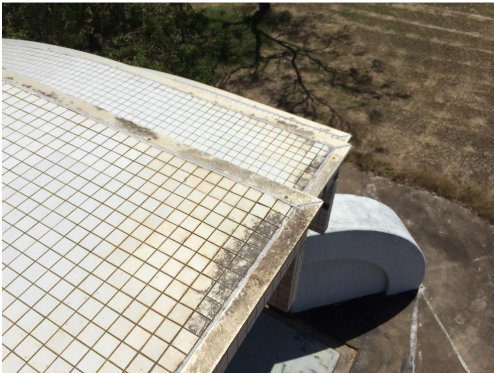
Photo 207 - Horizontal tiled surface with aluminium edge capping. Evidence of water ponding
