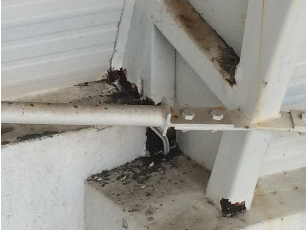
Photo 114 - Heavy corrosion to truss at concrete interface, heavy corrosion to inside corner of tie
