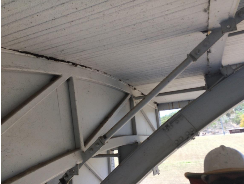
Photo 055 - Heavy corrosion to top plate
