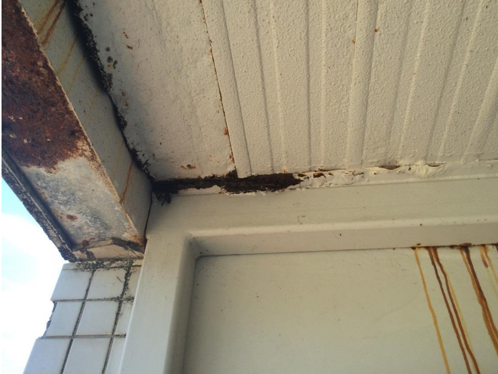
Photo 192 - Heavy corrosion to top plate, minor corrosion to metal formwork, heavy corrosion to fascia
