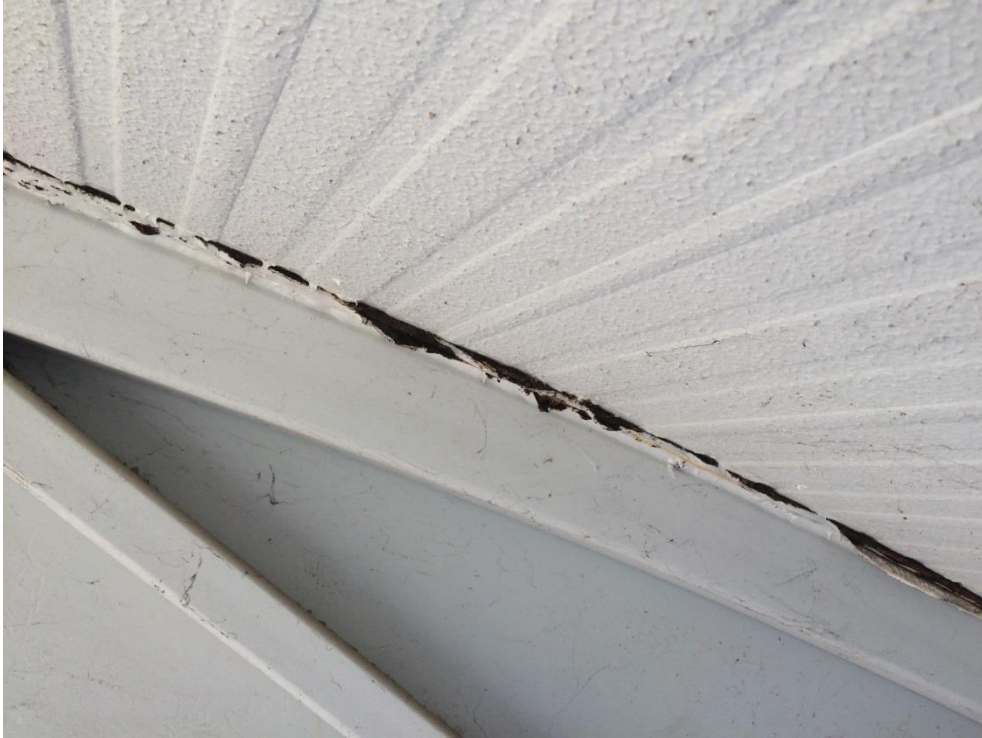
Photo 144 - Minor corrosion to top plate
