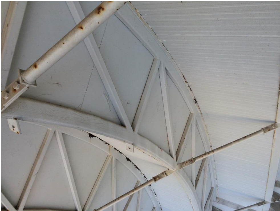
Photo 159 - Minor corrosion to top plate
