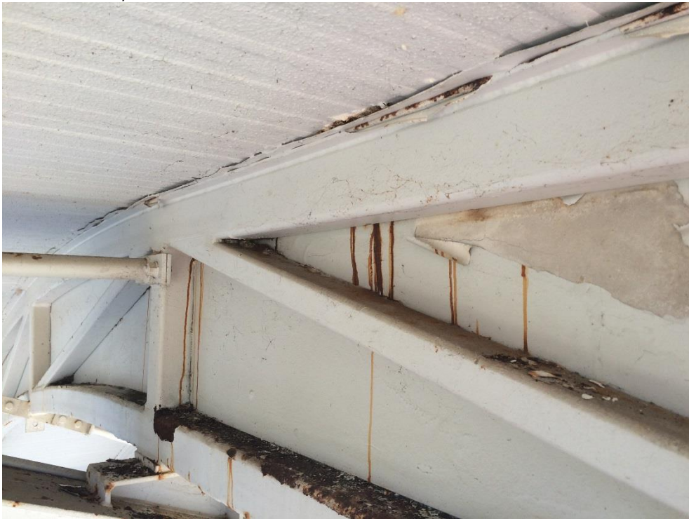
Photo 086 - Heavy corrosion to truss bottom chord
