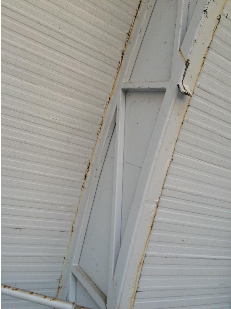
Photo 121 - Minor corrosion to truss top and bottom plate
