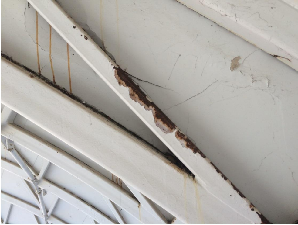
Photo 134 - Minor corrosion to web of truss
