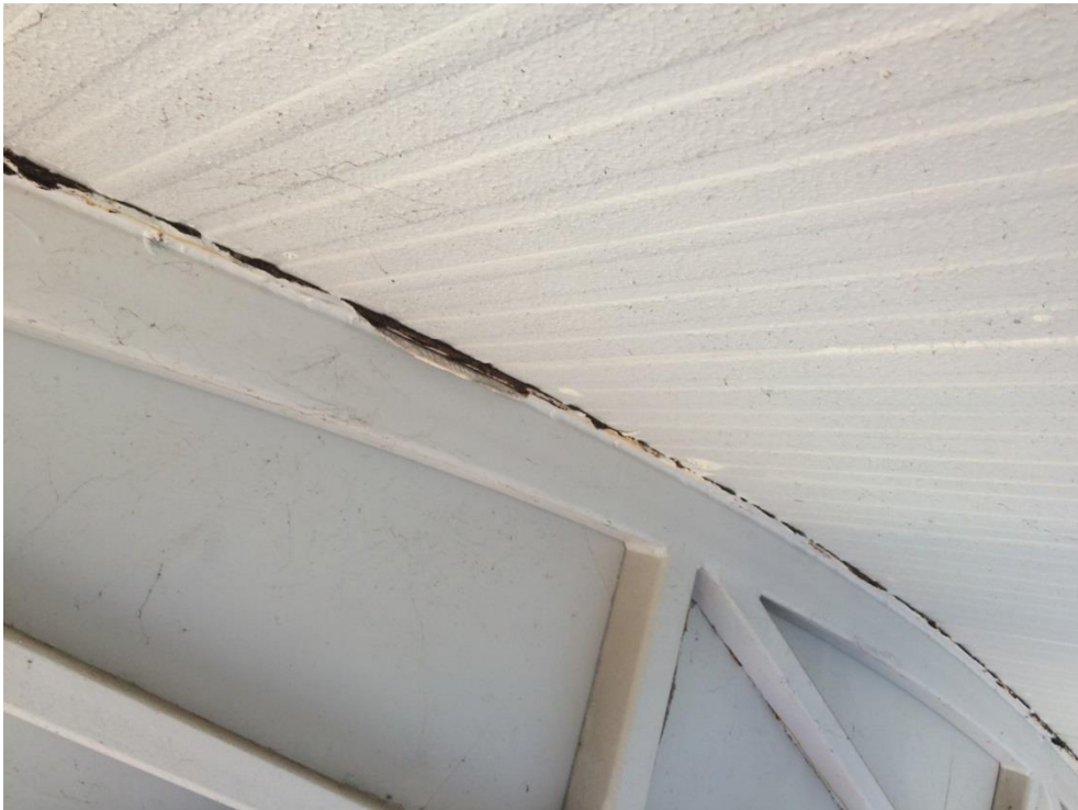
Photo 145 - Minor corrosion to top plate
