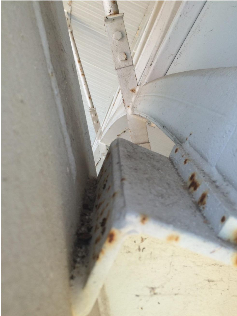
Photo 017 - Minor corrosion in corner of stub
