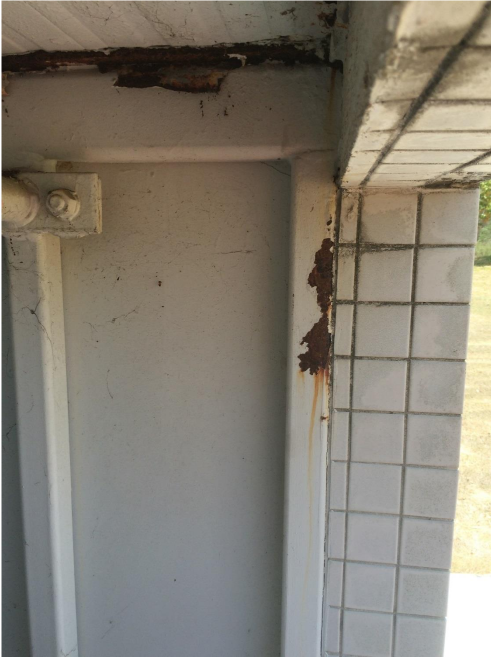
Photo 001 - Corrosion to truss web at end
