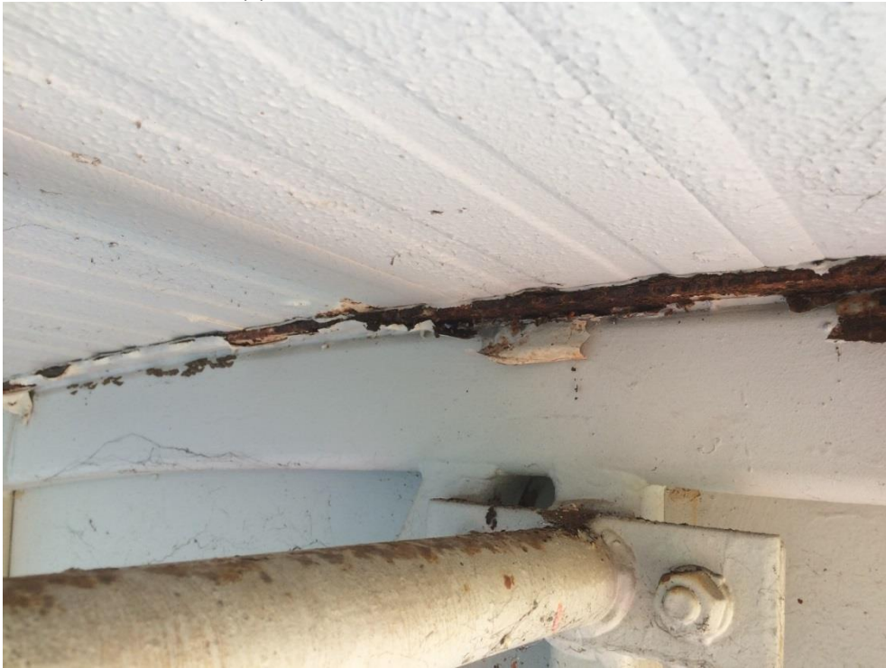
Photo 004 - Corrosion to top plate
