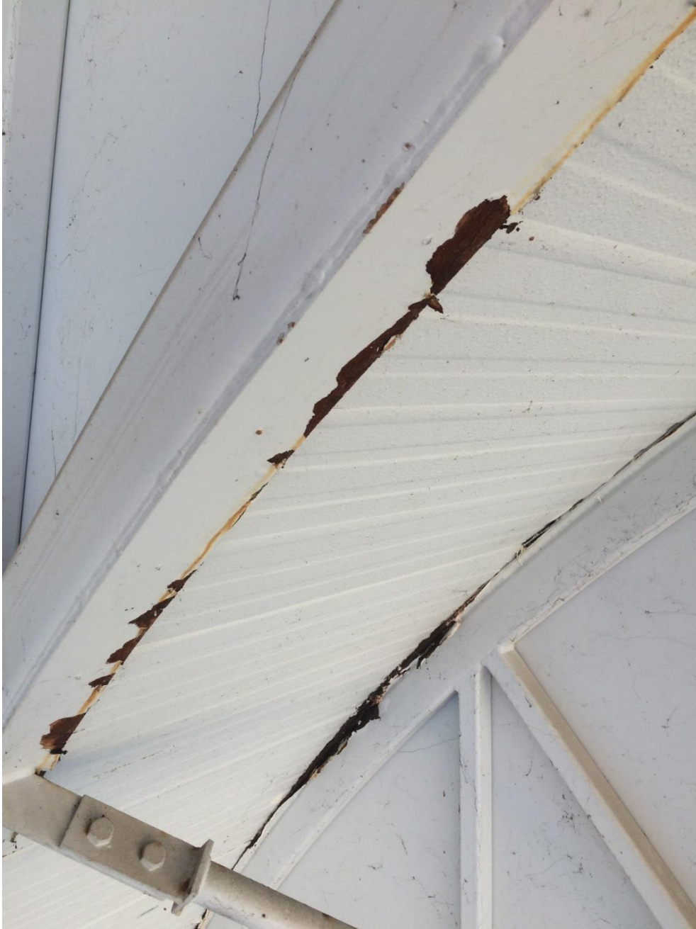
Photo 052 - Minor corrosion to bottom plate
