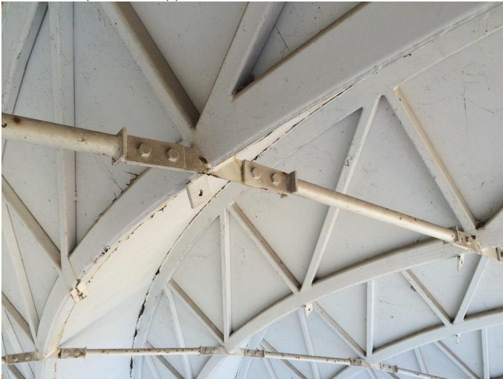
Photo 060 - Minor corrosion to bottom plate
