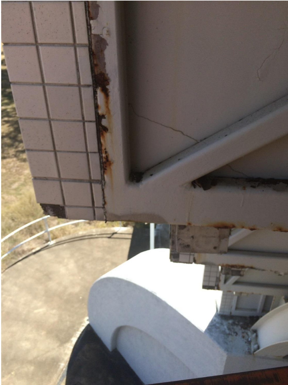
Photo 185 - Heavy corrosion to end web of truss
