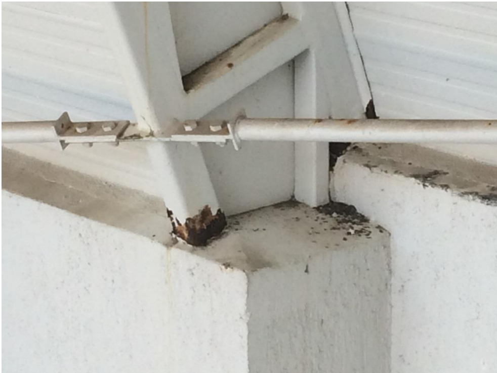
Photo 131 - Heavy corrosion to bottom chord of truss at concrete interface
