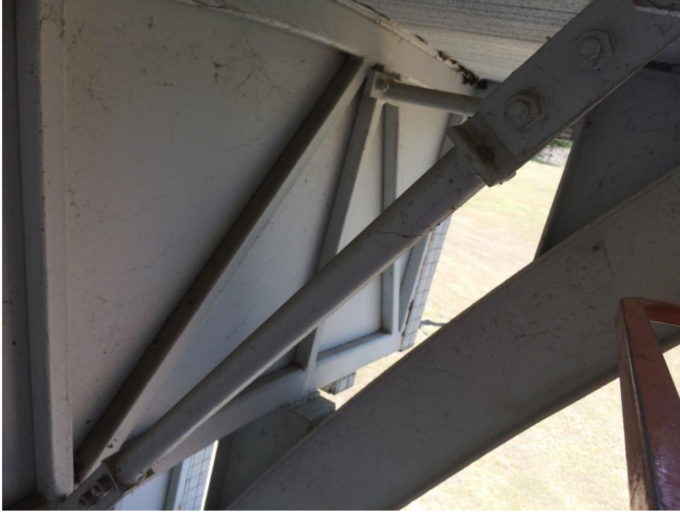
Photo 037 - Minor corrosion to struts
