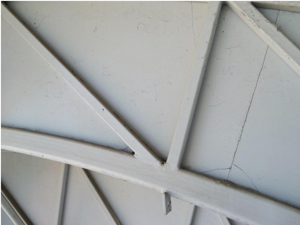
Photo 155 - Minor corrosion to bottom chord
