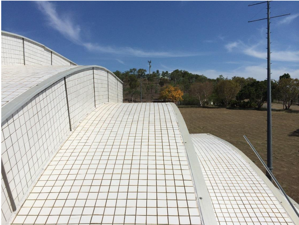
Photo 220 - Loose aluminium capping on rear of sound shell
