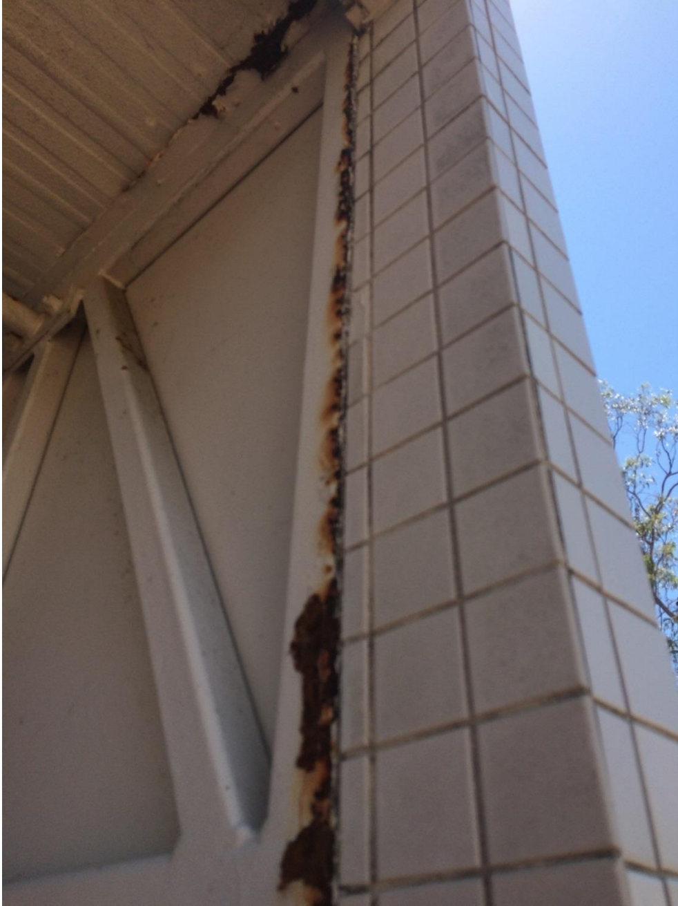
Photo 009 - Corrosion to truss bottom chord and web at end
