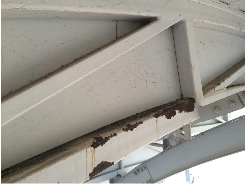
Photo 107 - Minor corrosion to bottom chord
