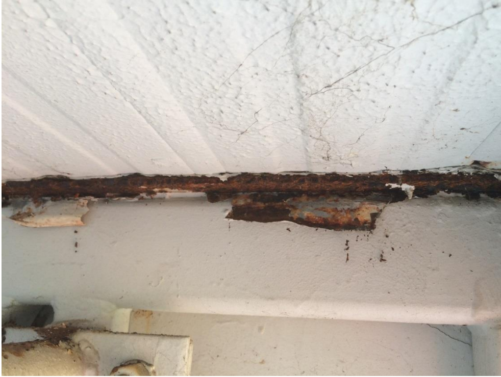
Photo 003 - Corrosion to top plate
