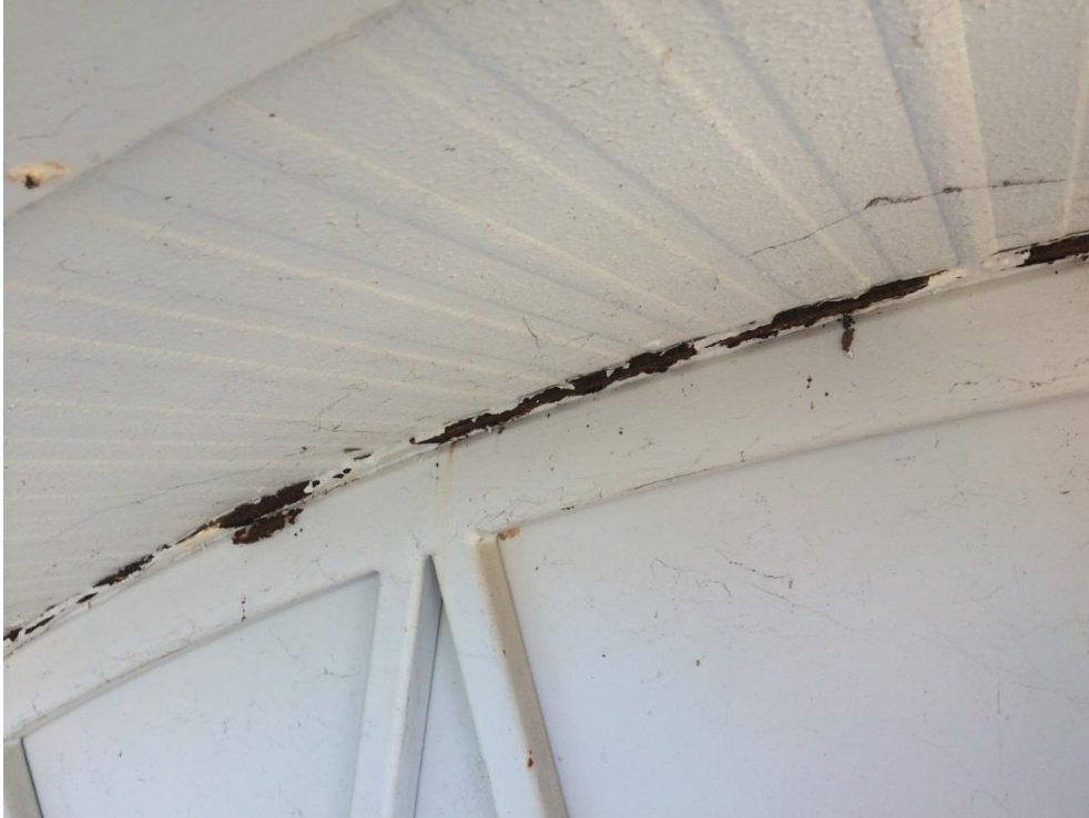
Photo 023 - Heavy corrosion to top plate all along
