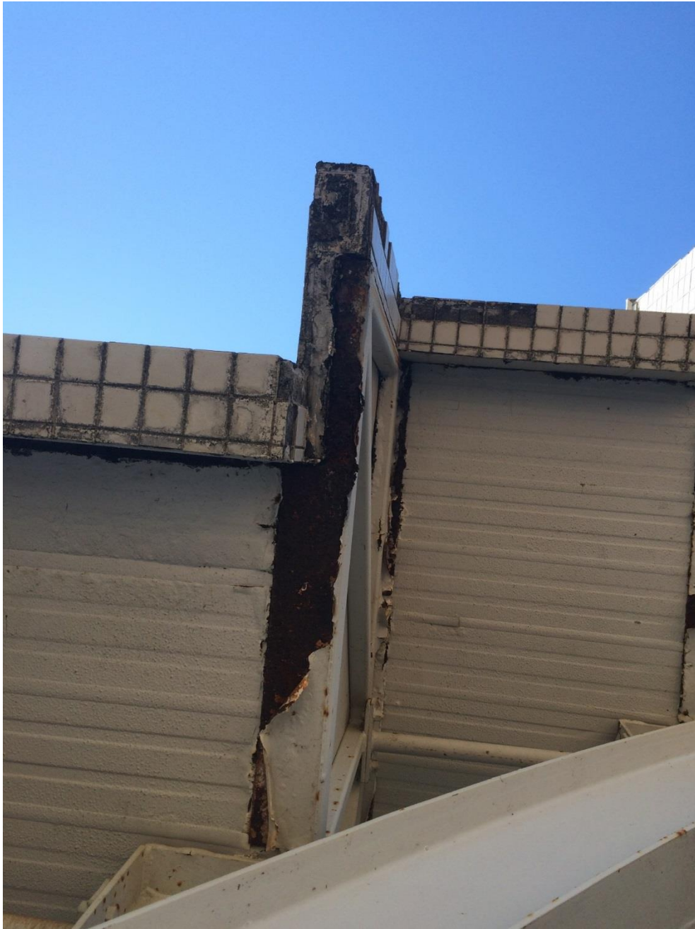
Photo 177 - Heavy corrosion to end web of truss
