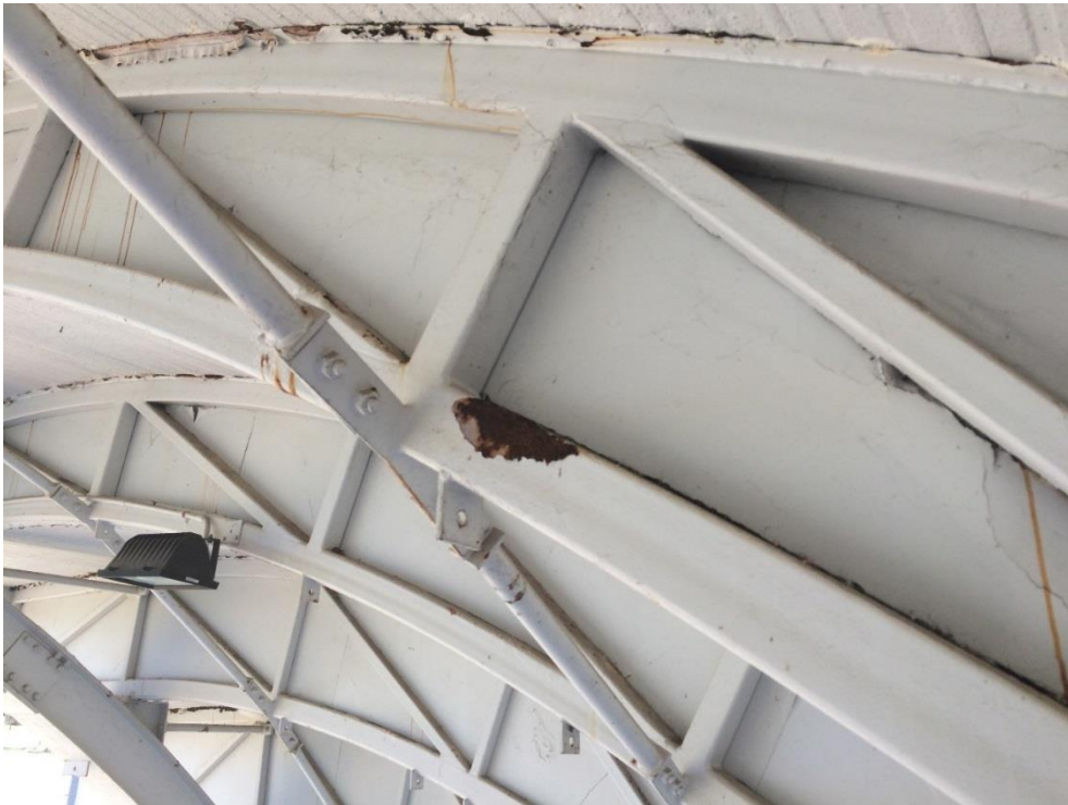
Photo 135 - Minor corrosion to bottom chord
