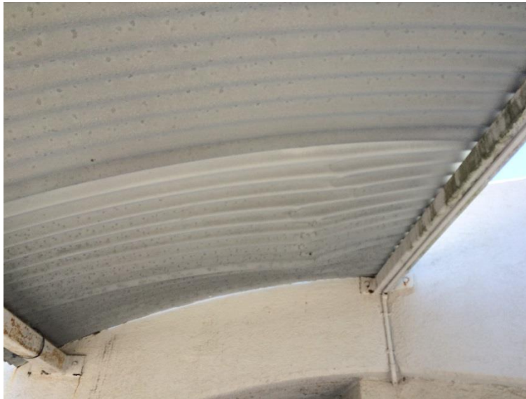
Figure 19 - Dent in roof sheeting
