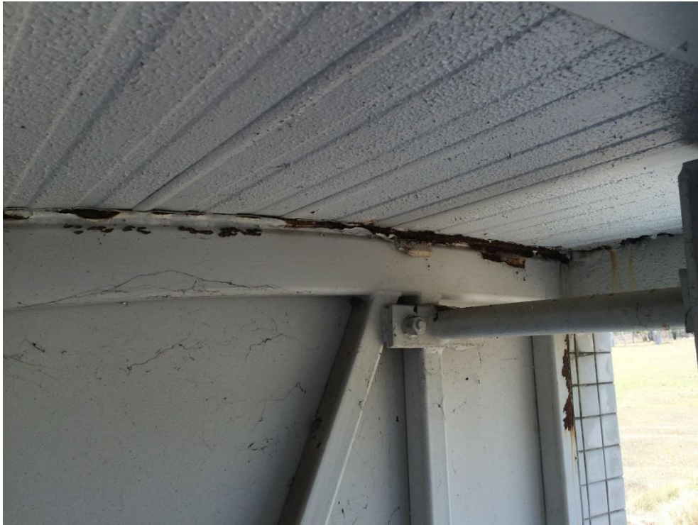
Photo 021 - Heavy corrosion to top plate all along
