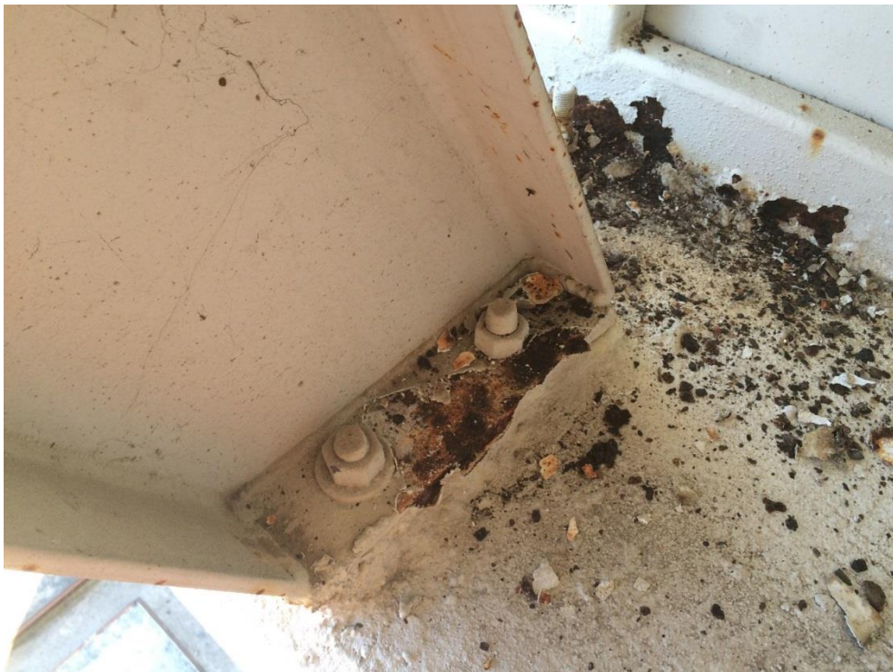
Photo 175 - Minor corrosion to main arch base plate
