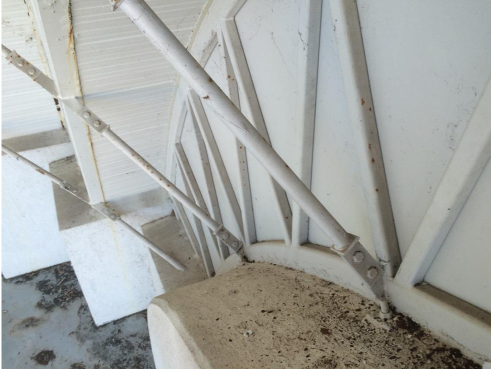
Photo 029 - Heavy corrosion to side of bottom chord
