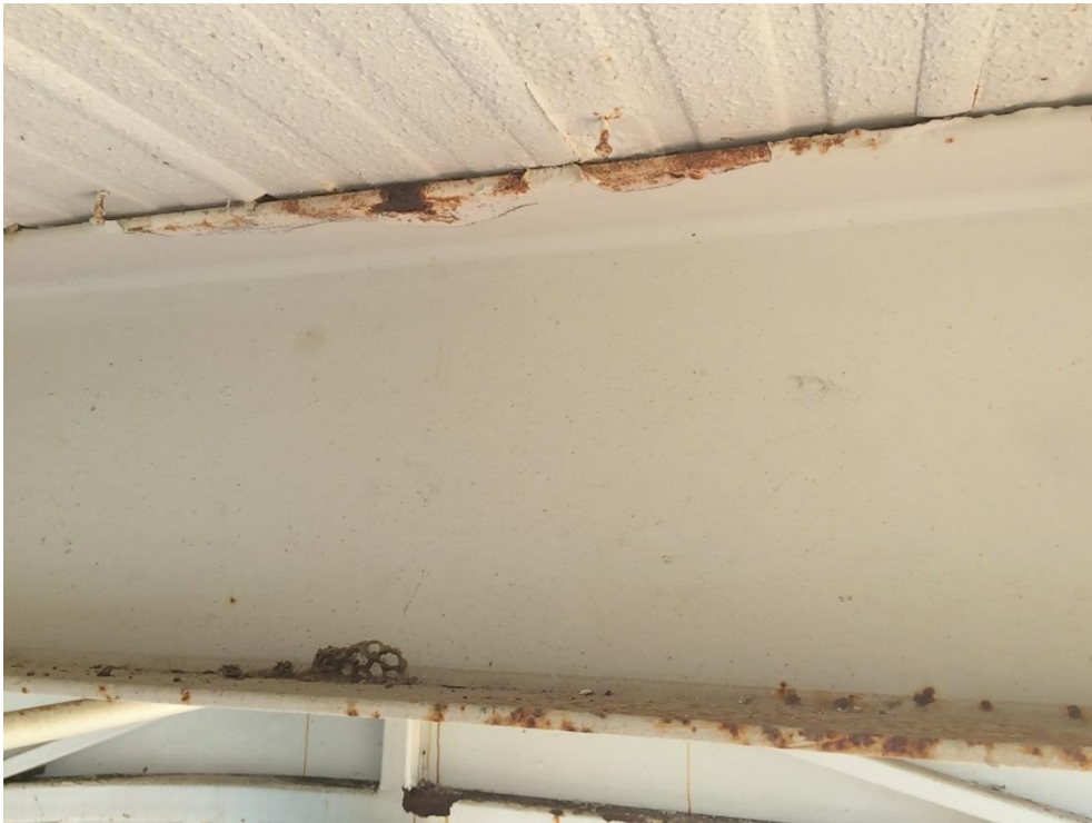
Photo 100 - Minor corrosion to roof beam
