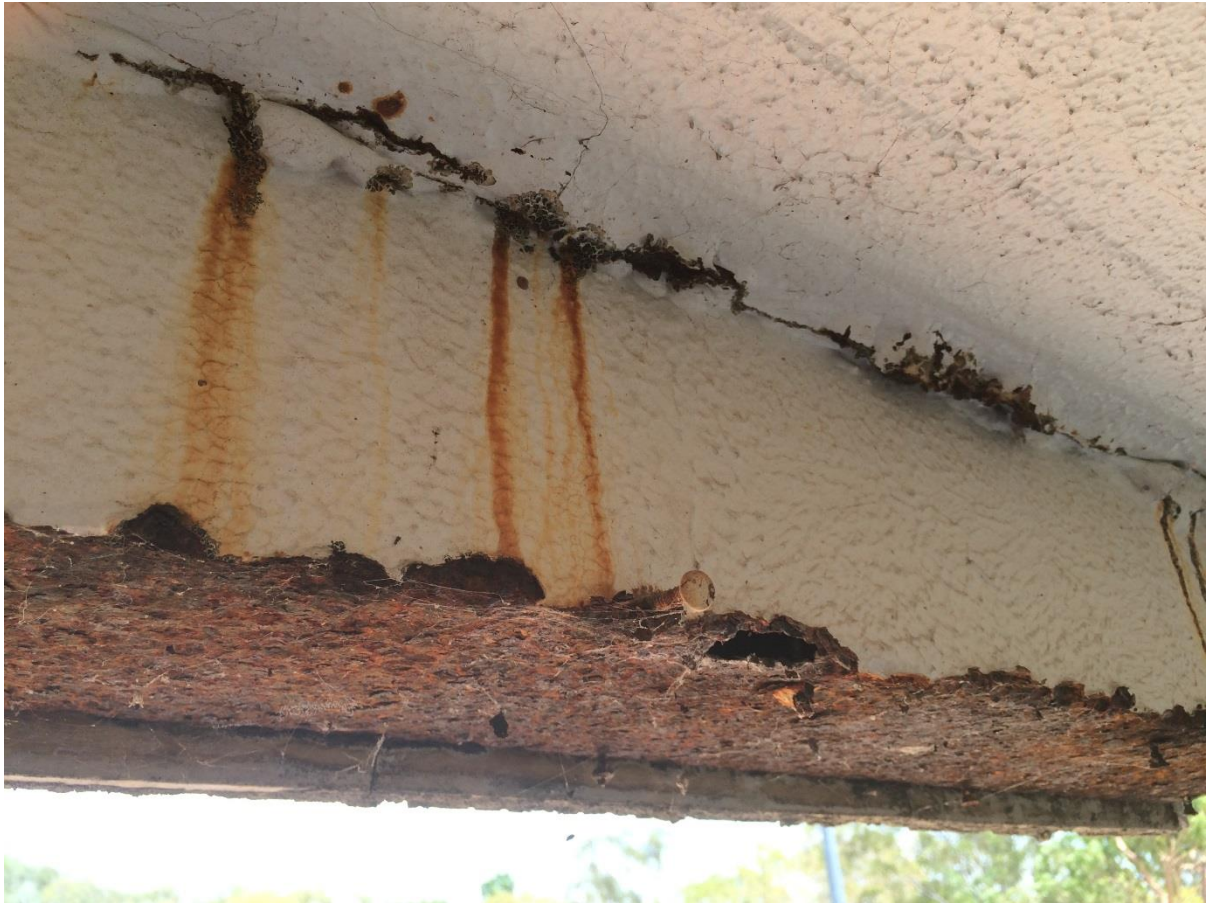
Photo 095 - Heavy corrosion to fascia
