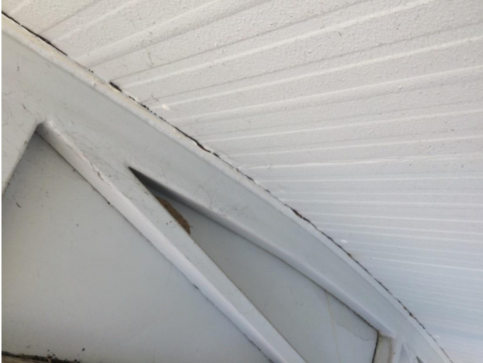
Photo 138 - Heavy corrosion to top plate
