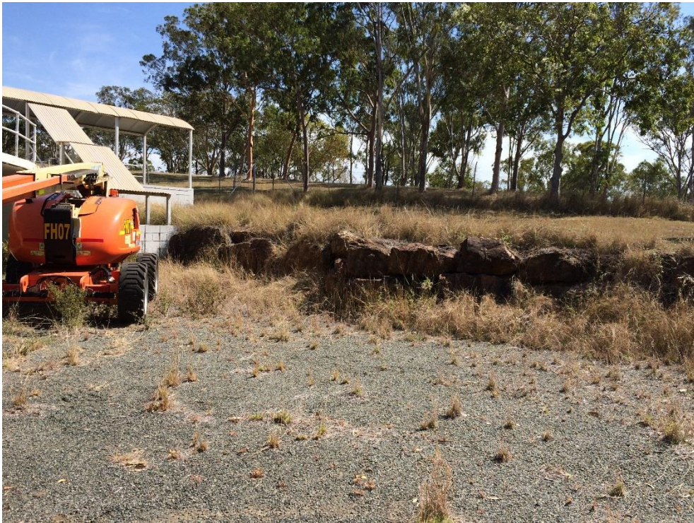
Photo 233 - Boulder wall to north west of sound shell
