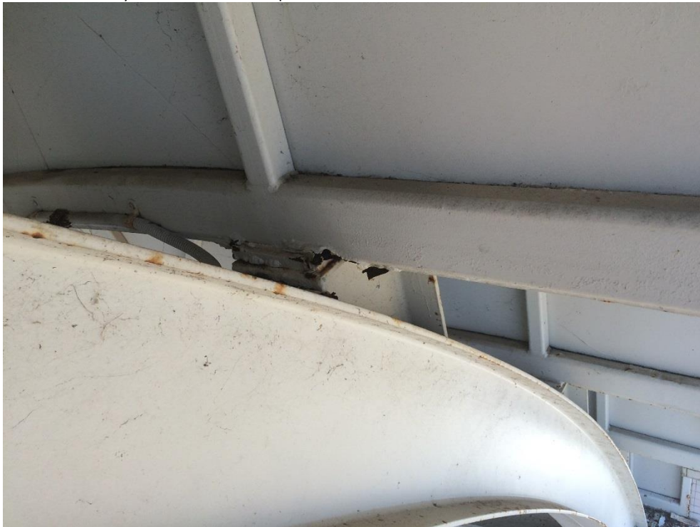
Photo 071 - Minor corrosion to stub
