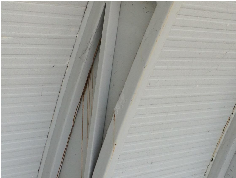
Photo 115 - Heavy corrosion to truss bottom chord, paint peeling off
