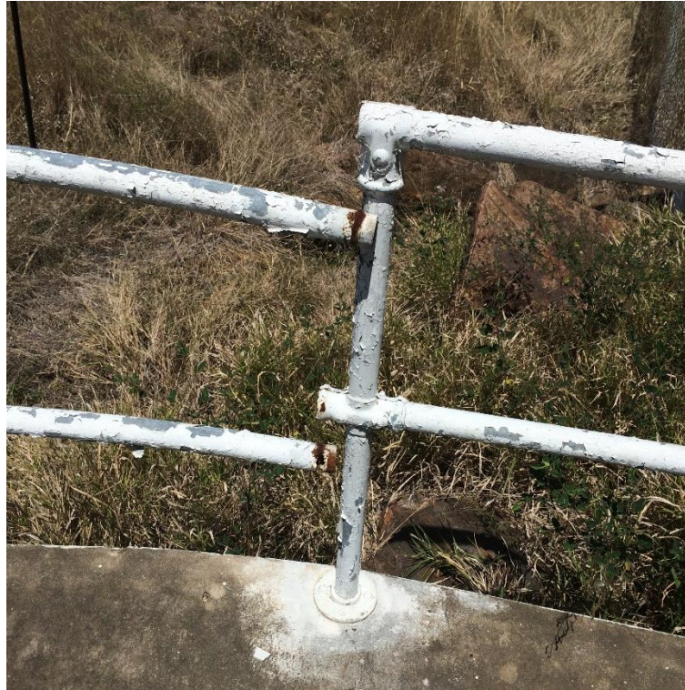
Figure 21 - Handrails disconnected from stanchions and coating deteriorated
