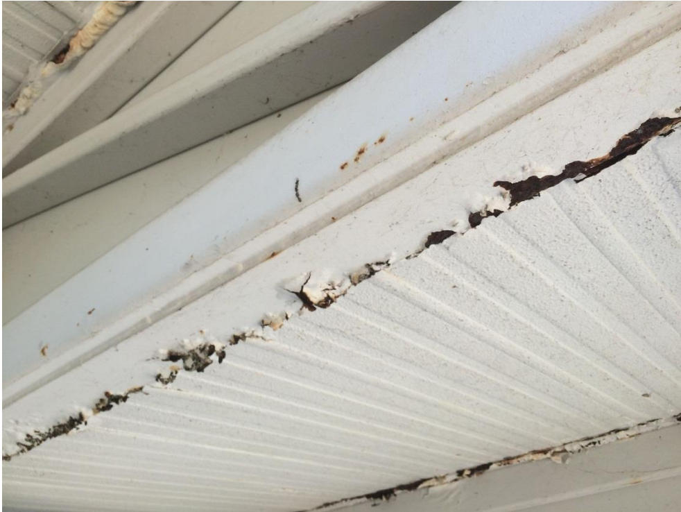
Photo 079 - Minor corrosion to bottom plate
