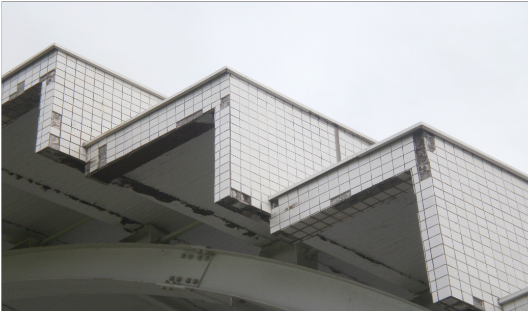
Missing tiles (photo 10)
