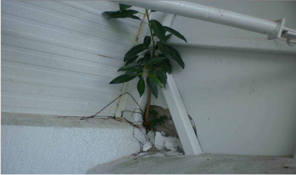
Tree growing in the building (photo 7)
