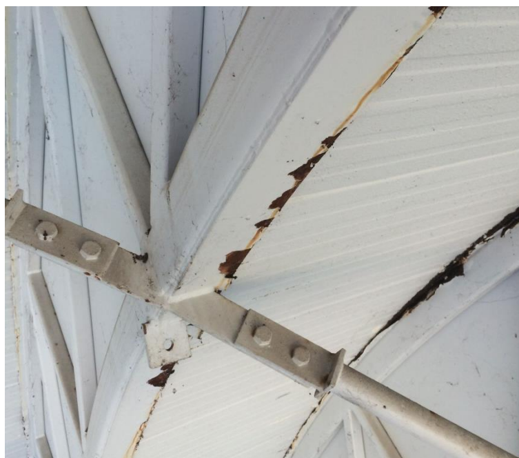
Figure 11 - Corrosion of bottom plate
