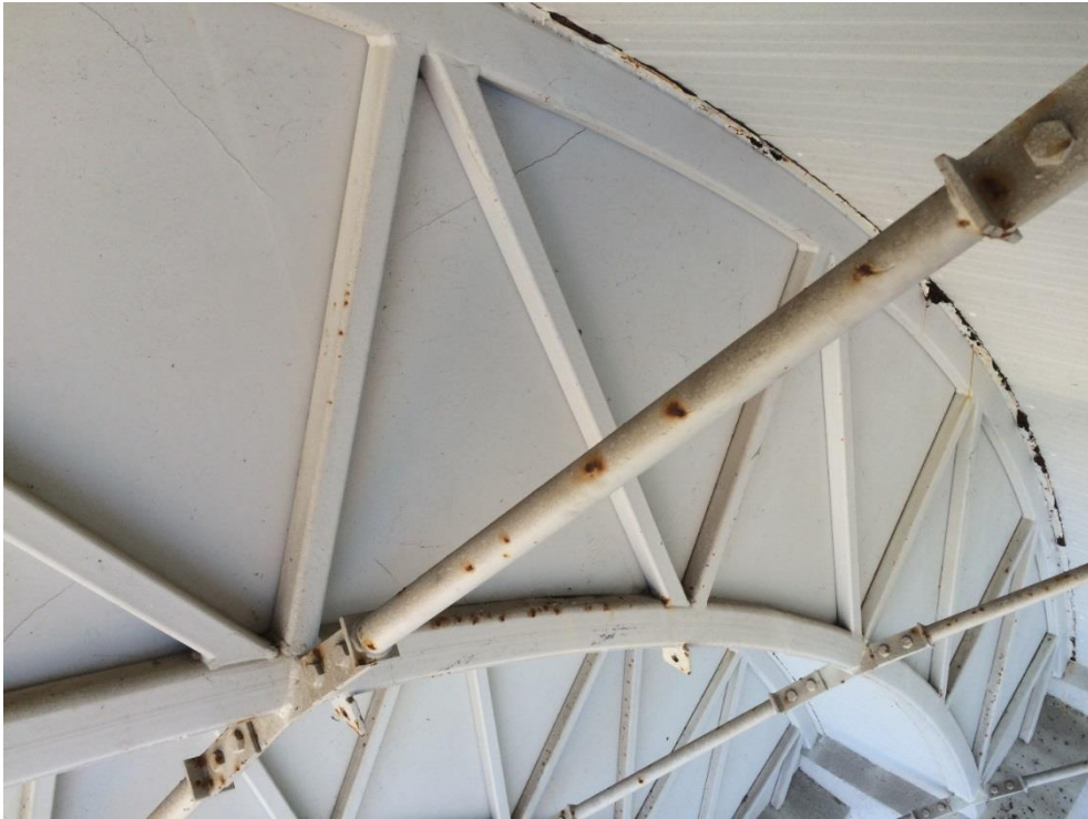
Photo 167 - Minor corrosion to bottom chord
