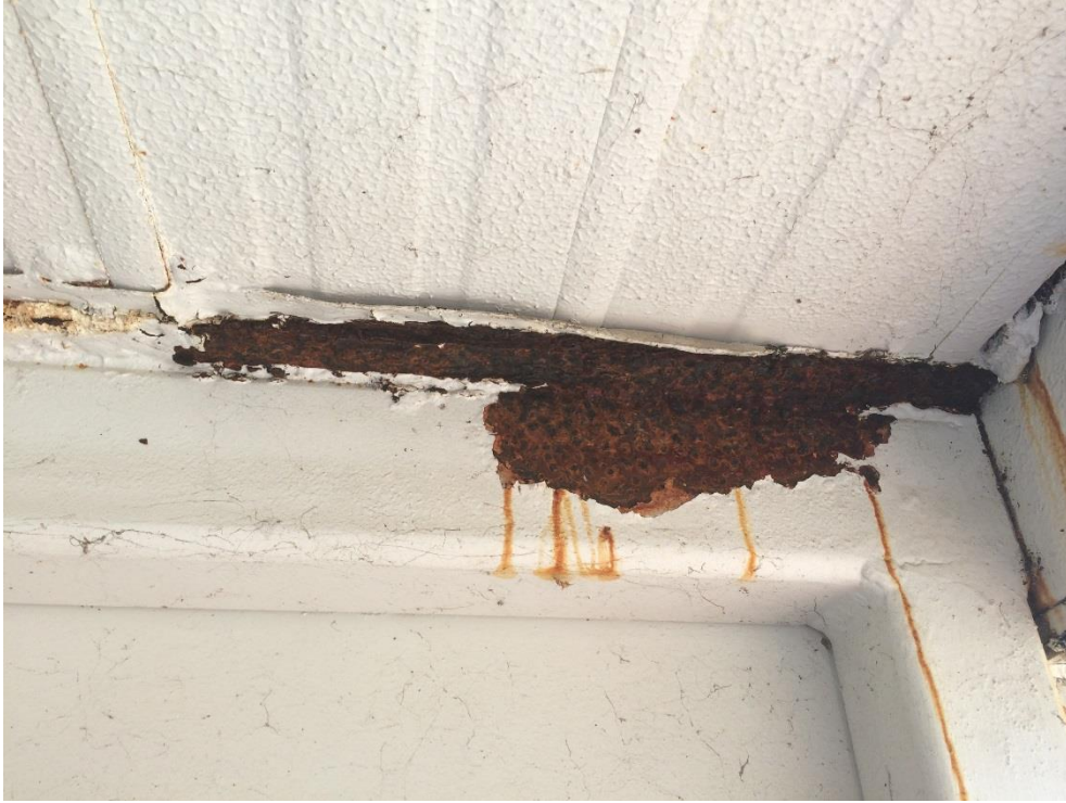
Photo 076 - Heavy corrosion to top plate and top chord
