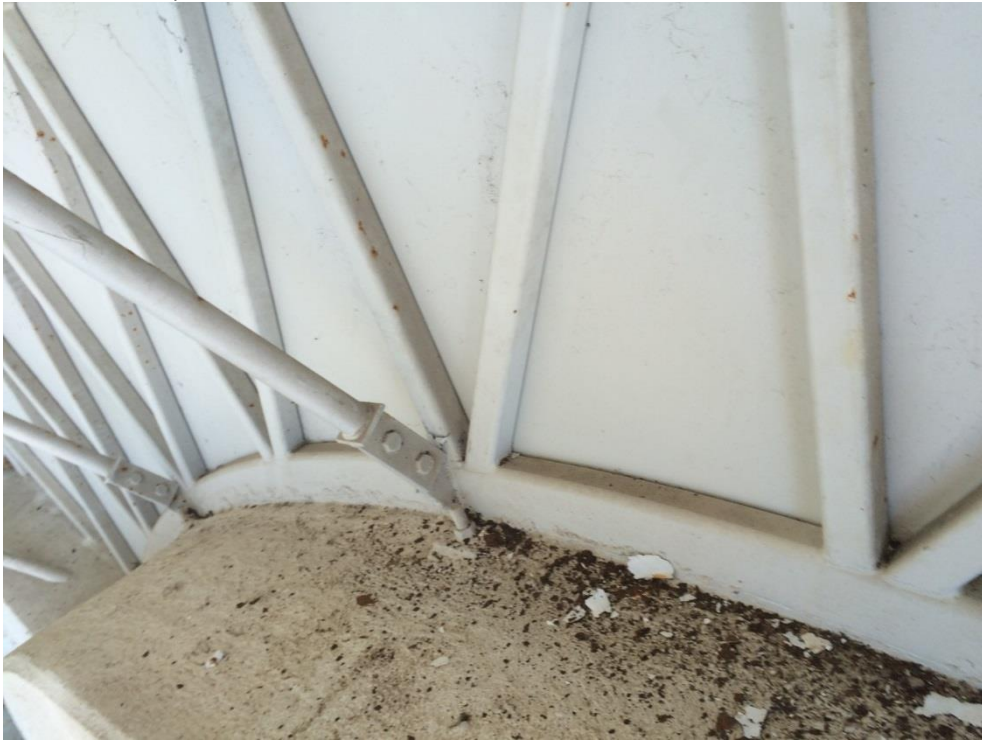
Photo 028 - Heavy corrosion to side of bottom chord
