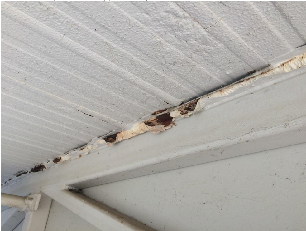
Photo 077 - Heavy corrosion to top plate all along
