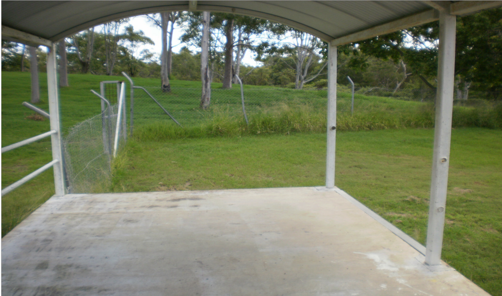
Section of balustrade missing (photo 17)
