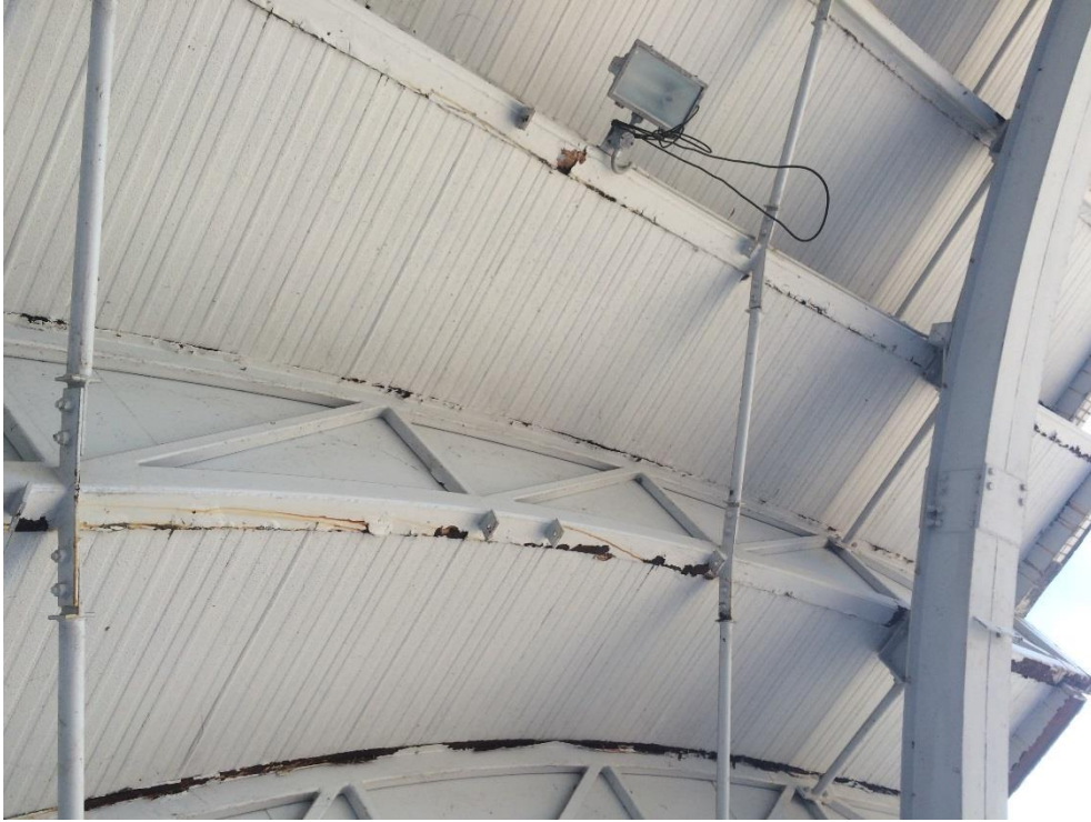
Photo 124 - Minor corrosion to truss top and bottom plate
