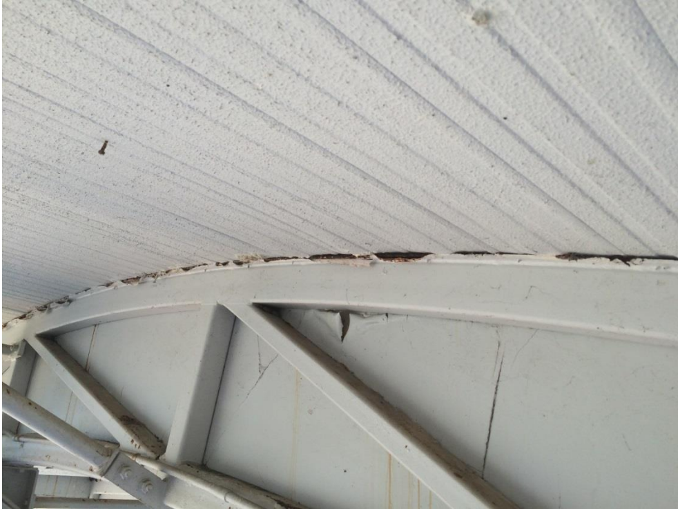
Photo 142 - Minor corrosion to top plate
