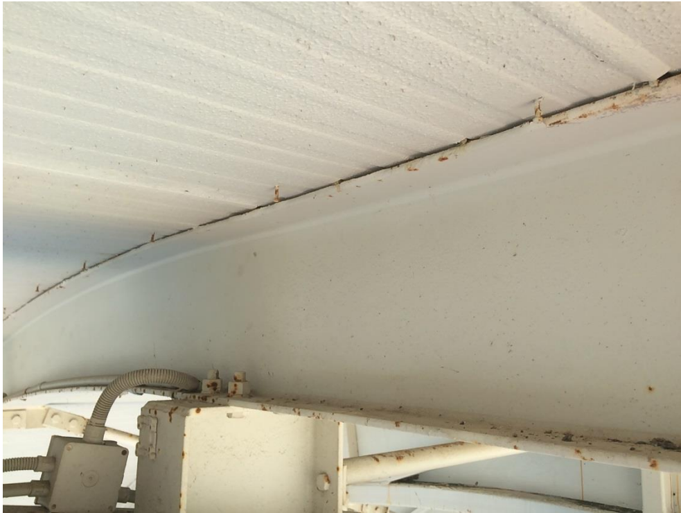
Photo 101 - Minor corrosion to roof beam
