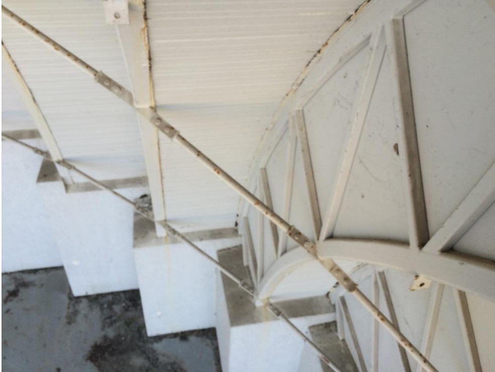
Photo 045 - Minor corrosion to struts
