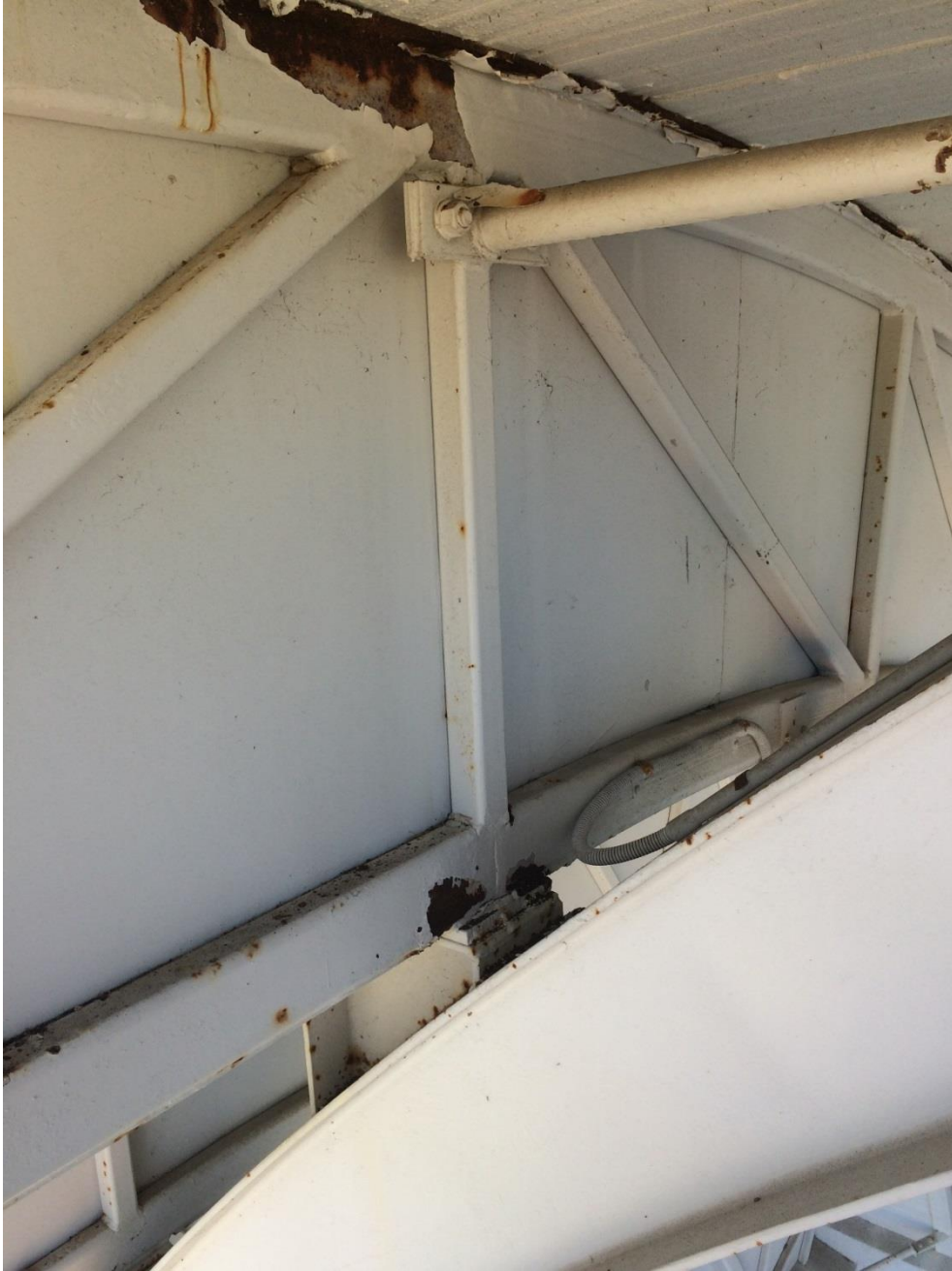
Photo 182 - Heavy corrosion to top plate and top chord of truss
