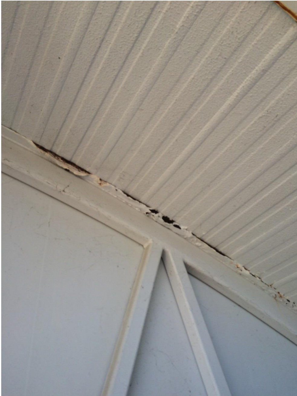
Photo 170 - Minor corrosion to top plate
