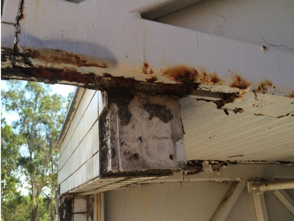
Photo 178 - Heavy corrosion to bottom chord at front face of soundshell
