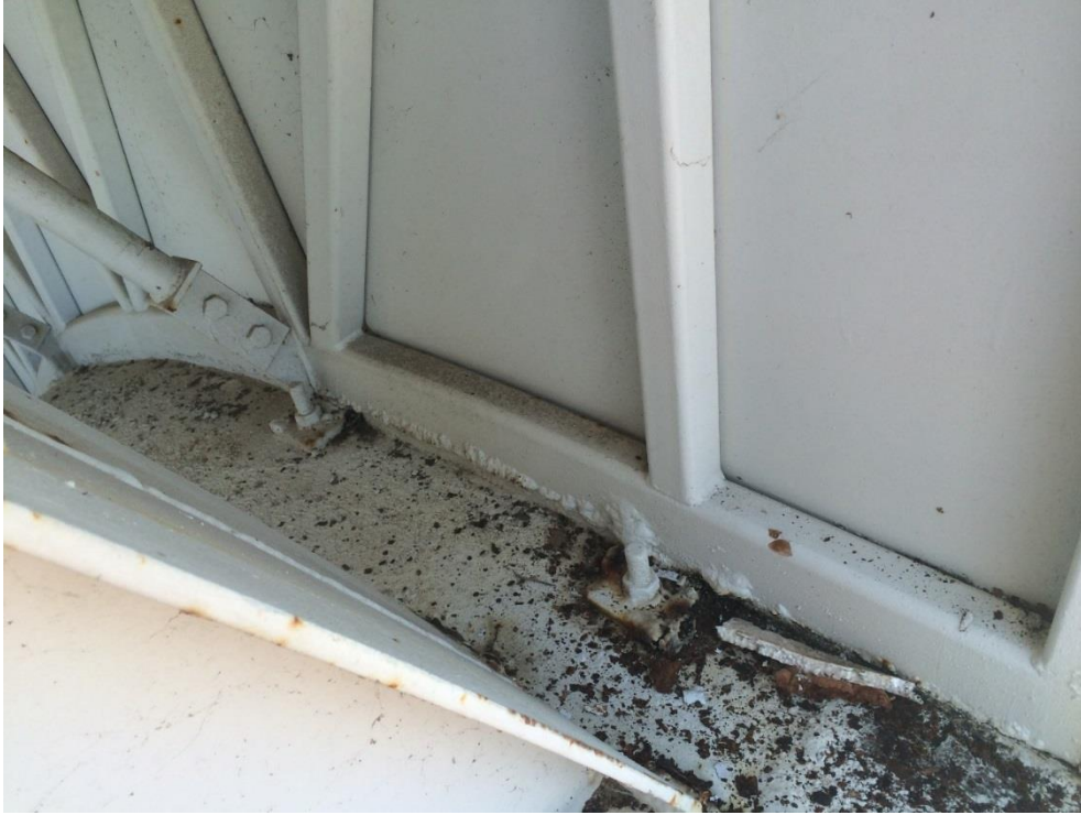
Photo 005 - Corrosion to truss tab plate
