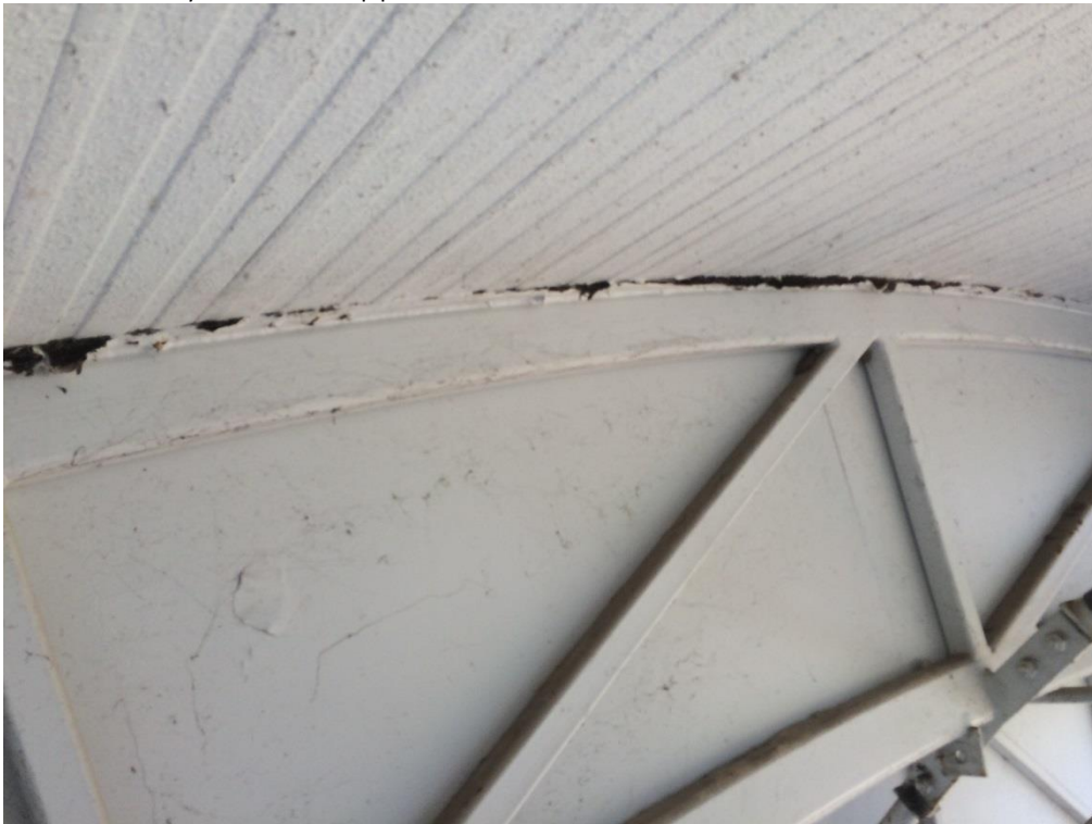
Photo 056 - Heavy corrosion to top plate
