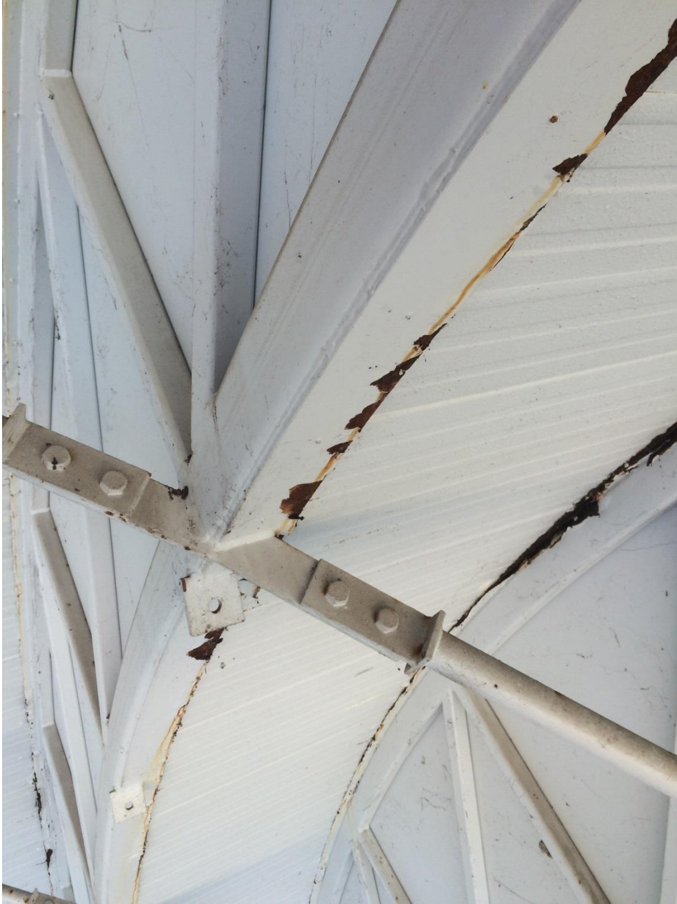
Photo 053 - Minor corrosion to bottom plate
