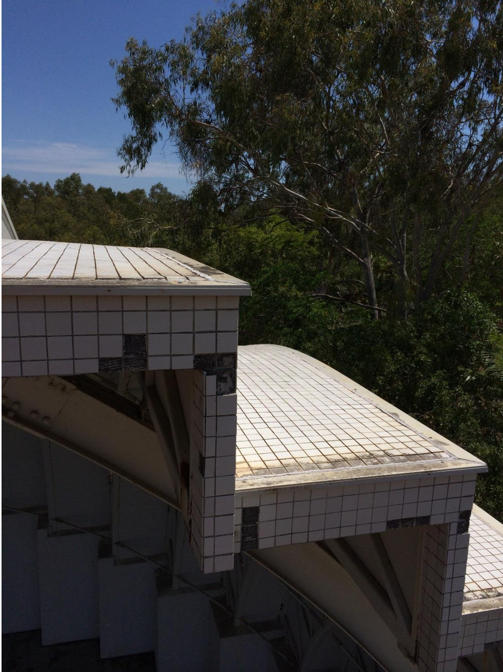
Photo 209 - Front fascia, tiles missing, aluminium edge capping slightly higher than horizontal tiles with evidence of water ponding
