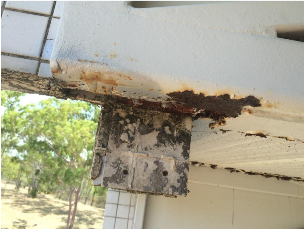
Photo 186 - Heavy corrosion to bottom chord at front face of soundshell
