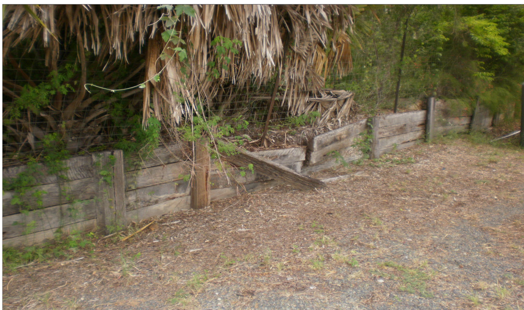
Retaining wall falling down (photo 24)
