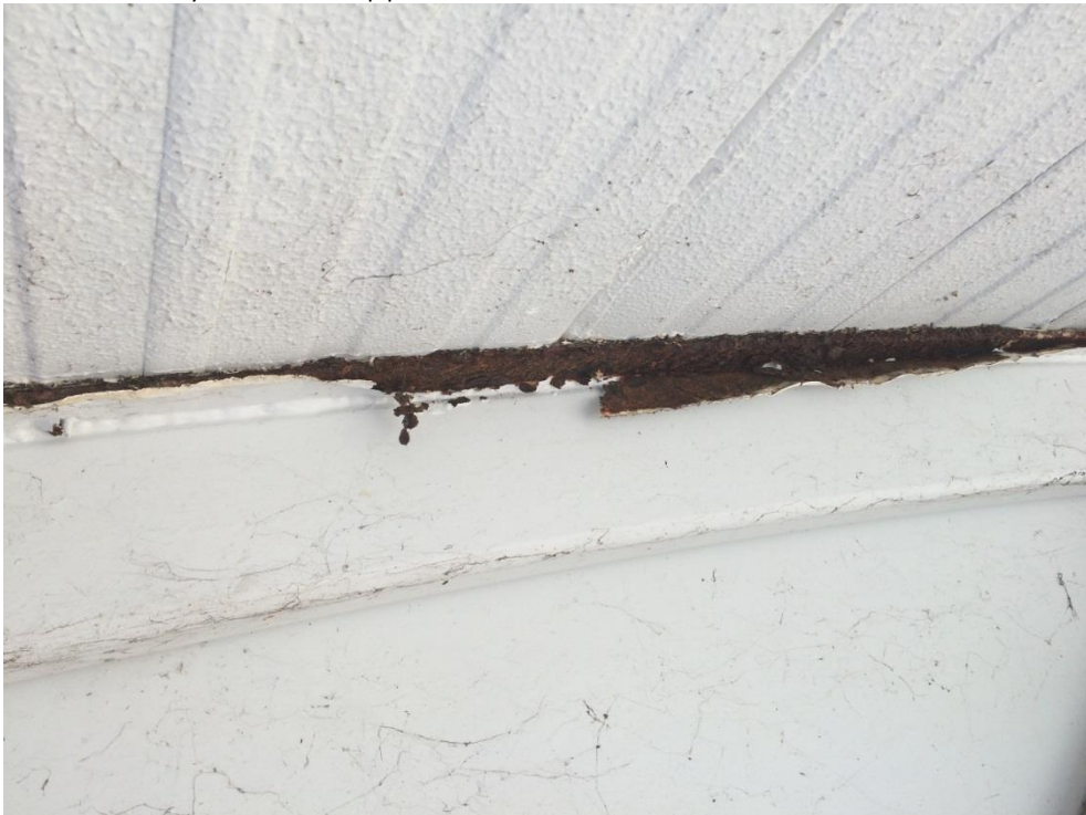
Photo 048 - Heavy corrosion to top plate
