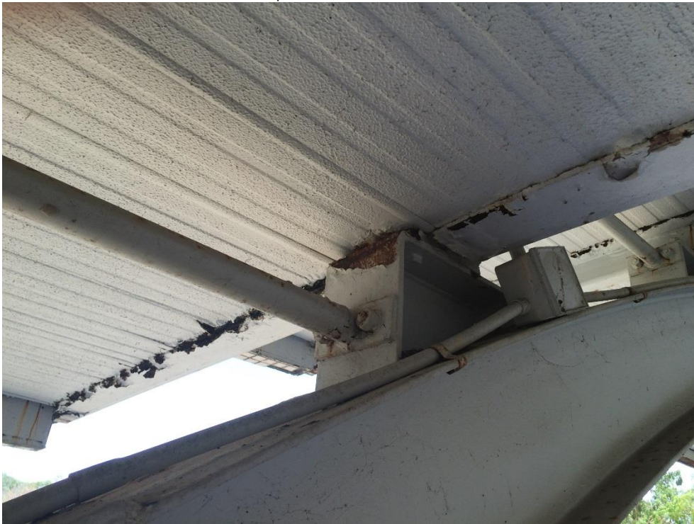
Photo 066 - Heavy corrosion to bottom plate
