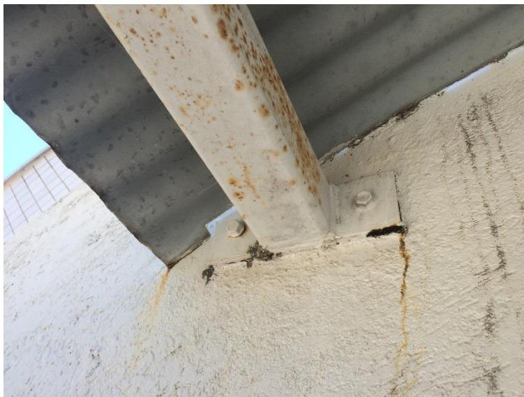
Figure 20 - Minor corrosion to connections
