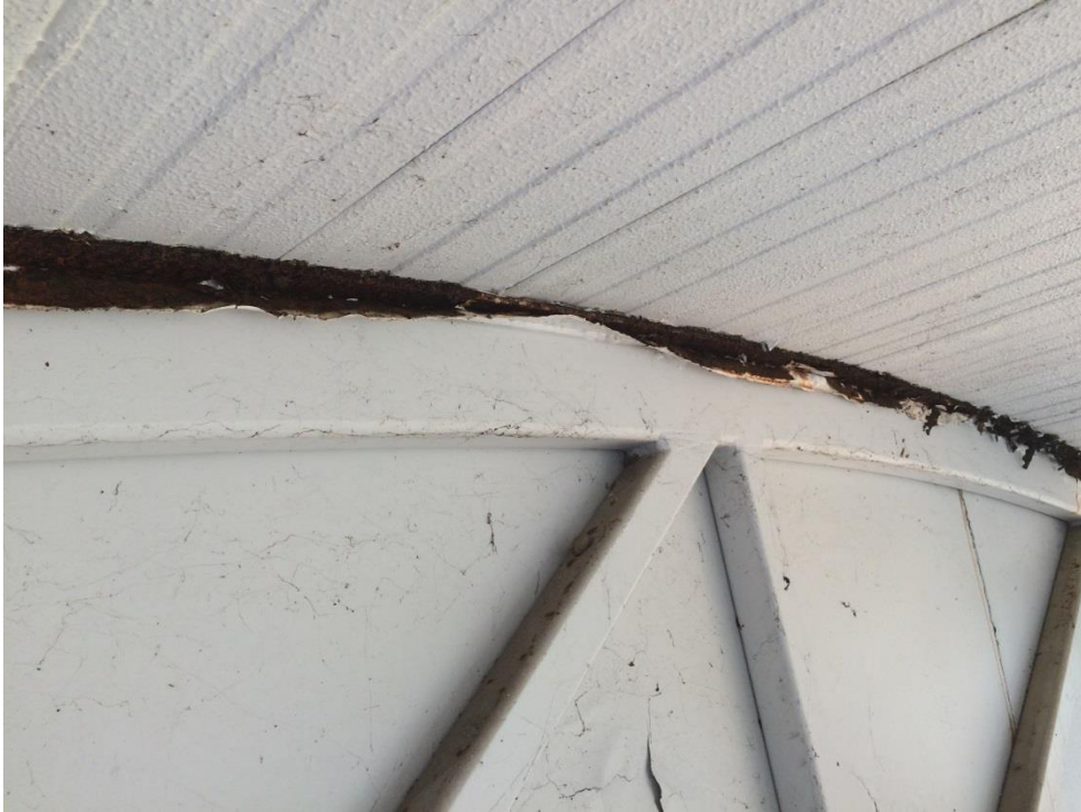
Photo 047 - Heavy corrosion to top plate
