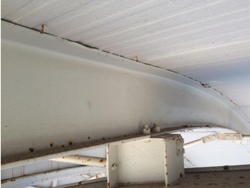
Photo 202 - Minor corrosion to roof beam
