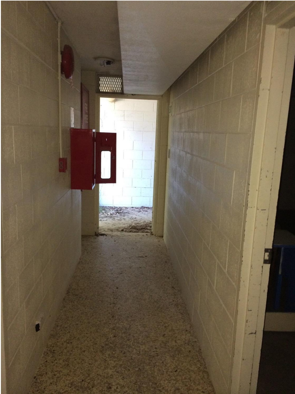
Photo 244 - Lower ground floor corridor
