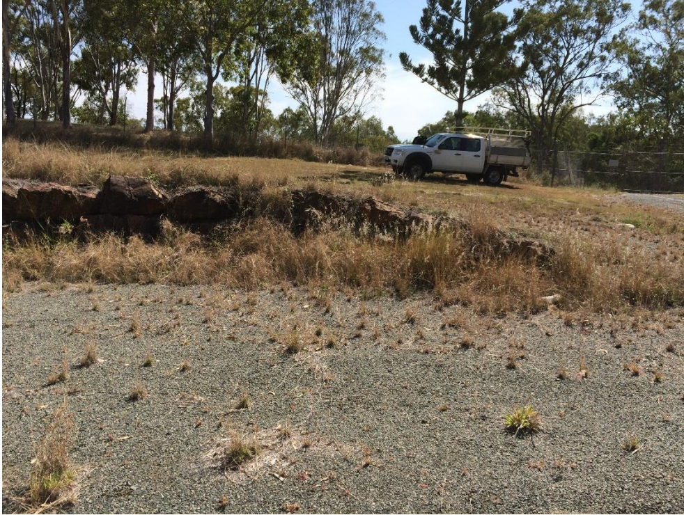
Photo 234 - Boulder wall to north west of sound shell
