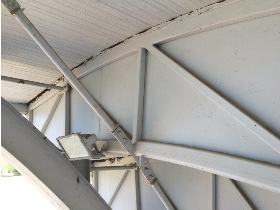
Photo 162 - Minor corrosion to top plate
