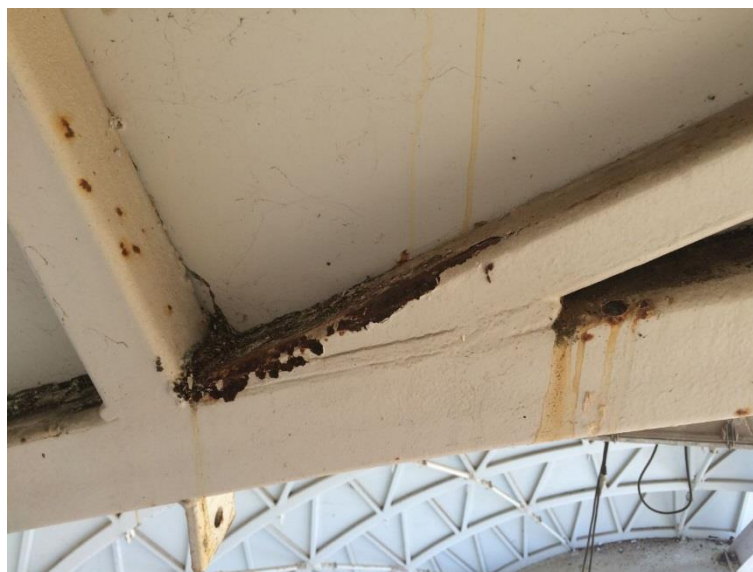
Figure 14 - Corrosion to the truss web members at the bottom chord
