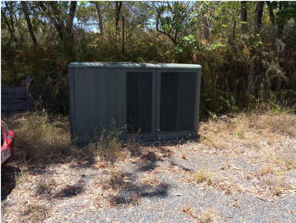
Photo 227 - Substation to rear of soundshell
