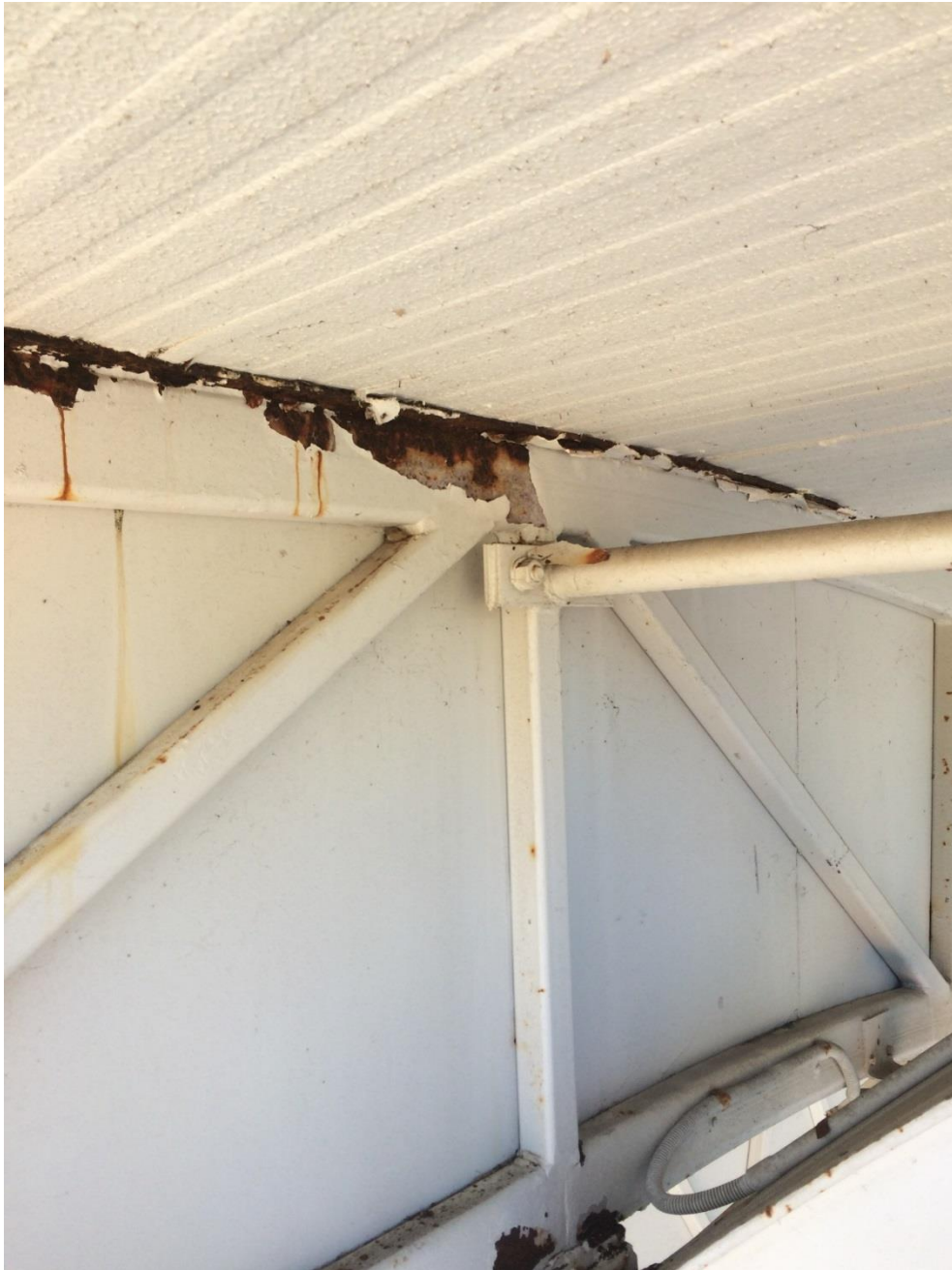
Photo 183 - Heavy corrosion to top plate and top chord of truss
