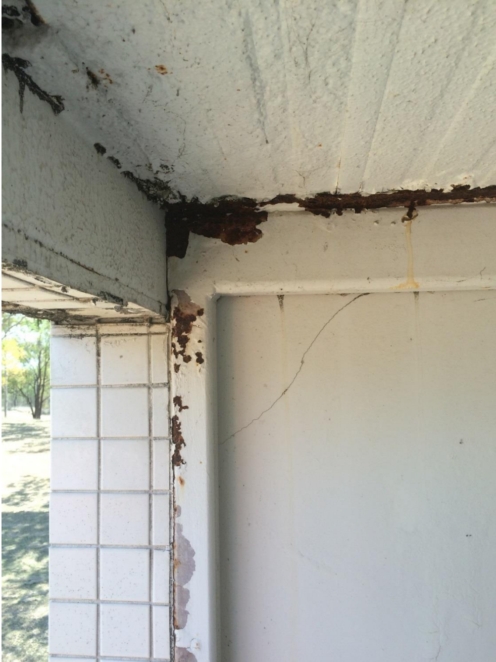
Photo 184 - Heavy corrosion to top plate, minor corrosion to end web of truss
