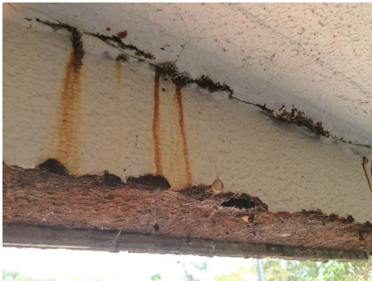
Figure 13 - Corrosion of the steel fascia section at top front of the sound shell
