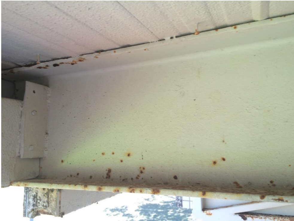
Photo 198 - Minor corrosion to roof beam
