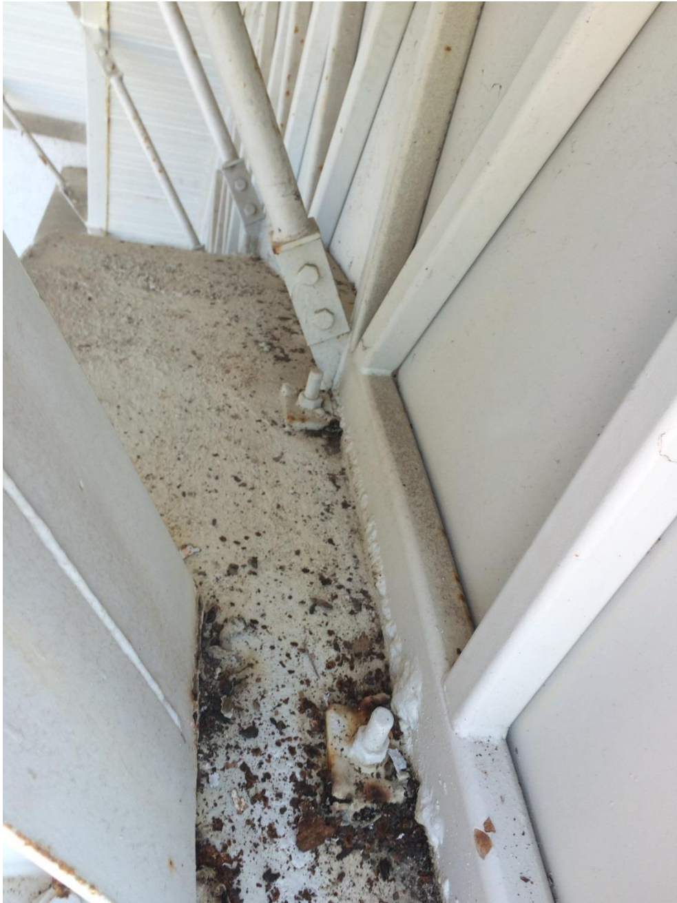
Photo 015 - Minor corrosion to bottom chord along concrete
