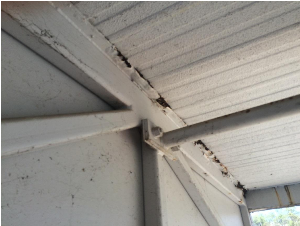
Photo 064 - Heavy corrosion to top plate
