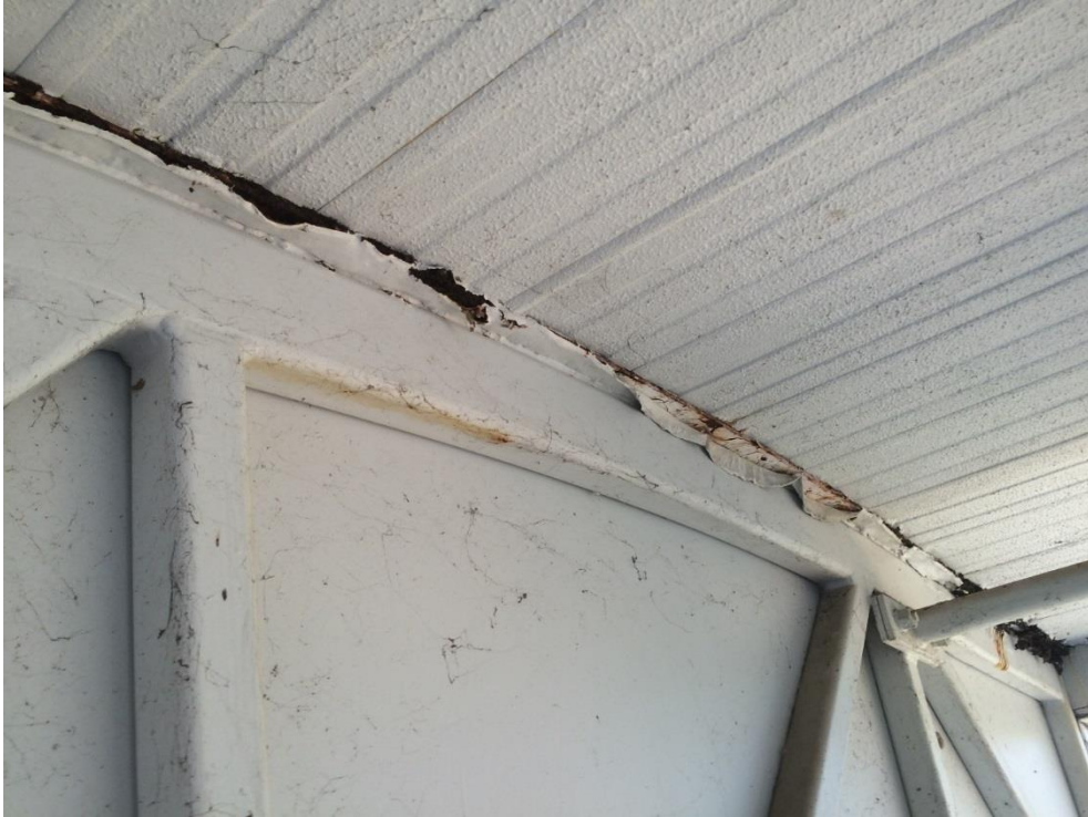
Photo 039 - Heavy corrosion to top plate
