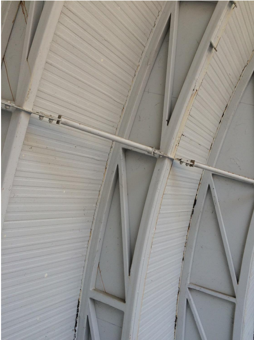
Photo 126 - Minor corrosion to truss top and bottom plate
