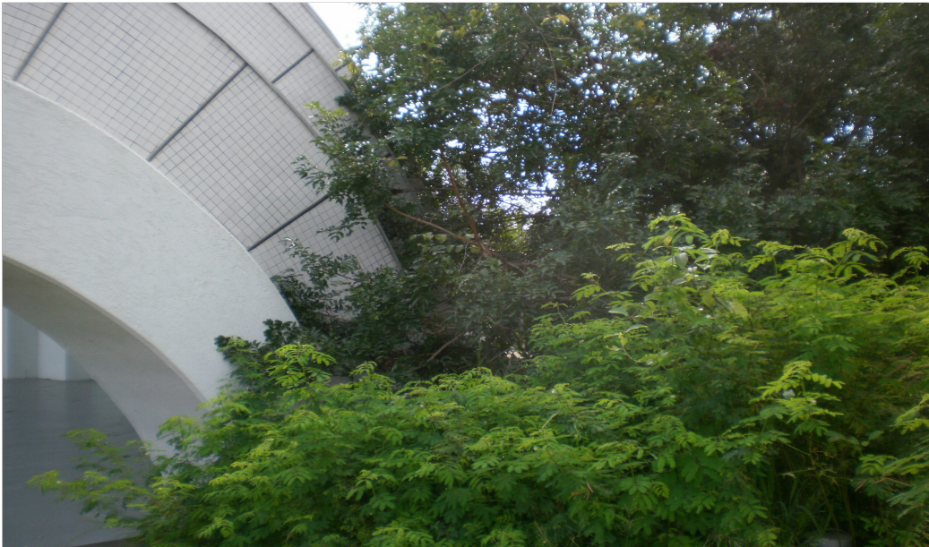
Trees overgrown next to the building (photo 12)
