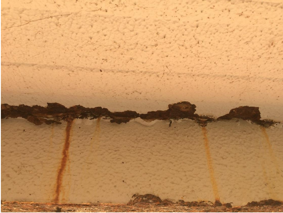
Photo 097 - Minor corrosion to metal formwork
