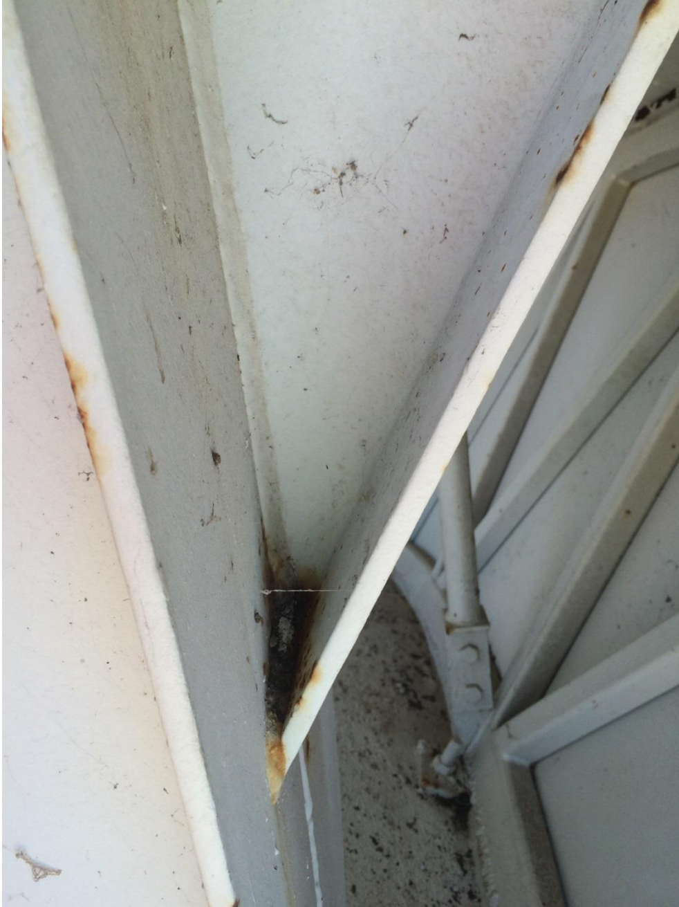
Photo 016 - Minor corrosion in corner of stub
