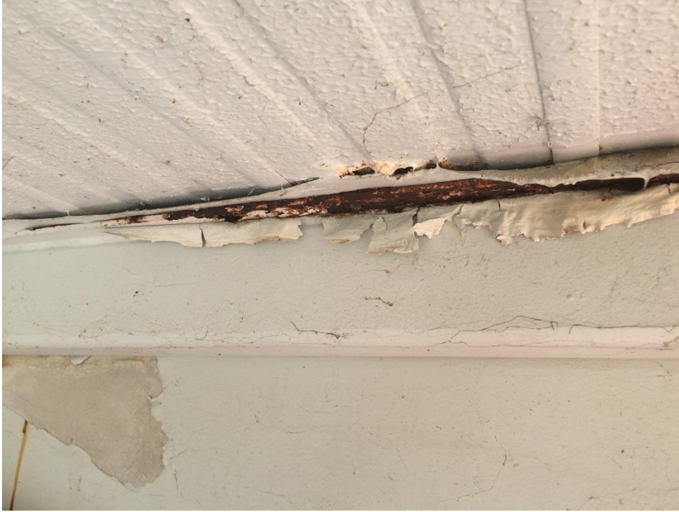
Photo 087 - Heavy corrosion to top plate
