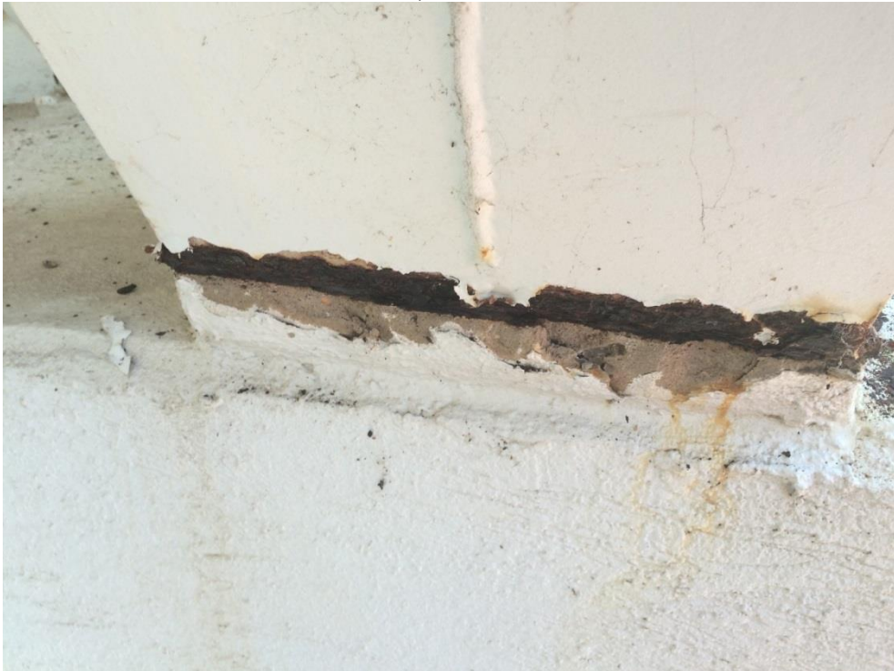
Photo 013 - Minor corrosion to main arch bottom flange at baseplate
