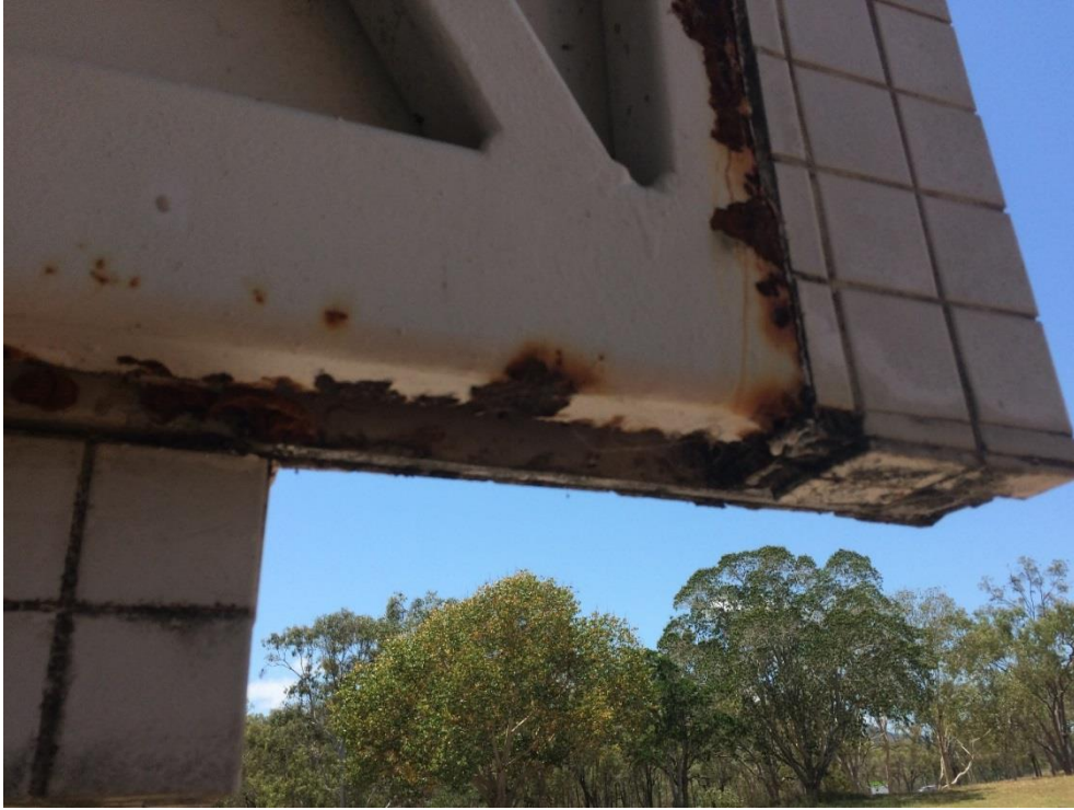
Photo 018 - Heavy corrosion to bottom chord
