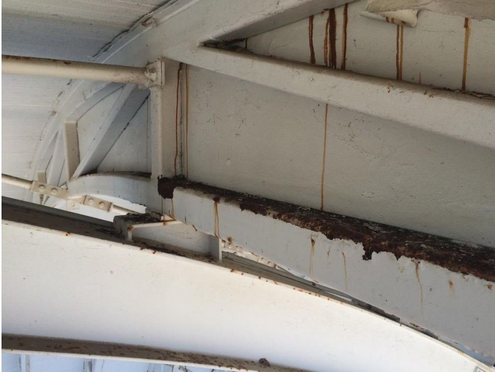
Photo 085 - Heavy corrosion to truss bottom chord
