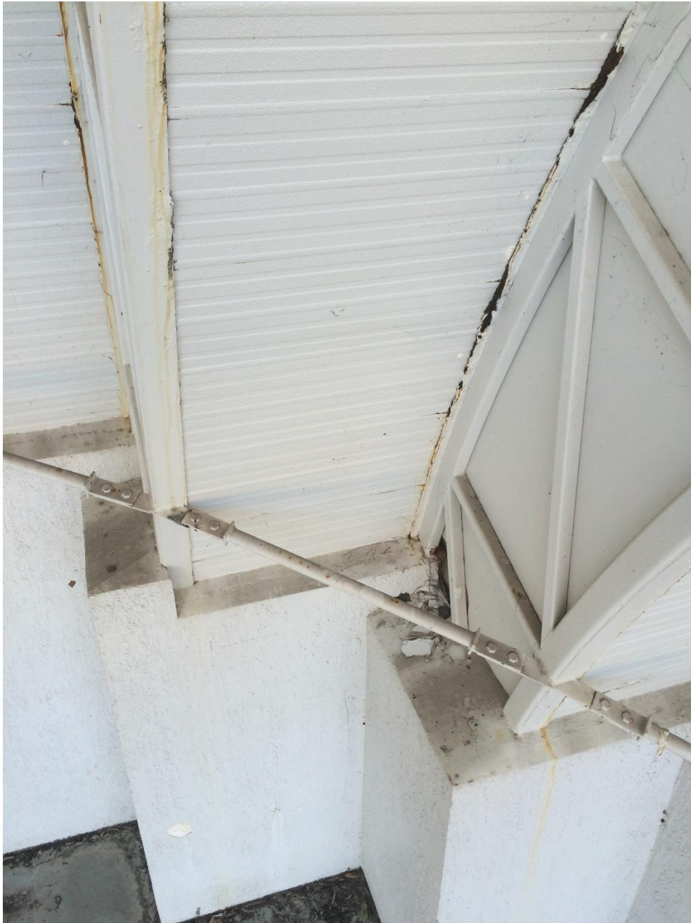
Photo 118 - Minor corrosion to truss to concrete interface
