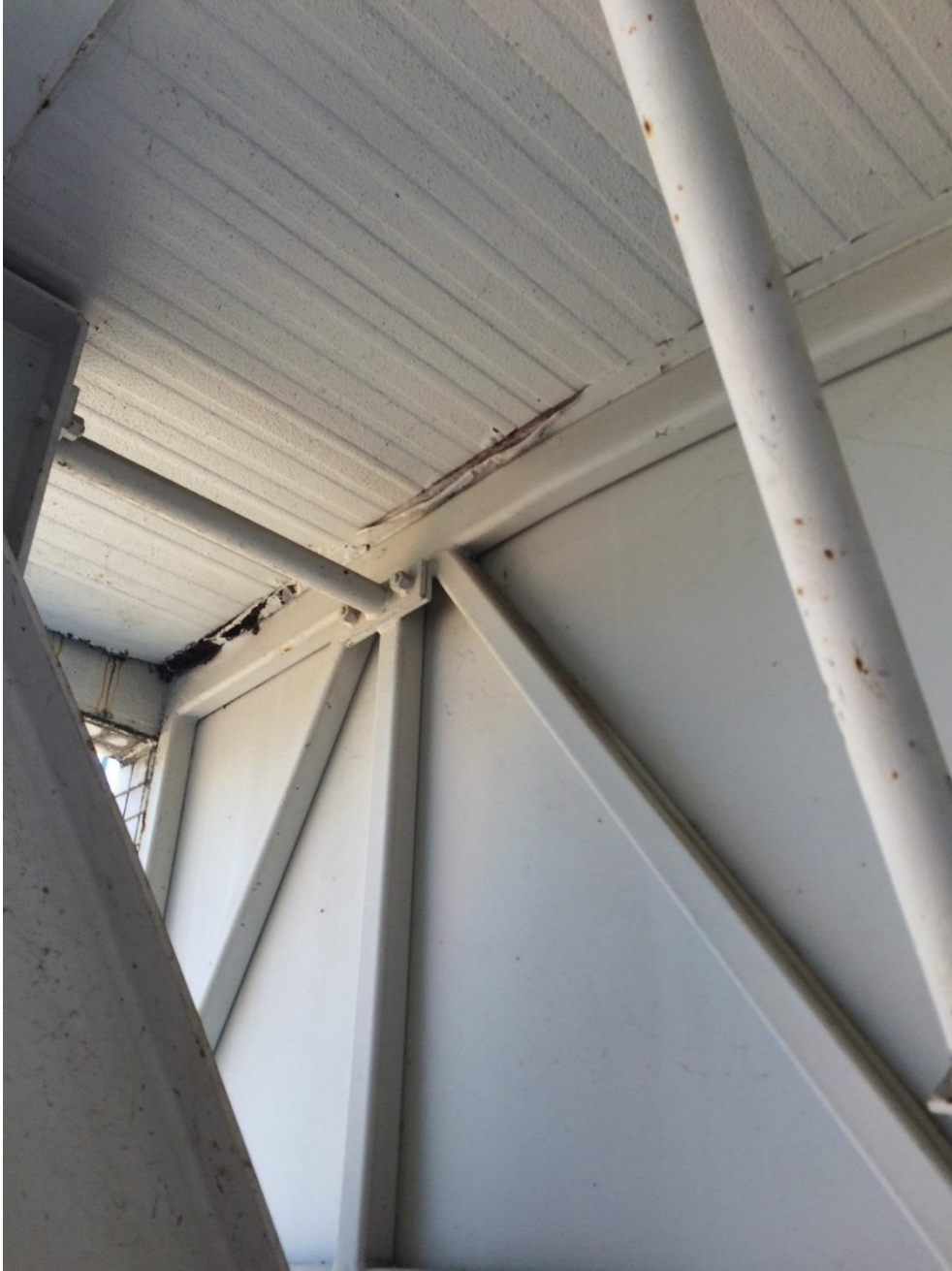
Photo 171 - Minor corrosion to top plate
