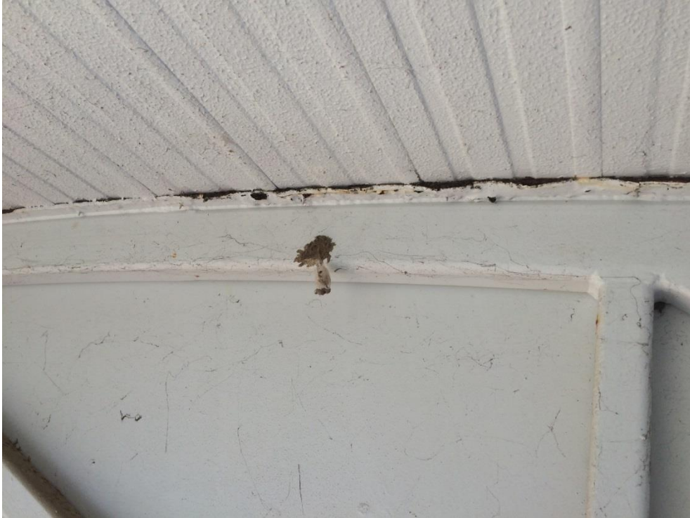
Photo 148 - Heavy corrosion to top plate
