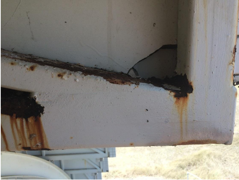
Photo 083 - Heavy corrosion to truss bottom chord and web at the exterior face of the soundshell
