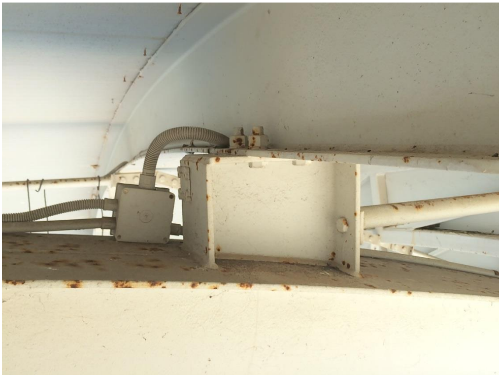
Photo 102 - Minor corrosion to roof beam
