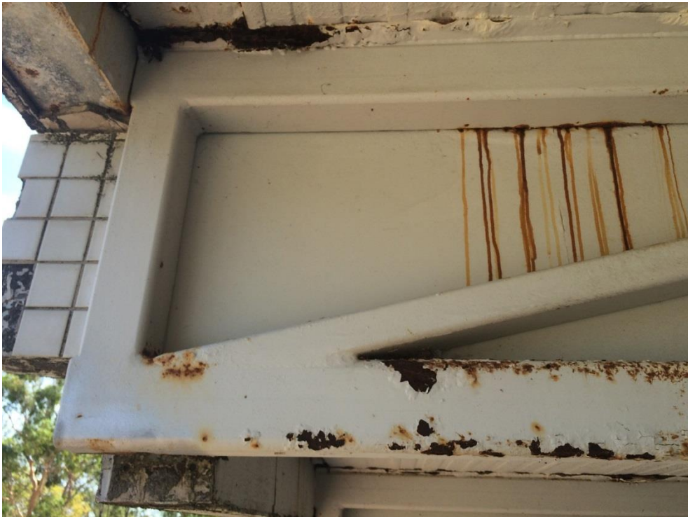
Photo 193 - Heavy corrosion to top plate and bottom chord
