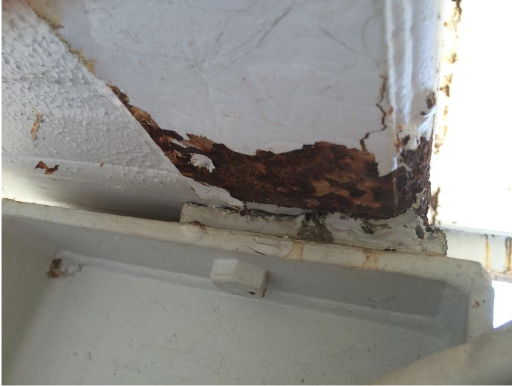
Photo 063 - Minor corrosion to bottom chord at stub
