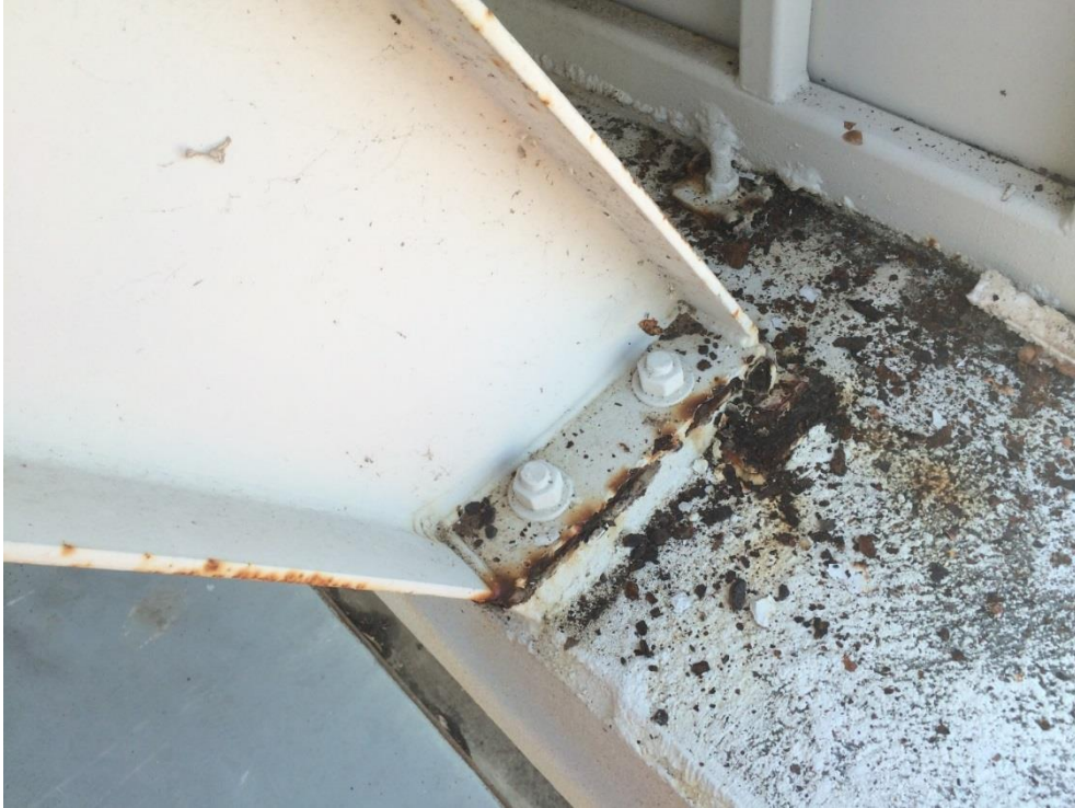
Photo 012 - Minor corrosion to main arch baseplate
