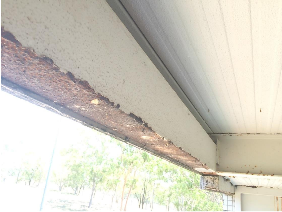
Photo 105 - Heavy corrosion to fascia
