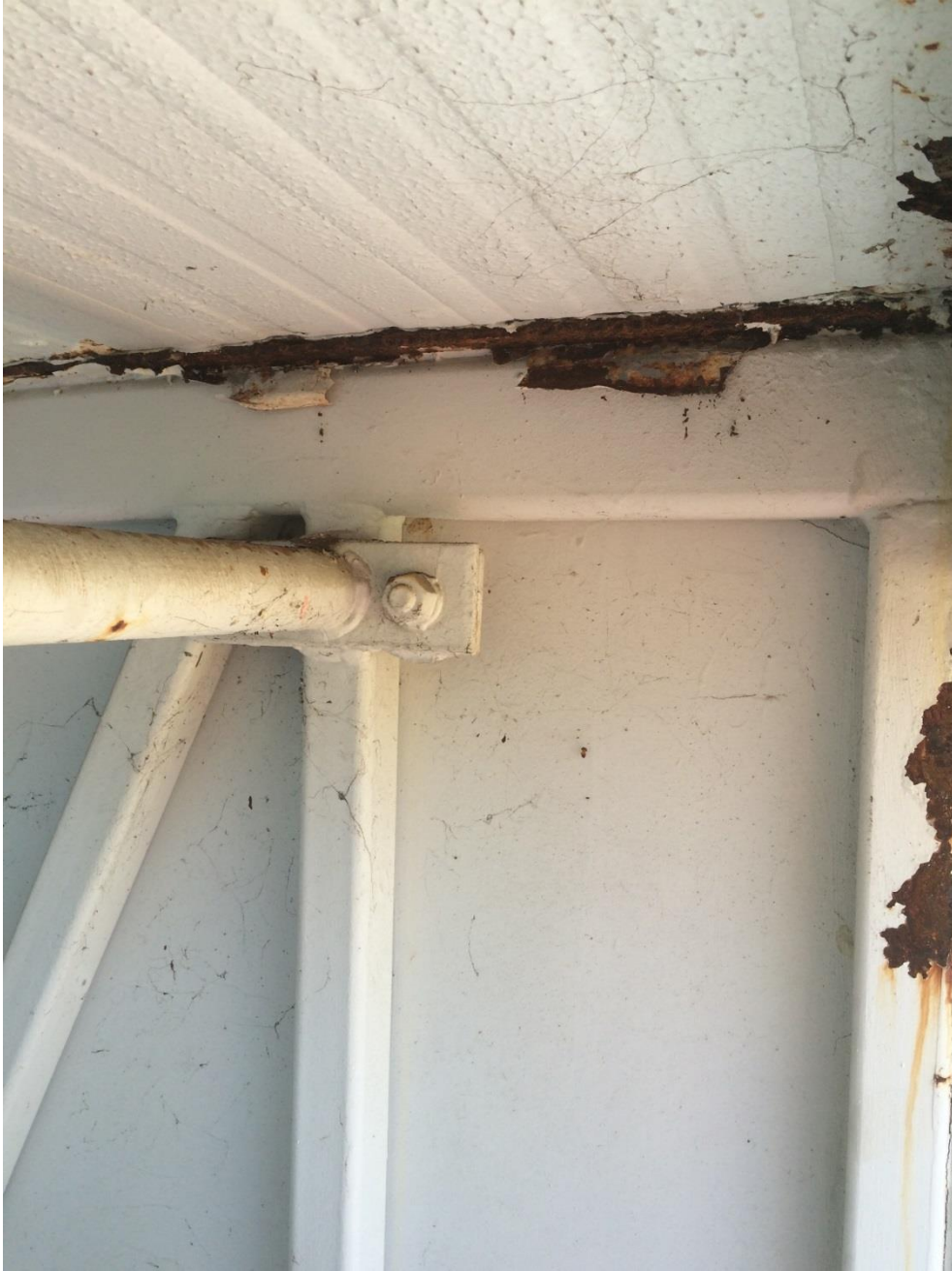
Photo 002 - Corrosion to top plate
