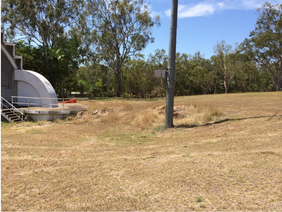
Photo 232 - Boulder wall to south east of sound shell
