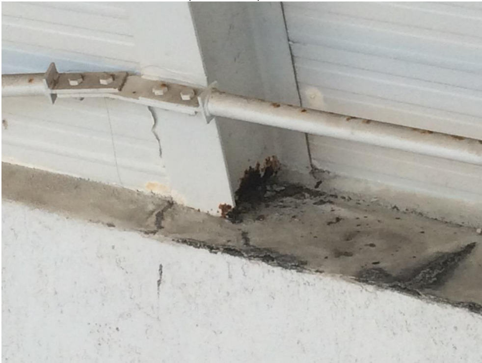
Photo 129 - Heavy corrosion to web of roof beam
