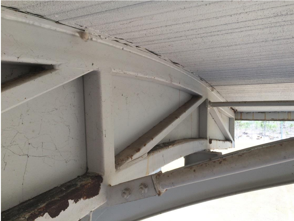
Photo 108 - Minor corrosion to bottom chord
