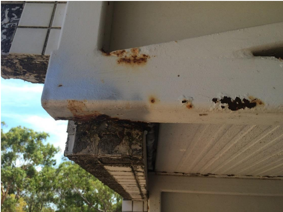
Photo 191 - Minor corrosion to bottom chord at front face of soundshell
