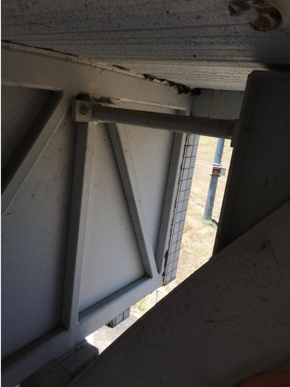
Photo 030 - Heavy corrosion to top plate
