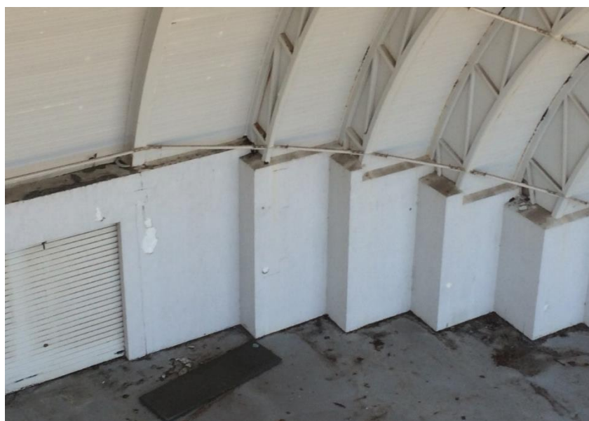
Figure 4 - Roof trusses enclosed in masonry wall
