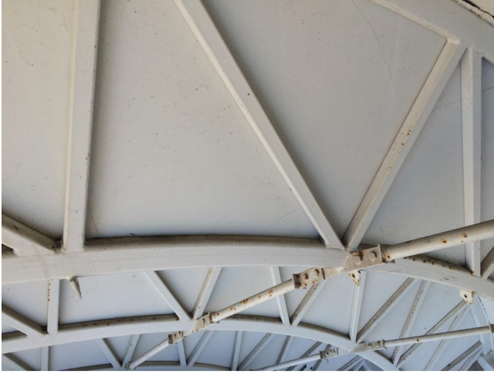
Photo 166 - Minor corrosion to bottom chord
