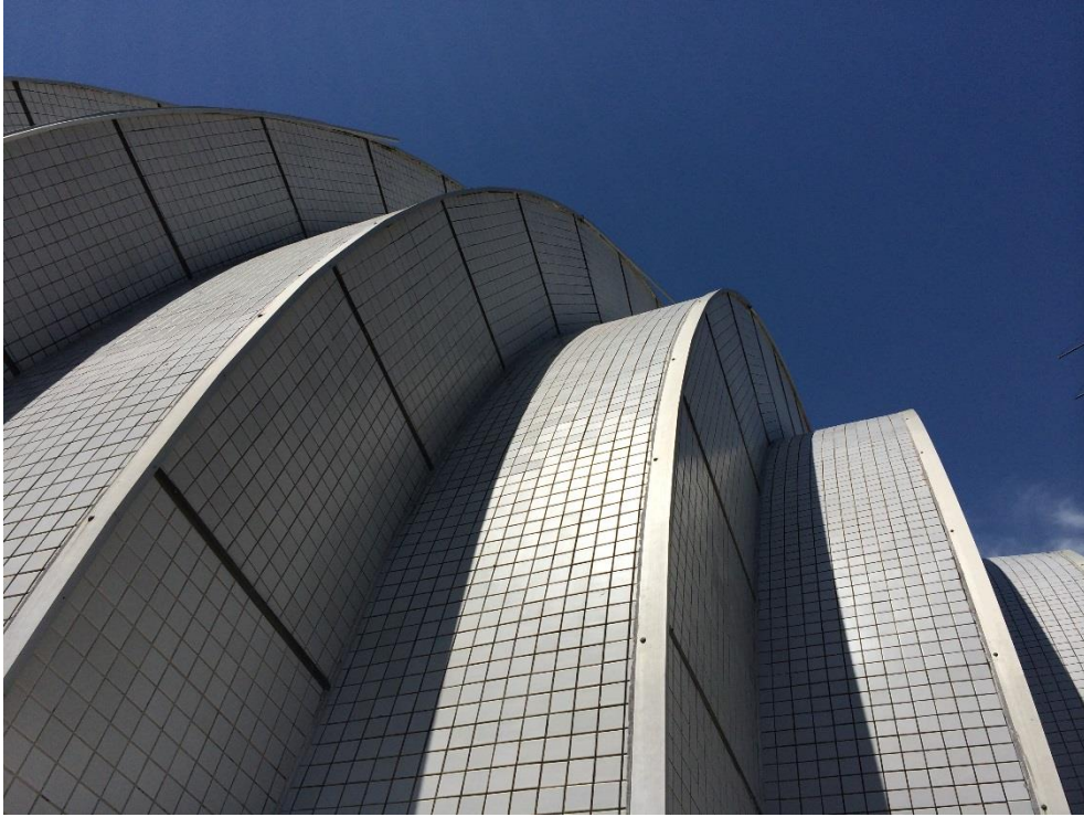
Photo 210 - Rear surface of sound shell, some aluminium edge capping coming loose on curved surfaces
