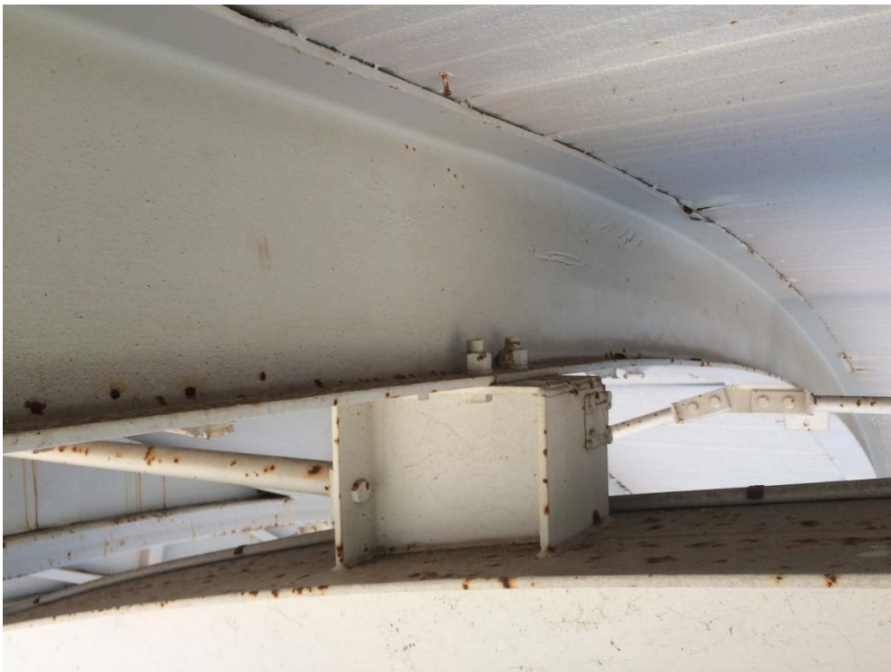
Photo 203 - Minor corrosion to roof beam
