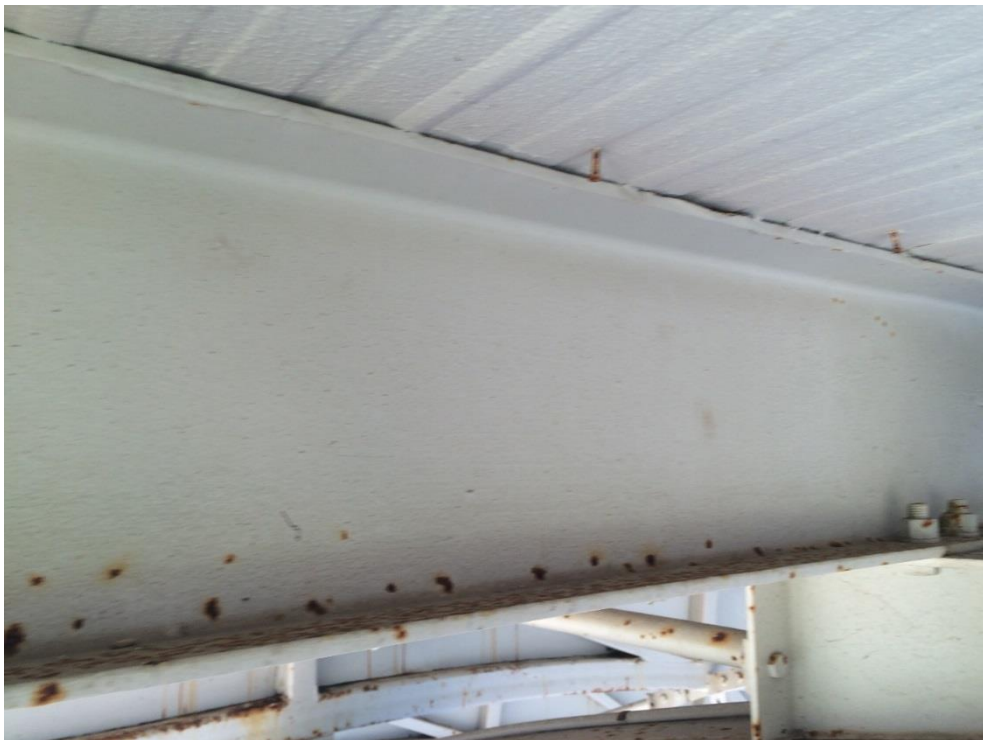
Photo 201 - Minor corrosion to roof beam
