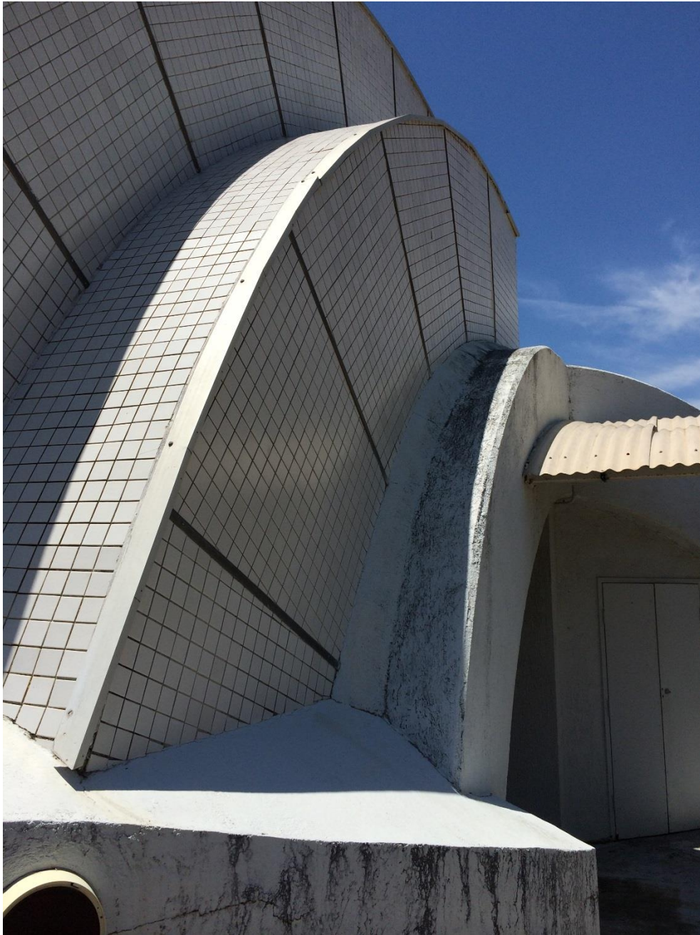
Photo 211 - Rear surface of sound shell and main arch support abutment
