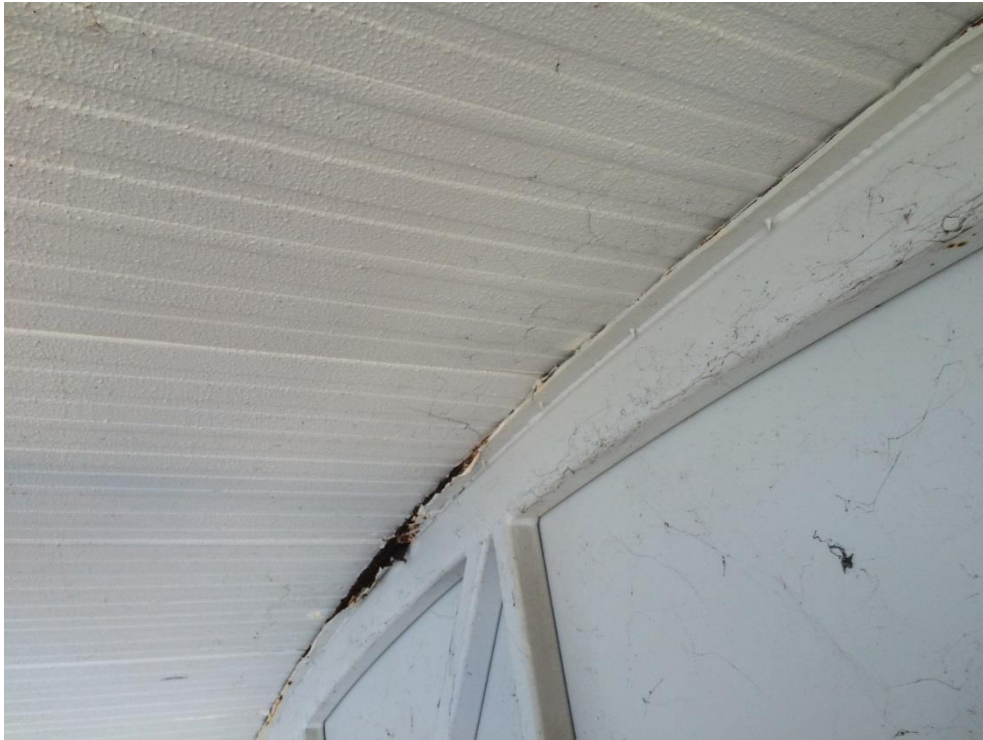
Photo 043 - Heavy corrosion to top plate
