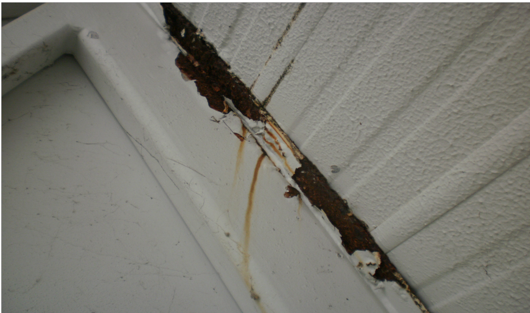
Rusted Structural Steel (photo 4)
