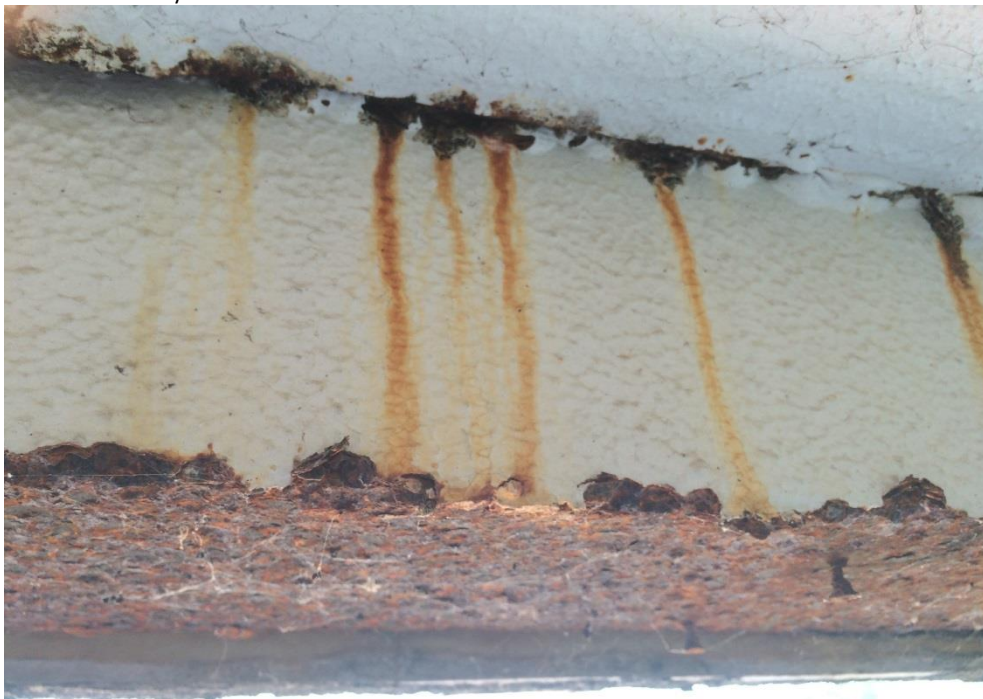
Photo 093 - Heavy corrosion to fascia
