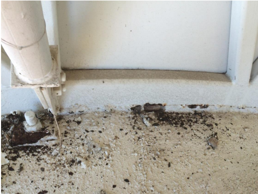
Photo 174 - Heavy corrosion to the side of bottom chord
