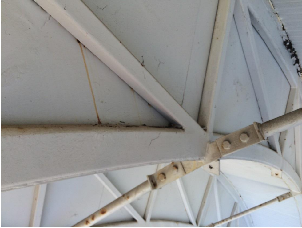
Photo 152 - Minor corrosion to bottom chord
