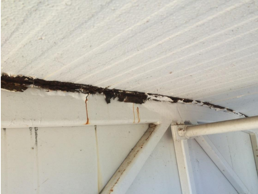
Photo 180 - Heavy corrosion to top plate and top chord of truss
