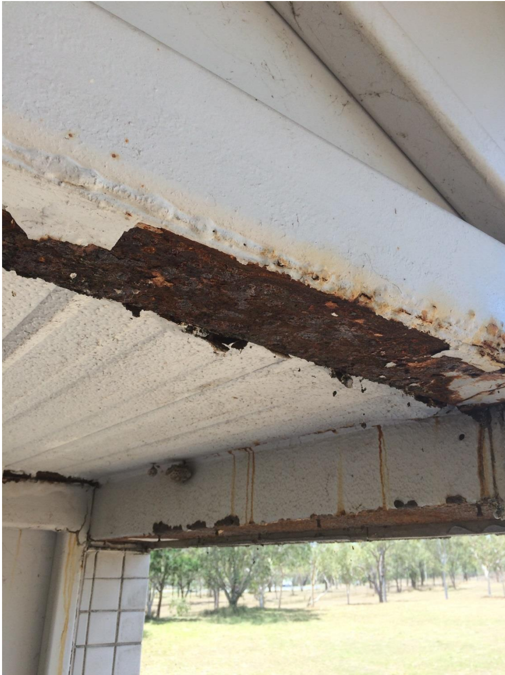
Photo 074 - Heavy corrosion to bottom plate
