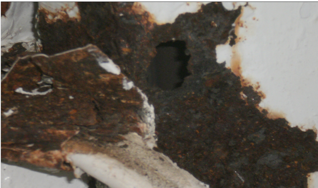
Rusted Structural Steel (photo 2)
