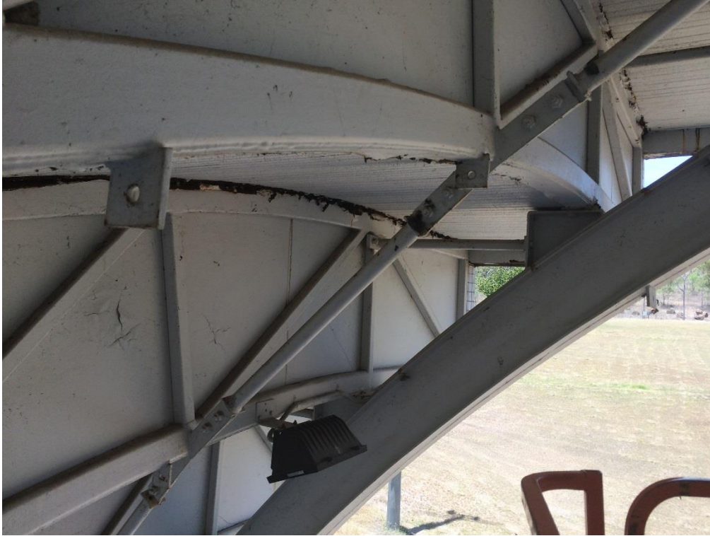
Photo 061 - minor corrosion to bottom plate
