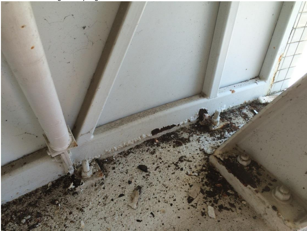
Photo 026 - Heavy corrosion to side of bottom chord
