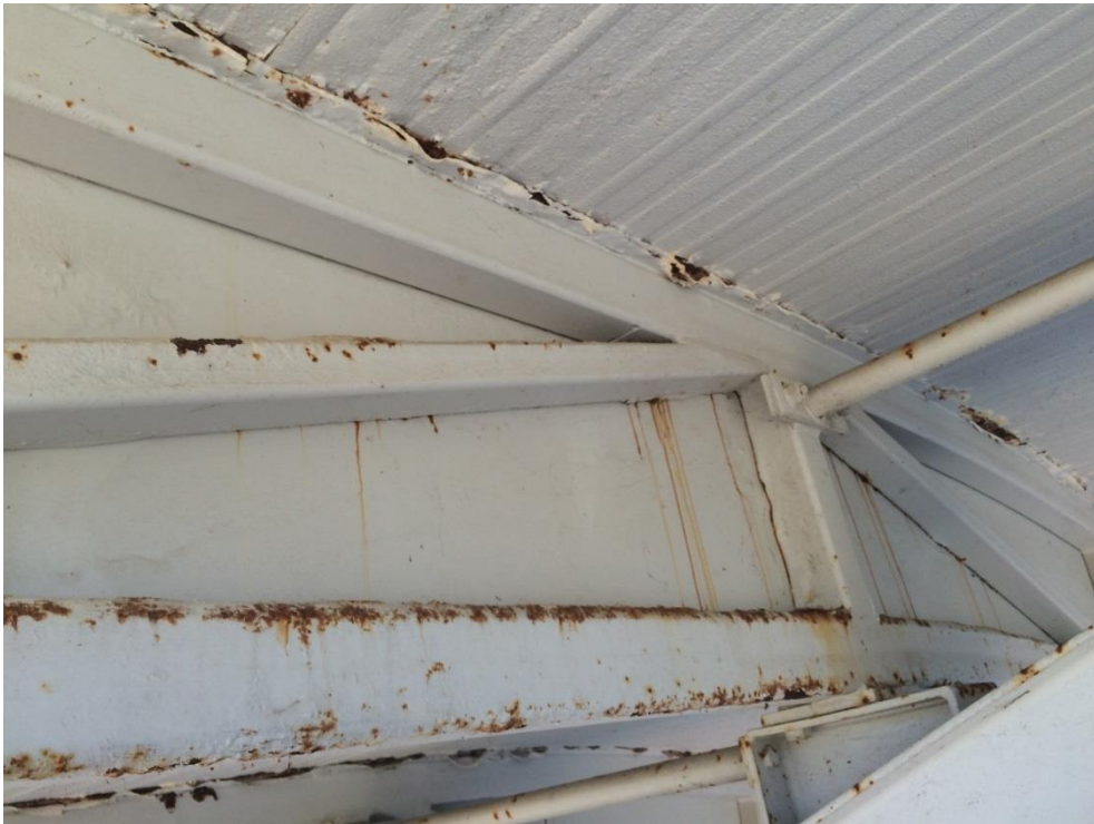
Photo 195 - Heavy corrosion to top plate and bottom chord
