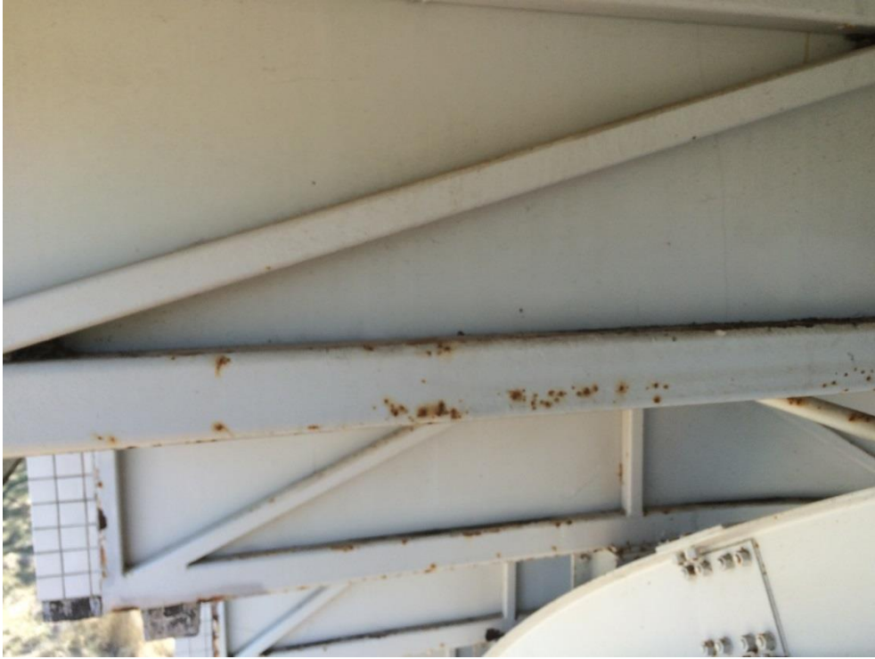
Photo 188 - Minor corrosion to bottom chord
