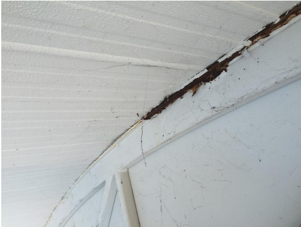
Photo 051 - Heavy corrosion to top plate
