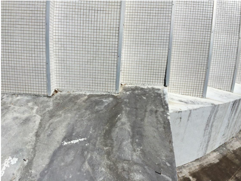
Photo 216 - Rear of sound shell, junction of tiled cladding, aluminium capping coming loose
