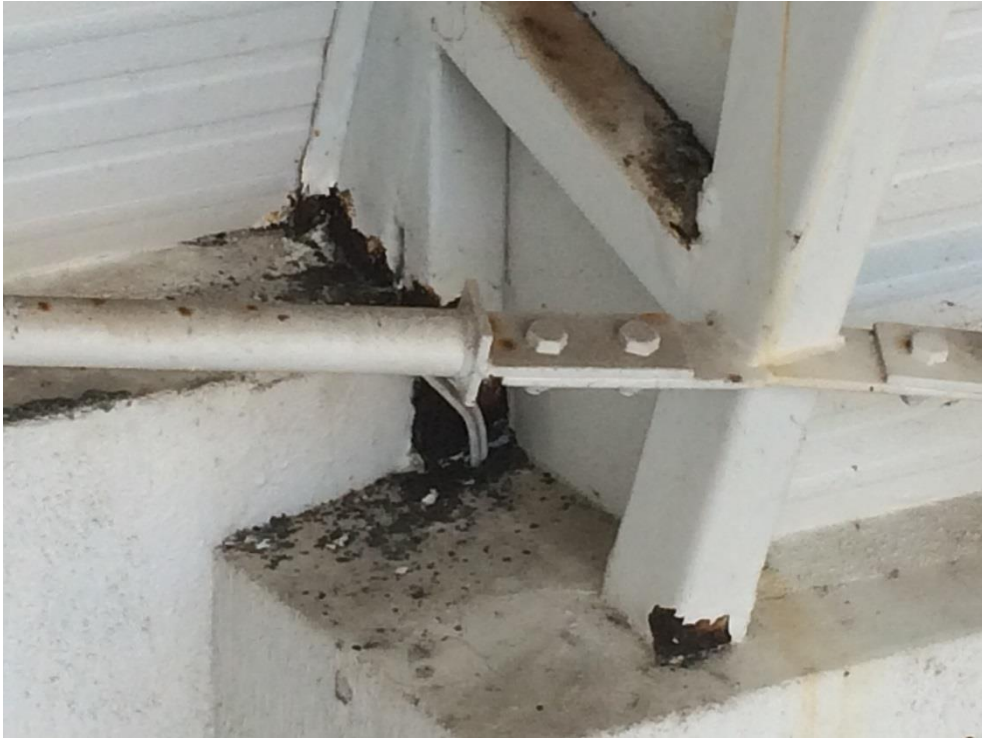
Photo 113 - Heavy corrosion to truss at concrete interface
