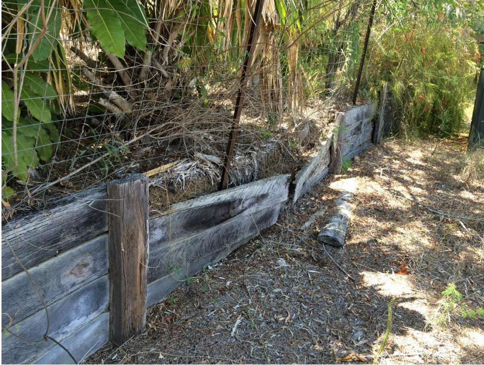
Photo 226 - Timber retaining wall, rotted and collapsed
