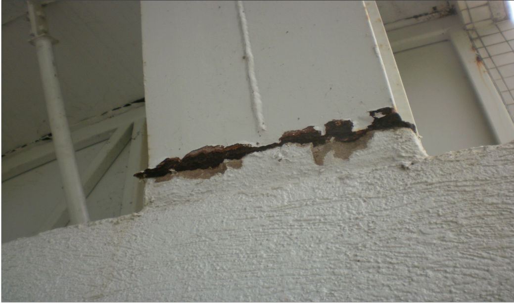
Rusted Structural Steel (photo 3)
