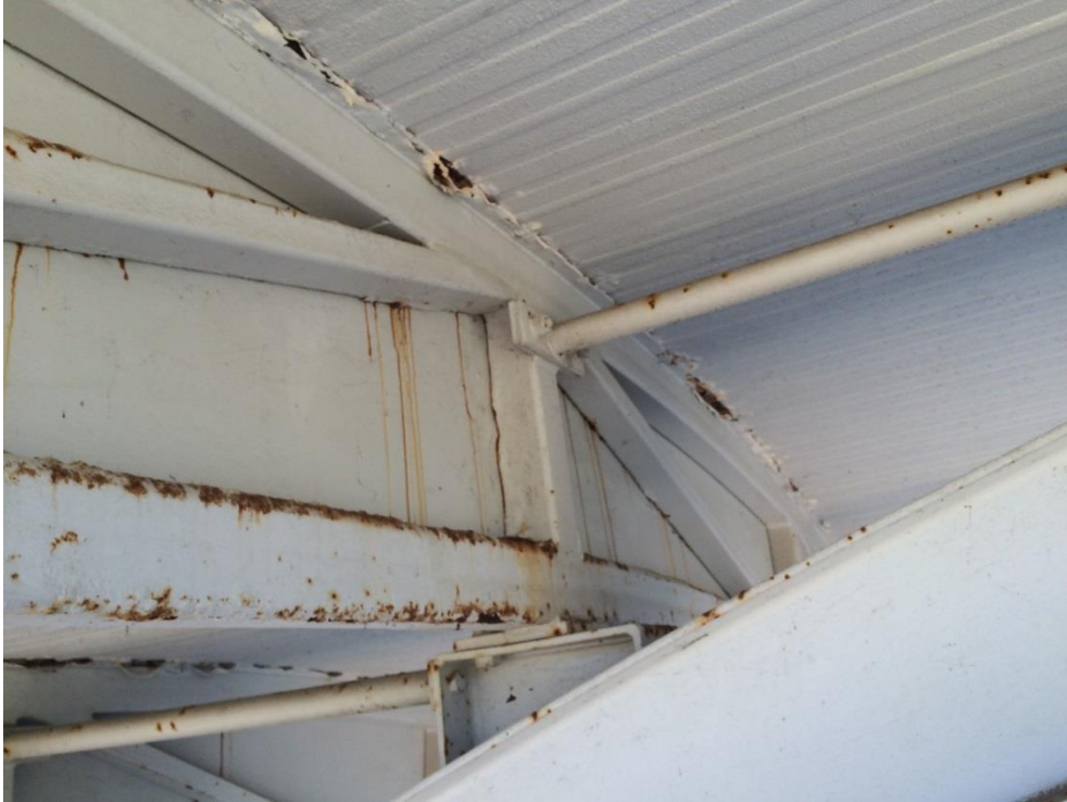
Photo 196 - Heavy corrosion to top plate and bottom chord
