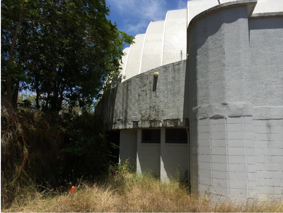
Photo 249 - Rear view of external substructure
