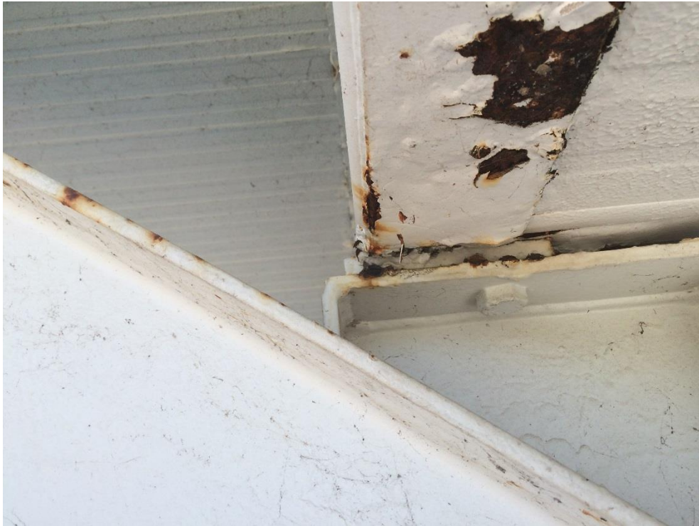
Photo 068 - Heavy corrosion to bottom plate
