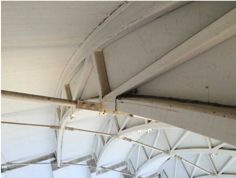
Photo 110 - Minor corrosion to web member
