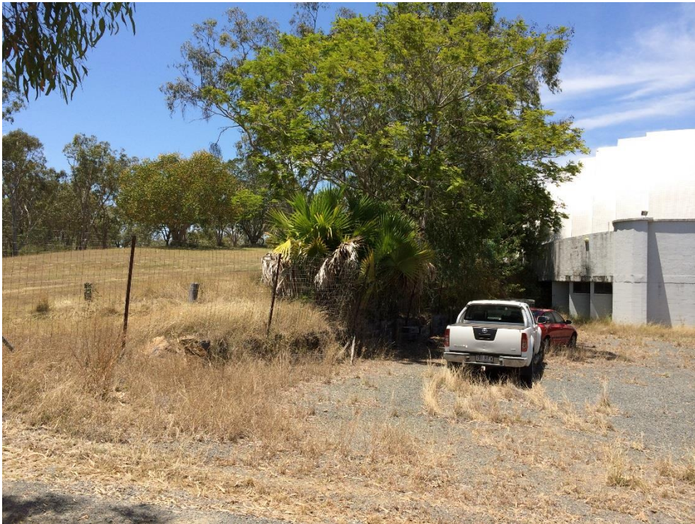
Photo 223 - Landscaping and retaining wall to north east of sound shell
