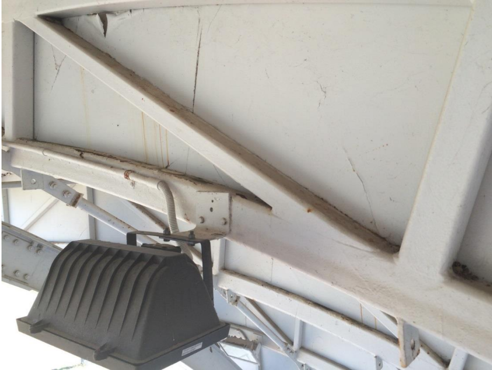
Photo 140 - Minor corrosion to bottom chord of truss
