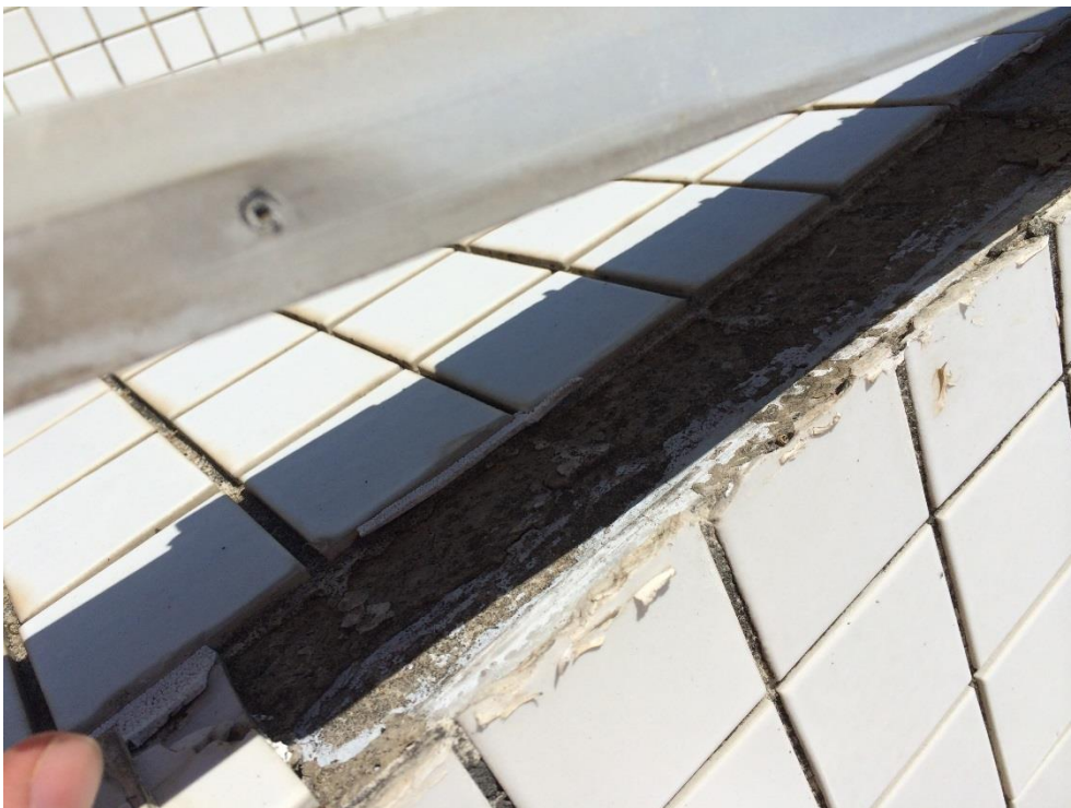
Figure 8 - Loose aluminium capping
