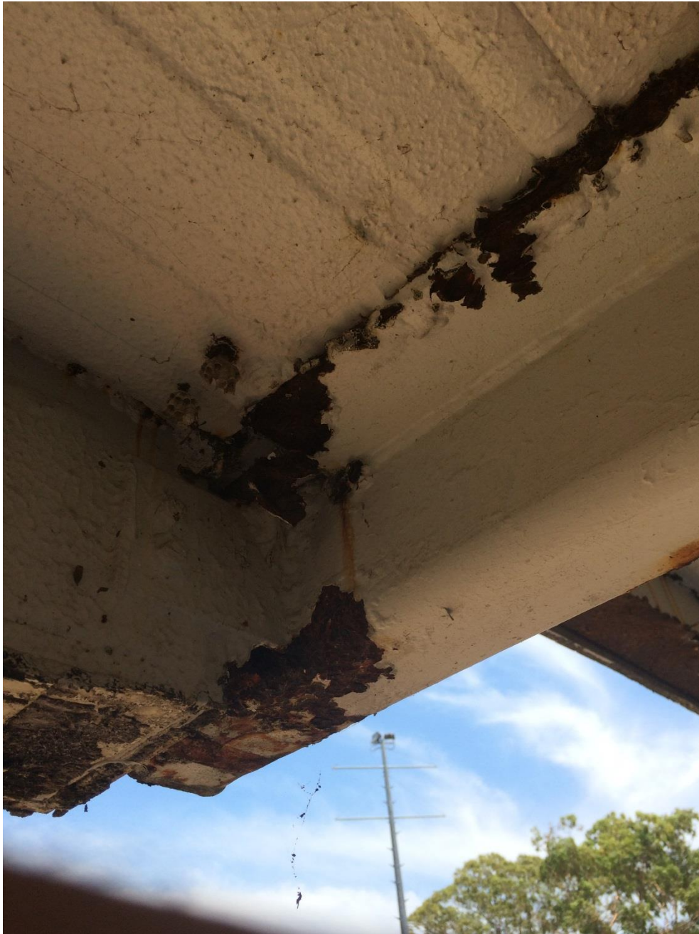
Photo 081 - Minor corrosion to truss bottom chord at the exterior face of the soundshell
