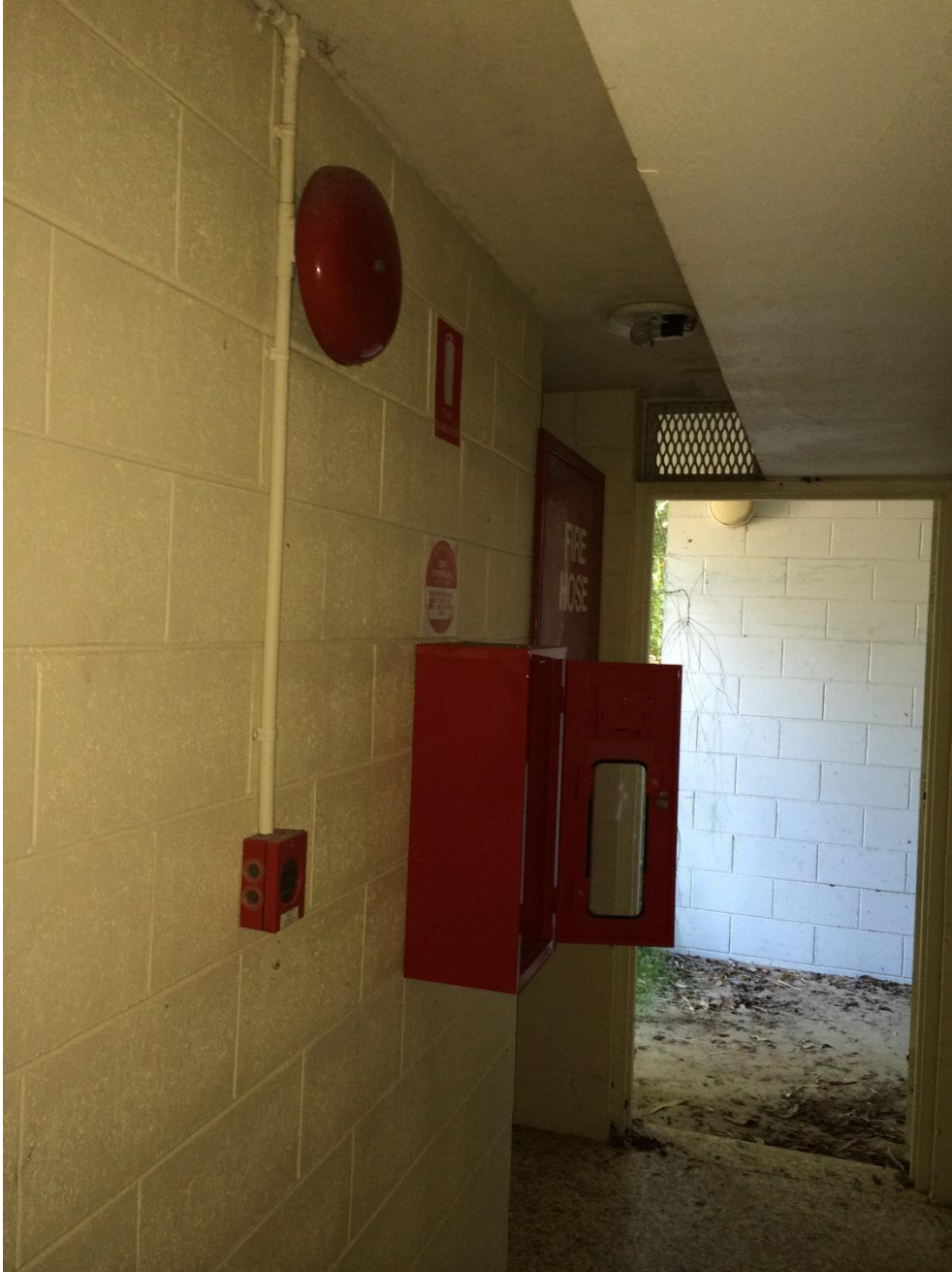
Photo 247 - Lower ground floor corridor
