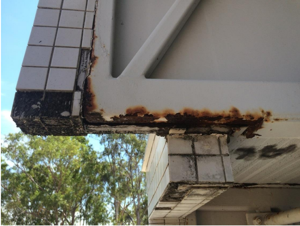
Photo 176 - Heavy corrosion to bottom chord at front face of soundshell
