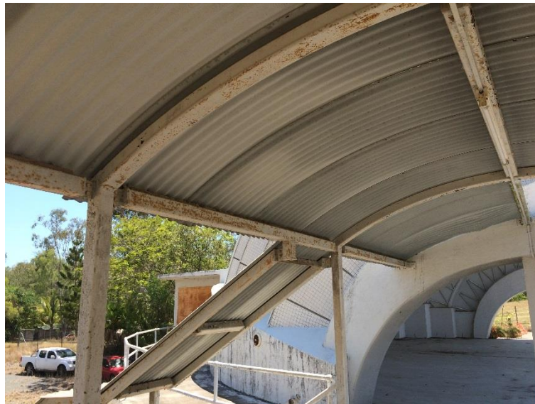
Figure 18 - Minor corrosion across covered walkway structure
