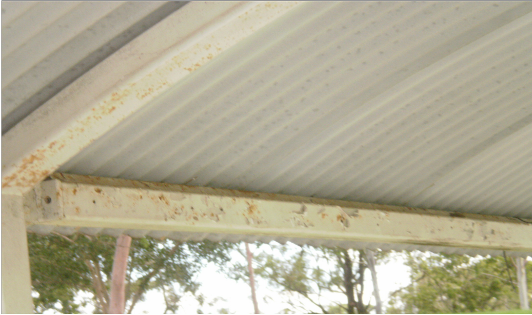
Rusted steel work on covered walk way (photo 11)
