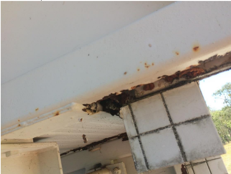
Photo 019 - Heavy corrosion to bottom chord
