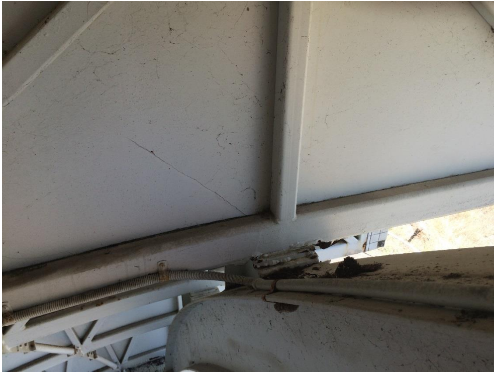
Photo 067 - Heavy corrosion to bottom plate
