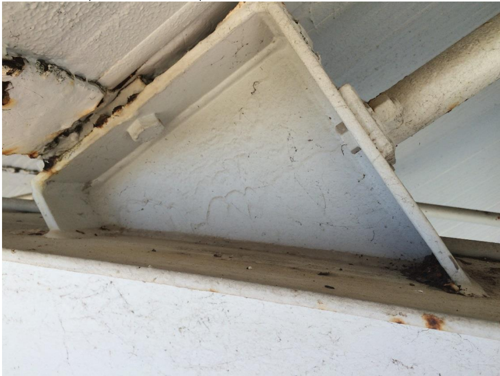
Photo 069 - Minor corrosion to stub
