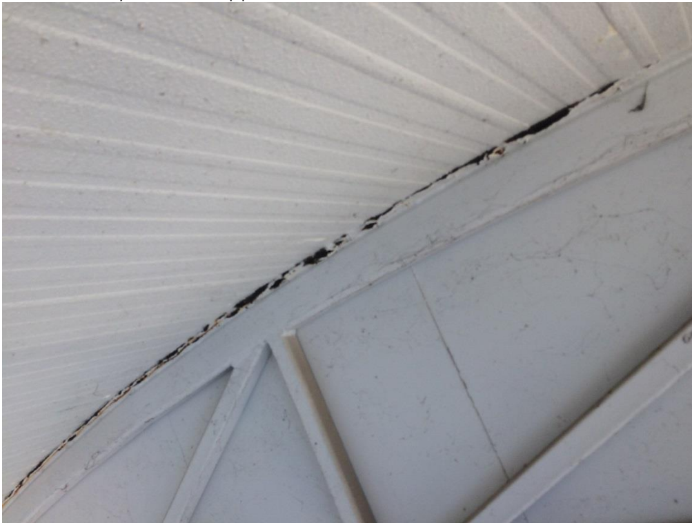
Photo 058 - Heavy corrosion to top plate
