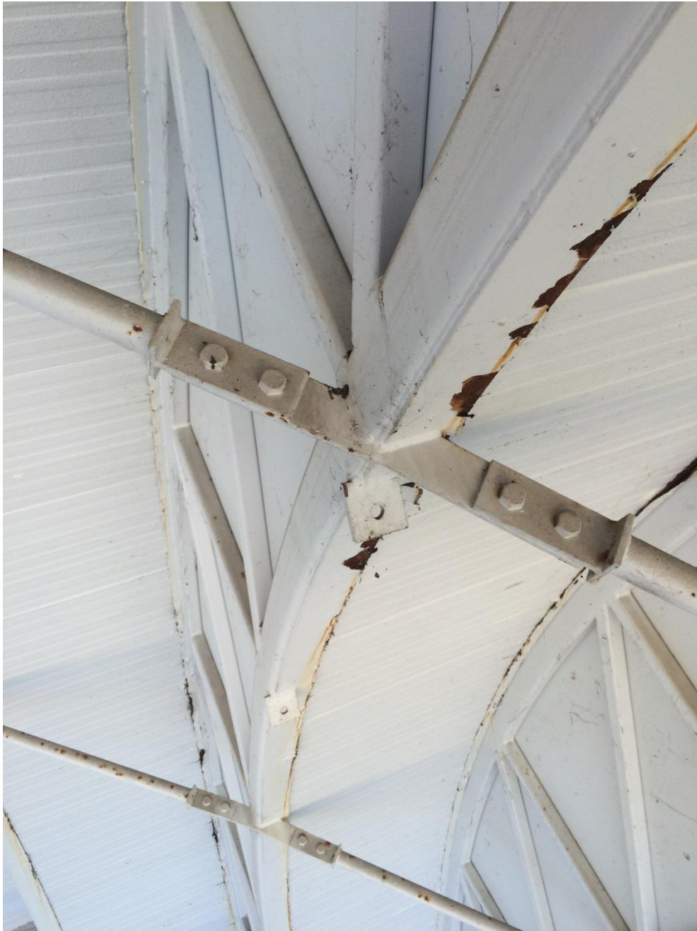
Photo 054 - Minor corrosion to bottom plate
