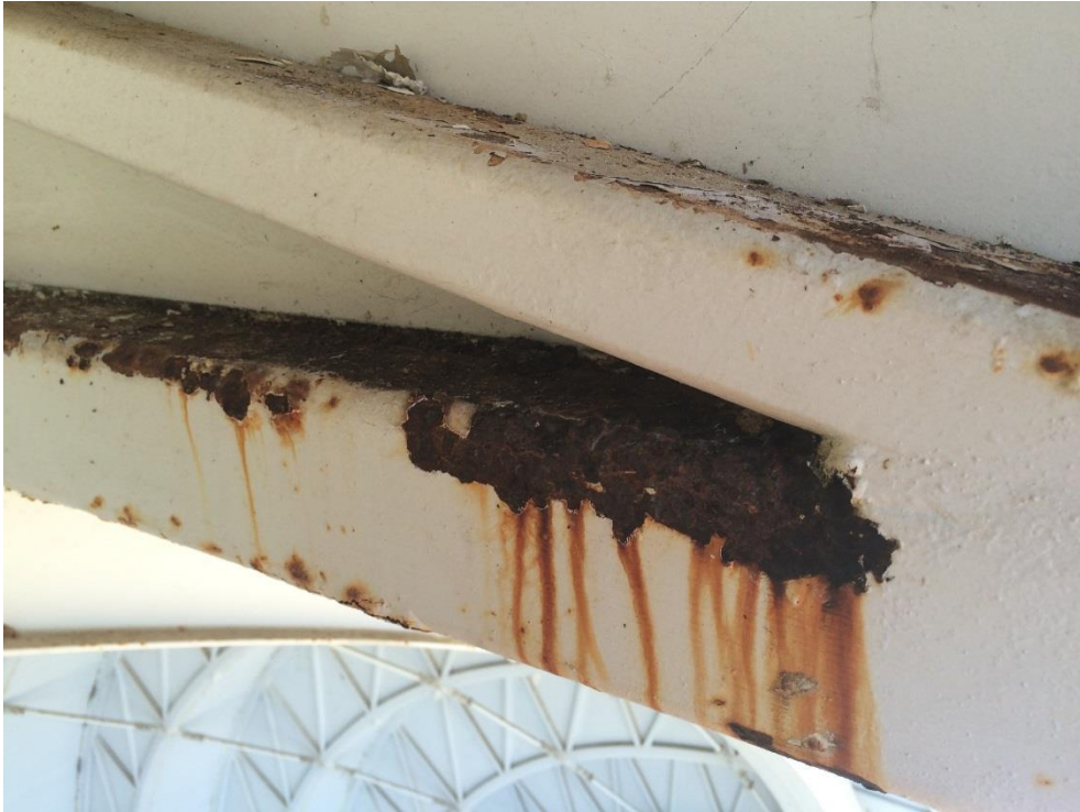
Photo 084 - Heavy corrosion to truss bottom chord at the exterior face of the soundshell
