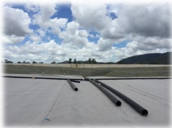
Figure 2: Leachate drainage pipes
