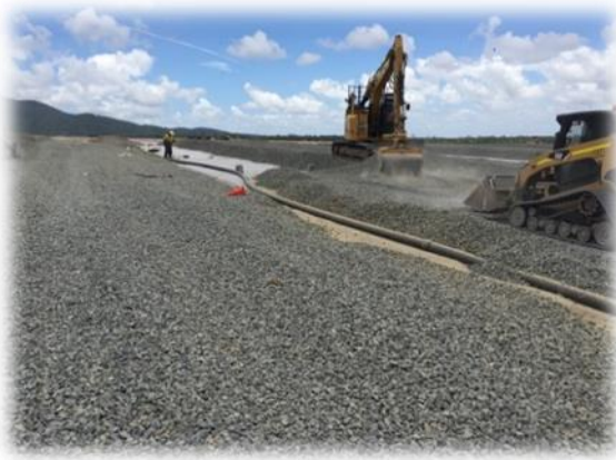
Figure 1: Leachate drainage aggregate placement
