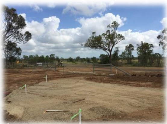
Figure 3: Main Entrance Bajool WTS
