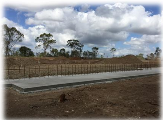
Figure 4: Retaining wall main footing Bajool WTS
