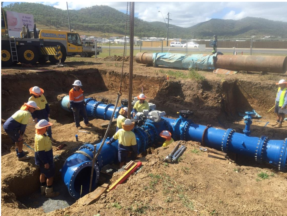
Photograph of the old section of main removed and the newly installed pipework.
