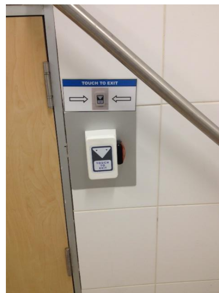
Touch switch next to pedestal
