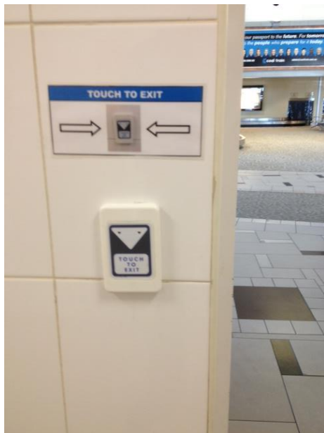
Touch switch next to door
