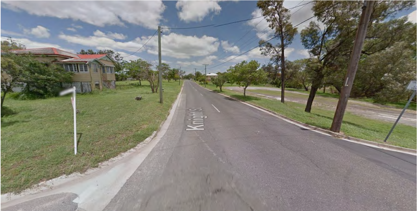
Figure 17 Knight Street looking Northbound from Park Street
