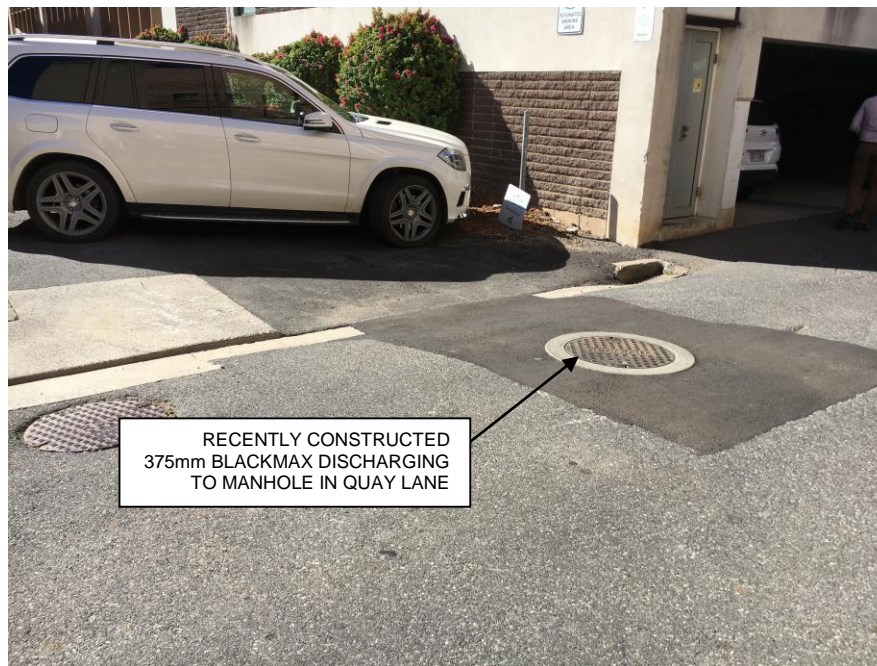
Figure 5.2 Existing 375mm BlackMAX Stormwater Connection in Quay Lane
