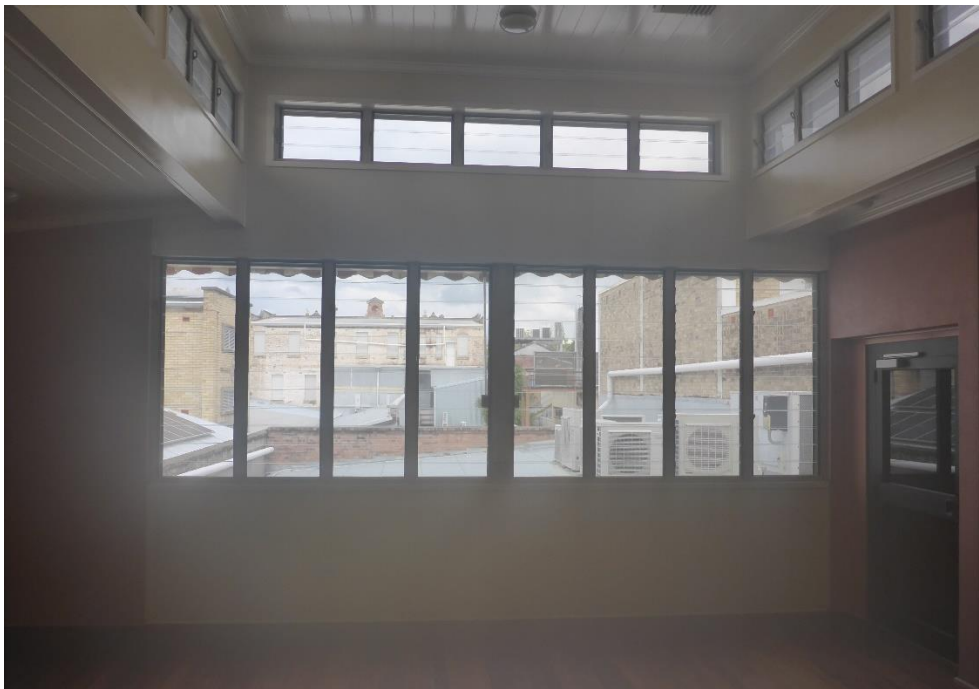
Figure 73: At the rear of the first floor level, a large open plan space - with clerestory lantern structure over – has been added beyond the rear wall alignment of the original bank building. This space also incorporates an access lift (at image right) that provides equitable access to the upper level of the building. (Source: VAULT)
