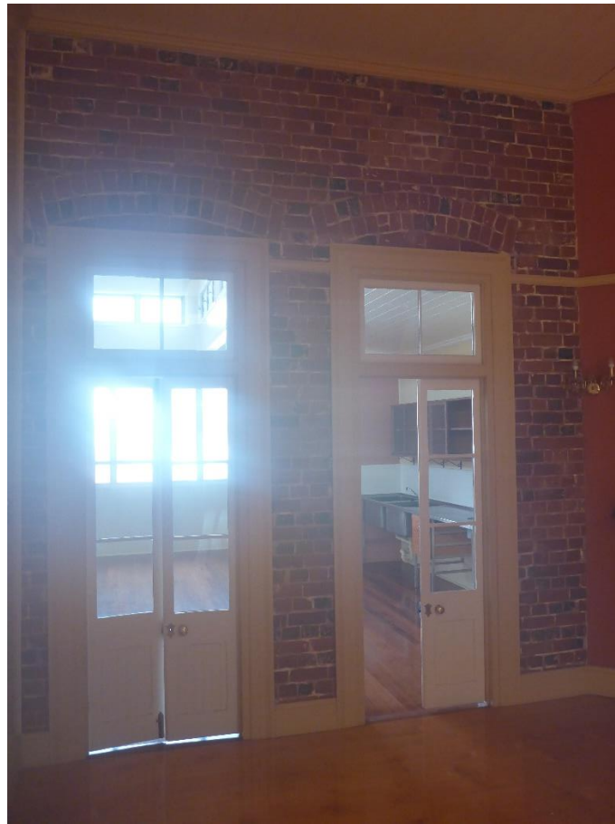
Figure 72: A more detailed view of the pair of French door assemblies extant within the rear wall of the (former) Bank building. Note the arched brick door heads that are visible above the rectangular top light panels integral to these doorways. (Source: VAULT)
