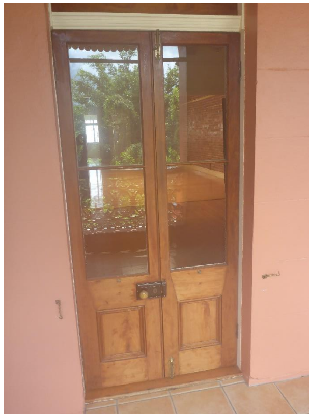
Figure 67: A more detailed view of the French doors for accessing the first floor front balcony. The form and detailing of these doors appears entirely consistent with the late-Colonial era construction of the subject heritage building. (Source: VAULT)
