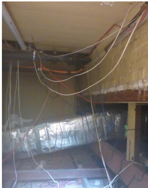
Figure 55: The view inside the ceiling cavity space extent between the original, timber VJ ceiling plane (top of image) and the more recent suspended ceiling below same. This ceiling cavity provides ample space to run the required air conditioning ductwork through the various ground level spaces. (Source: VAULT)
