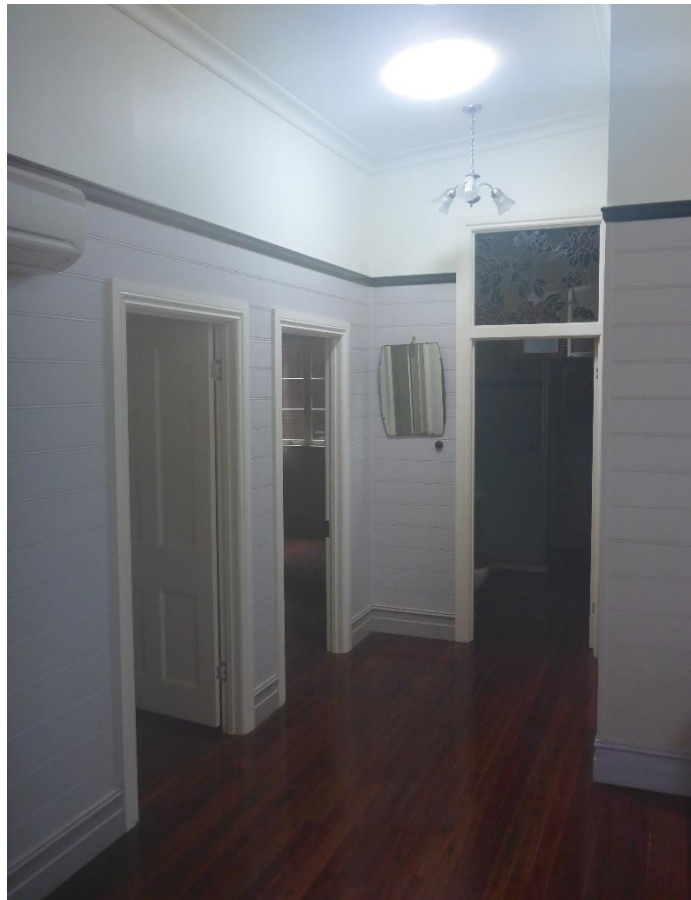
Figure 44: The interior spaces of the contemporary addition at the rear of the ground level have been finished with traditional materials and finishes (timber flooring and wall cladding) in another faux heritage configuration. (Source: VAULT)
