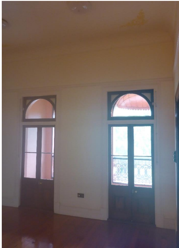
Figure 64: The open plan Living space at the front of the first floor incorporates another two sets of French doors for front balcony access. Note the consistency on the glazed / arched top light panels above these doorways. (Source: VAULT)
