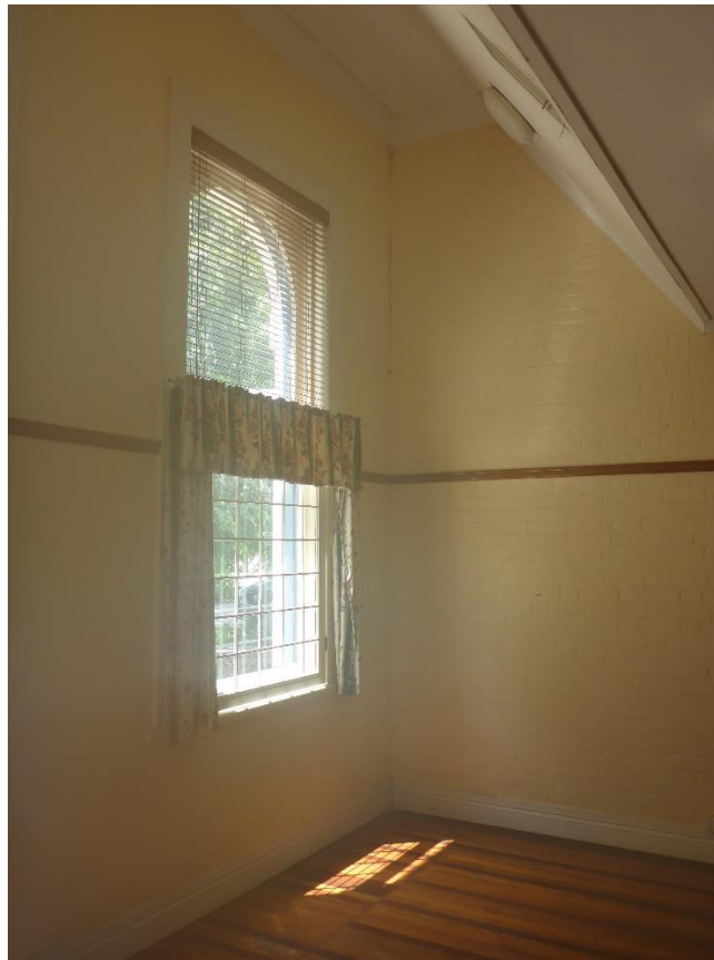
Figure 34: A wider view of the same window and the front corner of the banking chamber interior. Also shown is the transition between the original (higher) ceiling level and the lower suspended ceiling (at image top), which was installed within the banking chamber to accommodate the installation of air conditioning plant within the new ceiling space created. (Source: VAULT)
