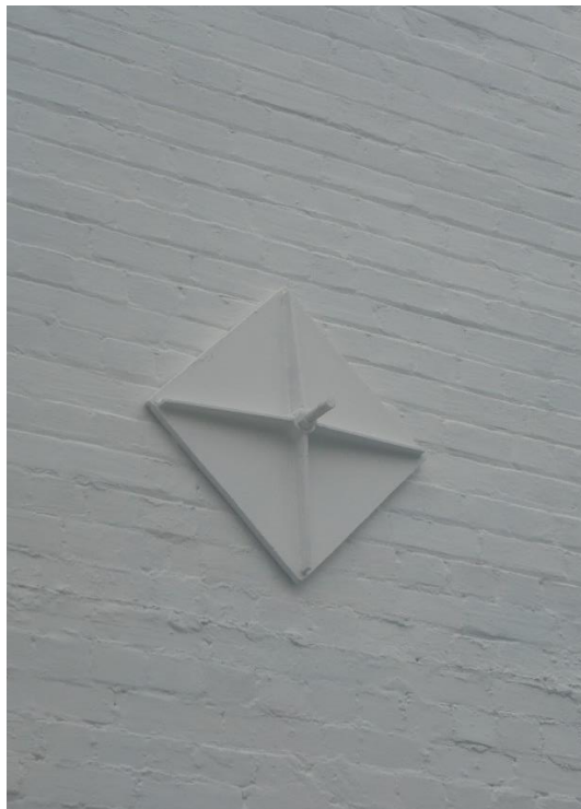
Figure 17: A more detailed view of the steel tie-rod plate set within the north-western (side) façade of the subject heritage building, which indicates prior rectification works have been undertaken to address structural stability issues. (Source: VAULT)
