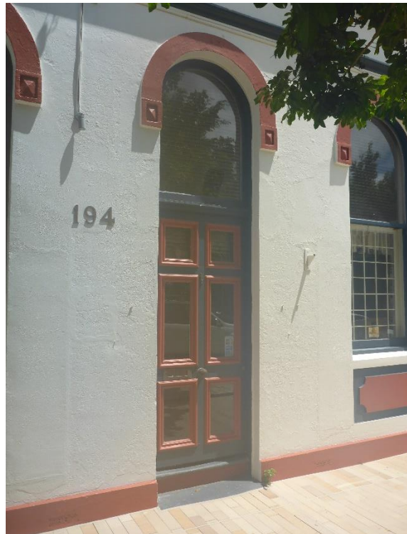
Figure 14: The adjacent entrance doorway leads into what was originally the banking chamber of the subject heritage building, which is largely the same as that shown in the preceding image apart for the glazing panels inserted into the door leaf. (Source: VAULT)
