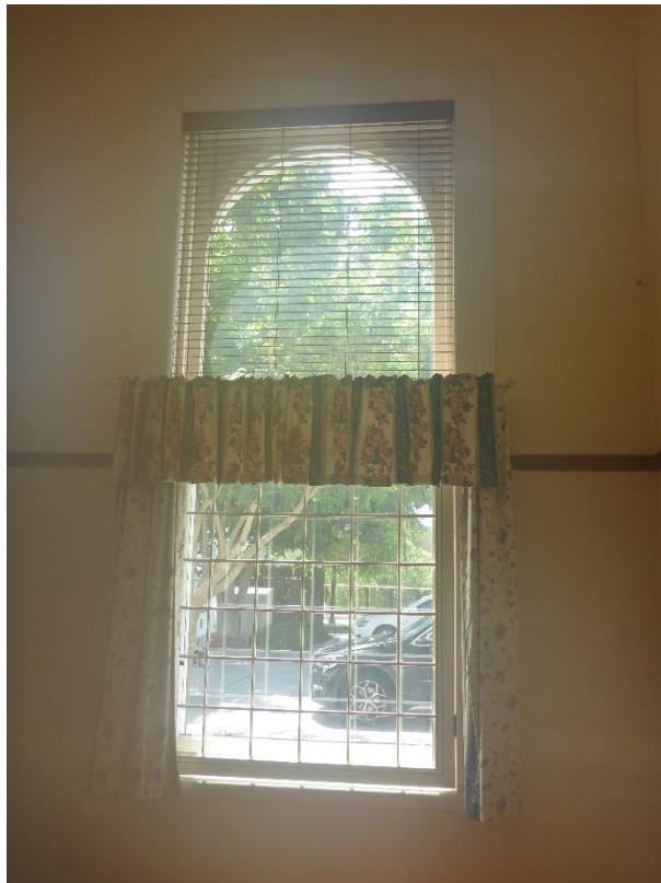
Figure 33: An interior view of the front window – as previously depicted at Figure 15 – showing the arched window head of the top sash within this double-hung window unit. (Source: VAULT)
