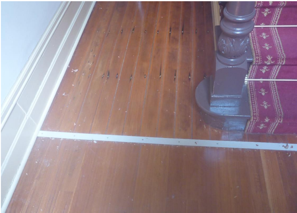
Figure 26: The timber flooring within the entrance hallway includes a more recent infill panel within the front section of the hallway (in foreground of image), which indicates a prior repair to the original flooring. (Source: VAULT)
