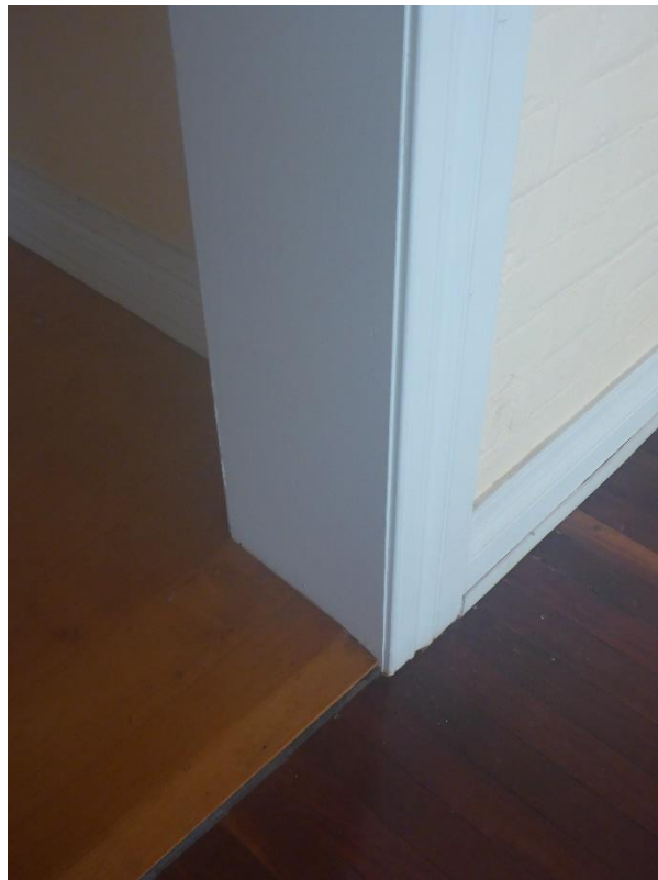
Figure 37: The junction between the original timber flooring within the banking chamber (lower right corner of image) and the pine flooring installed within the “back-of-house” spaces located behind the banking chamber (at image left). (Source: VAULT)
