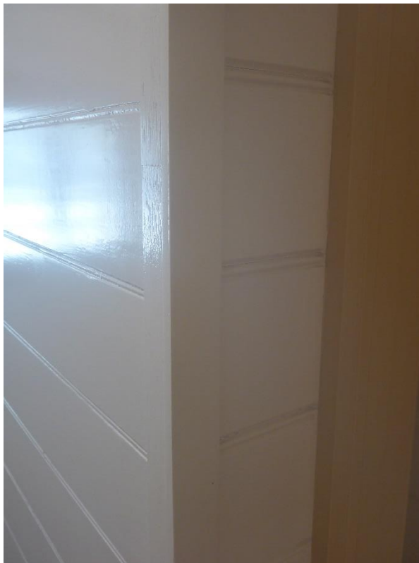
Figure 59: A close view of the corner detail where the original timber wall cladding of the stairwell (at image left) interfaces with the later additions to the rear of same. Note the differential in timber VJ profile and module between the two intersection wall planes, which is clearly evident from the misaligned board module at this corner. (Source: VAULT)
