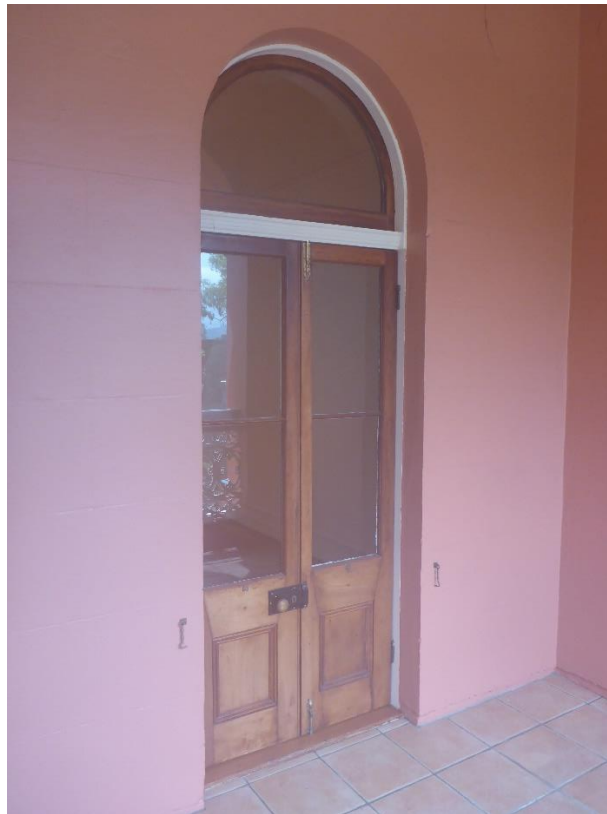
Figure 66: A detailed view of one of the French door assemblies showing the original, low-waisted door leaf and associated door furniture as well as the arched and glazed top light panel. (Source: VAULT)
