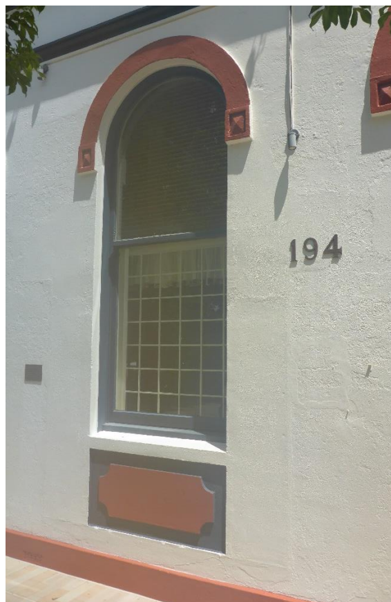
Figure 15: The Quay Street façade also incorporates an array of arched windows with equivalent proportions as the adjacent door openings and integrates a decorative spandrel panel set beneath the window sill. (Source: VAULT)
