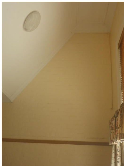
Figure 35: Another interior view of the transitional ceiling profile within the former banking chamber space. This view shows the original ceiling level within this space (at image top right) and the chamfered ceiling plane dropping back to the suspended ceiling level now extant throughout the balance of this space. (Source: VAULT)
