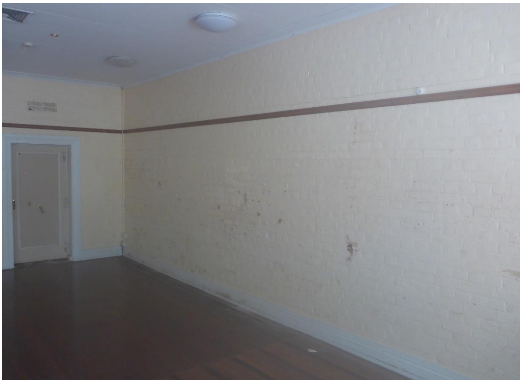
Figure 29: The interior view of the banking chamber showing the painted brickwork of the side wall of the heritage building, the steel strongroom door (at image left) and also indicating the more recent suspended ceiling within this space. (Source: VAULT)
