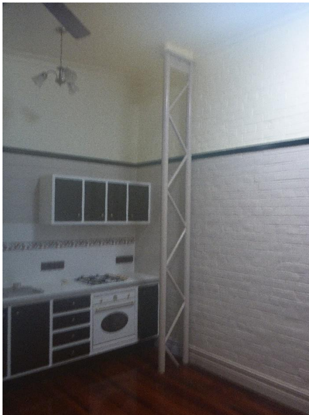
Figure 43: The upper level of the dwelling space above combines original / early painted face brickwork with a steel portal frame and contemporary kitchen fit out of this more recent building addition. (Source: VAULT)
