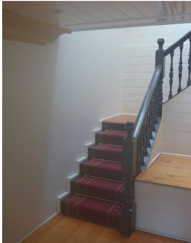
Figure 54: Within the residential entrance hall set along the side of the subject building, a mid-level landing provides access into the services space created within the cavity beneath the original ceiling plane and the more recent suspended ceiling. The upper run of the internal staircase extends from this landing level up to the residential level above. (Source: VAULT)
