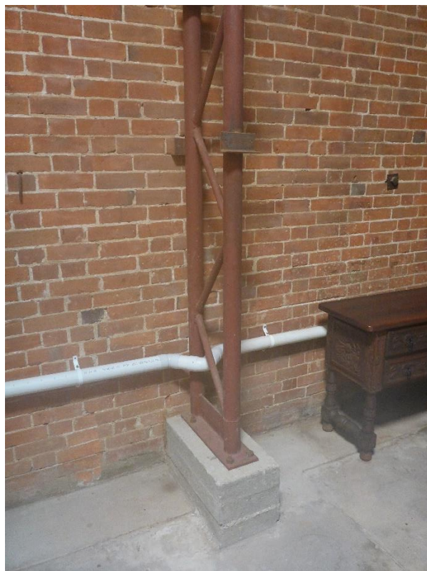
Figure 49: A detailed view of the original brickwork of the side walls at the rear of the subject site showing the Flemish bond pattern of the brick courses. Also noted is the interface between this original construction and the contemporary, steel portal frame and its elevated concrete pad footing. (Source: VAULT)
