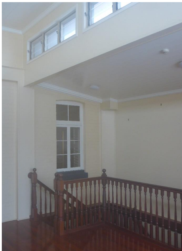
Figure 75: From within the upper level rear addition, the form and detailing of the original rear wall of the (former) Bank building is still evident; such as the window and concrete sill assembly that has been internalized by this addition. The staircase visible in this photo connects with that shown in the preceding Figures 41 & 42 (above). (Source: VAULT)
