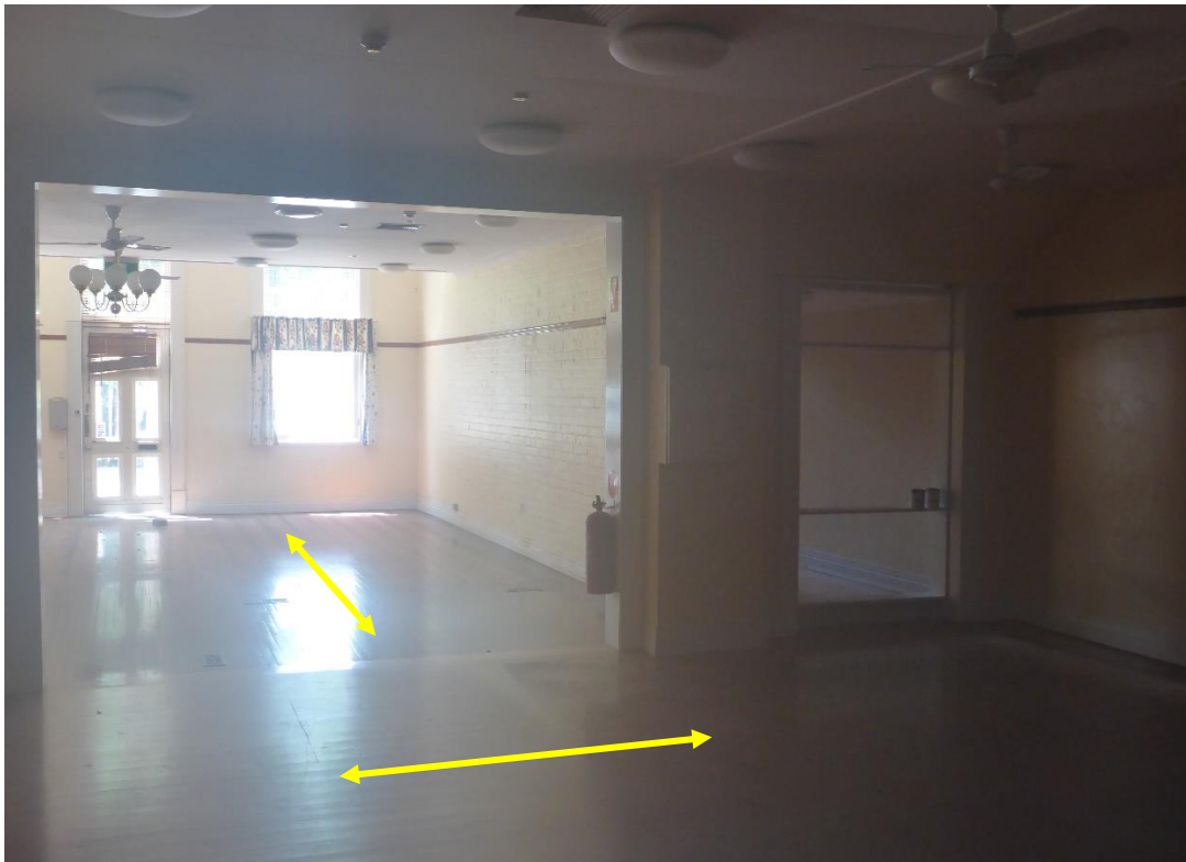
Figure 38: The view through the ground level of the subject building; as viewed from the rear / within the “back-of-house” space located behind the original banking chamber. Note the opposite direction of the flooring layout between these two spaces, which has been arrowed for clarity. The wall opening visible at image right connects through to the entrance hall shown in the preceding photos. (Source: VAULT)
