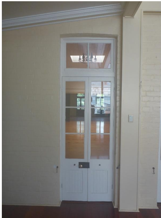
Figure 76: On the opposite side of the building, there is another example of the form and detailing of the original rear wall of the (former) Bank building still evident; in this instance showing one of the French door assemblies with arched brickwork door head over – as shown above at Figure 72. (Source: VAULT)
