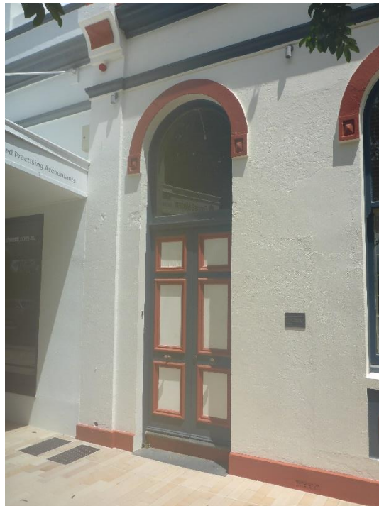
Figure 13: The secondary (residential) street entrance into the (former) Royal Bank Building , which features a glazed, arched top light panel over the solid timber, six-panel entrance door. (Source: VAULT)
