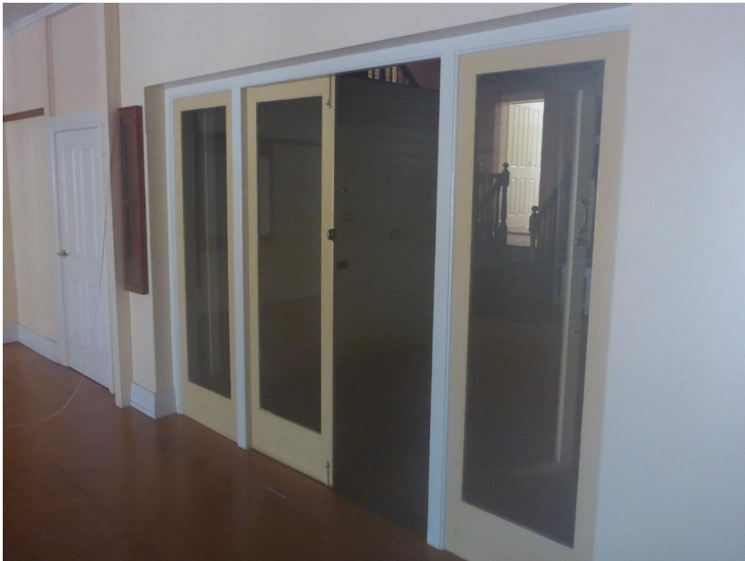
Figure 40: The original rear wall within the ground level of the former Bank building has been subsequently opened up with these contemporary windows and doors that connect through to the internal courtyard beyond. (Source: VAULT)
