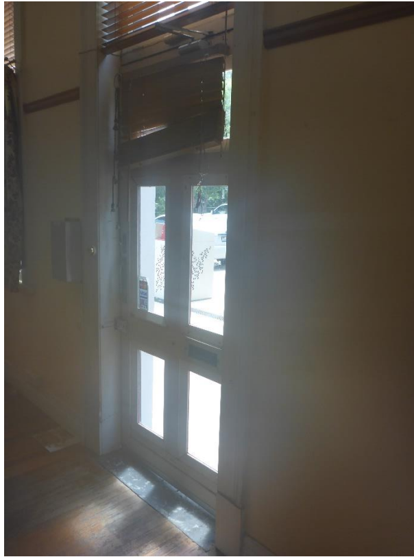
Figure 32: The interior view of the entrance door into the banking chamber, which shows the various glazing panels integrated into the entrance door leaf and the stone threshold set beneath same. (Source: VAULT)
