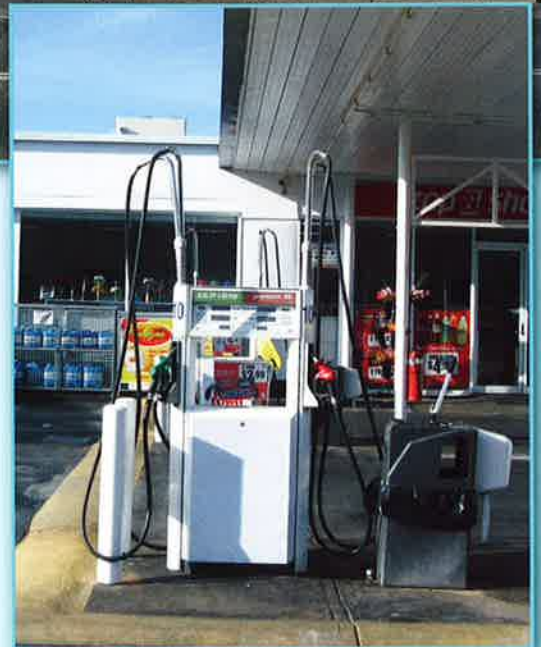
Picture shows an under-sized canopy with fuel pumps outside the canopy dripline
