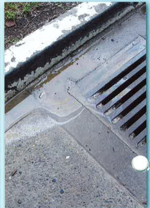
Unseemly & highly visible hydrocarbons polluting the stormwater. The concentration in the picture is in excess of 100ppm
