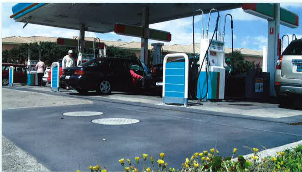
Petrol forecourt and surrounds at a busy metropolitan petrol station rendered compliant. The catchment consists of a grated drain encompassing the complete perimeter of the under-sized canopy. Surface water and forecourt runoff drains to the Puraceptor located under the two trafficable covers in the foreground.
