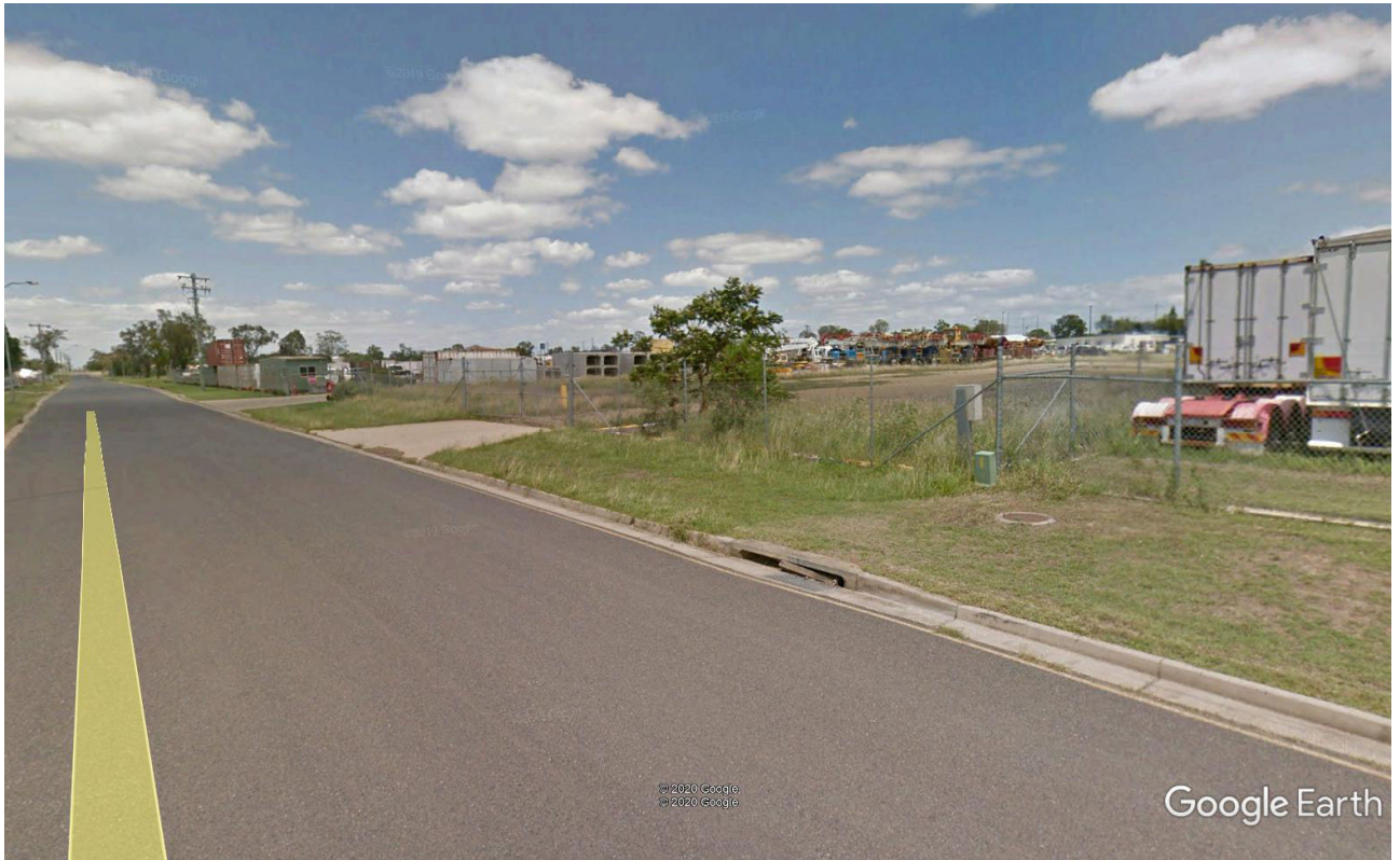
Image 1 – Foster Street showing existing gully pit in front of site (Dec 2018)
