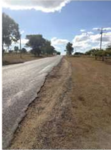
Photo 21: Edge wear at CH1350
