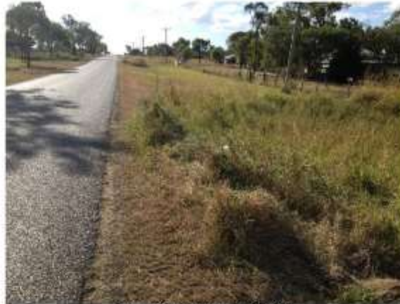
Photo 34: Culvert at CH 820
