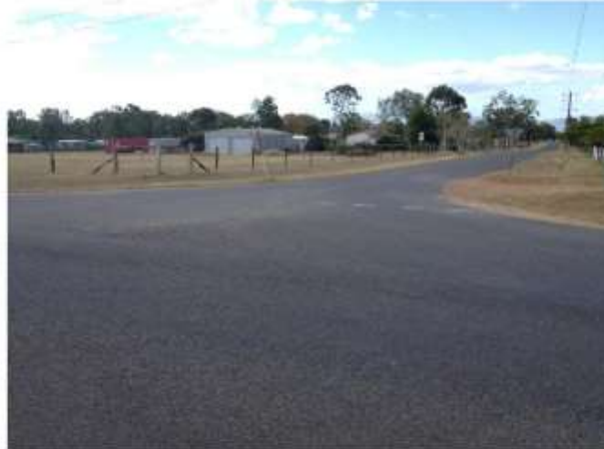
Photo 25: Existing Line Marking and loose gravel at Middle Road / Stewart Street intersection
