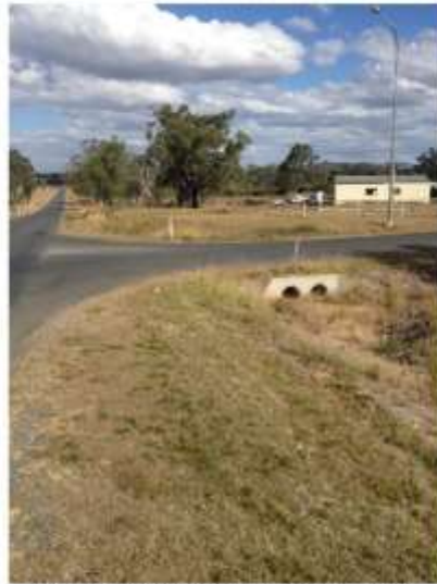
Photo 23: Culvert at Latimer Avenue.
