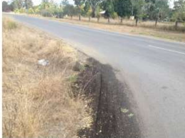
Photo 1: Macquarie Street culvert.
