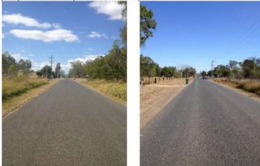
Photo 5: Middle Road (Western Approach) Photo 43: Macquarie St (Southern Approach)
