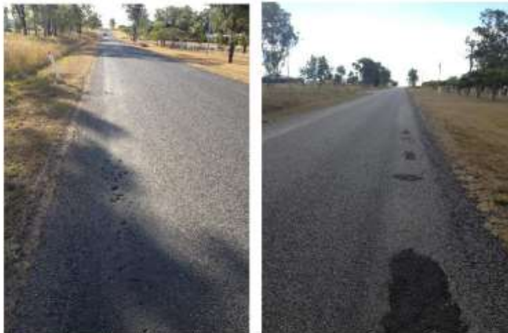
Photo 41 and Photo 18: Pavement failures along Stewart Street
