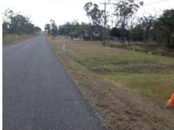
Photo 16: Culvert at CH 1681
