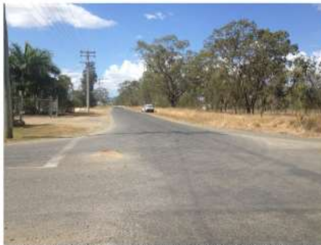
Photo 3: Existing Line Marking and loose gravel at intersection
