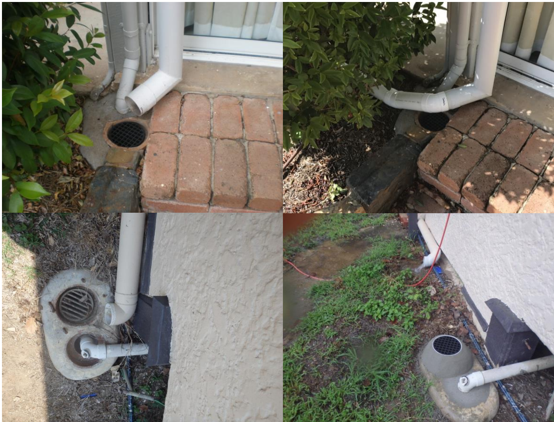
Figure 1. Examples of non-compliant plumbing (left side) identified during the inspection program and the same plumbing post-modification to prevent stormwater inflow (right side).
