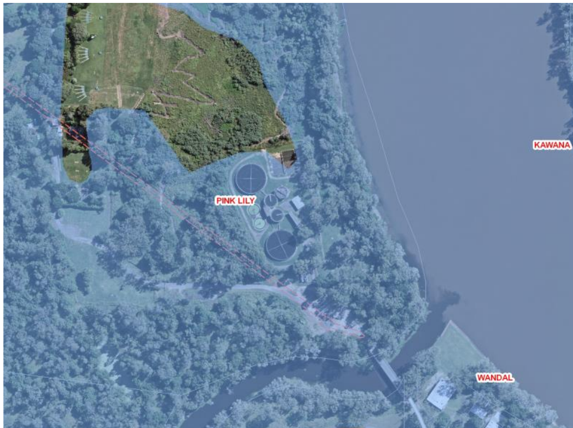
Figure 3. Aerial image showing the WRSTP surrounded by the Fitzroy River Barrage storage, Lion Creek and Harman St. The blue shading indicates the 2011 flood level and area not shown as flooding is some of the area that contains the abandoned landfill, which possibly explains why it is slightly above flood level.
