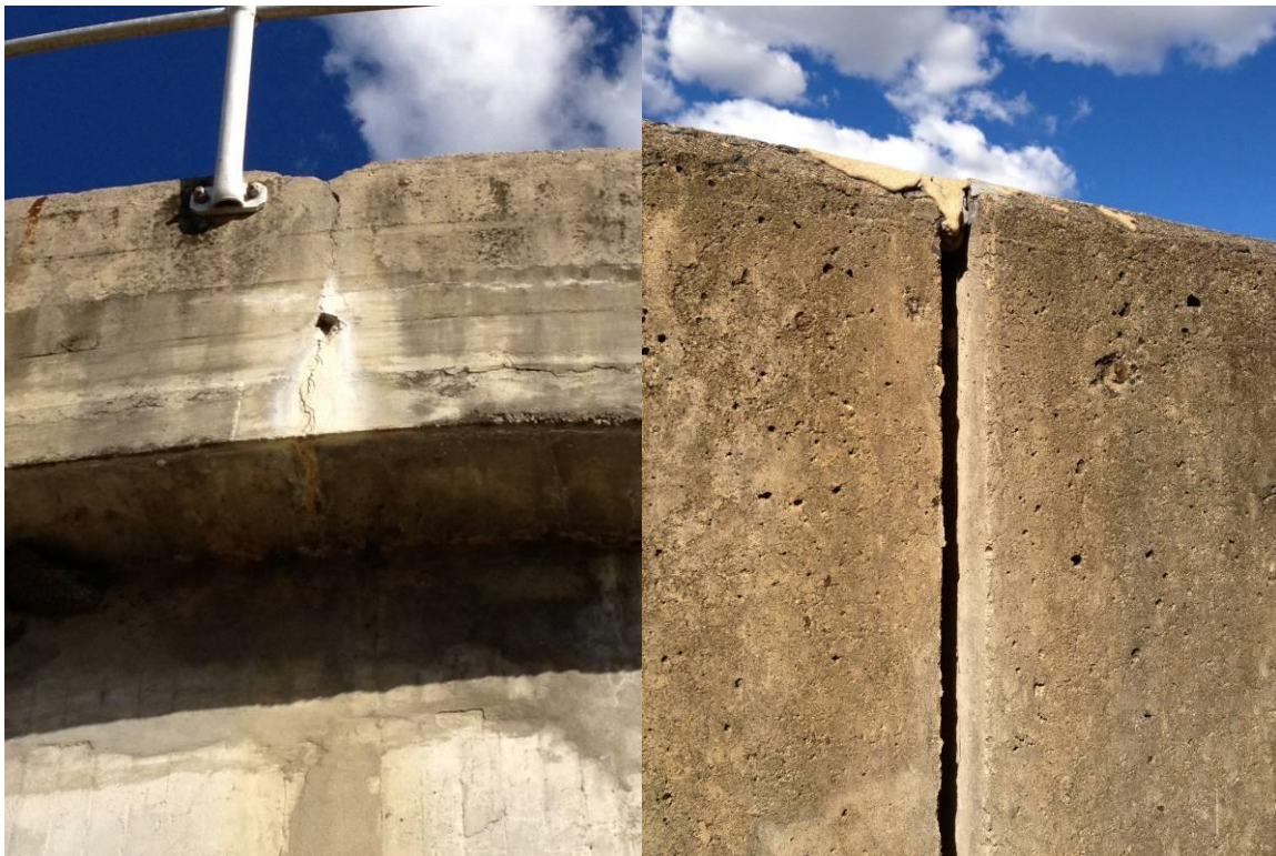
Figure 1. Photographs showing the ageing electrical switchboard (top) and the commencement of structural failure in the clarigester (bottom left) and separating wall structures of the trickling filter tank (bottom right).
